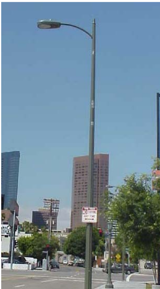
30' Electrolier with Steel Fluted Pole
