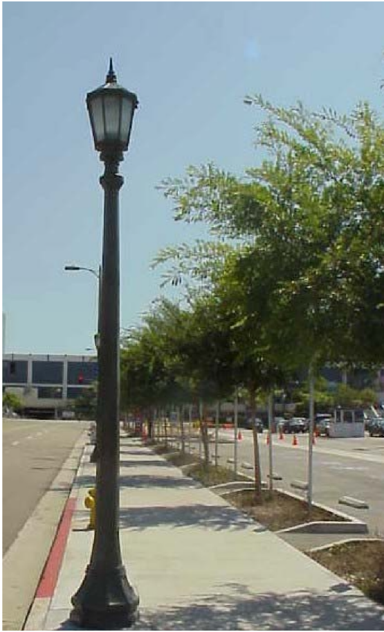
12' Octagonal Pole With Post Top Fixture
