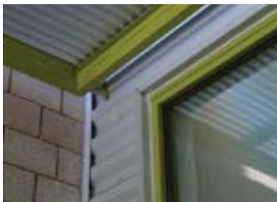
Material transitions between corrugated metal, window framing and block wall are detailed with thicknesses that add depth while accommodating movement and waterproofing tolerances (4A.G4).
