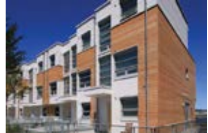
Example of concrete composite panels, which are encouraged, on a low-rise residential project (4A.G7).
