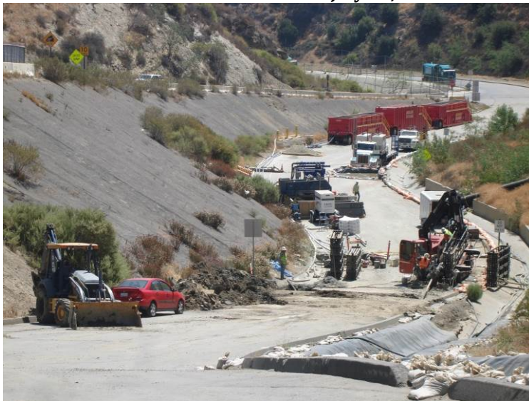
Photo 79: Underdrain Drilling: August 7, 2013
