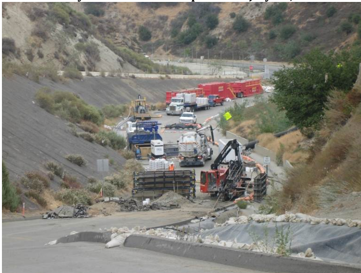
Photo 75: Underdrain Directional Drilling: July 10, 2013
