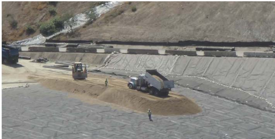
Photo 2: Thick layer under dump truck to reduce stresses on geosynthetics
