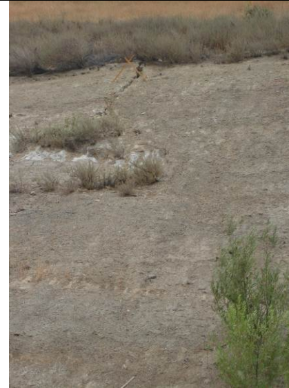
Photo 74: City South Hillside Slope Crack: July 10, 2013
