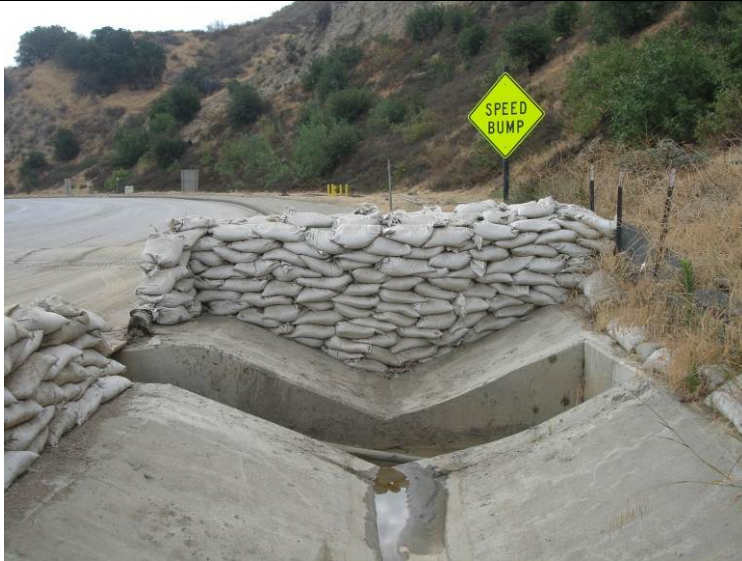
Photo 77: Underdrain Water Control: July 10, 2013
