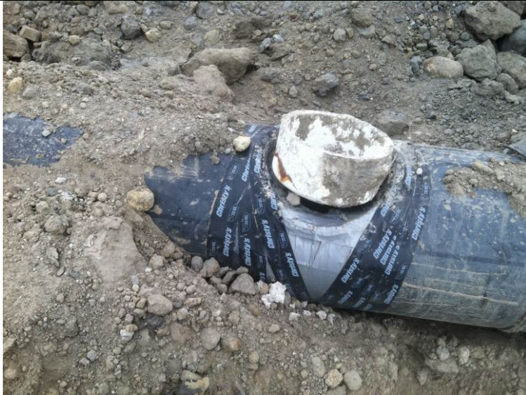
Photo 209: Head Pipeline Gas Collection Leaking: July 10, 2013
