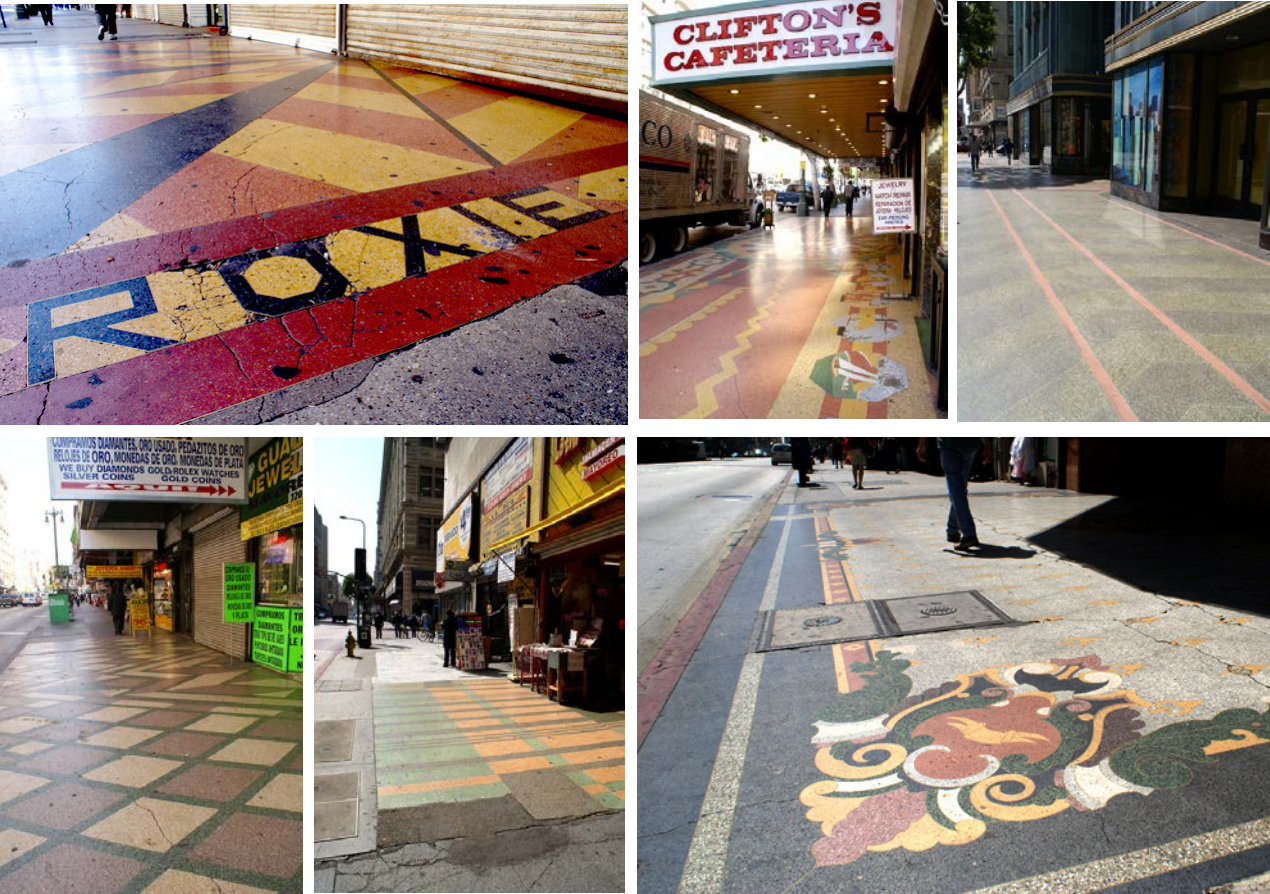
Examples of Historic Terrazzo in front of Historic Theatres and Buildings on Broadway, and in various states of disrepair. Some terrazzo serves as an entry statement, other carpets the sidewalk out to the existing curb following the building’s footprint.
