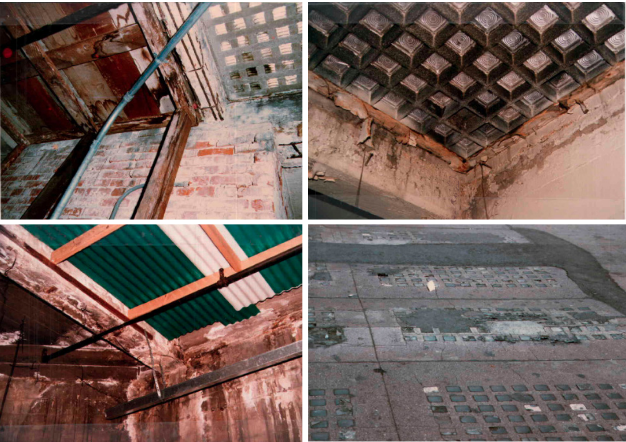
Most basements are in a serious state of deterioration, which can be seen both above and below ground.
