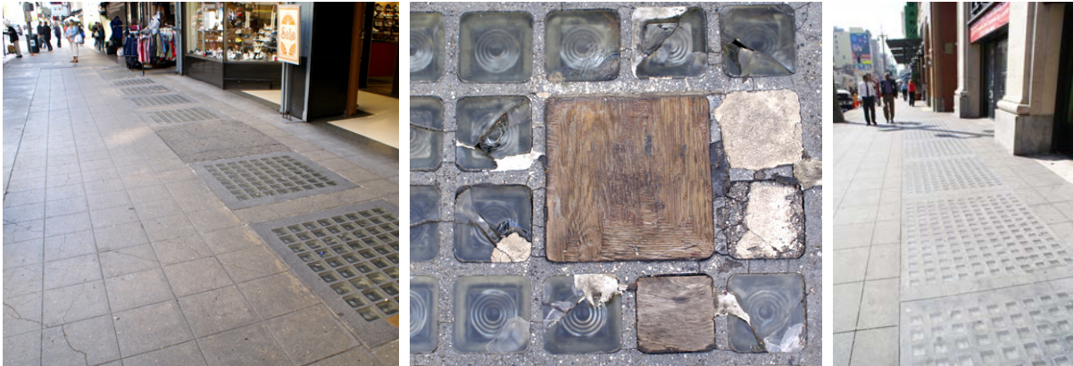
Glass Block Basement Skylights provide daytime illumination to basements below. Many are in need of critical repair and restoration.
