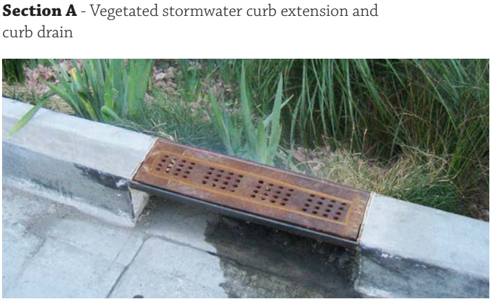
Curb drain (Condition #2) into vegetated stormwater curb extension with metal grate
