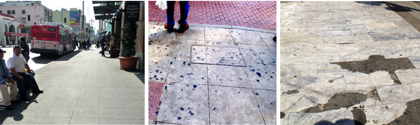
Some Sidewalk paving along Broadway has been laid in recent years, other shows its age. Other materials aside from concrete have been used, and are patched with asphalt.
