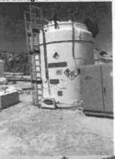
The tank is used to store bulk H<sub>2</sub>O<sub>2</sub> while the tote is used for temporary storage of the oxidant
