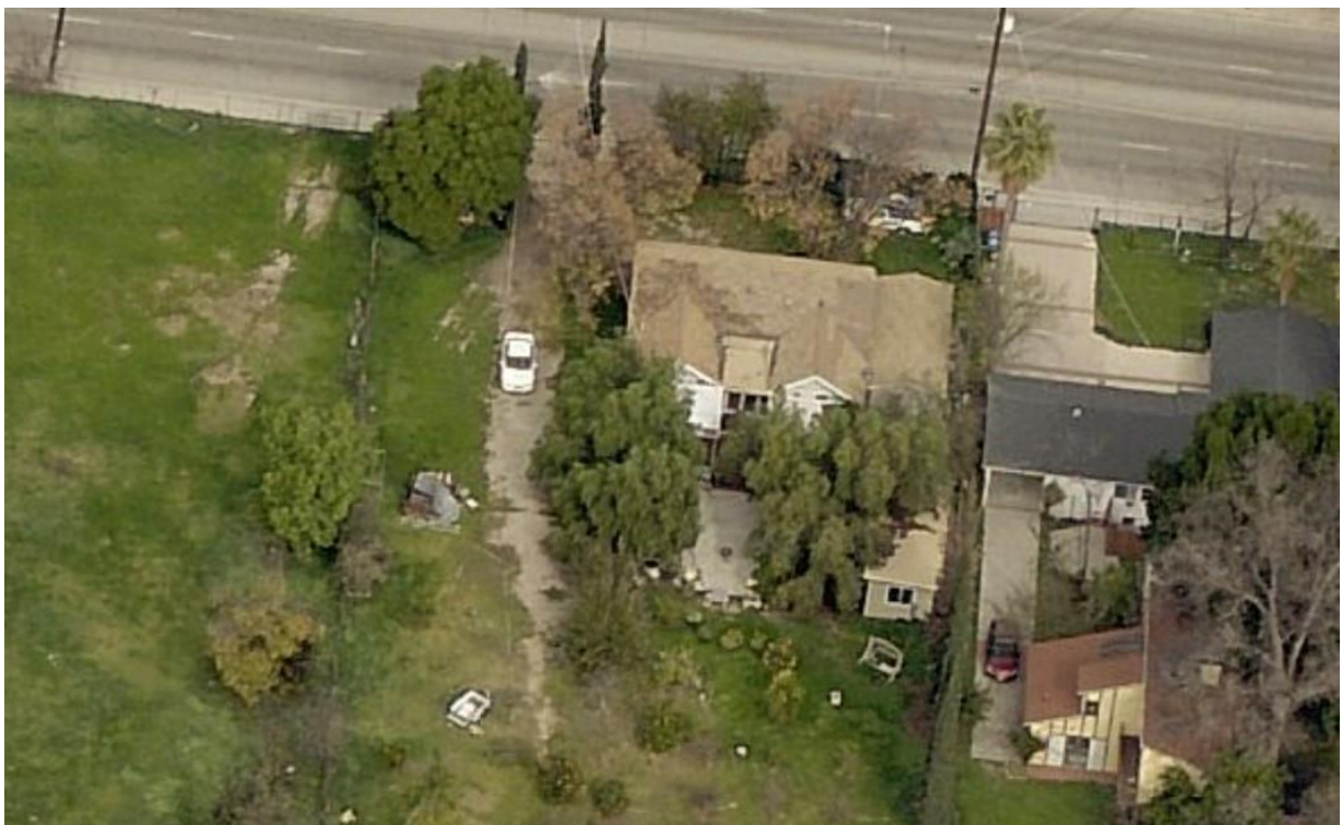
Overview of subject property's rear (south) elevation showing twin gables with infilled center, concrete patio, shade structures, and rear temporary shed structure (view to north) [Navigate LA 2020]
