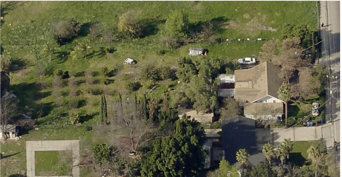
Overview of subject property's east elevation showing temporary shed blocking side of residence, temporary shed to the rear, awnings extending off the rear twin gables, and rear yard with plantings (view to west) [NavigateLA 2020].
