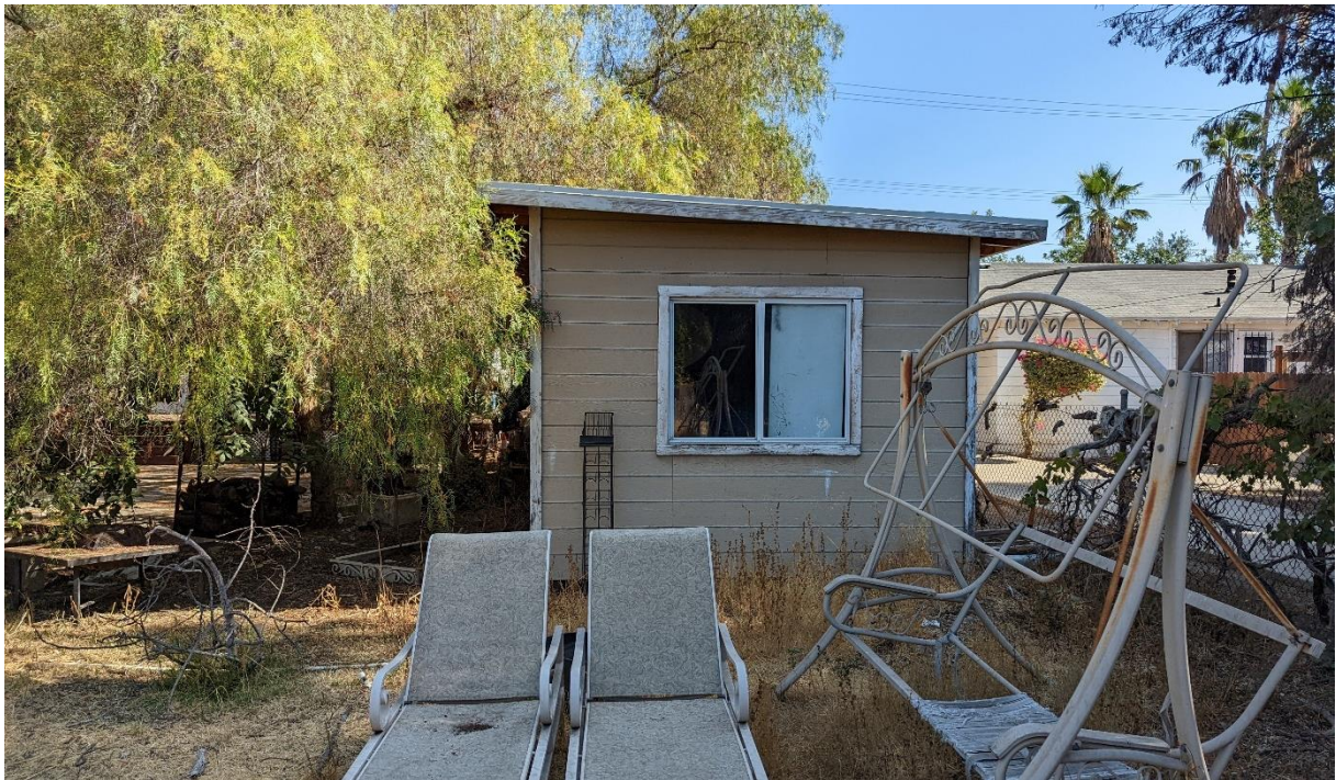
Photograph 14 Contemporary Shed Located to Rear of Subject Building
