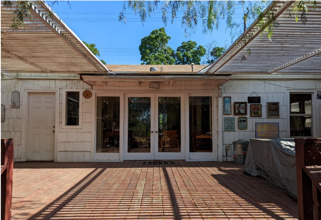
Photograph 12 Rear (South) Elevation of the Subject Building
