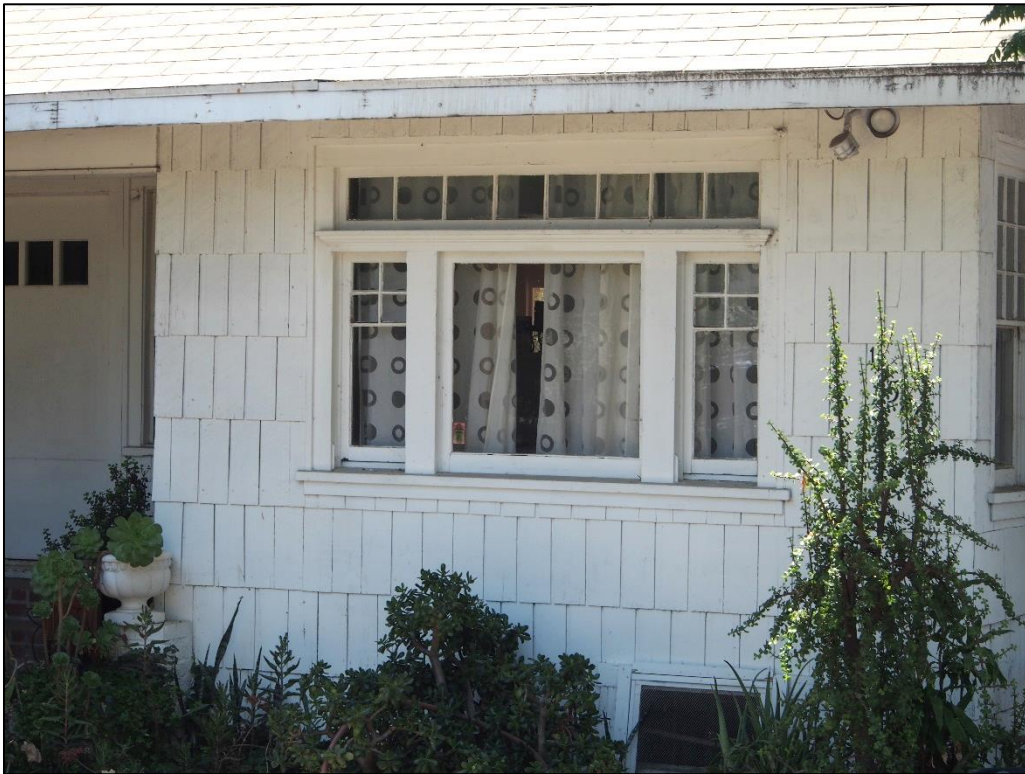
Detail of front window grouping
