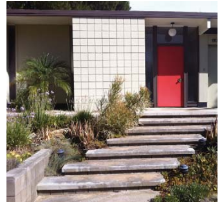
Rectilinear poured concrete steps with a modest lip are an appropriate front walk on an Eichler house
