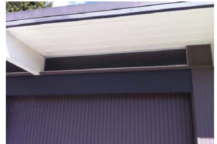
A clerestory window is shown. Such windows are indicative of the period and should always be preserved.
