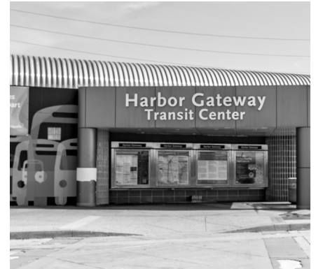
Harbor Gateway Transit Center
