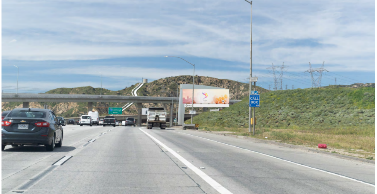
San Fernando Rd & Sepulveda Blvd (5 Freeway)
