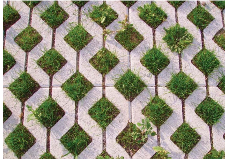
Pervious paving can be utilized along sidewalks, parking, sidewalk planting, and/or bikeways. More than just contributing to sustainability, these techniques aid in placemaking, help slow traffic in high pedestrian traffic areas, and contribute to a more pedestrian-scaled environment.
