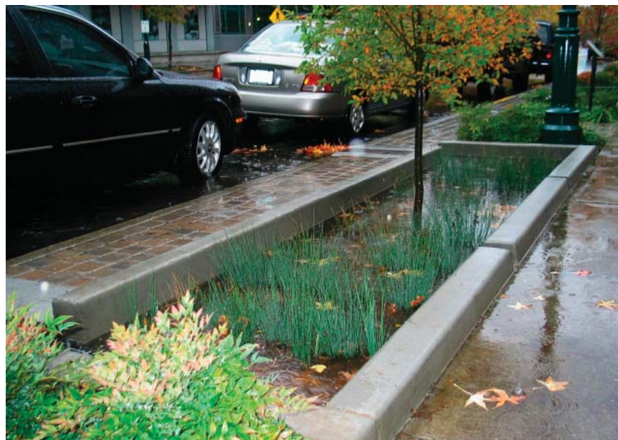
The use of bio-swales, appropriately located curb breaks, roof gutter diversions and other low-impact design (LID) “green infrastructure” techniques are all encouraged.
