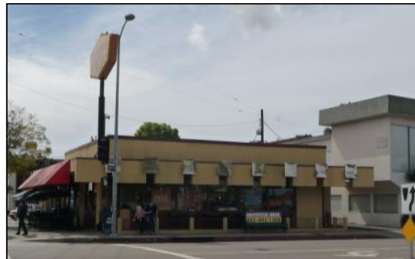
Address: 5700 W. Manchester Ave. Name: Denny's Architect: Armet and Davis Date: 1959
