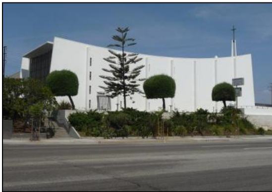
Address: 7831 Sepulveda Blvd. Name: Westchester Lutheran Church Architect: Orr, Strange, Inslee and Senefeld Date: 1964
