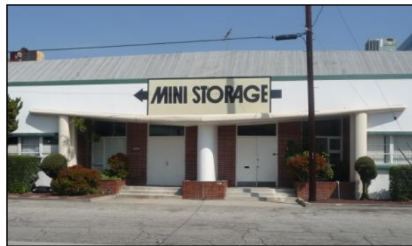
District: Airport Industrial Tract Historic District Address: 5221 W. 102 nd St. Architect: S. Charles Lee Date: 1953
