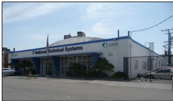
District: Airport Industrial Tract Historic District Address: 5320 W. 104 th St. Architect: S. Charles Lee Date: 1950
