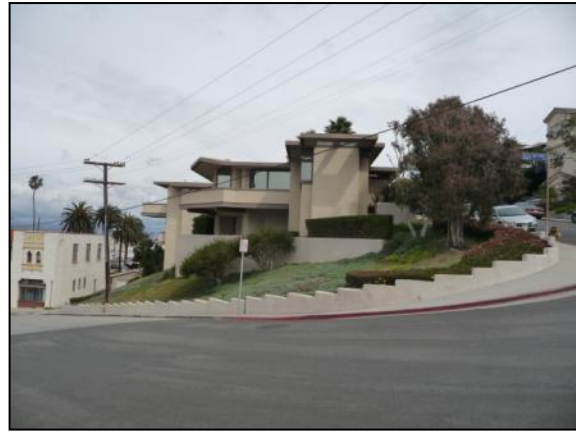
Address: 209 E. Montreal St. Name: N/A Architect: Unknown Date: 1959
