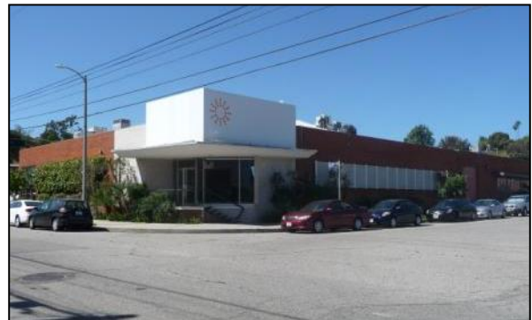
District: Arizona Circle Industrial Historic District Address: 6300 W. Arizona Circle Architect: Unknown Date: 1959
