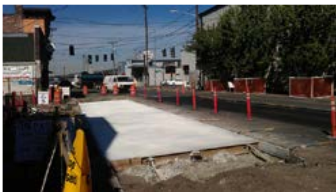
A concrete bus pad under construction
