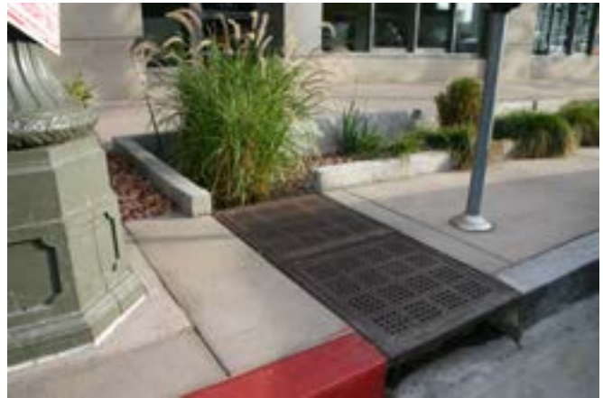
(Above and below) On Hope Street in downtown Los Angeles, several infiltration planters capture stormwater runoff through curb cuts. Stormwater enters the facility, is temporarily detained, and is treated as it slowly infiltrates natural soils.
