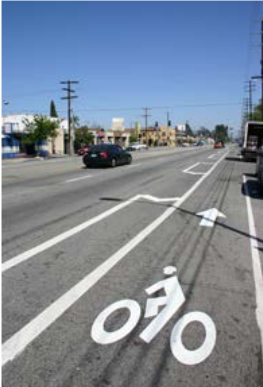
Painted striping provides a spatial buffer from passing vehicles, providing protection from fast-moving vehicles. Note that, in this case, there is insufficient space to also incorporate a buffer in the “door zone” next to parked vehicles.
