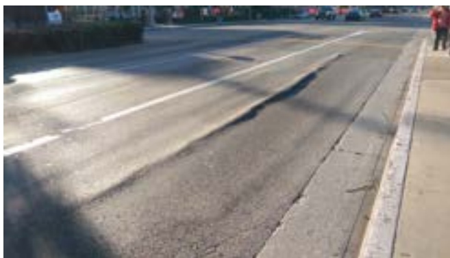
Where no bus pad exists, the weight of heavy vehicles causes rippling and cracking of the asphalt surface.
