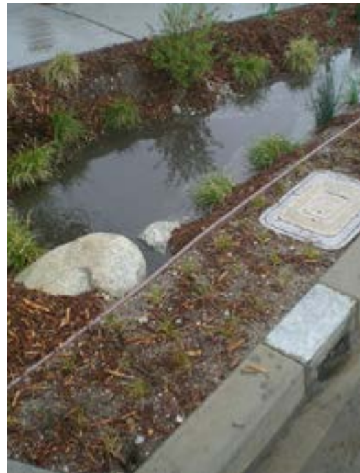
When the bioswale has reached full retention capacity, excess water can leave the facility through small curb openings.
