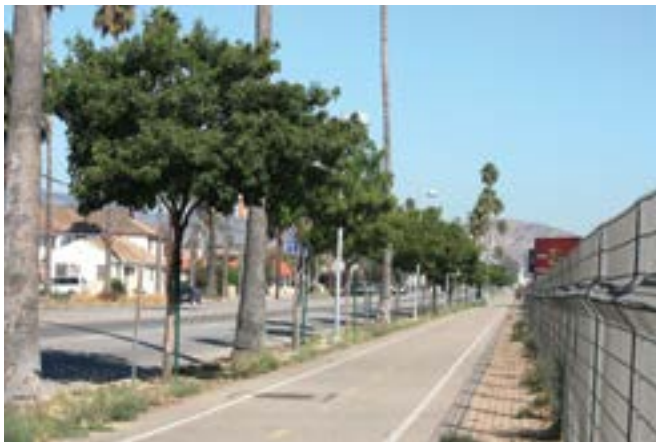
A bicycle path next to a roadway should include physical barriers to prevent bicyclists from encroaching on highway traffic.
