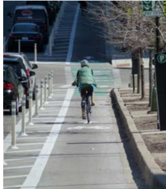
Painted buffers and soft-hit posts (as seen here in Chicago, Illinois) are inexpensive interim treatments to establish protected bicycle lanes before more-costly permanent facilities can be constructed.
