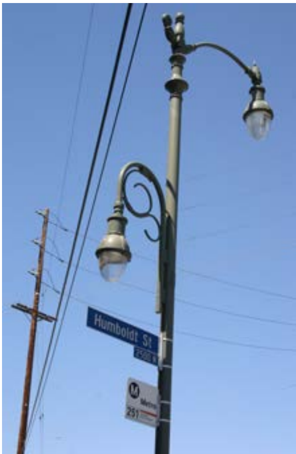
A pedestrian-oriented light fixture can share a single pole with a roadway light fixture. In some instances, new pedestrian-oriented lighting fixtures can be affixed to existing roadway light poles.
