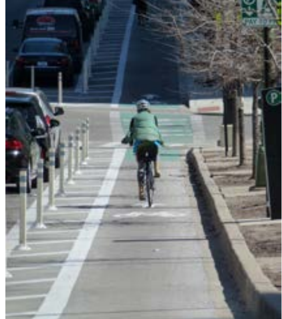
Painted buffers and soft-hit posts (as seen here in Chicago, Illinois) are inexpensive interim treatments to establish protected bicycle lanes before more-costly permanent facilities can be constructed.
