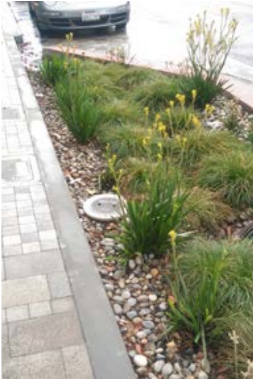
An example of an infiltration planter within a curb extension
