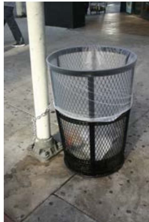
Wire basket waste receptacles are unattractive and its contents are open to the effects of wind.
