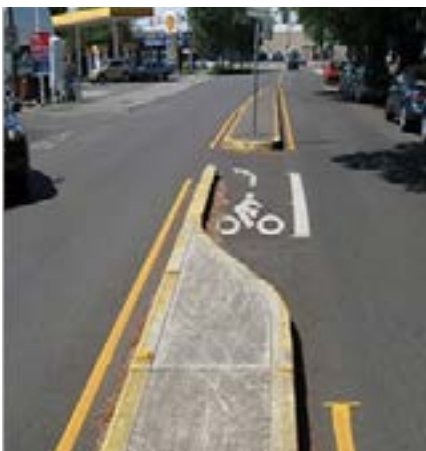
A bicycle-only Left Turn Pocket grants bicyclists exclusive left-turn access from the center turn lane.
