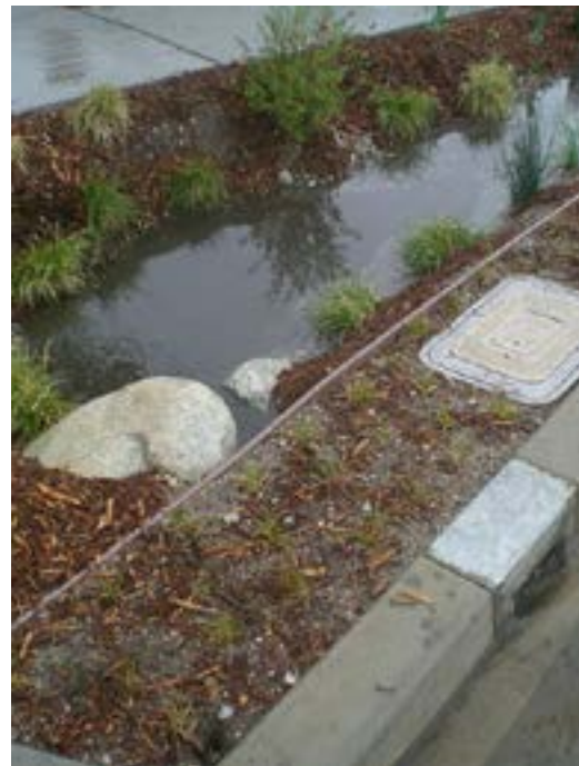
When the bioswale has reached full retention capacity, excess water can leave the facility through small curb openings.
