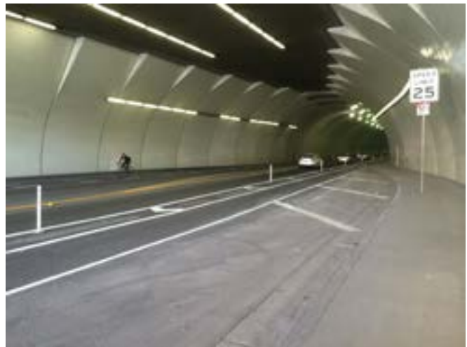
A buffered bicycle lane on 2nd Street in downtown Los Angeles provides separation and protection from vehicular traffic.
