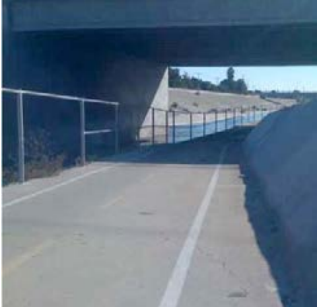
When a bicycle path follows a low-lying flood control channel, an undercrossing is often necessary.
