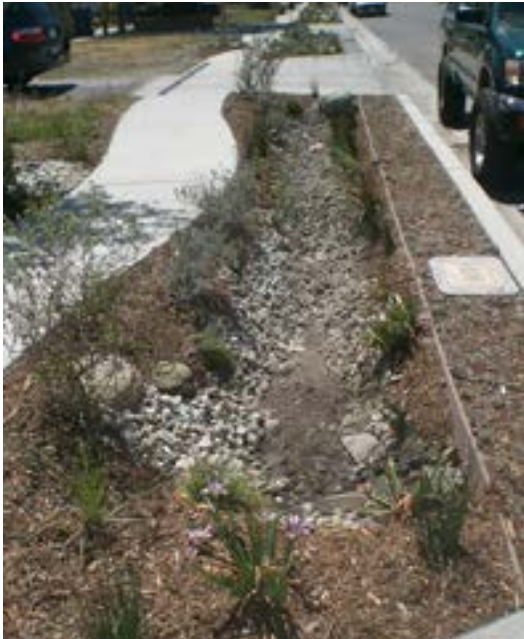
A bioswale on Elmer Avenue in Los Angeles during a dry period.
