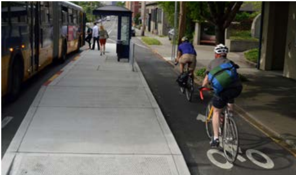
A median boarding island ensures access while allowing a protected cycle track to continue along an existing curbline. In this instance, the boarding island is accessed via a curb ramp (somewhat visible in the foreground) that adjoins the crosswalk.
