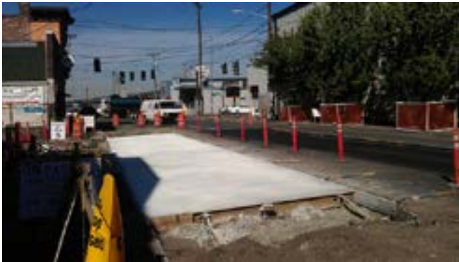
A concrete bus pad under construction
