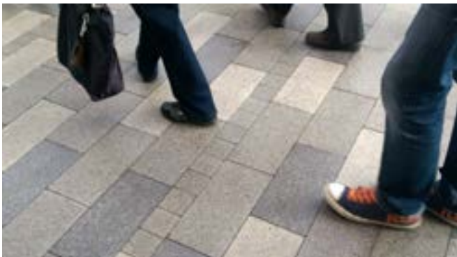
An example of permeable paving. Rainwater drains through gaps between the pavement stones.
