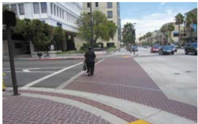
A bidirectional curb ramp (in yellow at the base of the image) orients users to the center of the intersection, requiring users to re-orient themselves toward the actual desired direction of travel.
