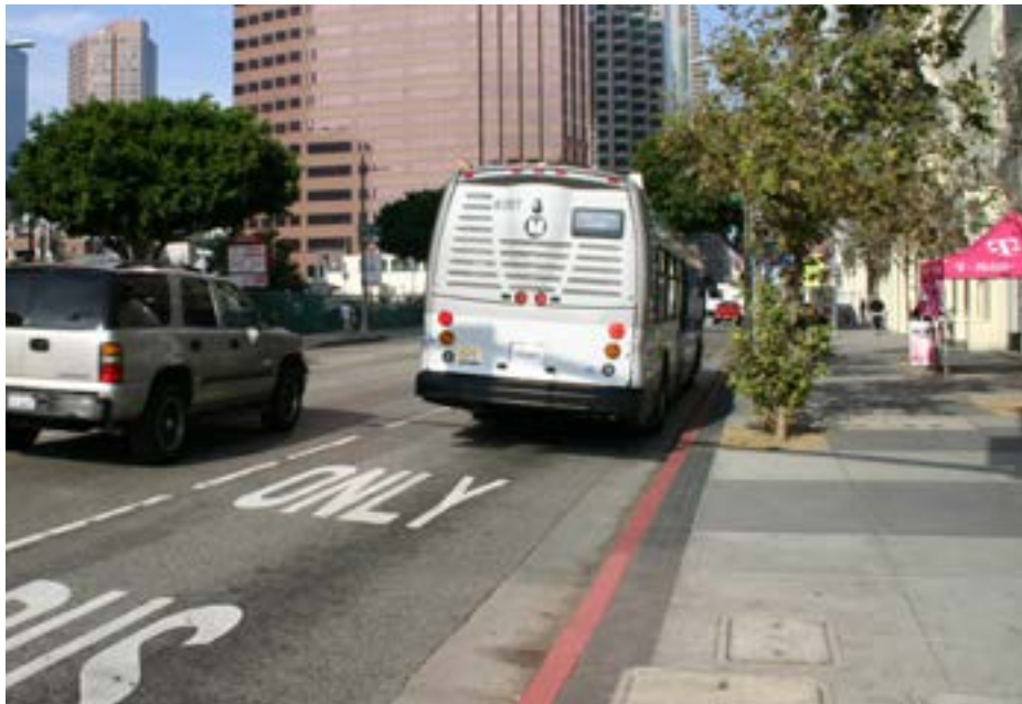
Red paint on the curb emphasizes the lane's exclusive dedication to bus use.
