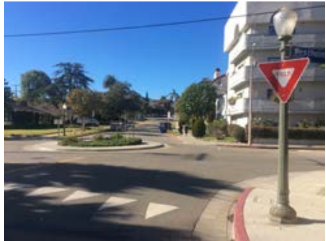
Signs at a Roundabout entrance instruct incoming traffic to yield.
