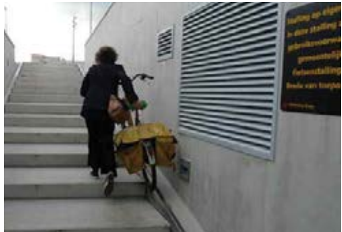
Bicycle Channel Ramps can allow bicyclists to travel more easily up and down stairways.
