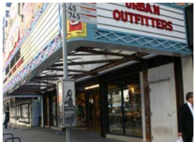
Marquees and entrance canopies mark important entries and can contribute to a vibrant, enjoyable street environment.
