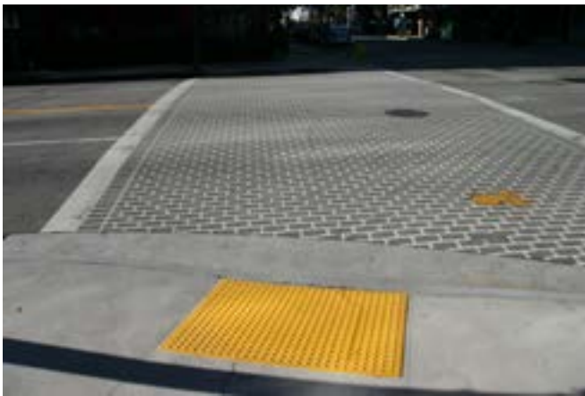
A unidirectional ramp leads directly to the crosswalk in the desired direction of travel.
