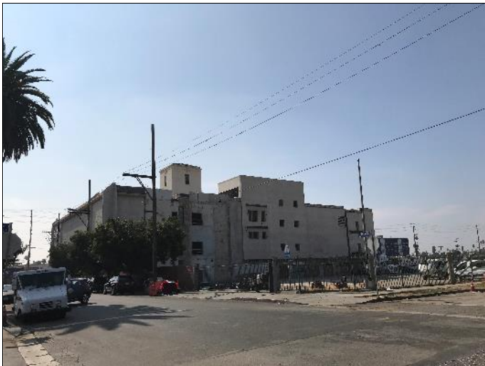
15. View looking at the subject property from off-site to the northeast
