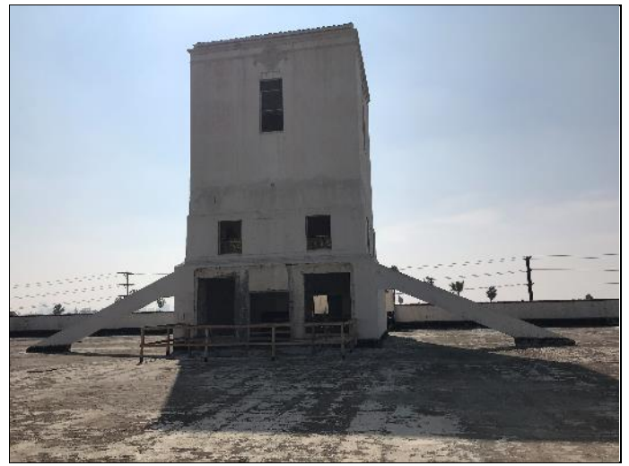
20. View of the rooftop mechanical penthouse
