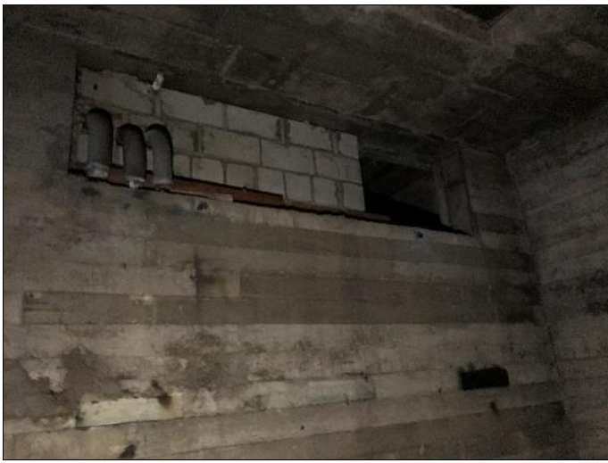
19. View of a former equipment room in the basement level
