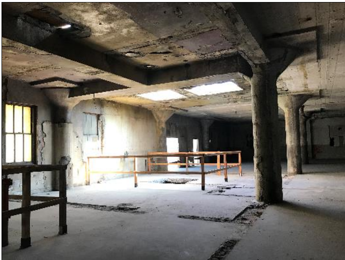
21. View of the interior of the subject property building – Second Floor
