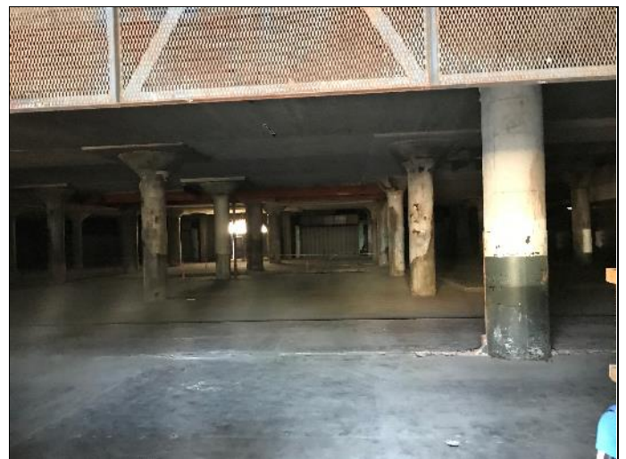
18. View of the interior of the subject property building – 1 st Floor
