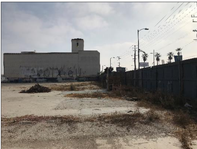
9. View east along the southern boundary with the subject building in the background
