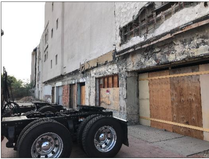
7. View of boarded entrances to the building on the northern side
