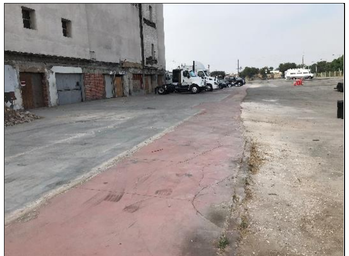
4. View across former building pads on the northern side of the subject building
