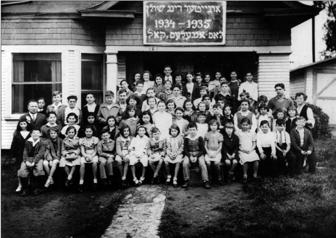
Arbeter Ring/Workmen's Circle School, Boyle Heights, 1935 (Los Angeles Public Library)
