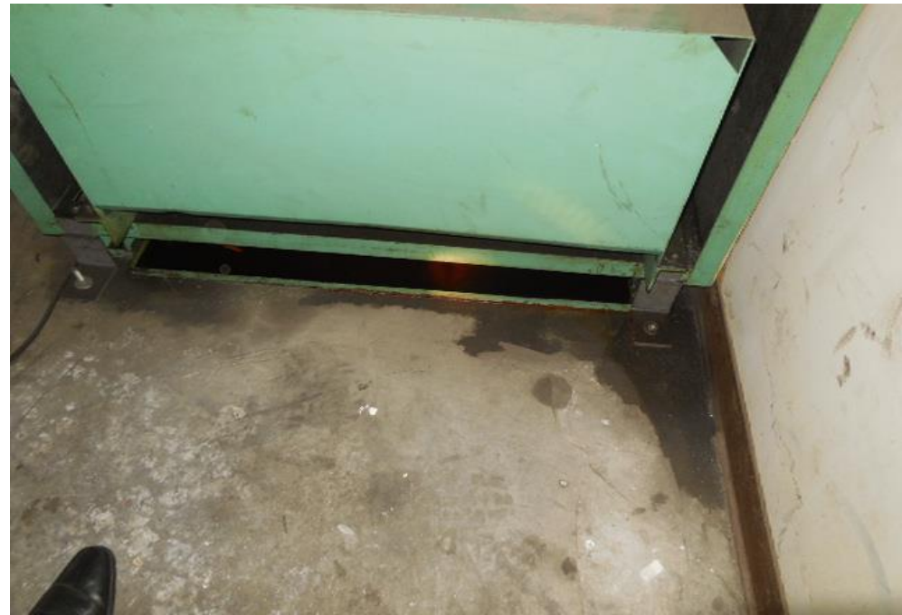
View of minor oil staining below the control equipment for the freight elevator.
