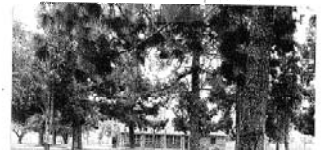
Exterior views of the Stonehurst Recreation Center.
