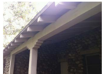
Many porches will use simple decorative features such as these brackets.
