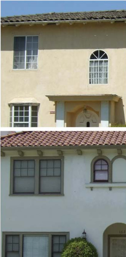
Flush, frameless, and oddly arranged windows may be inappropriate on a new house.
