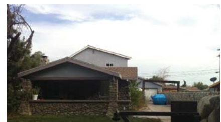
Though this second-story addition is set back from the front of the house, its roofline and window pattern could be better suited to the historic bungalow.
