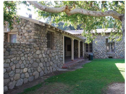
Important features such as the Stonehurst Recreation Center should be preserved..
