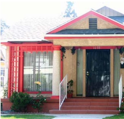
This doorway has been altered with a metal gate and plate glass sidelights.
