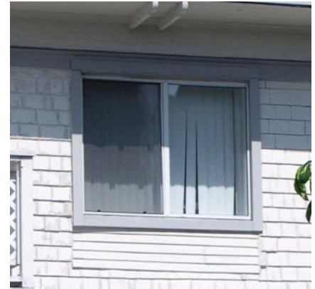
Replacement windows that are ill-suited for the original opening can negatively alter the look of a house.
