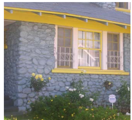
Stone and masonry should always be left to exhibit their natural finish qualities. Painting over the Arroyo stone on this house has muted the stone's texture.
