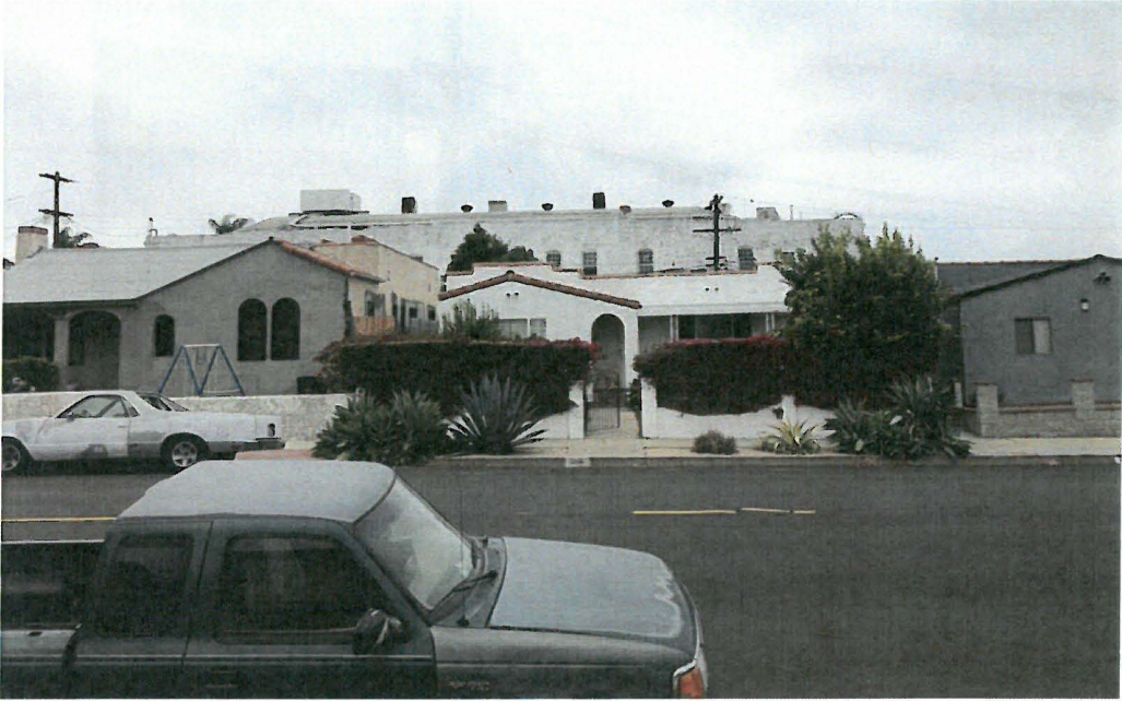
View from the South
