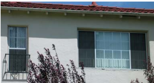
These replacement windows are inappropriate. When putting new windows on the front facade of a home, the new windows should match the historic windows in size, shape, arrangement of panes, materials, hardware, method of construction, and profile.
