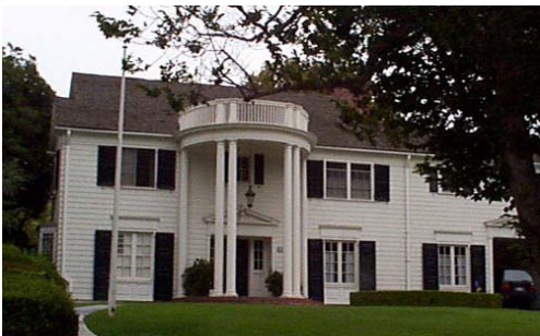
A house with wood siding should not be stuccoed over.
