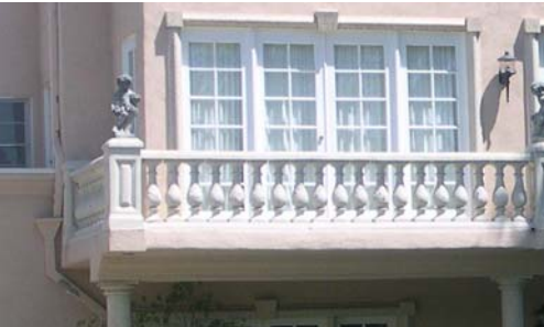
This addition of a balcony with closely spaced incompatible balustrades detracts from the historic character of the home.
