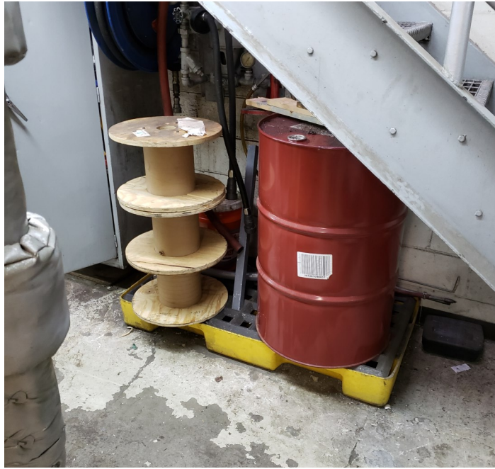
Photo 11—Hydraulic oil stored in maintenance area of northern site building.
