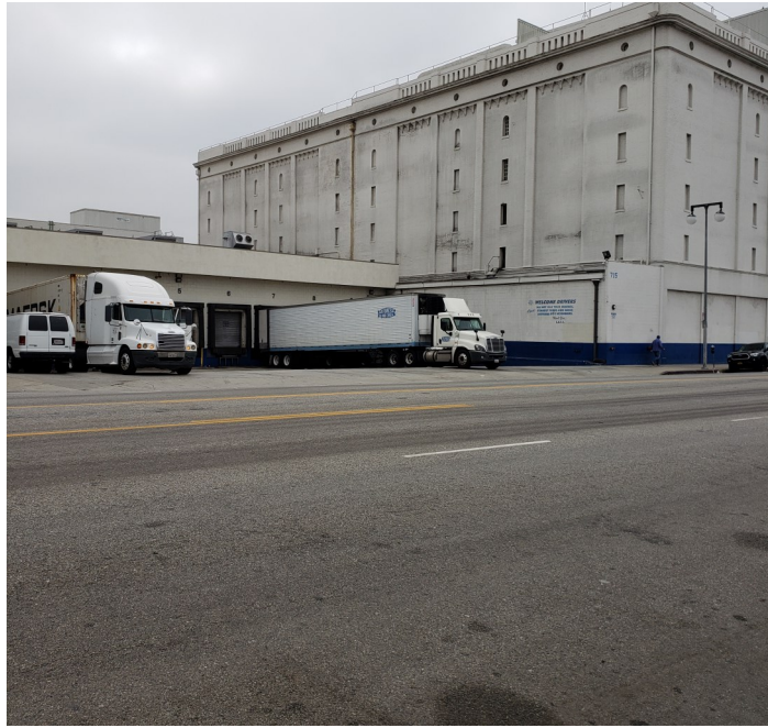
Photo 5—View southeast of northern building and loading dock area on north side of the building.
