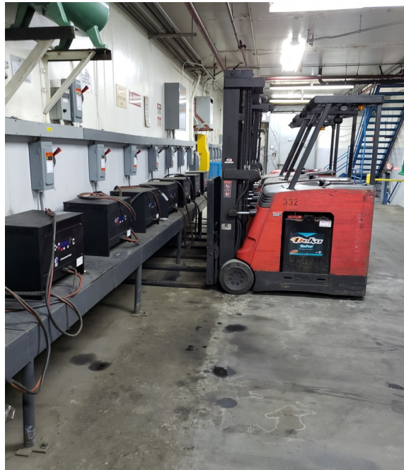
Photo 16—Forklift storage area in maintenance area of the southern site building.
