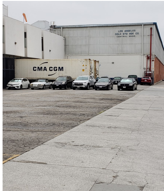
Photo 4—View south, along S. Central Avenue of the west side of the southern building on the Site.
