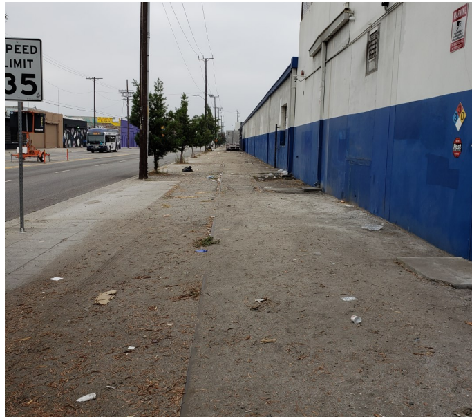
Photo 2—View south along Alameda Street from northeast corner of the Site showing railroad tracks on east side of southern building on the Site.
