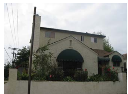
Apart from the inappropriate massing of this addition, the materials on the original house have been modified to suit the addition
