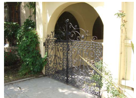
When used, gates should be transparent, well fitted for their opening, and appropriate to the style of the house. This ornate wrought iron is appropriate to the Spanish Colonial style
