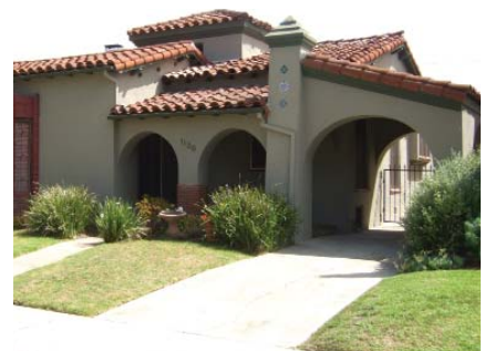
Arcades should read as open voids and not as fully enclosed space.
