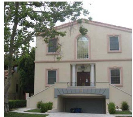
The Carthay Circle setting is characterized by garages located in the rear and modest front walkways leading directly to front doors. This newer home eschews that pattern and would be inappropriate in the HPOZ.
