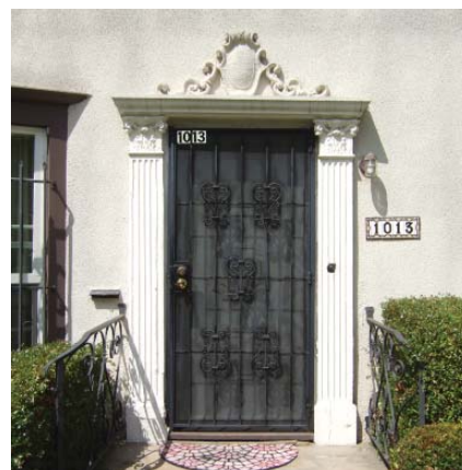
Security gates on visible doors diminish the character of the neighborhood and should be avoided.
