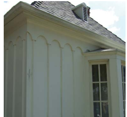
Wood cladding such as these decorative batten boards are rarely off the shelf
