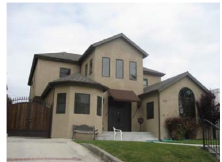
The original single-story cottage has been lost to this second story addition..
