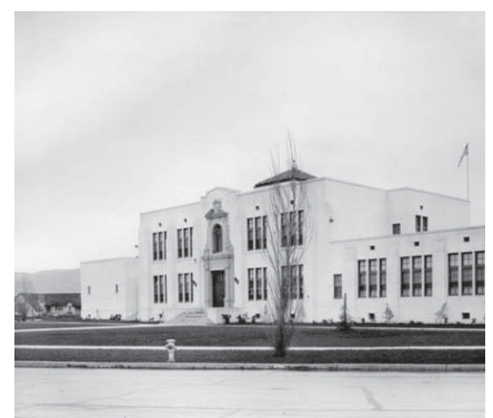
Carthay Center School building.
