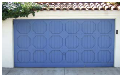
Historic garage doors are designed to match the unique decorative details found elsewhere on the house. Off-the-shelf replacement doors should be avoided.
