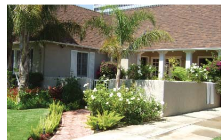
Low-slung garden walls create a gradual transition from public to private space.
