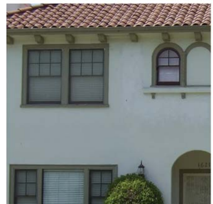
Flush, frameless, and oddly arranged windows may be inappropriate on a new house.
