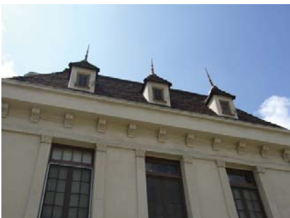
Decorative features such as dormers and finials should always be preserved in-place.
