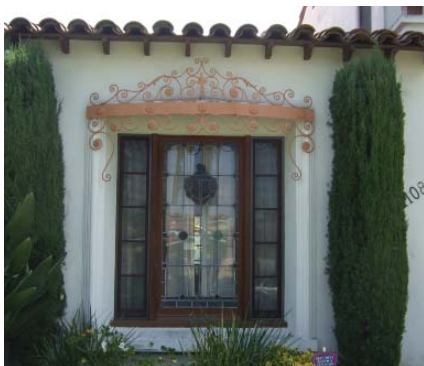
Prominent picture windows and bay windows with decorative art glass are oft found on Carthay Circle houses.
