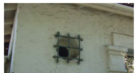
Original grille-work complements fenestration rather than obscuring it.
