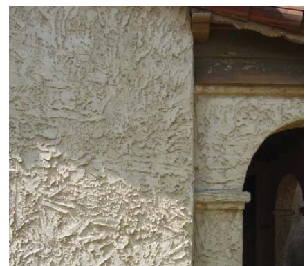
Original stucco surfaces in Carthay Circle were hand troweled and smooth. Heavily textured stucco or sprayed stucco is inappropriate
