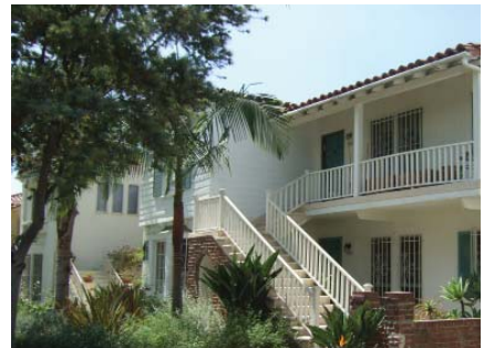
Stair railings, balcony posts and balustrades and other features should always be preserved in place.
