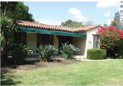
An awning provides shade and is a reversible, non-permanent alteration to this house that was originally constructed without a porch
