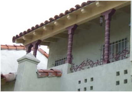
Turned wood accents and decorative wrought iron are important details on a Spanish Colonial house.
