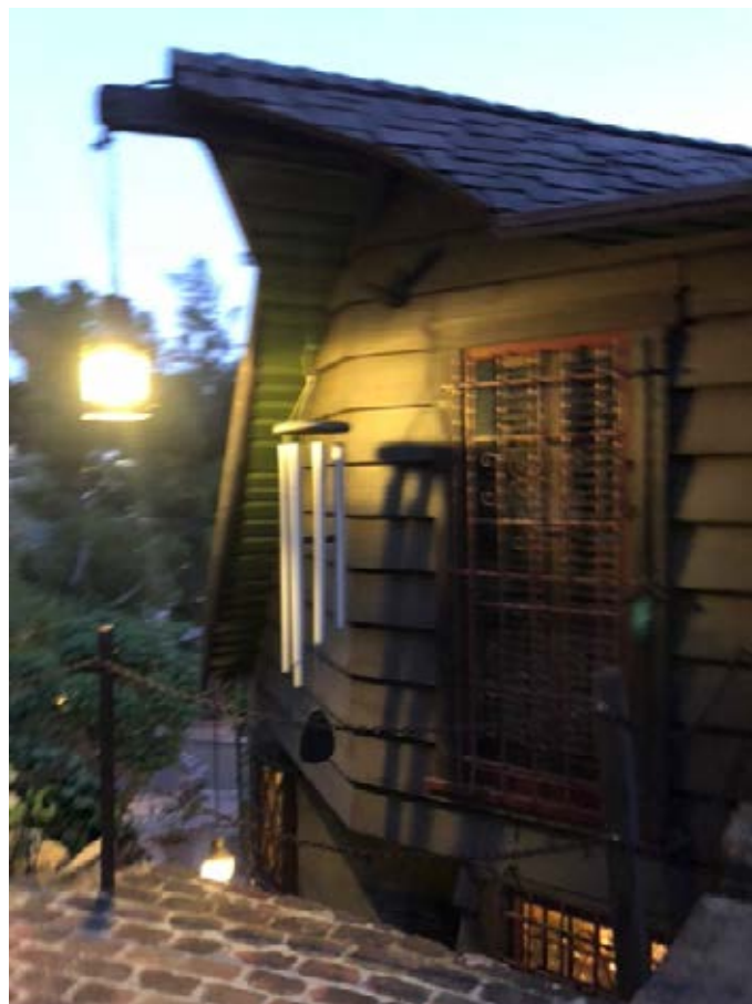
16. Whimsy Hall: Gable. View: S.
