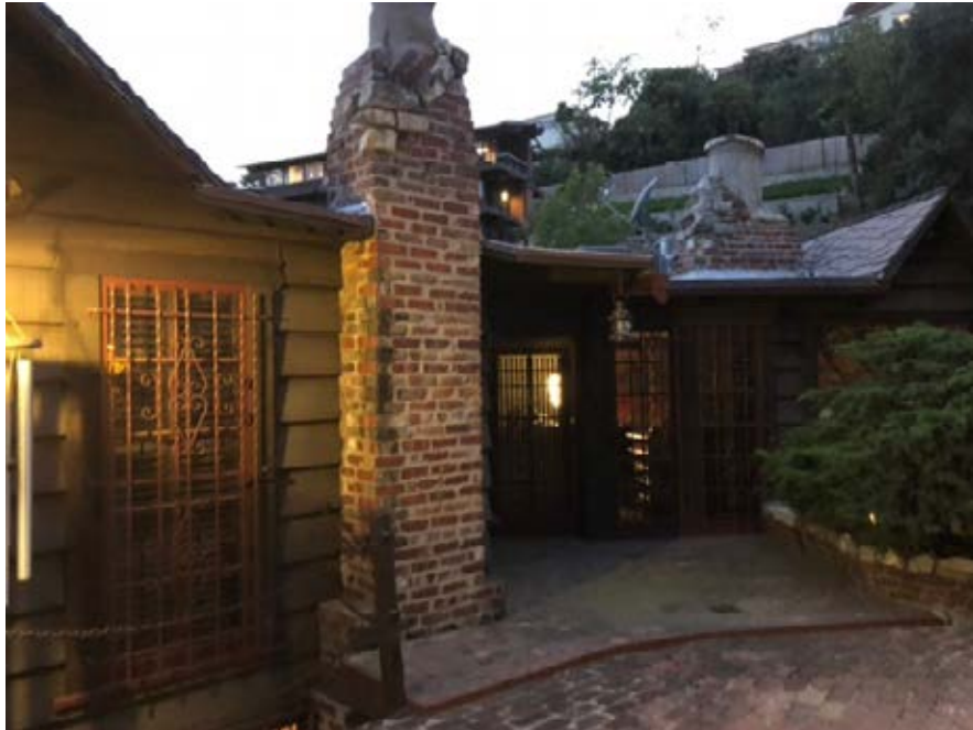
15. Whimsy Hall: Chimneys. View: W.
