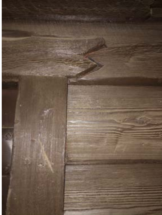
18. Standalone Kitchenette behind Whimsy Hall: doorframe detail. View: S.
