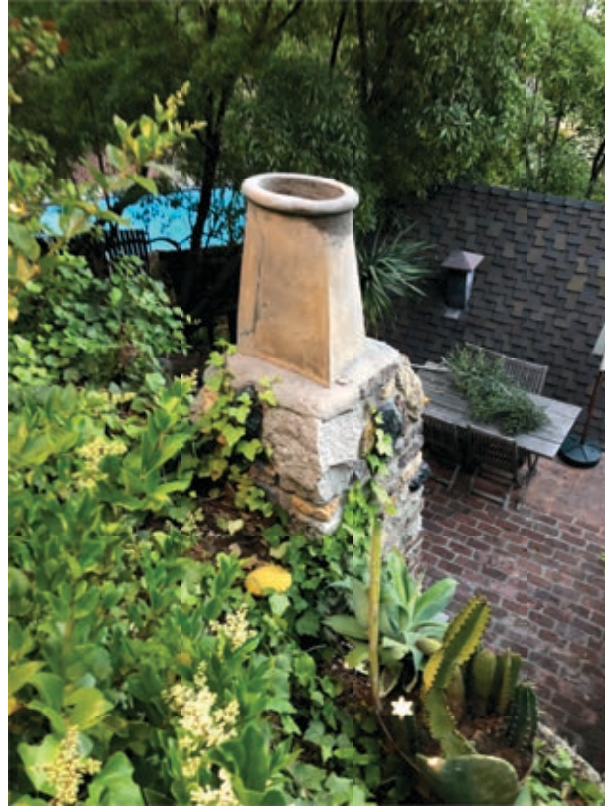
7. Star Sailer Manor, Chimney Pot detail. View: E.
