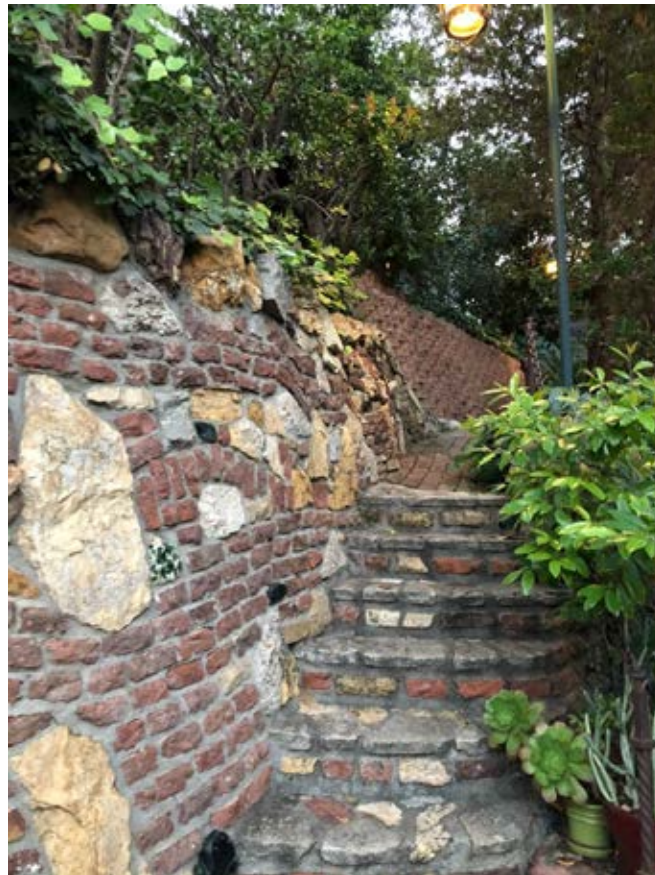
28. Rubble course walkway.
