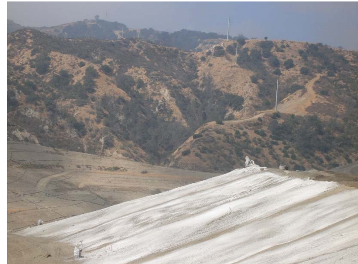
Photo 216: Closure Turf & Posi-Shell: August 14, 2017
