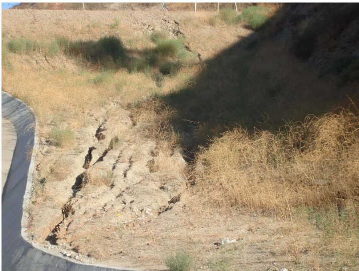
Photo 411: Terminal Basin Inlet Channel Deep Erosion: September 12, 2017
