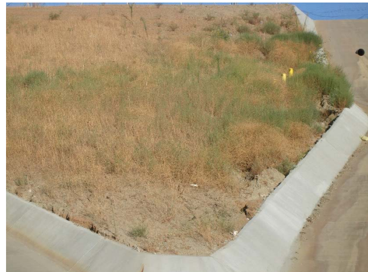
Photo 412: Terminal Basin Inlet Channel Deep Erosion: September 12, 2017
