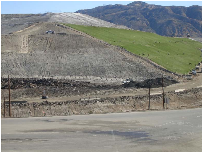
Photo 243: Closure Turf & Posi-Shell: September 26, 2017
