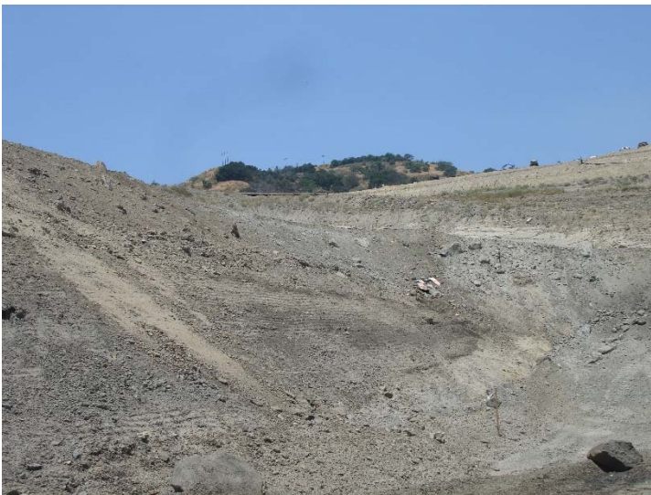
Photo 111: CC4A Part 2 Excavation Area Slide: July 11, 2017
