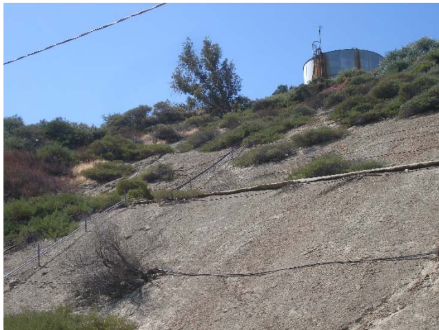
Photo 635: Slope Drainage above Flare 1 Erosion: September 12, 2017
