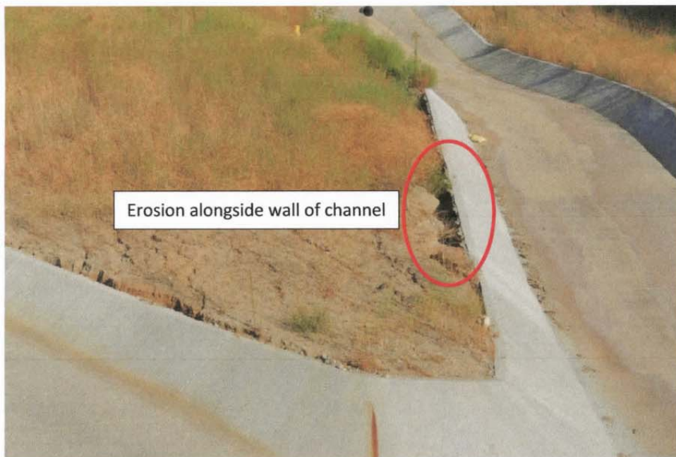
Photo 5: Erosion gullies at temporary earthen basin above Terminal Basin
