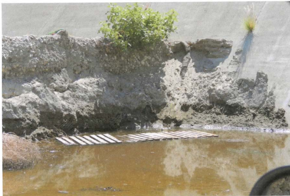
Photo 2: Water behind gabion wall and vegetation growing in Terminal Basin
