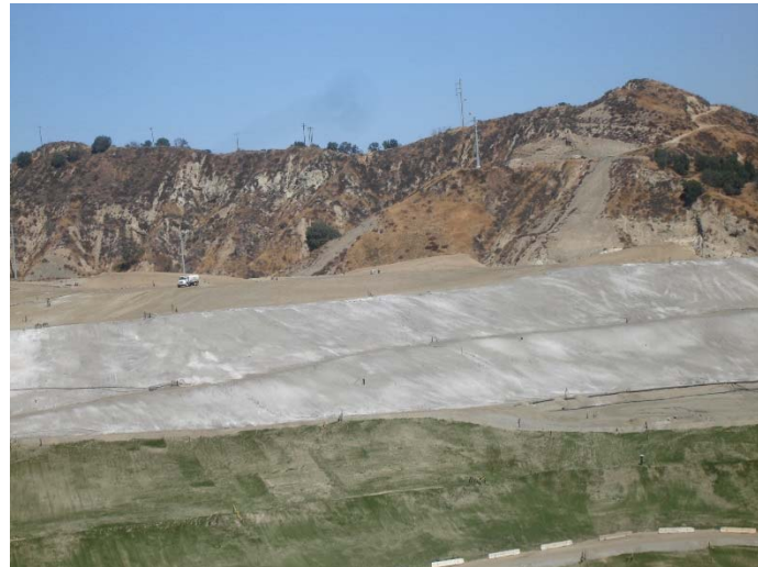
Photo 247: Closure Turf & Posi-Shell: September 26, 2017
