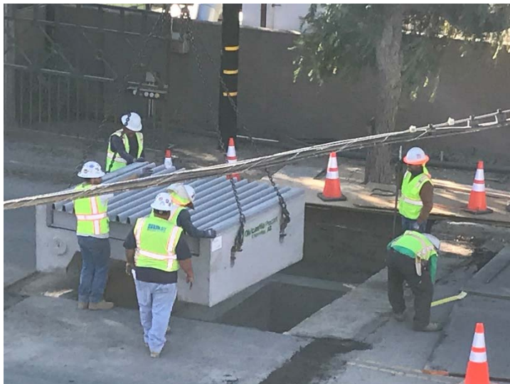
Photo 507: Terminal Basin Outlet Roadway Cattleguard Construction: September 26, 2017
