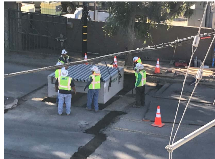
Photo 508: Terminal Basin Outlet Roadway Cattleguard Construction: September 26, 2017
