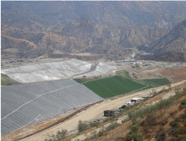
Photo 209: Closure Turf & Posi-Shell: August 14, 2017
