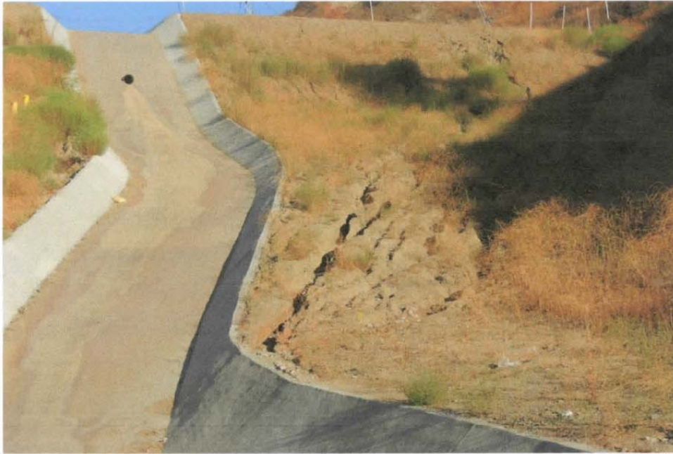
Photo 5: Erosion gullies at temporary earthen basin above Terminal Basin
