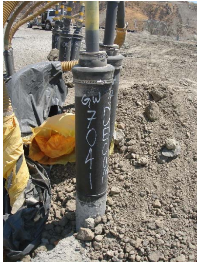
Photo 173: Decommissioned Gas Well with Liquids Backing Up: July 11, 2017
