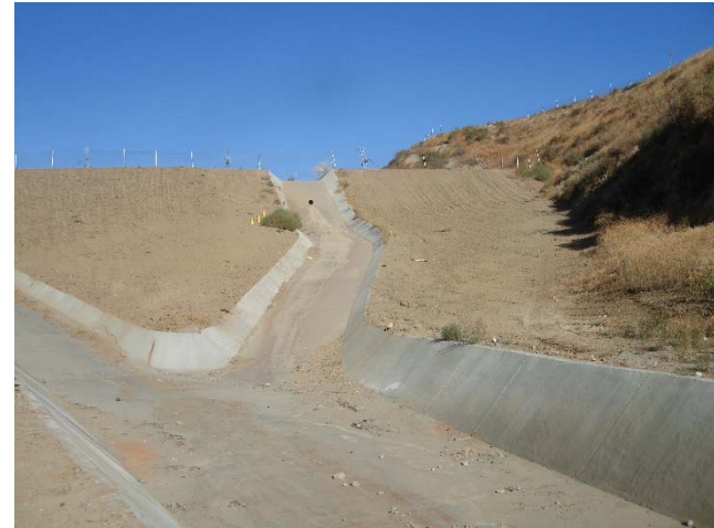
Photo 418: Terminal Basin Inlet Channel Erosion Repaired: September 26, 2017
