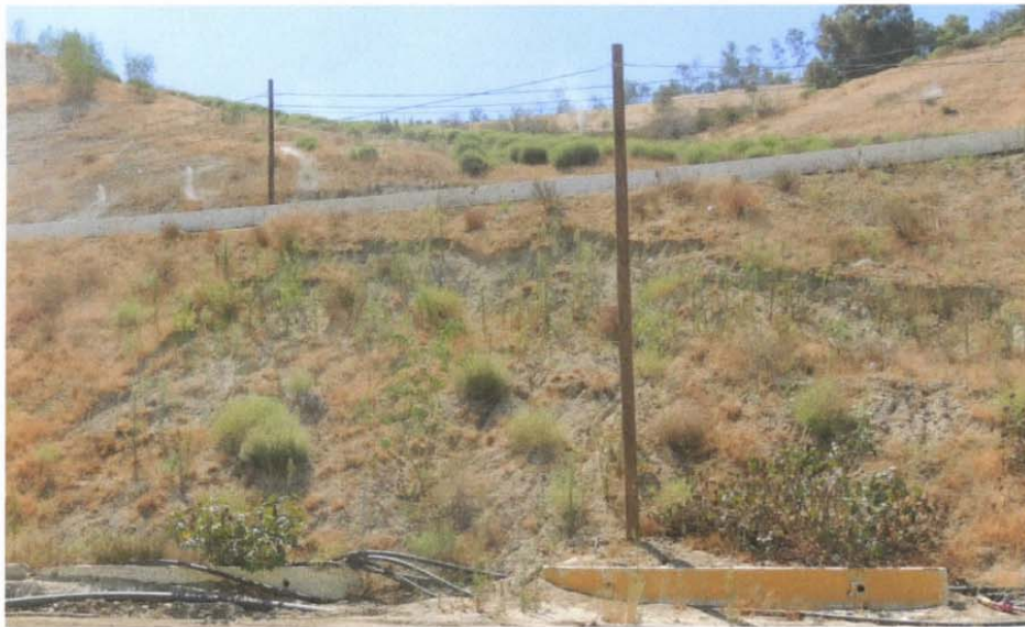
Photo 8: Sloughing on embankment of new access road
