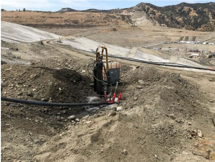
Photo 155: Cell CC3A Slope Gas Well Liquid Surge: July 25, 2017
