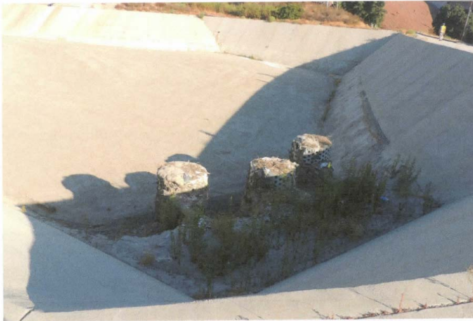
Photo 1: Sediments behind decant towers at Terminal Basin
