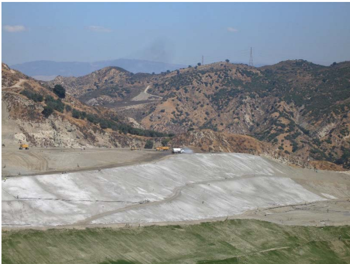
Photo 223: Closure Turf & Posi-Shell: September 12, 2017
