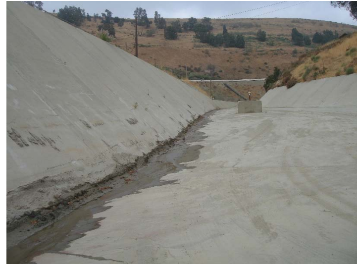
Photo 446: Terminal Basin Alluvial Water Seep: August 14, 2017
