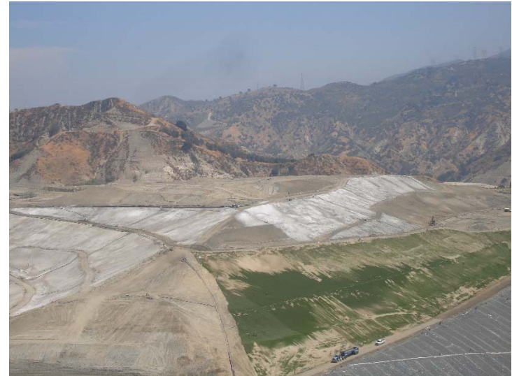
Photo 206: Closure Turf & Posi-Shell: August 14, 2017
