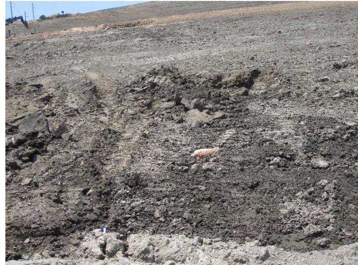
Photo 114: CC4A Part 2 Excavation Area Slide: July 11, 2017
