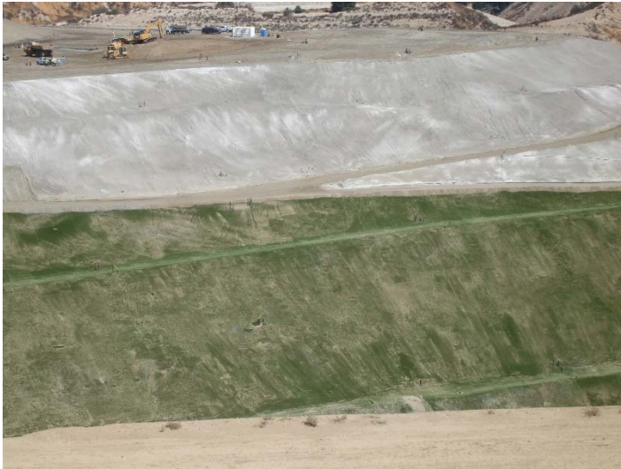
Photo 241: Closure Turf & Posi-Shell: September 26, 2017
