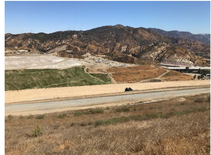
Photo 236: Closure Turf & Posi-Shell: September 26, 2017
