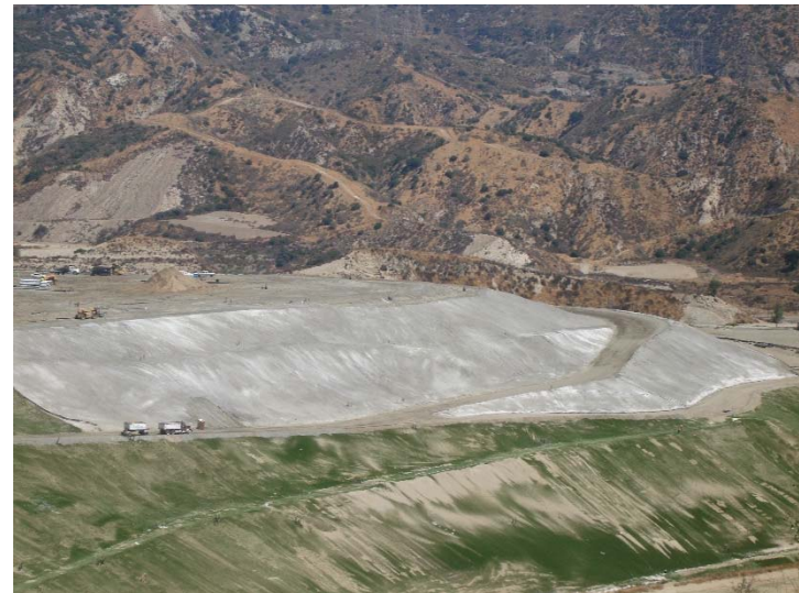
Photo 224: Closure Turf & Posi-Shell: September 12, 2017
