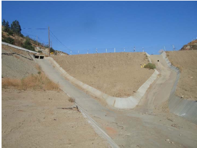
Photo 417: Terminal Basin Inlet Channel Erosion Repaired: September 26, 2017
