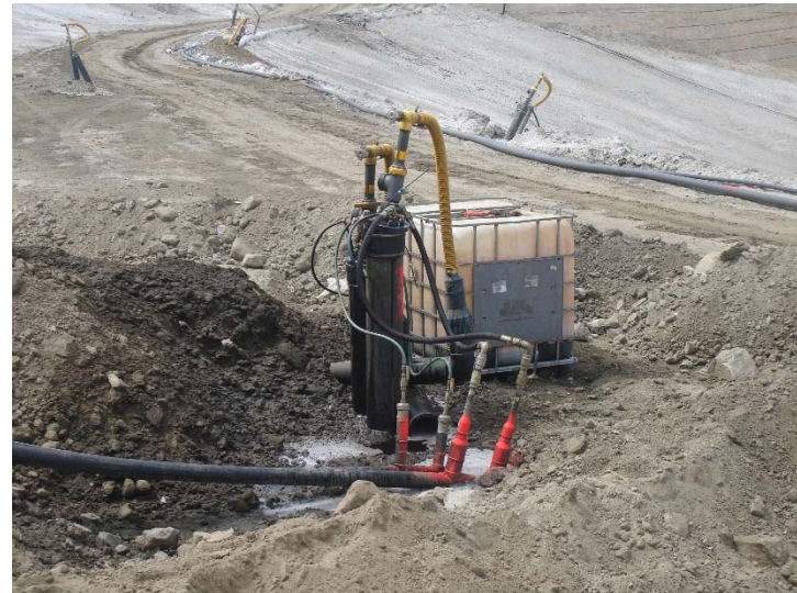
Photo 156: Cell CC3A Slope Gas Well Liquid Surge: July 25, 2017
