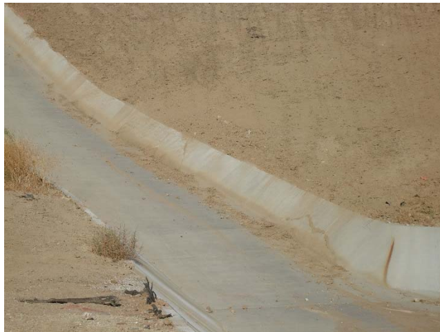
Photo 419: Terminal Basin Inlet Channel Erosion Repaired: September 26, 2017
