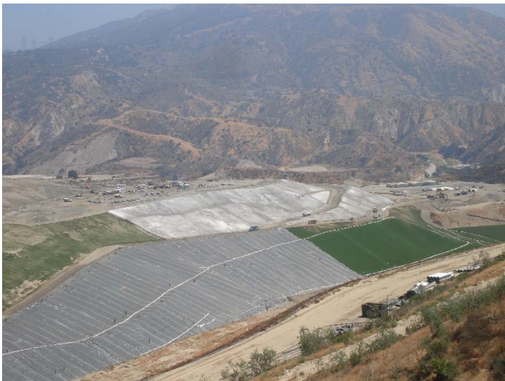
Photo 207: Closure Turf & Posi-Shell: August 14, 2017
