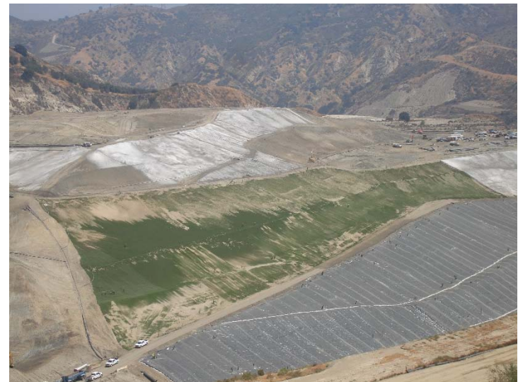
Photo 208: Closure Turf & Posi-Shell: August 14, 2017
