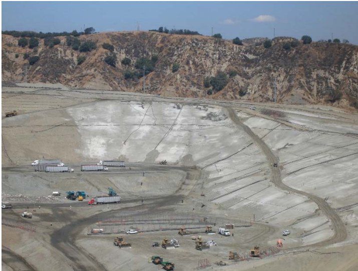
Photo 221: Closure Turf & Posi-Shell: September 12, 2017
