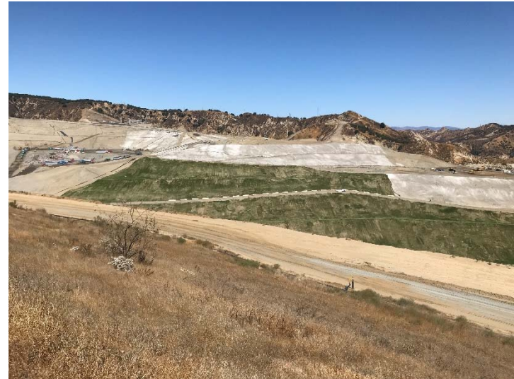
Photo 234: Closure Turf & Posi-Shell: September 26, 2017
