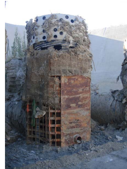
Photo 492: Terminal Basin Outlet Risers: September 26, 2017
