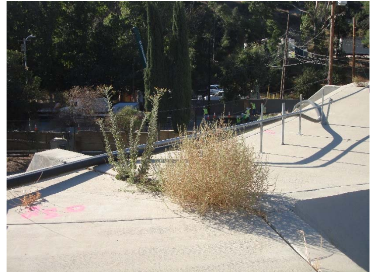
Photo 502: Brush Growing in Terminal Basin Concrete Cracks: September 26, 2017
