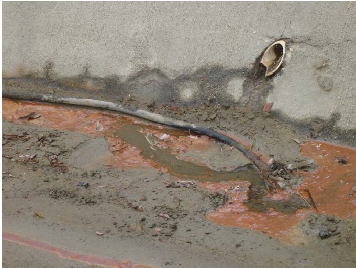
Photo 445: Terminal Basin Alluvial Water Seep: August 14, 2017
