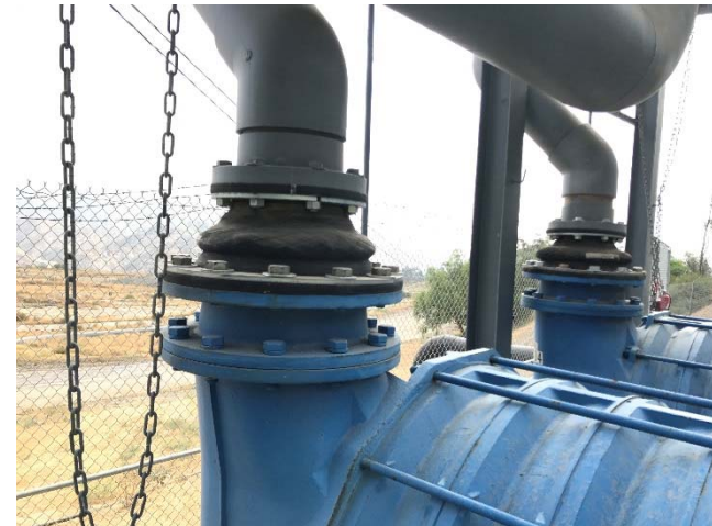
Photo 632: Flare 1 Leaking Flange: July 25, 2017
