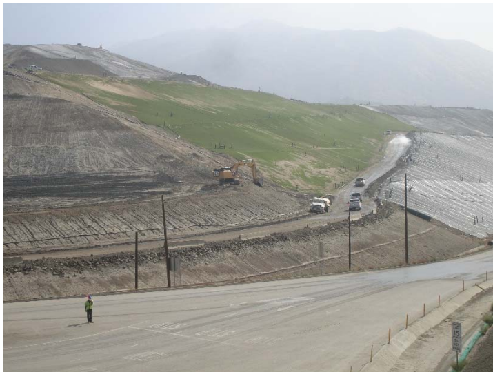
Photo 211: Closure Turf & Posi-Shell: August 14, 2017
