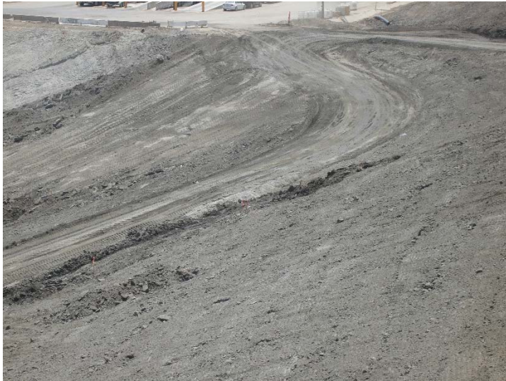
Photo 113: CC4A Part 2 Excavation Area Slide: July 11, 2017
