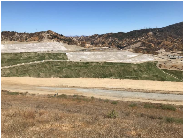
Photo 235: Closure Turf & Posi-Shell: September 26, 2017
