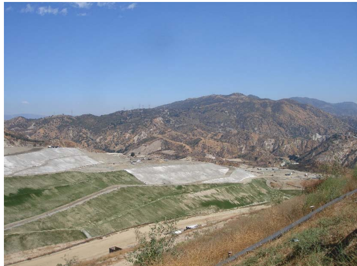
Photo 220: Closure Turf & Posi-Shell: September 12, 2017
