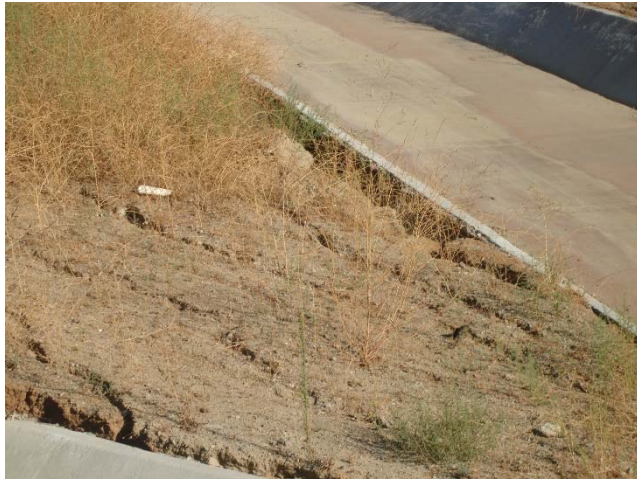
Photo 413: Terminal Basin Inlet Channel Deep Erosion: September 12, 2017
