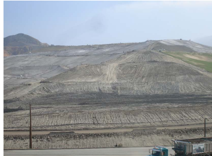
Photo 210: Closure Turf & Posi-Shell: August 14, 2017
