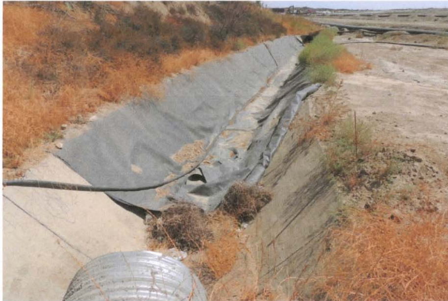
Photo 7: Geomembrane at channel between Basin B and D
