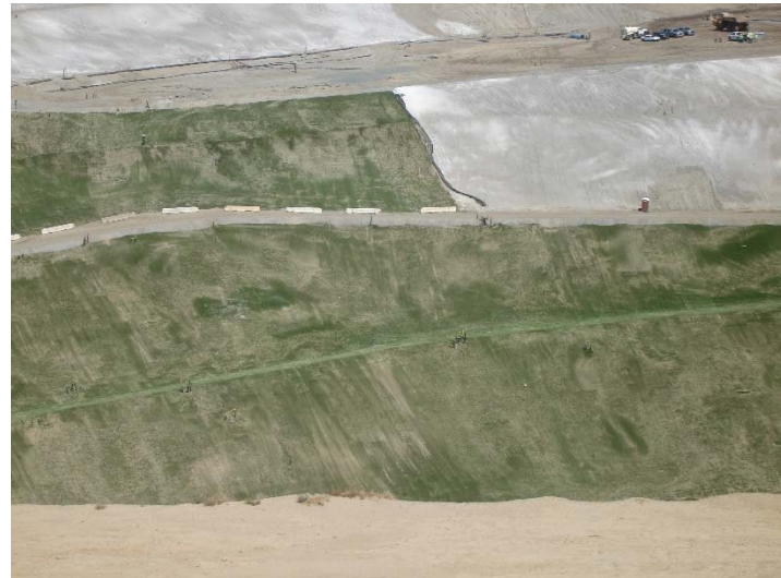
Photo 240: Closure Turf & Posi-Shell: September 26, 2017
