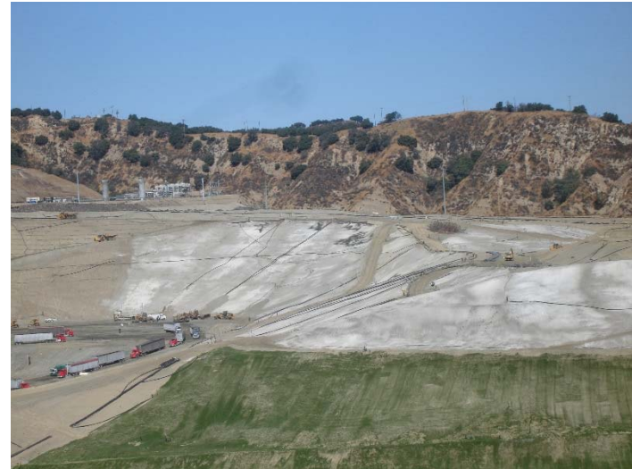
Photo 246: Closure Turf & Posi-Shell: September 26, 2017
