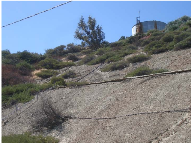
Photo 637: Slope Drainage above Flare 1 Erosion: September 26, 2017
