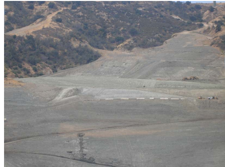
Photo 128: CC4A Part 2 Excavation Area Slide: July 25, 2017
