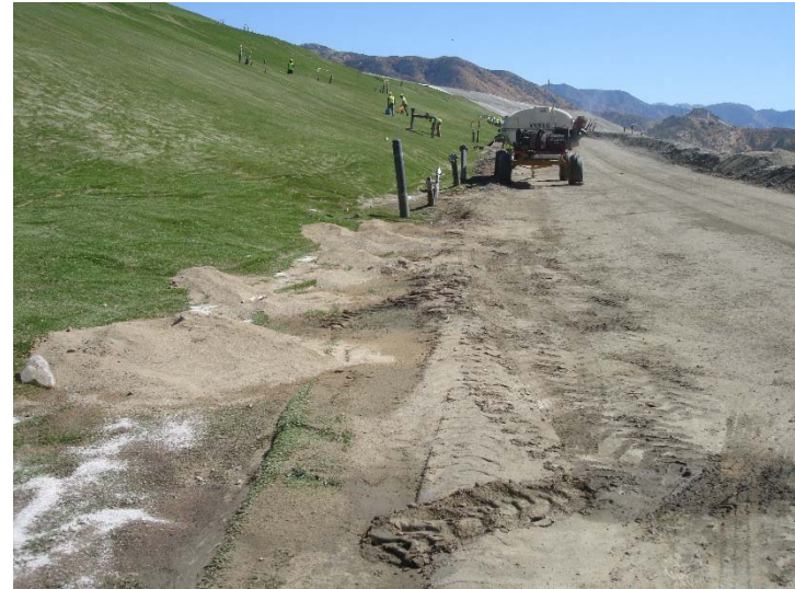
Photo 150: Cell CC3A Liquid Break-Out Area: July 11, 2017
