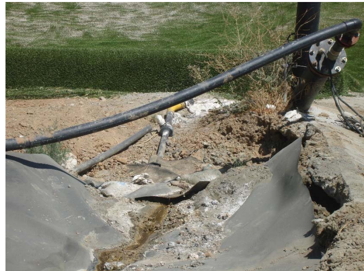
Photo 220: CC3B Alluvial Slope Leak: July 24, 2018
