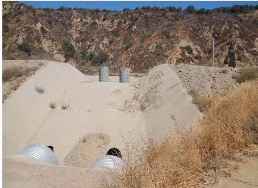
Photo 9: Cracked concrete spillway between two parts of Basin D and vegetation in crack
