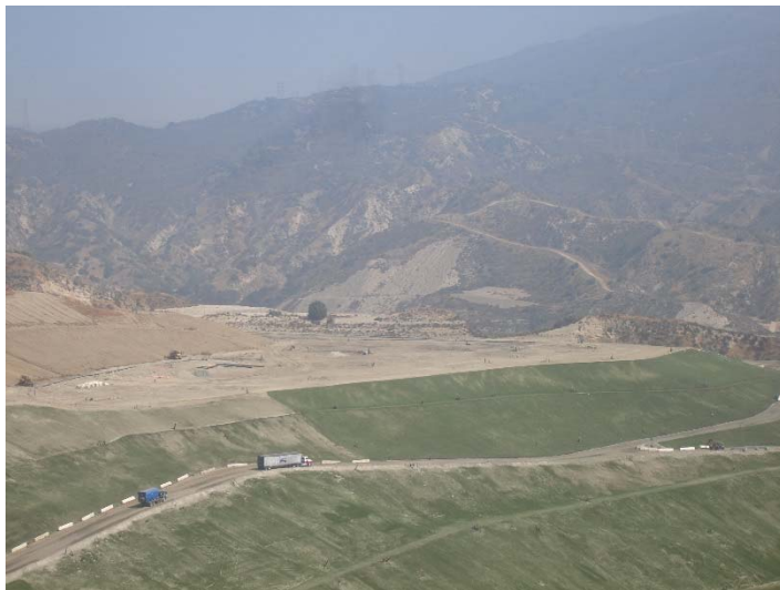
Photo 199: Posi-Shell and Closure Turf: September 25, 2018
