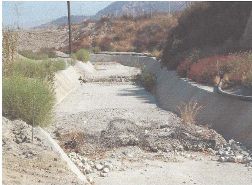
Photo 15: Debris in southern reach of east drainage channel
