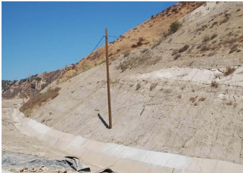
Photo 14: Repaired shotcrete sidewall of eastern drainage channel
