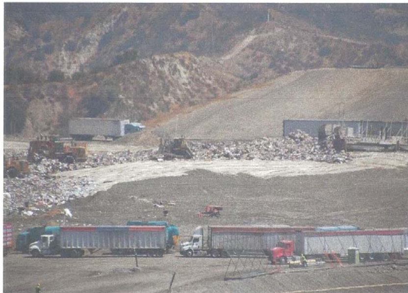
Photo 2: Alternative daily cover at Cell CC4 – Part 1
