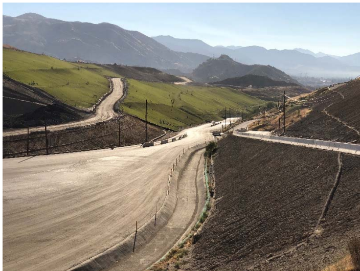
Photo 179: Posi-Shell & Closure Turf: July 5, 2018
