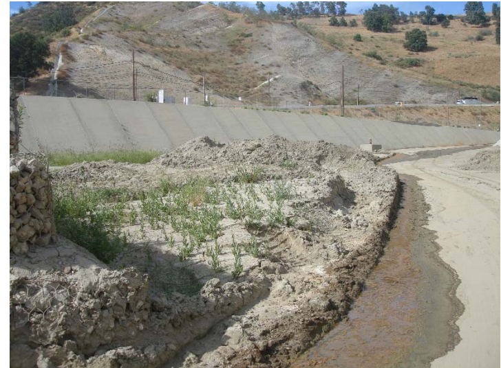
Photo 474: Alluvial Seep Flow into Terminal Basin: July 5, 2018
