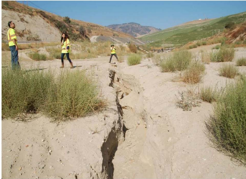
Photo 11: Gully in Cell CC3 basin
