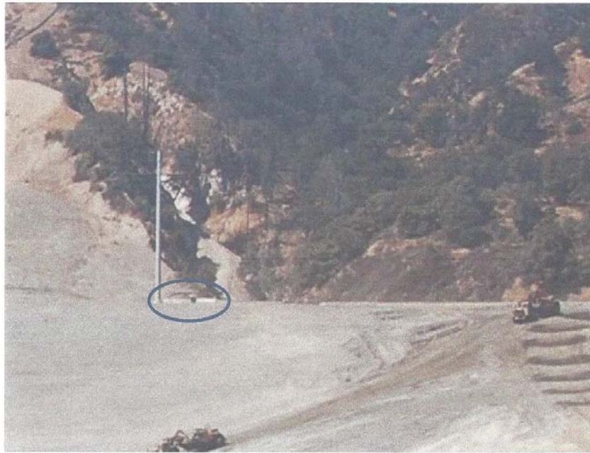
Photo 7: Spillway form Basin A shown in blue circle – Channel was removed downslope of basin
