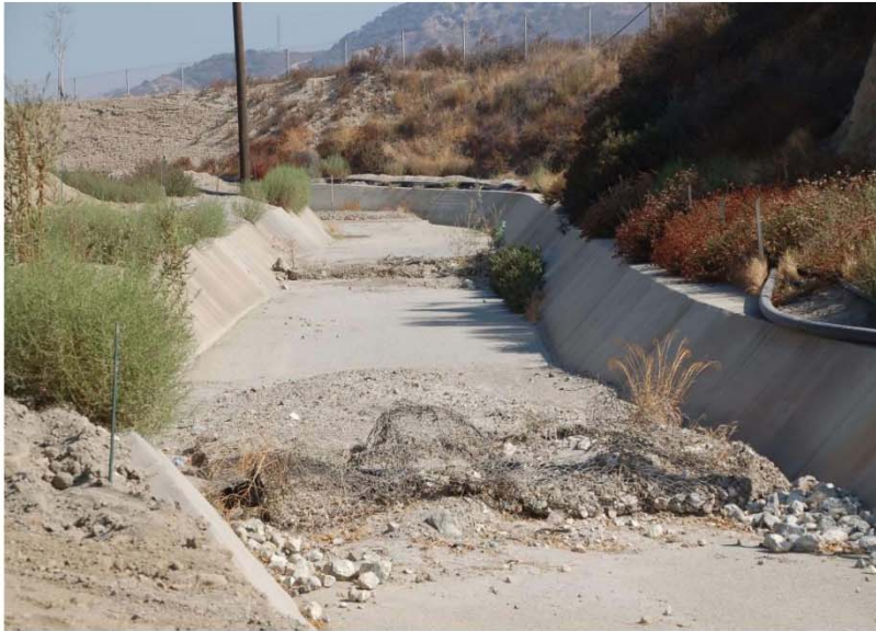
Photo 15: Debris in southern reach of east drainage channel
