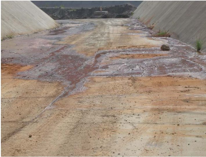
Photo 473: Alluvial Seep Flow into Terminal Basin: July 5, 2018
