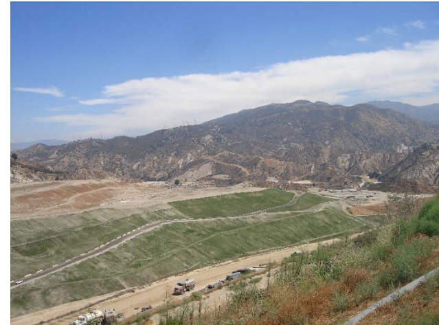
Photo 190: Posi-Shell and Closure Turf: August 29, 2018
