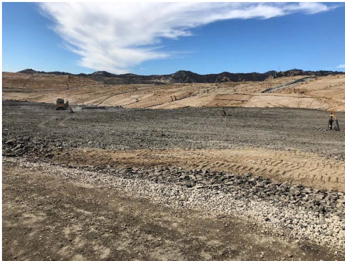
Photo 663: Landfill Perimeter Road Surfacing: August 29, 2018
