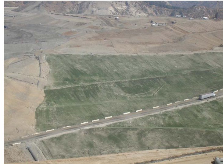
Photo 202: Posi-Shell and Closure Turf: September 25, 2018
