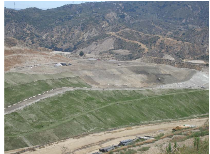
Photo 184: Posi-Shell & Closure Turf: July 5, 2018
