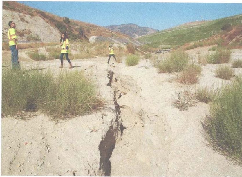
Photo 11: Gully in Cell CC3 basin
