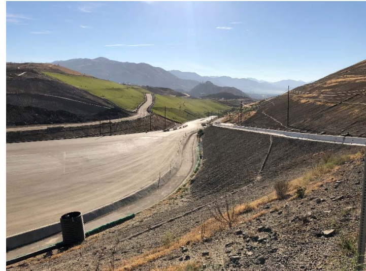
Photo 178: Posi-Shell & Closure Turf: July 5, 2018
