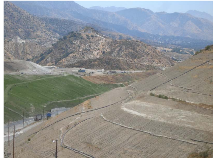
Photo 182: Posi-Shell & Closure Turf: July 5, 2018
