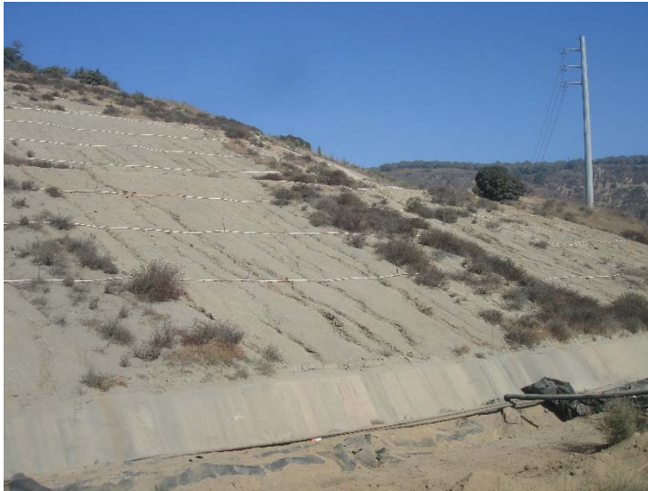
Photo 333: Sacrificial Liner Replacement Near County Sage Mitigation Area: September 25, 2018
