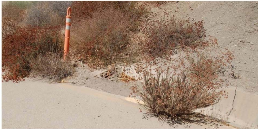
Photo 13: Sediments blocking the outlet drain of channel along the access road to the Flares 9-11
