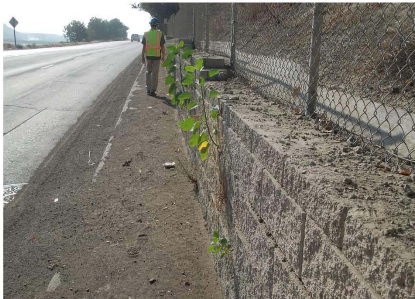
Photo 16: Retaining wall along San Fernando Road: Vegetation growing through precast elements of and sediments against curb blocking drains from swale
