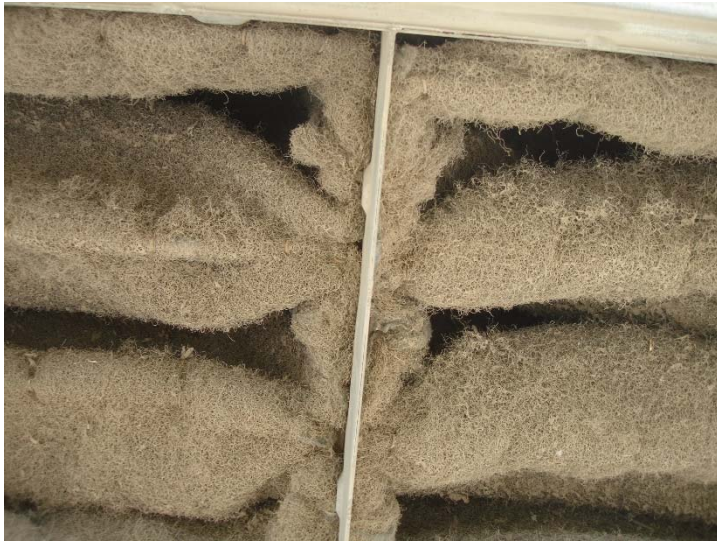
Photo 357: Old Flare 9 Blower Intake Air Filter: July 5, 2018
