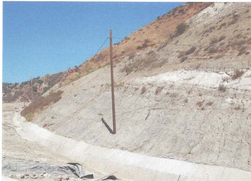
Photo 14: Repaired shotcrete sidewall of eastern drainage channel
