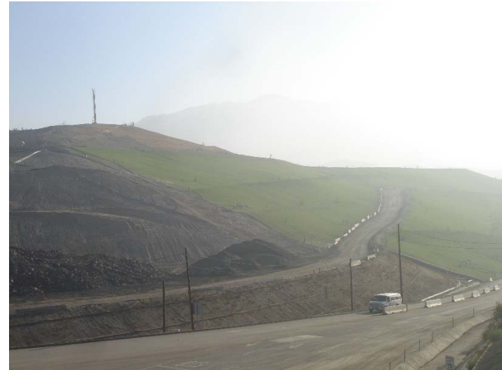
Photo 194: Posi-Shell and Closure Turf: September 12, 2018
