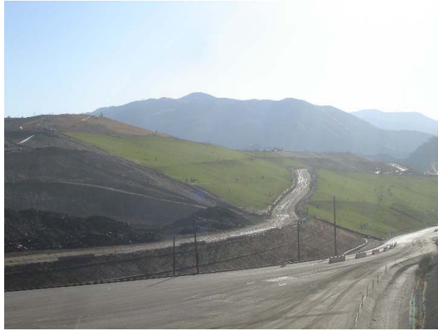
Photo 187: Posi-Shell and Closure Turf: July 24, 2018
