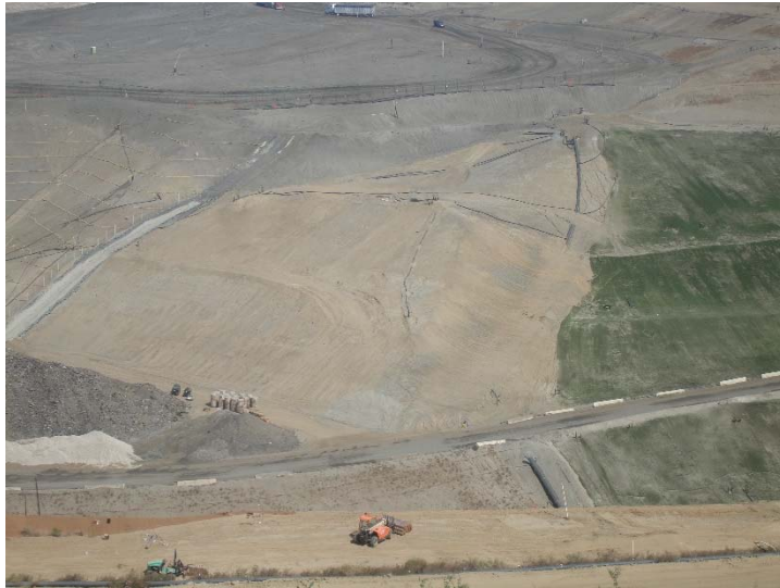
Photo 201: Posi-Shell and Closure Turf: September 25, 2018
