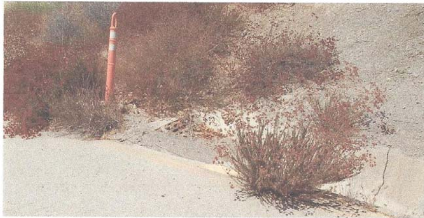
Photo 13: Sediments blocking the outlet drain of channel along the access road to the Flares 9-11
