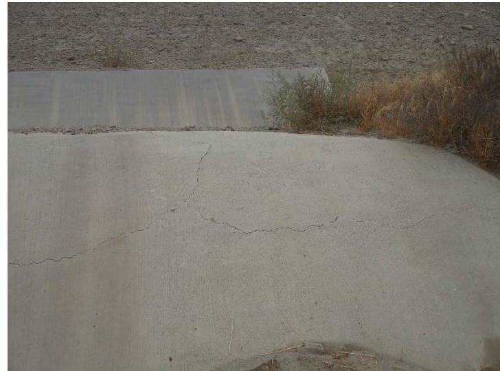
Photo 468: Basin B High Flow Channel Cracks: September 25, 2018
