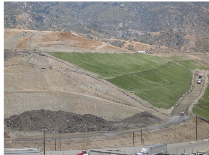
Photo 180: Posi-Shell & Closure Turf: July 5, 2018
