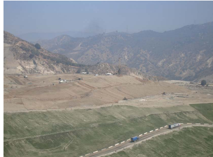
Photo 198: Posi-Shell and Closure Turf: September 25, 2018
