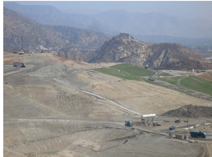
Photo 196: Posi-Shell and Closure Turf: September 12, 2018
