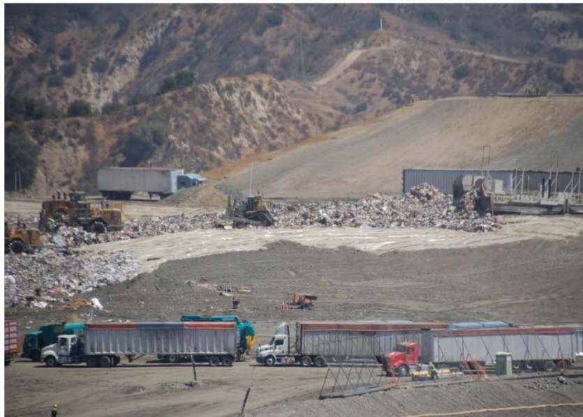
Photo 2: Alternative daily cover at Cell CC4 – Part 1
