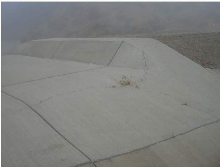
Photo 467: Basin B High Flow Channel Cracks: September 25, 2018
