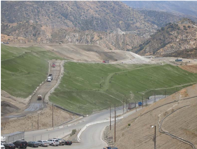
Photo 181: Posi-Shell & Closure Turf: July 5, 2018
