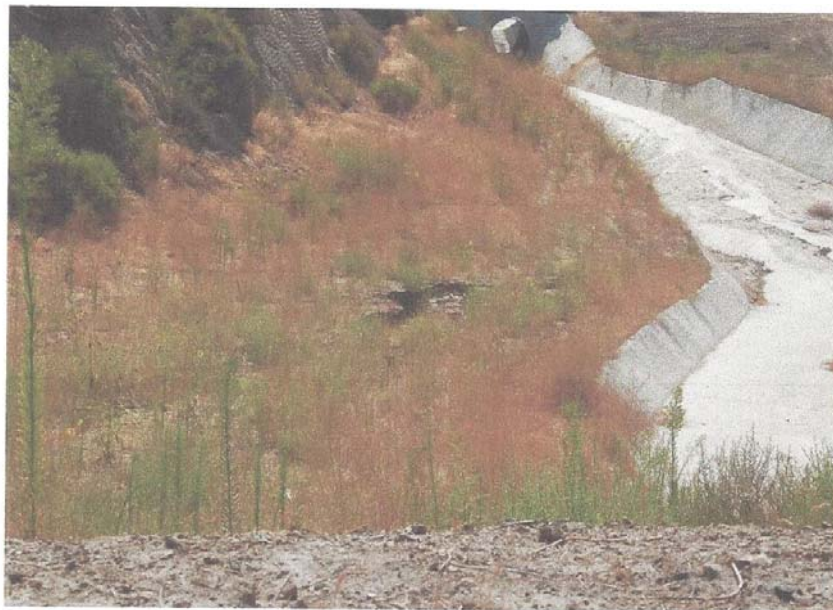
Photo 12: Erosion gully on downstream side of embankment of cell CC3 basin
