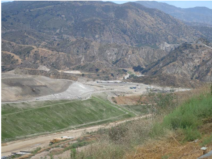
Photo 185: Posi-Shell & Closure Turf: July 5, 2018
