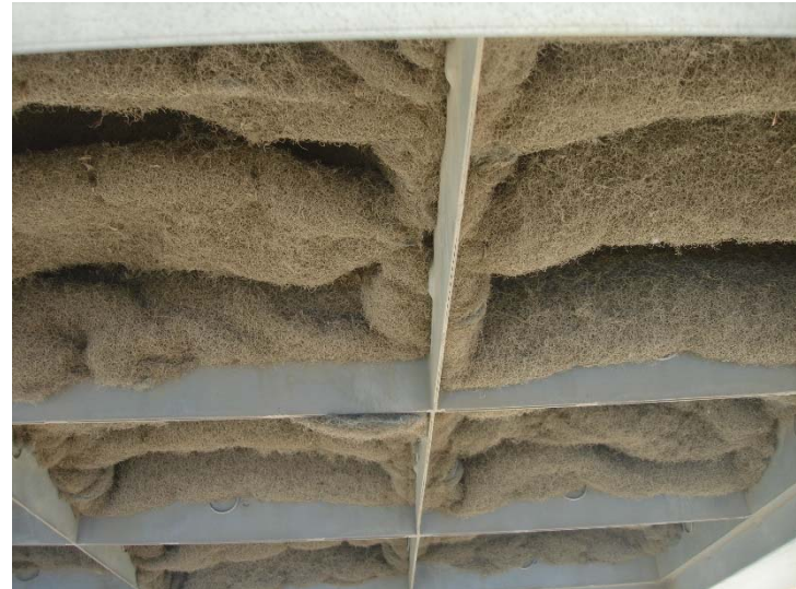
Photo 358: Old Flare 9 Blower Intake Air Filter: July 5, 2018
