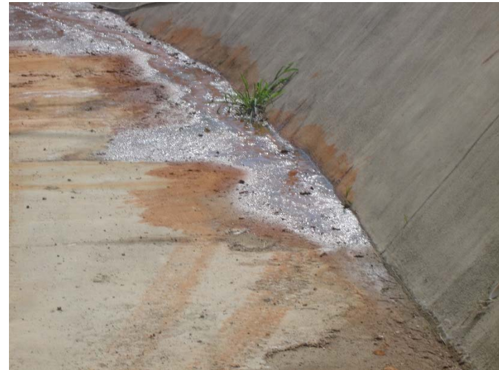
Photo 472: Alluvial Seep Flow into Terminal Basin: July 5, 2018
