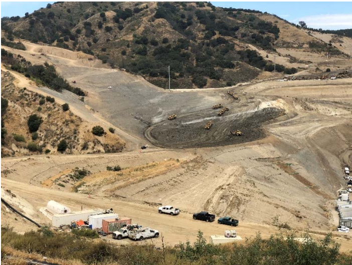
Photo 123: CC4 Part 3 & Buttress Excavation Area: July 05, 2018
