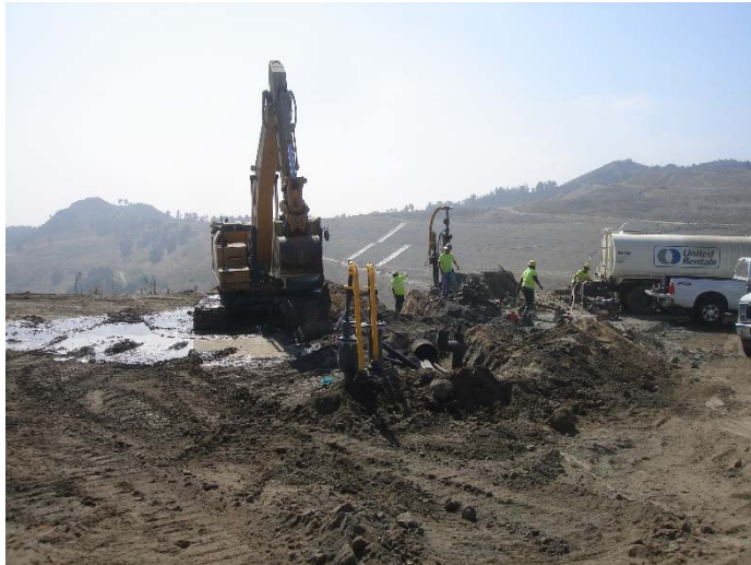
Photo 253: CC3A Top Deck Liquids Recovery Pipe Installation: September 25, 2018
