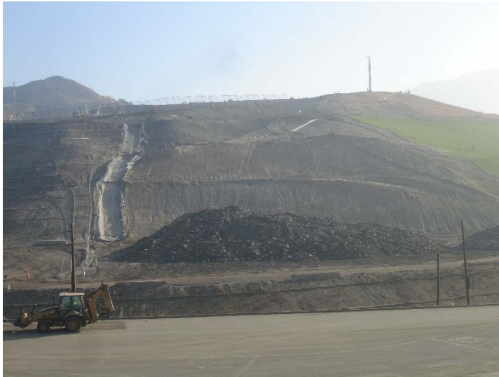
Photo 193: Posi-Shell and Closure Turf: September 12, 2018
