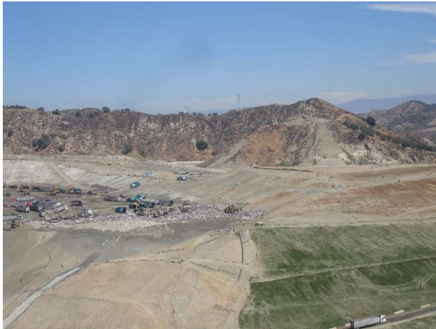
Photo 189: Posi-Shell and Closure Turf: August 29, 2018
