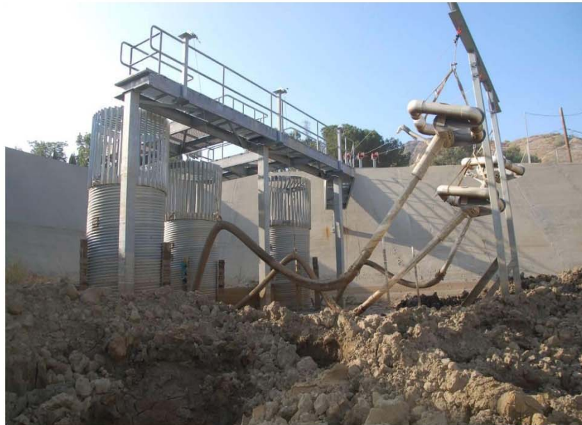
Photo 3: Sediment in terminal basin
