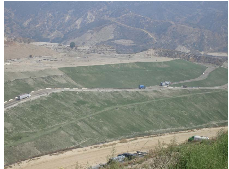
Photo 204: Posi-Shell and Closure Turf: September 25, 2018
