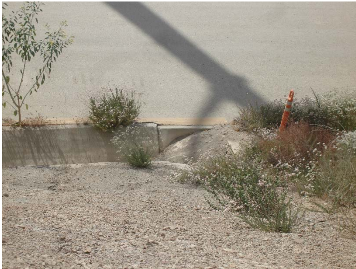
Photo 355: Plugged Drains at Bottom of Flare 9 Access Road: July 5, 2018
