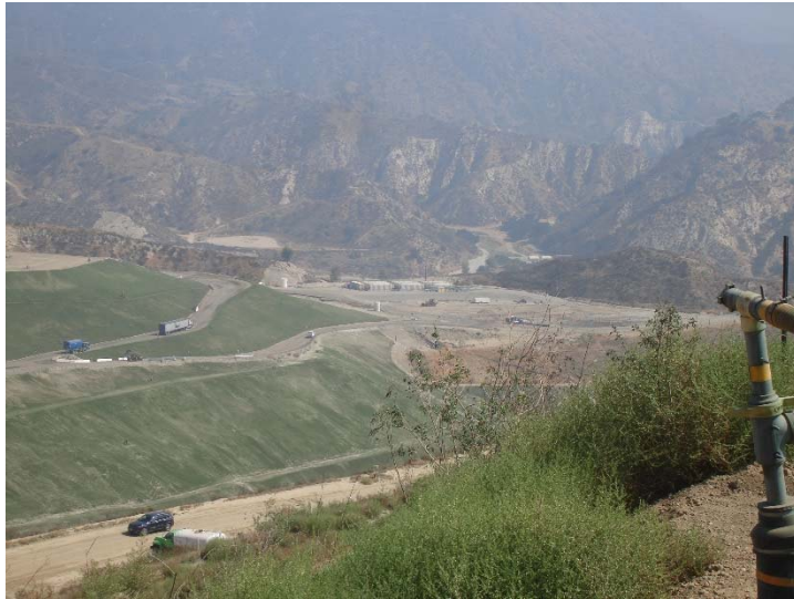
Photo 205: Posi-Shell and Closure Turf: September 25, 2018
