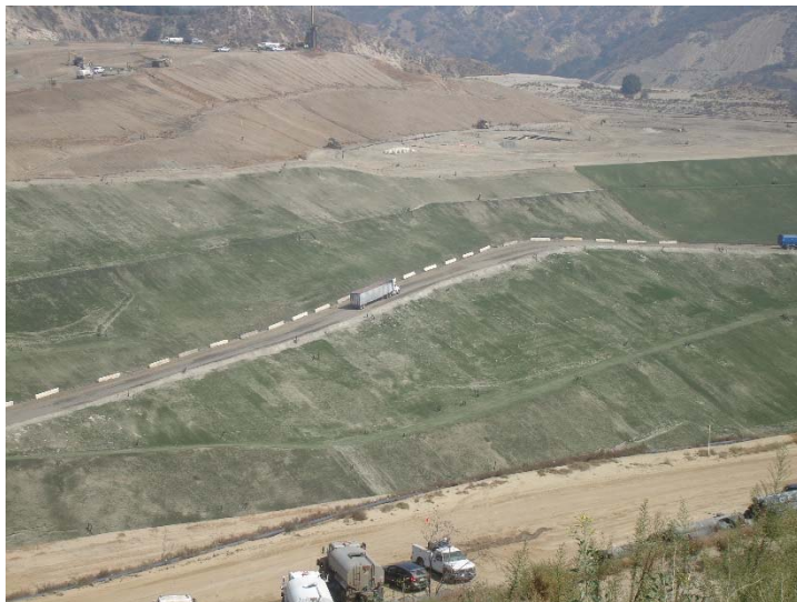
Photo 203: Posi-Shell and Closure Turf: September 25, 2018
