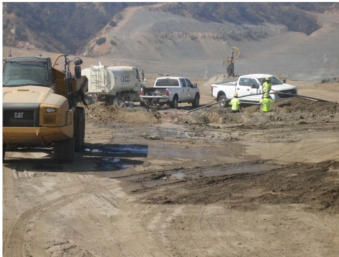
Photo 251: CC3A Top Deck Liquids Recovery Pipe Installation: September 25, 2018
