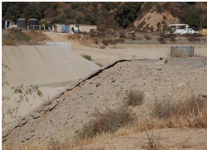
Photo 10: Separation between shotcrete and soil at Basin D
