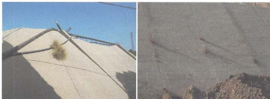
Photo 5: Plants growing in cracks in wall of Terminal Basin
