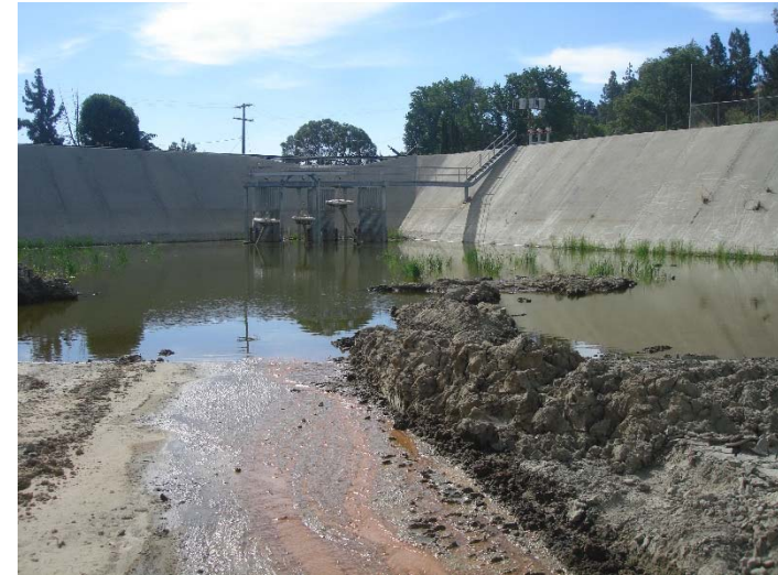
Photo 480: Alluvial Seep Flow into Terminal Basin: July 5, 2018
