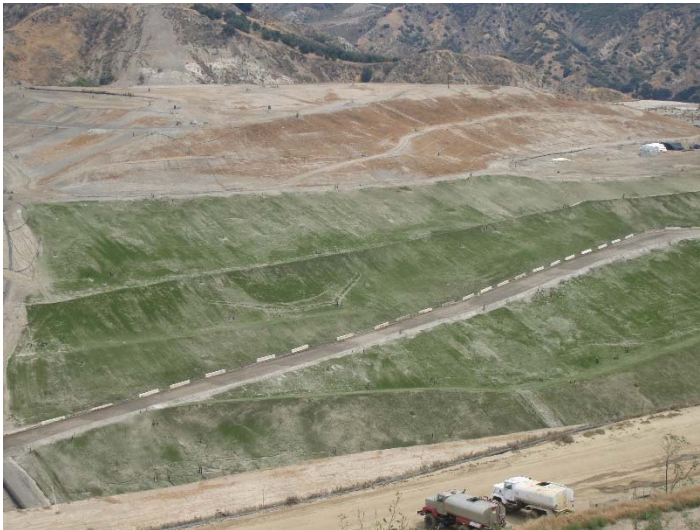
Photo 183: Posi-Shell & Closure Turf: July 5, 2018
