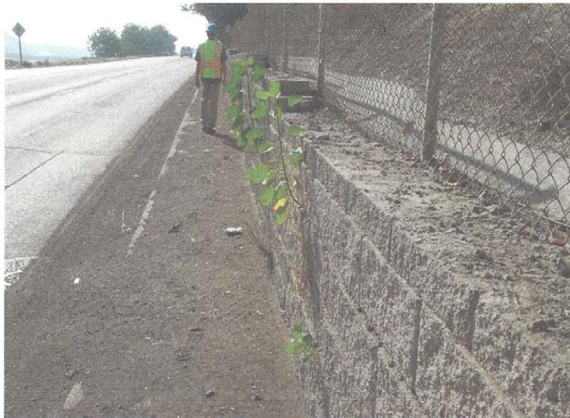
Photo 16: Retaining wall along San Fernando Road: Vegetation growing through precast elements of and sediments against curb blocking drains from swale
