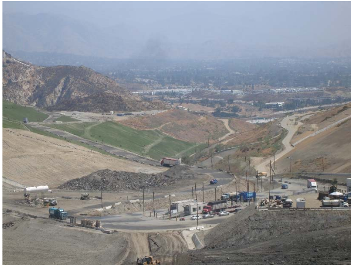
Photo 197: Posi-Shell and Closure Turf: September 12, 2018
