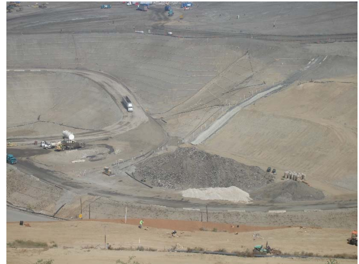
Photo 200: Posi-Shell and Closure Turf: September 25, 2018
