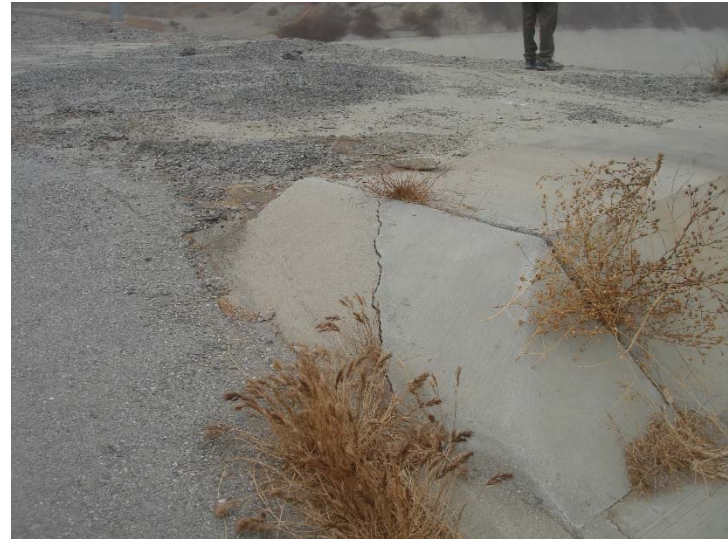
Photo 466: Basin B High Flow Channel Cracks: September 25, 2018
