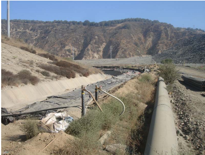
Photo 335: Sacrificial Liner Replacement Near County Sage Mitigation Area: September 25, 2018
