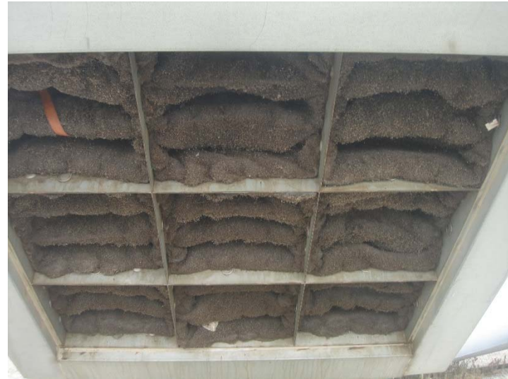
Photo 366: Flare 9 Blower Intake Air Filter: September 25, 2018
