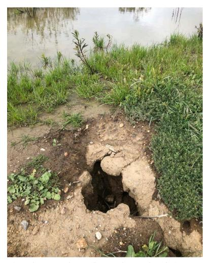
Slope Erosion where ponding spills over slope edge during storm events
