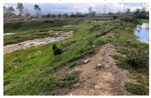
Ponding at top of slope and seepage at the toe of slope ARCHITERRA DESIGN GROUP 10221-A TRADEMARK STREET, RANCHO CUCAMONGA, CA 91730
