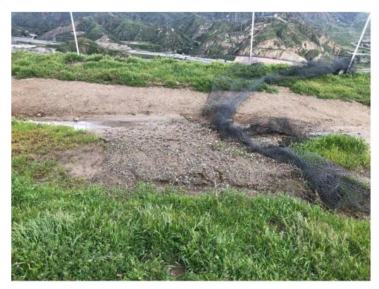
Sediment debris trapped by fallen trash net
