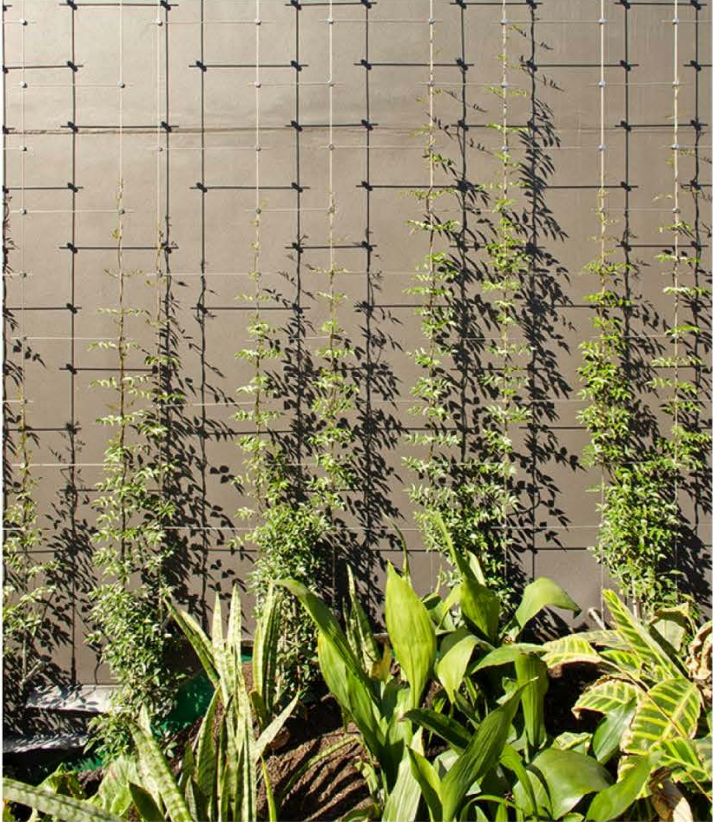
GREEN SCREEN WITH JACOB CABLE SYSTEM FOR LANE FACADE
