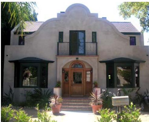
A house with wood siding should not be stuccoed over. Stucco is appropriate on a home in this architectural style, Mission Revival.
