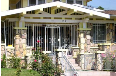
The security bars added to this porch obscure its historic character.
