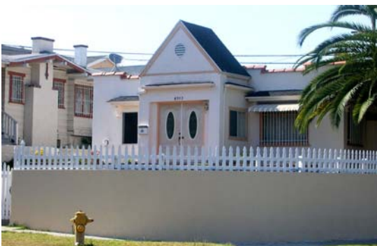
Solid fences in the front yard are inappropriate and block views of the structure.
