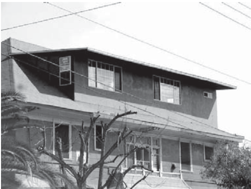
This rooftop addition is inappropriately located on the front of the house.
