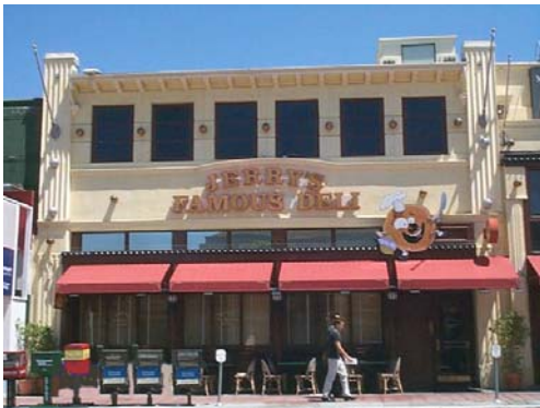
The parapet and other architectural details on this building help break up its physical bulk.
