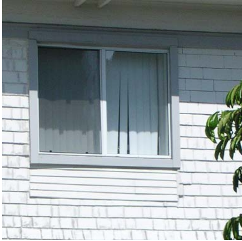
It is inappropriate to replace wood siding with siding that does not look the same as the original. It is important to use the same kind of wood, and to match the original in size, profile, and finish.
