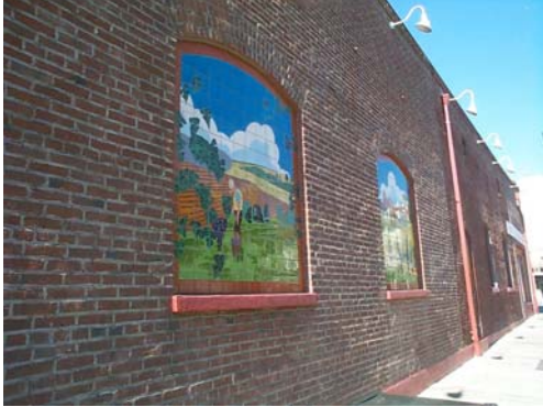
These guidelines encourage externally illuminated signs and buildings, utilizing lights such as goose neck lights.
