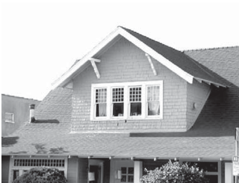
A second story dormer roof element.
