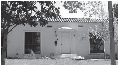
This door destroys the historic character of the home.
