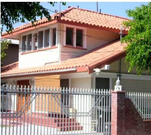
Inappropriate materials can also destroy the historic character of a structure. In this case, clay tiles should not be used on a Craftsman style home.
