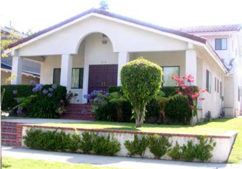
This front yard addition destroys the historic character of the main structure. Additions should always be placed at the rear of structures.
