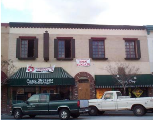
Multi-pane windows were common on the upper floors of commercial buildings.
