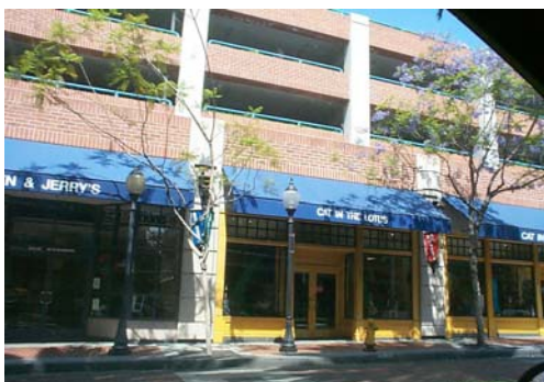
Designing the ground floor of a structure as retail, and placing parking above enlivens the street.
