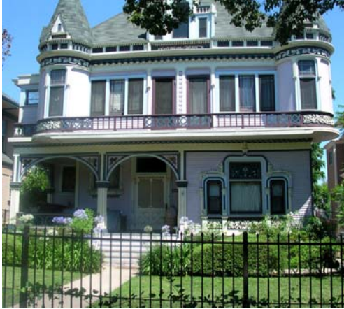
This home has decorative wood work, siding, and intricately carved arches and columns.
