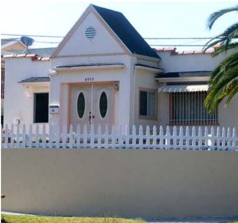
The porch addition with the pitched roof does not echo the flat roof of the main structure. Additions should never obscure the original building.
