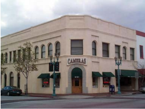
This building utilizes the same height and bulk of the adjacent building. The architecture also breaks up the building with awnings and storefront bays.
