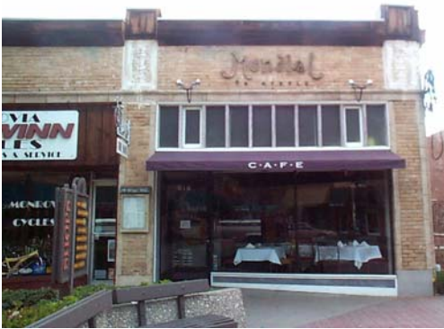
The flat roof with decorative cornices help unify the group of diverse storefronts.
