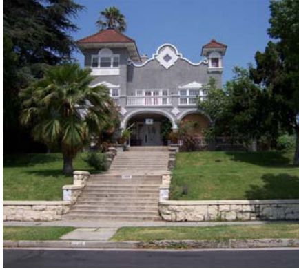
Topography helps define this home's character and should be retained. The mature trees in the front yard are another important element and should be retained.
