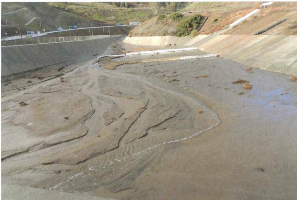
Photo 2: Sediments accumulation in terminal basin
