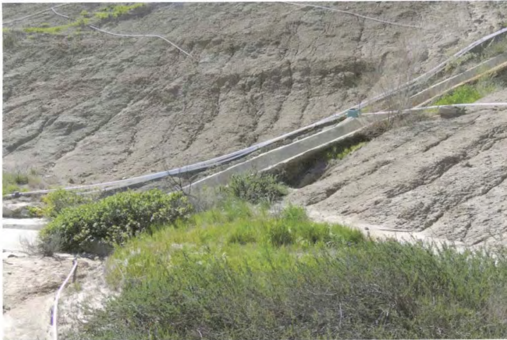
Photo 10: Erosion along edge of downchute at coastal sage mitigation area
