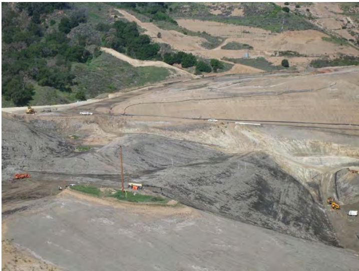
Photo 67: Site Grading South of Basin A: March 9, 2016
