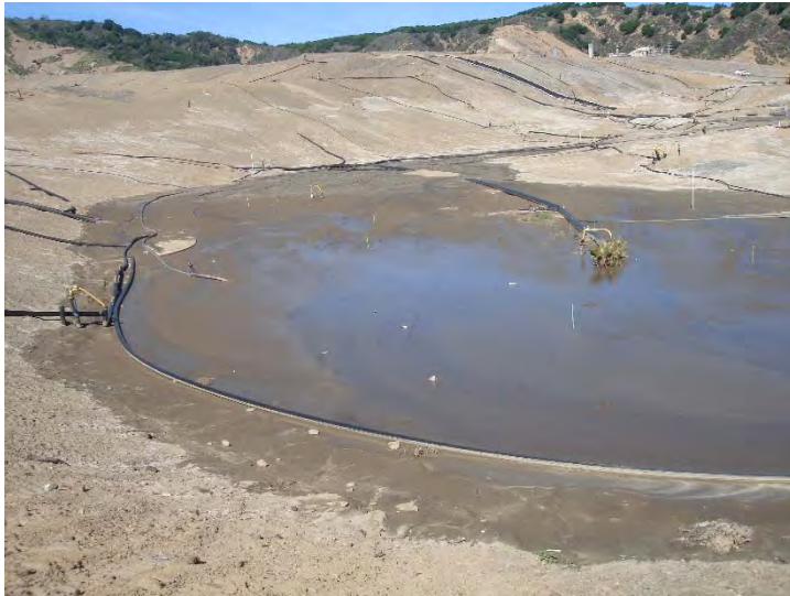
Photo 365: Ponding on City Top Deck: March 9, 2016
