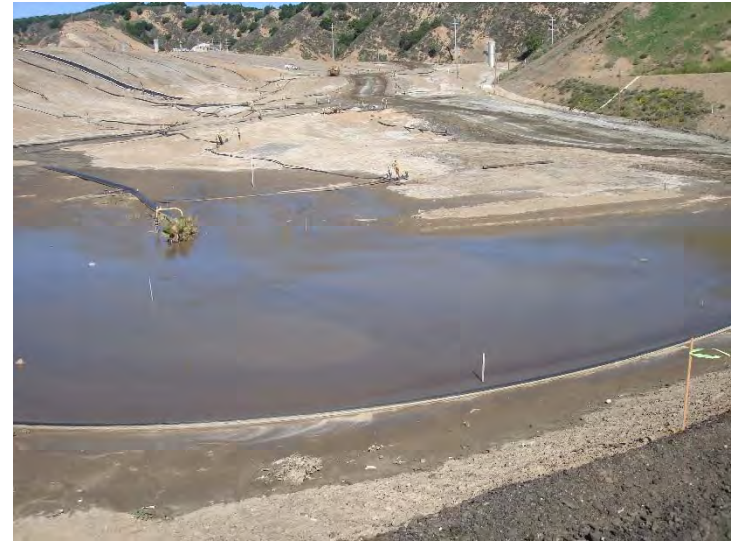
Photo 366: Ponding on City Top Deck: March 9, 2016
