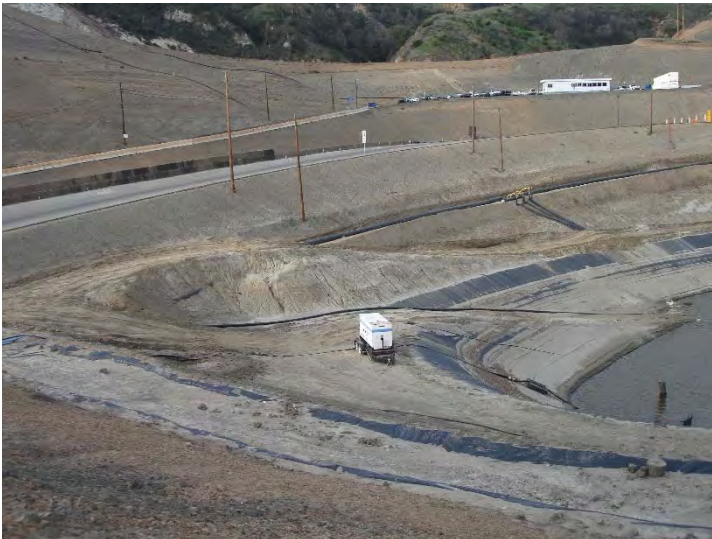
Photo 83: City Lined Drainage Lift Area: January 27, 2016
