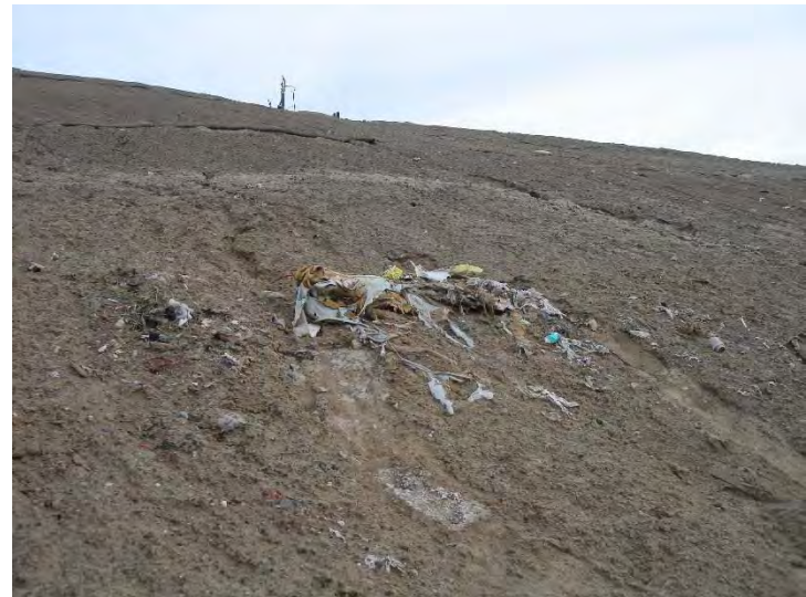
Photo 332: County South Slope Inert Waste Exposed: January 27, 2016
