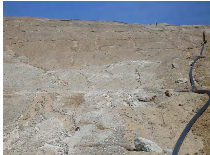
Photo 356: City Slope Erosion, Inert Waste Exposed: February 24, 2016
