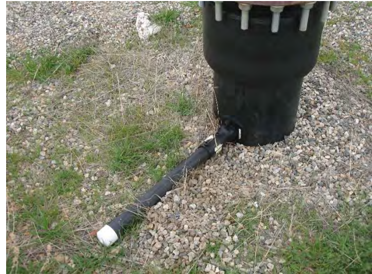
Photo 158: Flare 8 Vacuum Leak: January 27, 2016
