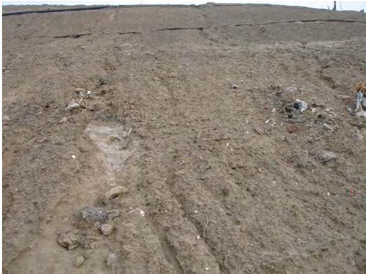
Photo 331: County South Slope Inert Waste Exposed: January 27, 2016
