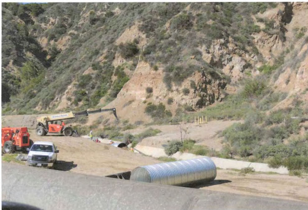
Photo 3: New CSP between Basin D and access road to Flare 9-10
