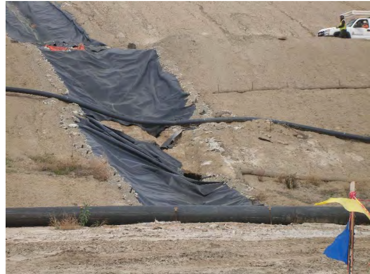
Photo 330: County South Slope Drainage Failure: January 27, 2016
