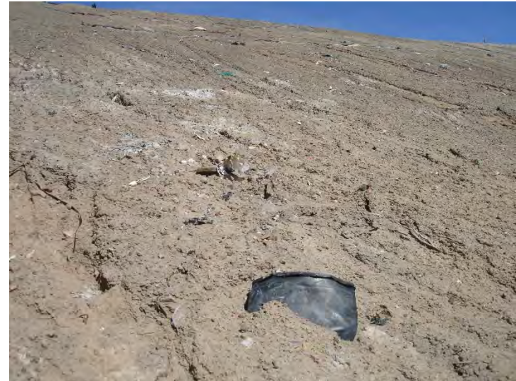
Photo 358: City Slope Erosion, Inert Waste Exposed: February 24, 2016
