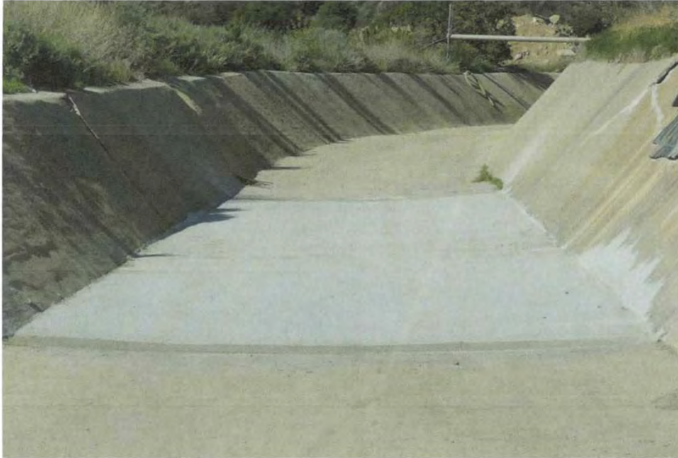
Photo 1: repaired bottom of channel between Basin A and Basin D
