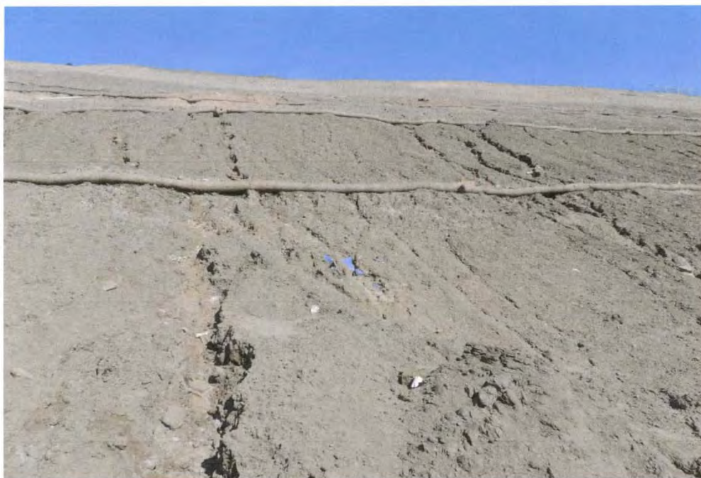
Figure 4: Erosion gullies on side slope at Cell II
