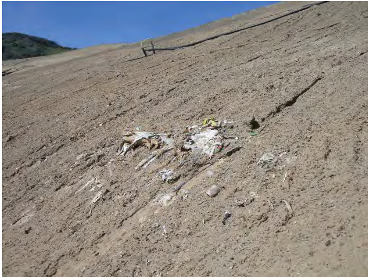
Photo 357: City Slope Erosion, Inert Waste Exposed: February 24, 2016
