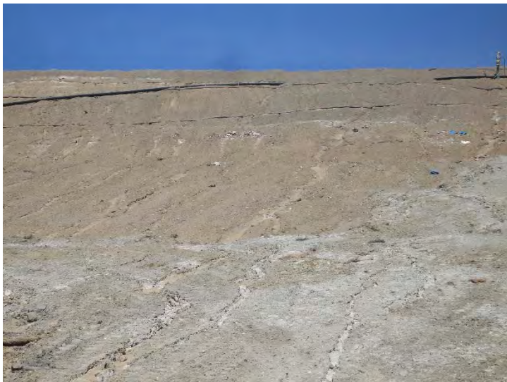
Photo 355: City Slope Erosion, Inert Waste Exposed: February 24, 2016
