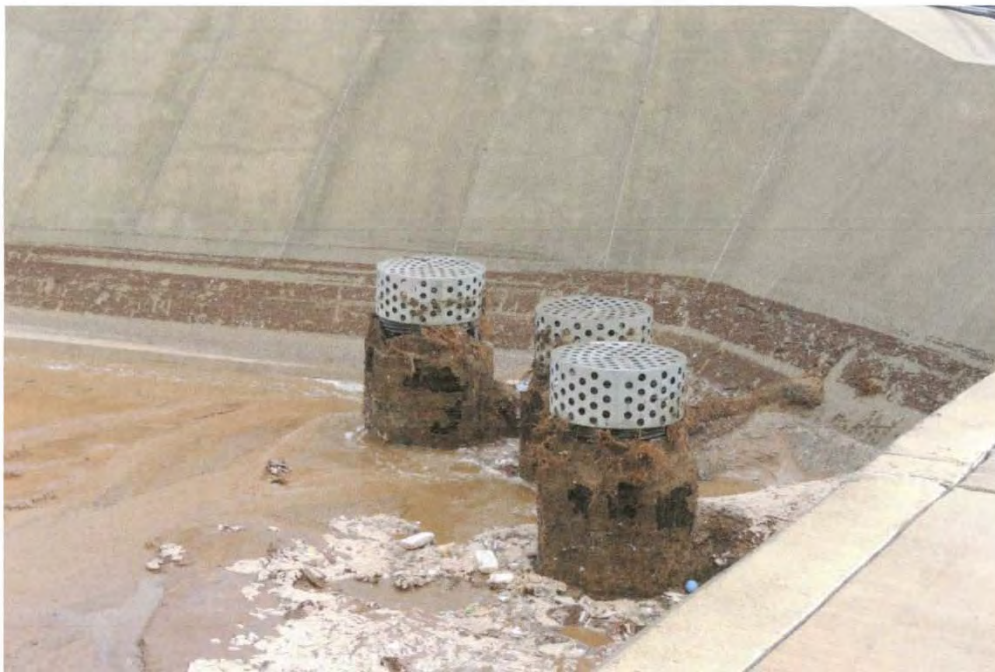
Figure 4: Risers in Terminal Basin
