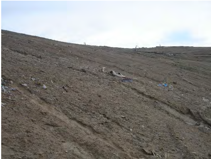
Photo 333: County South Slope Inert Waste Exposed: January 27, 2016
