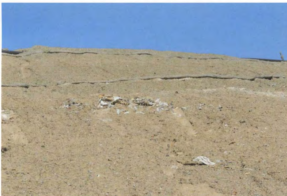
Photo 6: Inert waste showing on southeast facing slope of old county landfill
