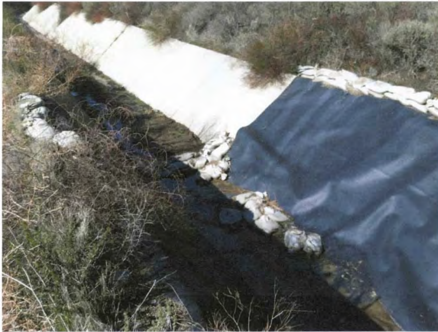
Photo 9: Geomembrane liner at beginning of lined portion between Basin D and Flare 9-10 access road
