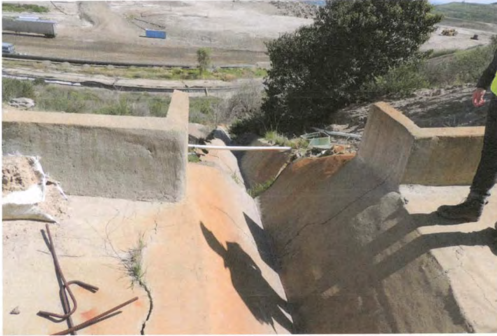
Photo 9: Crack in downchute at coastal sage mitigation area
