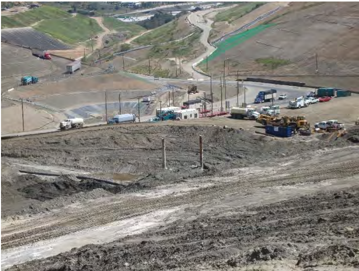
Photo 75: Oil Well Casings to be Abandoned: March 23, 2016
