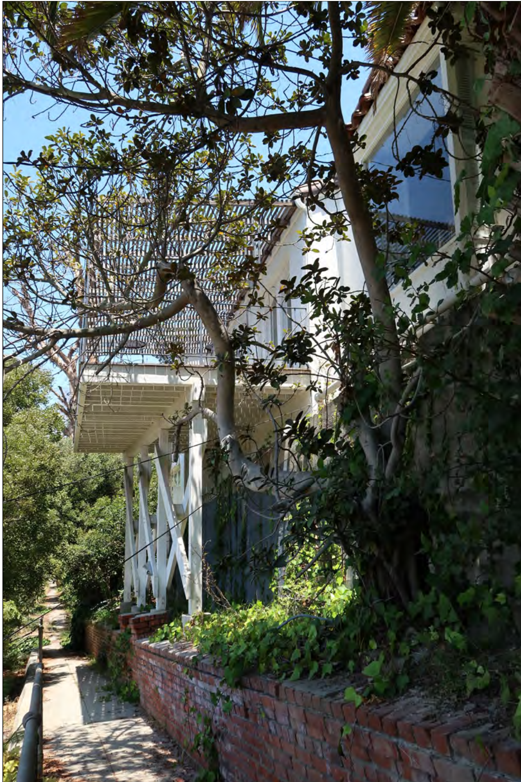
Photo 5: 145 Adelaide Drive, north elevation of residence, view east. Note abandoned public stair and walkway (bottom left) (Chattel, 2018)
