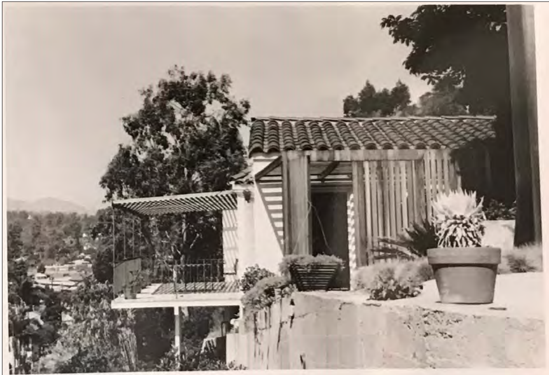
Image 12: 145 Adelaide Drive, residence, view northeast (Huntington Library, 1963)
