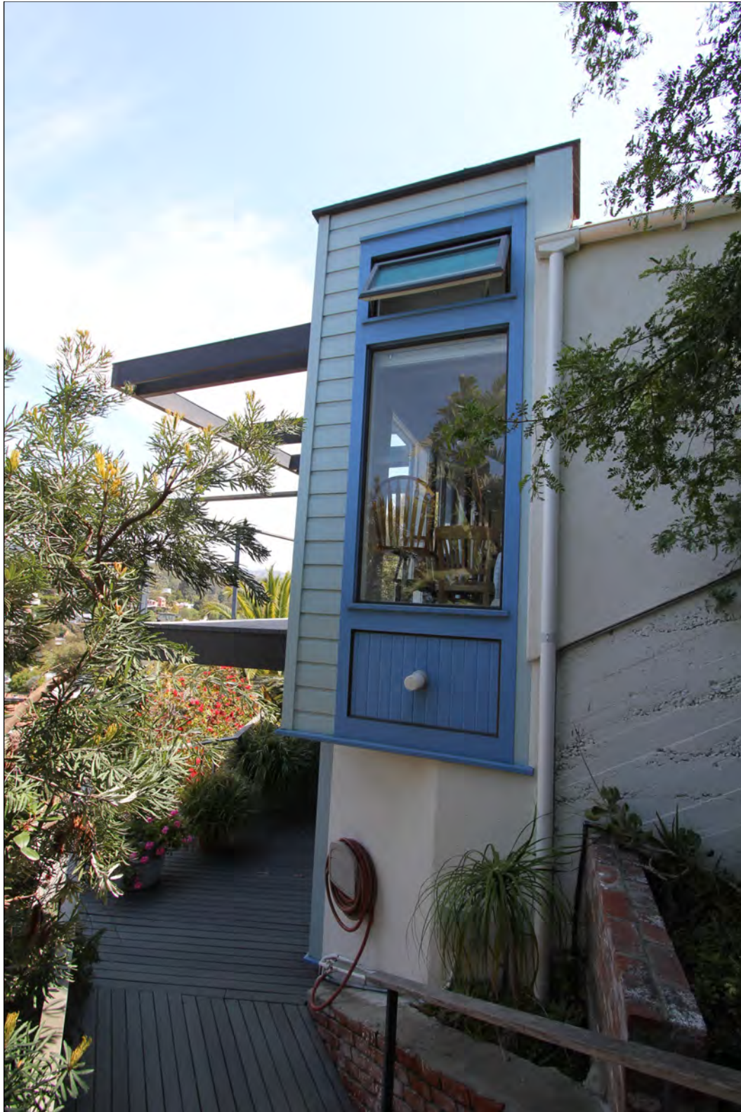
Photo 11: 145 Adelaide Drive, west elevation of studio, view east (Chattel, 2018)
