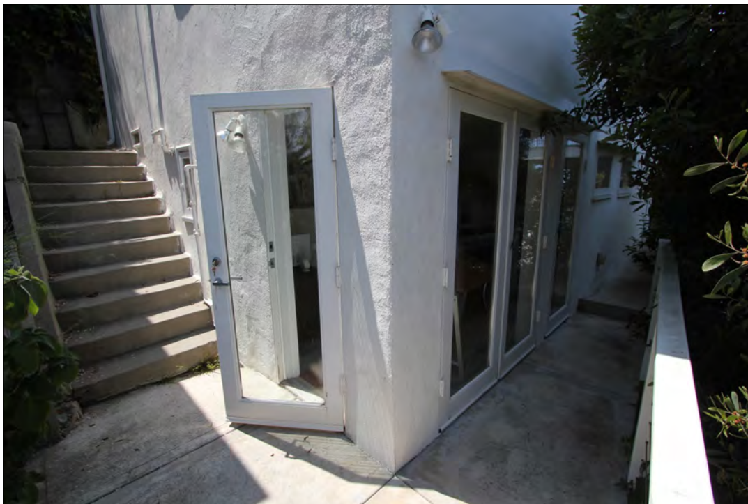
Photo 19: 145 Adelaide Drive, north and east elevations of residence, view southwest. Note the outside access to altered bedroom and bathroom at the tall basement crawlspace (Chattel, 2018)
