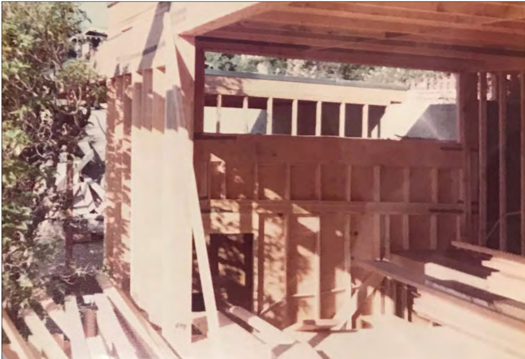
Image 30: 145 Adelaide Drive, construction of studio addition (Huntington Library, 1976)
