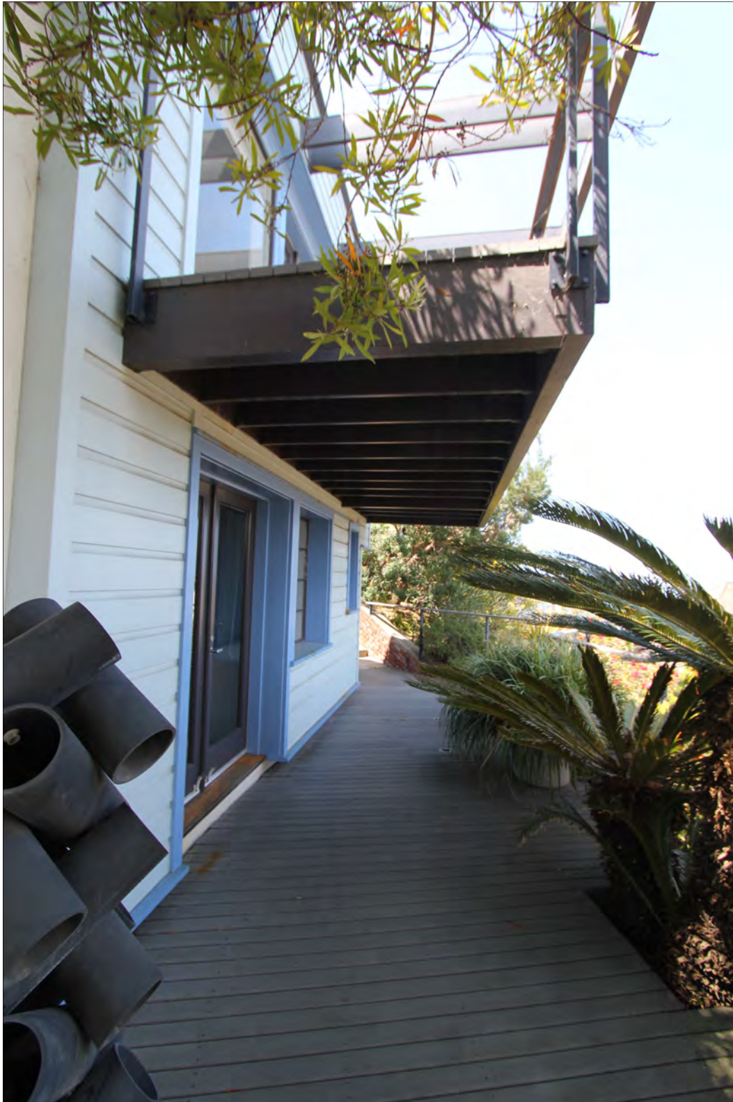
Photo 12: 145 Adelaide Drive, north elevation of studio, view west (Chattel, 2018)
