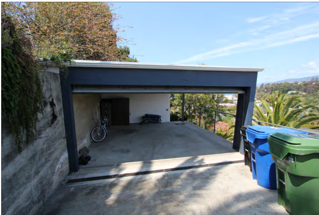
Photo 7: 145 Adelaide Drive, carport and stairway that leads to the residence and studio, view west (Chattel, 2018)
