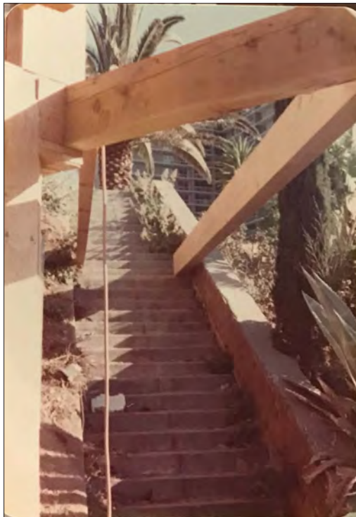
Image 35: 145 Adelaide Drive, construction of studio addition (Huntington Library, 1976)
