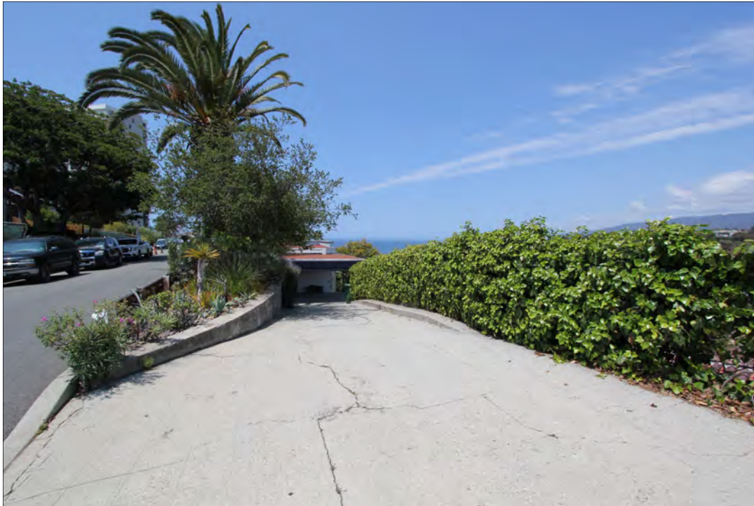
Photo 6: 145 Adelaide Drive, driveway and carport, view west (Chattel, 2018)
