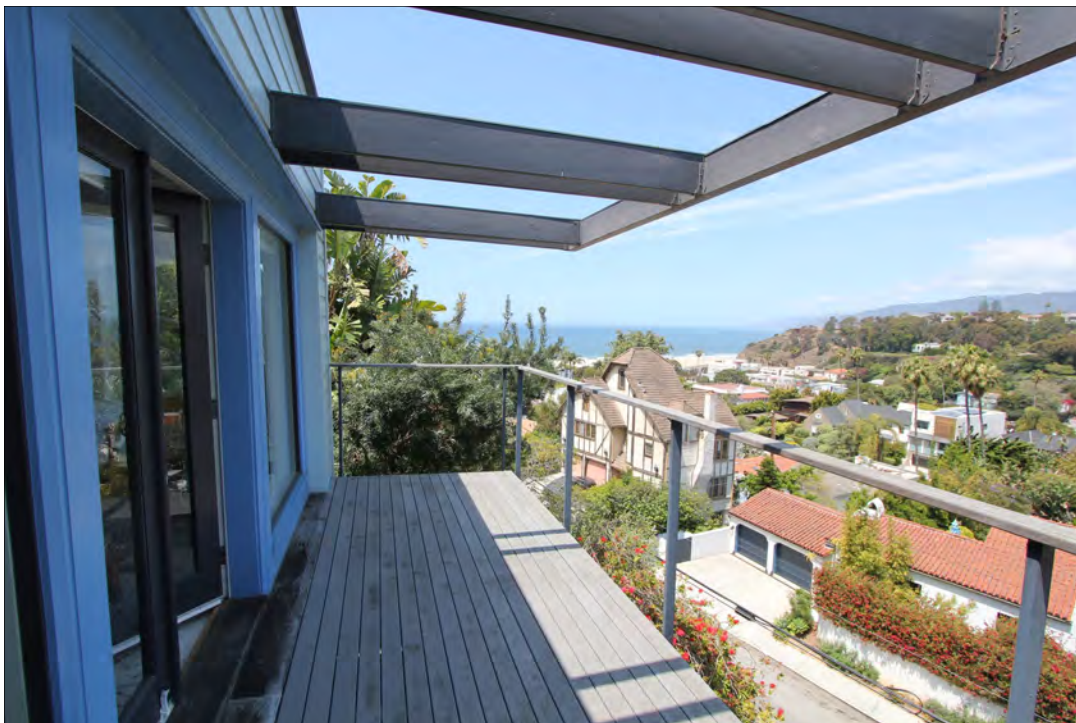
Photo 32: 145 Adelaide Drive, second floor, north elevation of studio, view northwest (Chattel, 2018)
