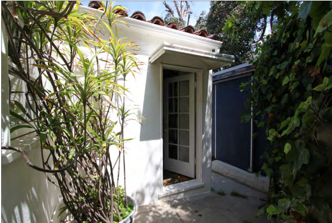
Photo 18: 145 Adelaide Drive, south elevation of residence, view northeast (Chattel 2018)
