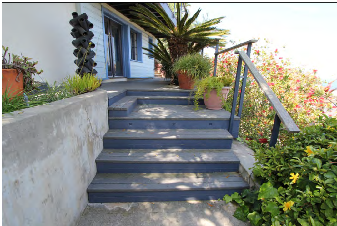
Photo 14: 145 Adelaide Drive, north elevation of studio, view west (Chattel, 2018)
