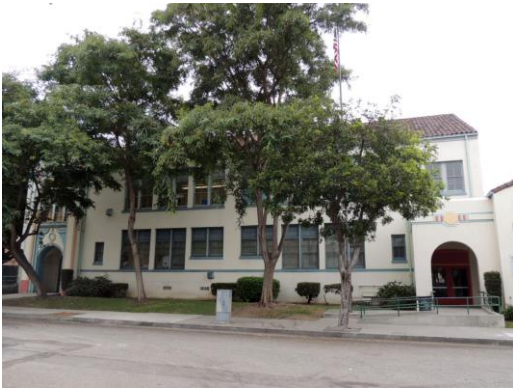
Address: 1000 S. Grattan St. Name: 10 th Street Elementary School Date: 1922
