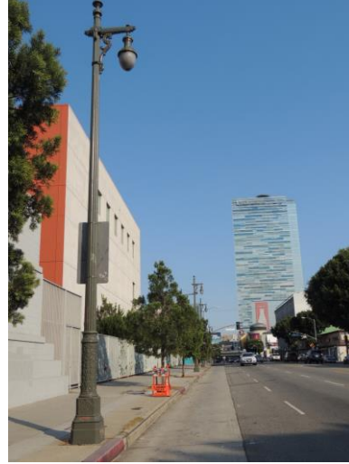
Location: Olympic Bl. between Hoover St. and 110 Freeway Name: Olympic Boulevard Streetlights Date: circa 1930
