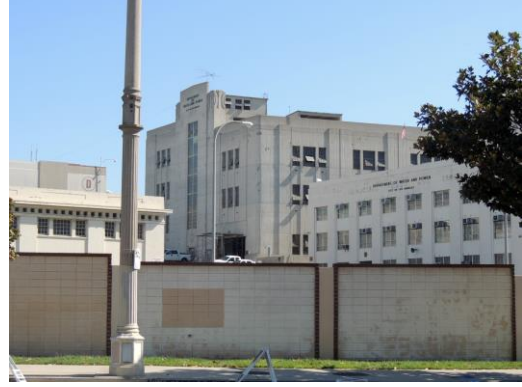
Location: Bounded by 1 st St., Beaudry Ave., 2 nd St., Bixel St. Name: DWP, Boylston Facility Date: 1910-present
