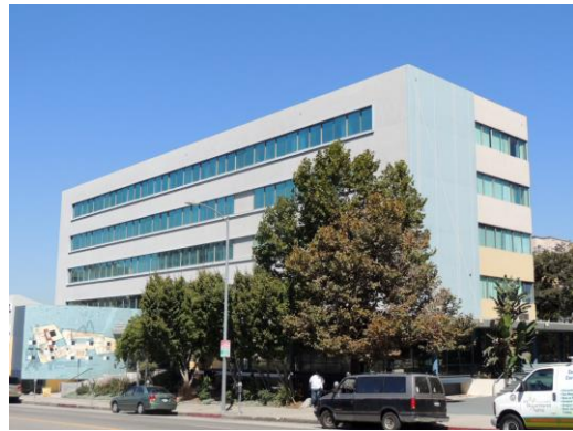
Address: 1125 W 6 th St. Name: Kidney Center of Los Angeles Date: 1955 Architect: Kistner, Wright & Wright
