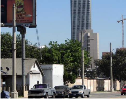
Location: 2 nd St. between Beaudry Ave. and the Beverly Bl. Bridge; Glendale Ave. to Rockwood St. Name: 2 nd Street Streetlights Date: circa 1925
