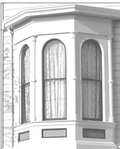
Rounded-top double-hung wood bay windows
