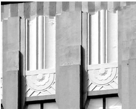
Concrete detail like this should not be cleaned with aggressive abrasive methods, or the detail may be lost.
