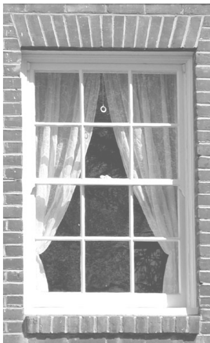
Six over six wood double-hung window
