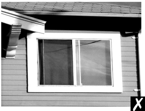
These sliding aluminum replacement windows are inappropriate.
