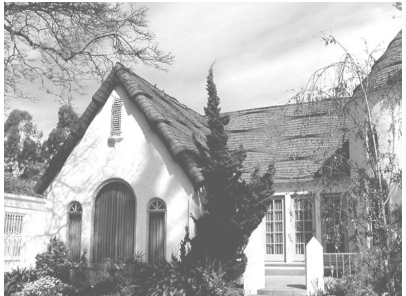
Built-up faux thatch shingle roof
