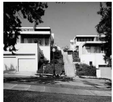
Richard J. Neutra's Strathmore Apartments in Westwood, built in 1937, are an example of the cutting-edge early International Style.
