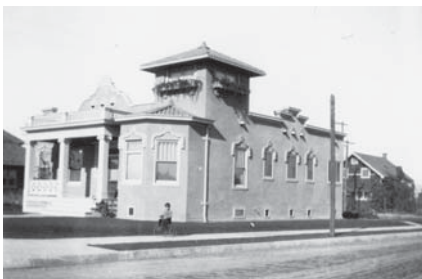
Mission Revival residence at Arlington Ave & 21st Street, displaced by Santa Monica Freeway.
