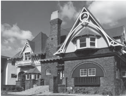
Fitzgerald Mansion located at the corner of Arlington Avenue and Adams Boulevard.
