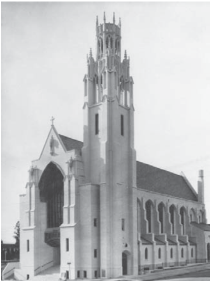
Exterior view of McCarty Memorial Christian Church, located at 4101 West Adams Boulevard in Los Angeles.
