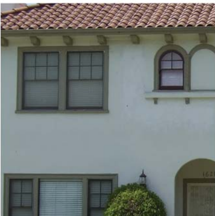
Flush, frameless, and oddly arranged windows may be inappropriate on a new house.
