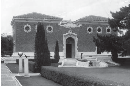
Library on the grounds of the mansion of William A. Clark, Jr. on West Adams. This later became the Williams Andrews Clark Memorial Library at 2520 Cimarron (at Adams). The library was gifted to UCLA. Architect: Robert Farquhar. Photo dated: June 15, 1934.
