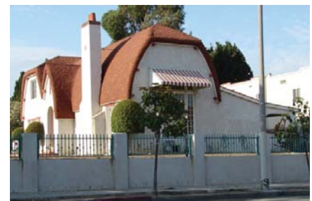
The pitch, rolled-eaves, brackets, and unique materials are all components of this roof that should be preserved.
