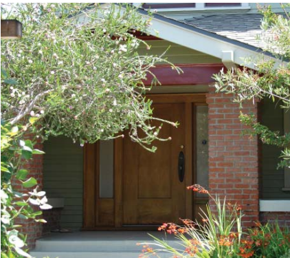
The brick masonry porch columns are left to display their natural finish quality.
