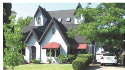
This second-story addition, with its noticeable dormers, calls attention to itself, overwhelming the original cottage.
