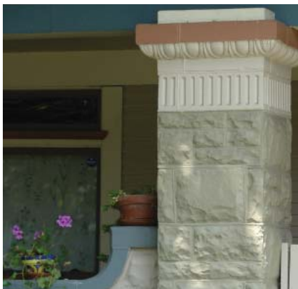
Stone column should remain unpainted, but if painted the color should match as close as possible the original stone color..
