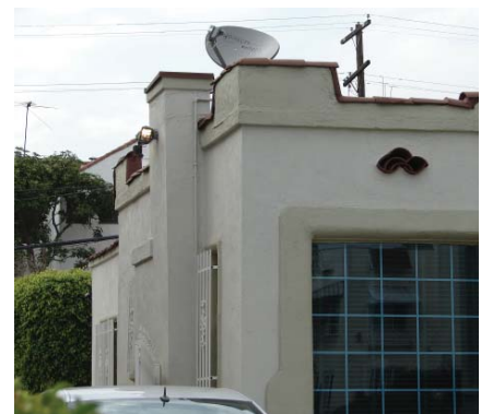
Television antennae and satellite dishes create an unnecessary visual obstruction and should be placed out of sight-
