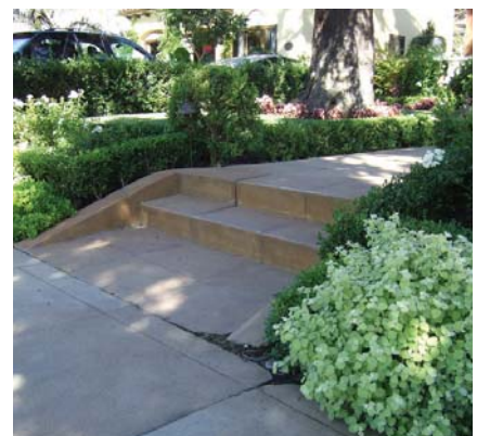
A typical front walkway and steps are shown. Concrete colors and score patterns should be carefully preserved.
