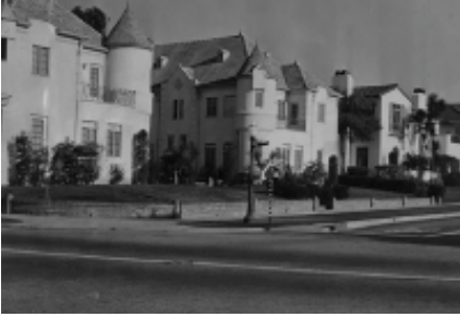
Small retaining walls are not uncommon in the HPOZ. Attention should be paid to the wall materials and decoration.
