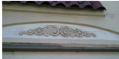
Standard 5a example. Original terracotta detailing should be preserved.
