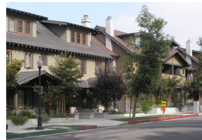
Standard 6a-7a example. Example of well-articulated new construction.
