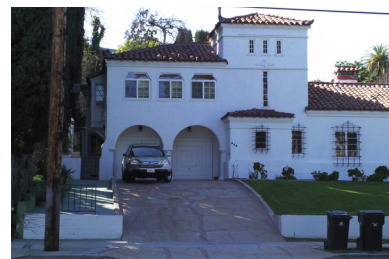
Standard 7f example. The third floor of this home does not occupy more than 75% of the second floor.
