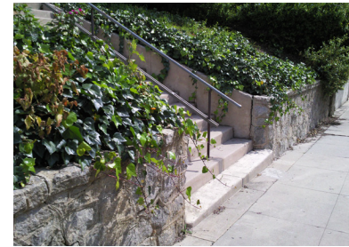
Standard 1d example. Historic retaining wall.
