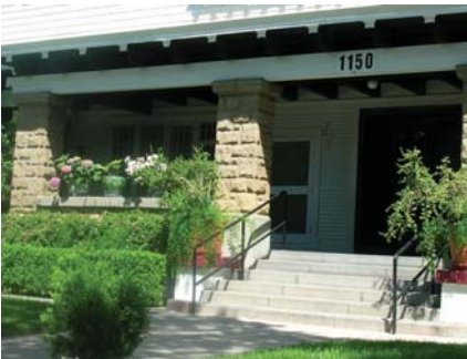
The sandstone porch columns are left to display their natural finish quality.
