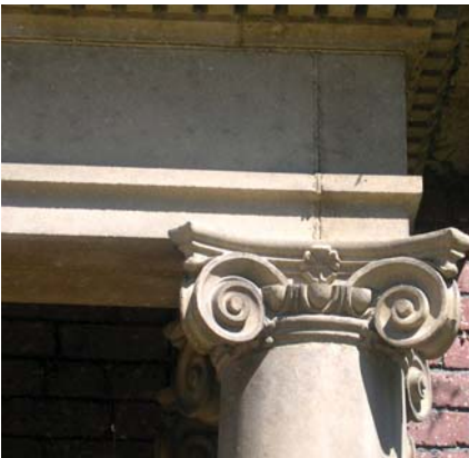
Ionic column details are shown on this Classical Revival building.
