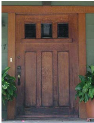
This Craftsman style door shows off a rustic wood finish, original hardware and a rectilinear design.
