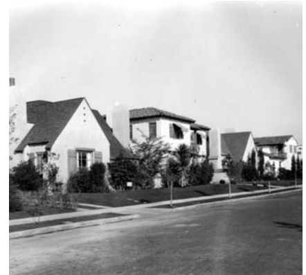
The Eclectic Revival (or Period Revival) movement presents a number of romantic building styles to this single streetscape.
