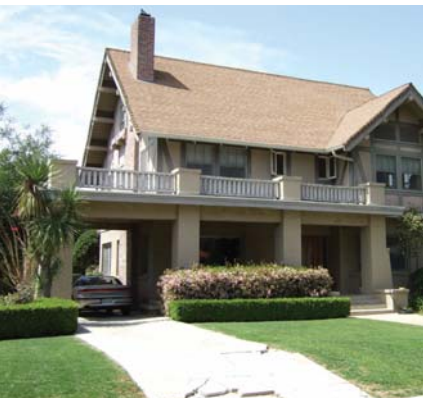
The porch, porte-cochere and balcony are a prominent feature on this Tudor-Craftsman house.
