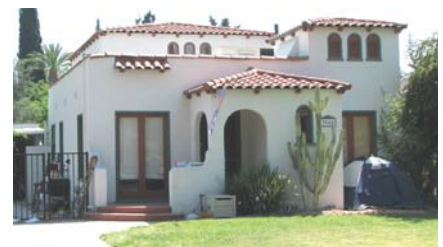
This second-story addition is set-back and preserving the look and scale of the original bungalow.
