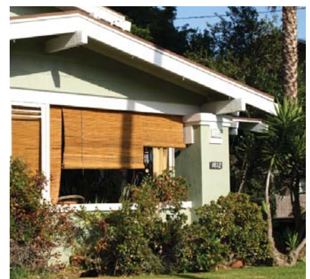
Non-permanent devices such as this bamboo screen may effectively screen a porch without altering the home and disrupting the streetscape.
