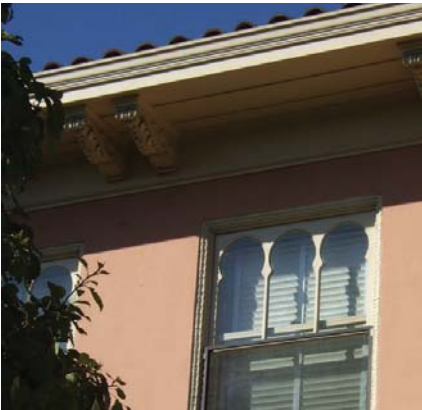
Smooth, hand-troweled stucco is an appropriate finish for this Italian Renaissance Revival home.
