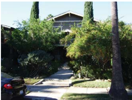
Overly-dense landscaping can obscure views of both the house and the greater streetscape.
