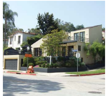
Though different in style, this house's deep, and vertical openings help it to blend with its neighbors.
