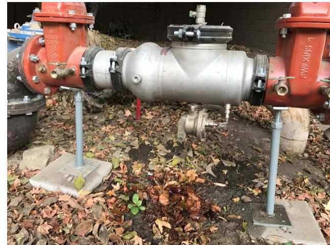
Photo 248: Potable Water Leak in Graywater Handling area: October 11, 2016
