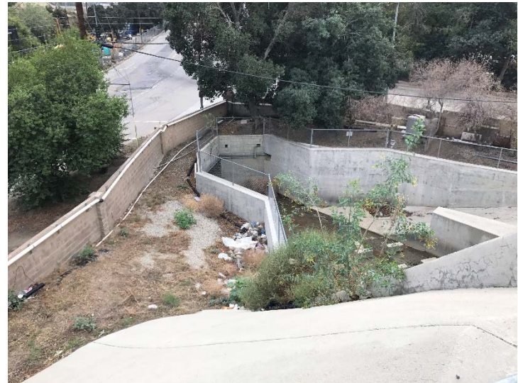
Photo 208: Vegetation in Concrete on Terminal Basin Wall: November 1, 2016
