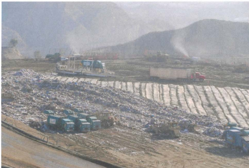
Photo 6: Placement of waste at CC3
