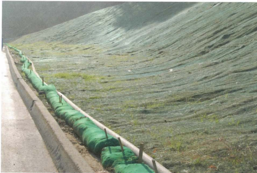
Photo 8: Grass growing through erosion protection system
