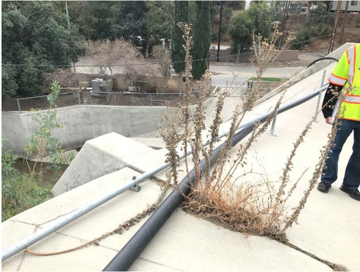
Photo 209: Vegetation in Concrete on Terminal Basin Wall: November 1, 2016
