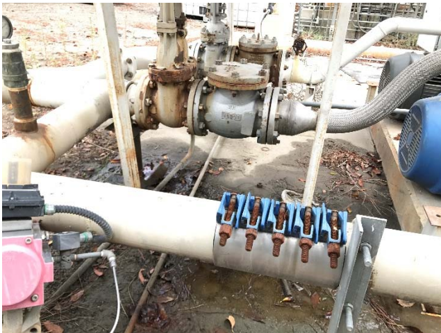
Photo 251: Potable Water Leak in Graywater Handling area: October 11, 2016
