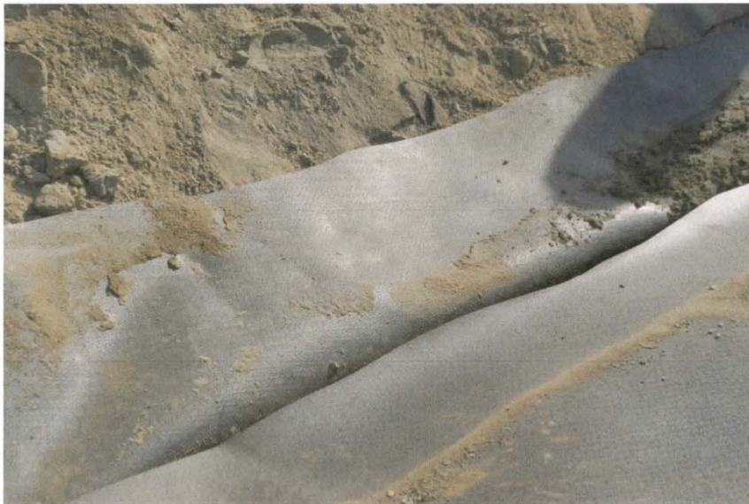
Photo 2: Connection of CC3 Geomembrane to CC4 Geomembrane
