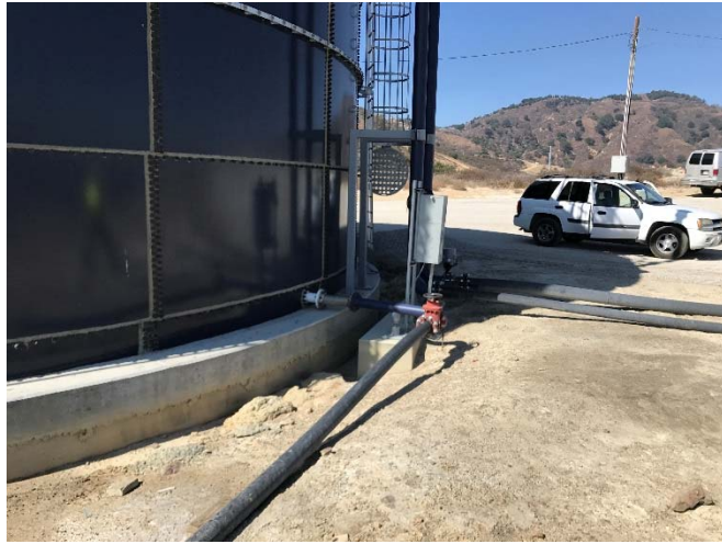
Photo 261: Deck A Water Tank Foundation Not Backfilled: October 11, 2016
