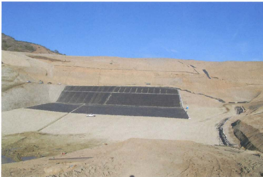
Photo 1: Liner installation at Cell CC4
