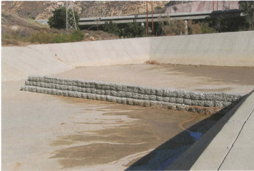
Photo 7: Gabion Structure in Terminal Basin retained fines
