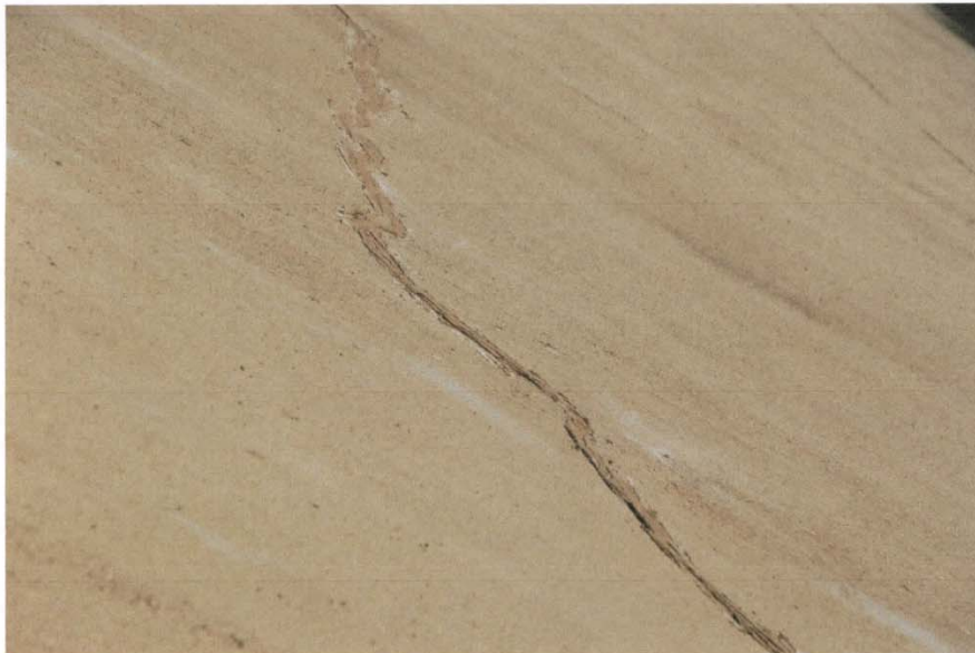
Photo 8: Cracks repaired on wall of terminal basin
