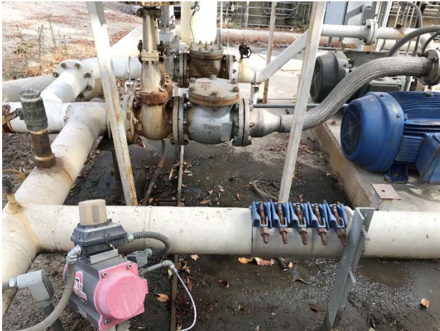
Photo 249: Potable Water Leak in Graywater Handling area: October 11, 2016
