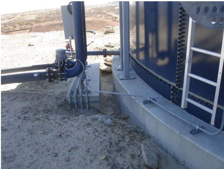
Photo 259: Deck A Water Tank Foundation Not Backfilled: October 11, 2016
