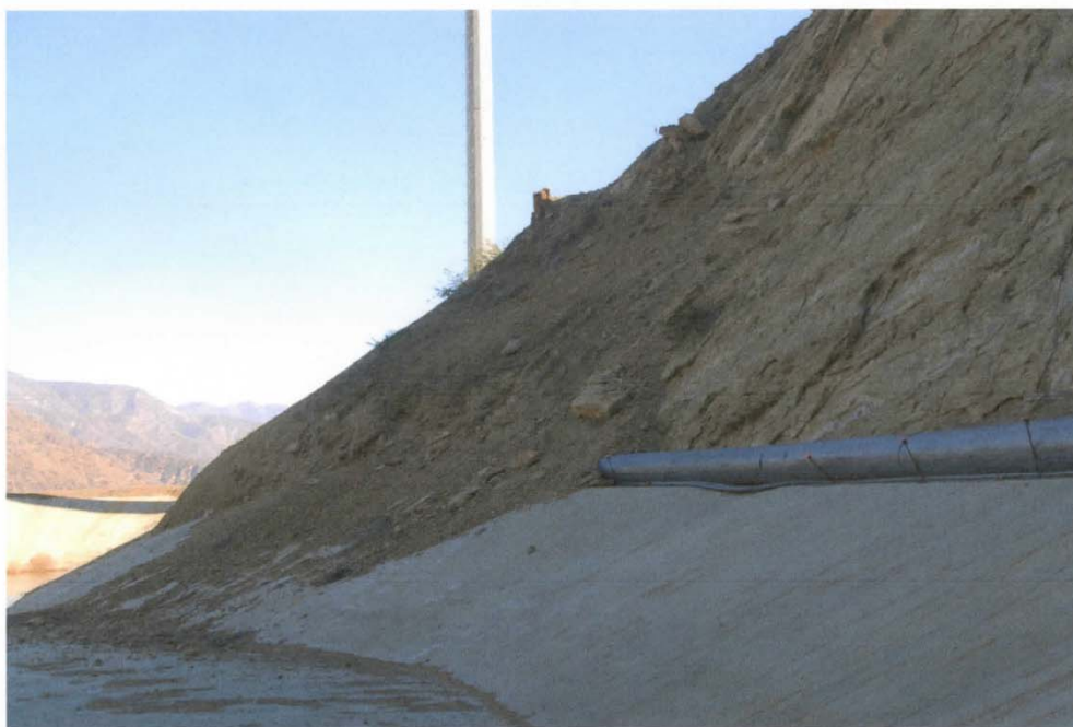
Photo 4: Basin A – little to no slough-off of soil
