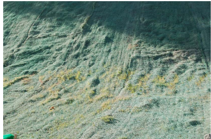
Photo 152: Seeded Slope Mat above Westside Drainage: November 29, 2016
