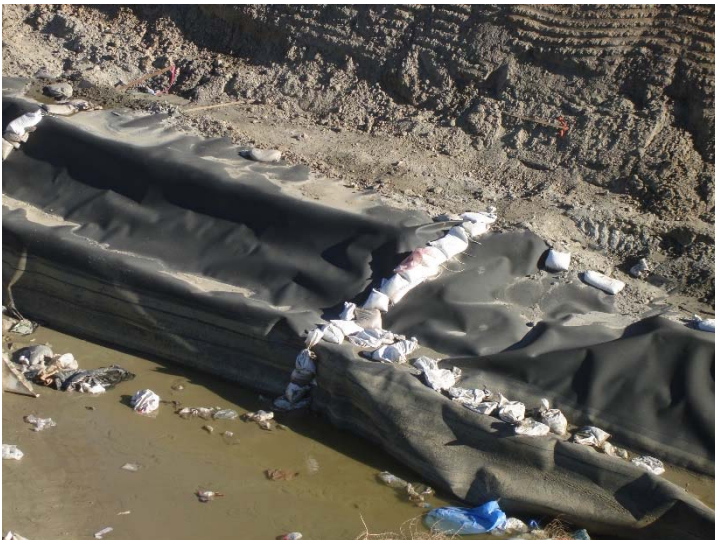
Photo 83: CC4 Liner Tie-in Area: November 29, 2016
