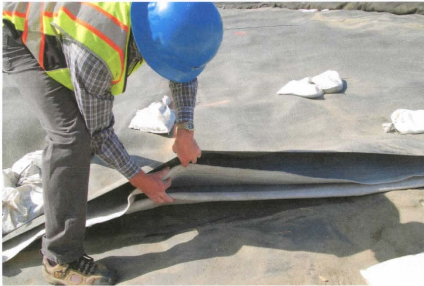
Photo 5: GCL within liner system on slopes of CC4
