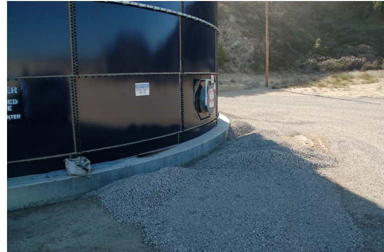
Photo 262: Deck A Water Tank Foundation Not Backfilled: December 14, 2016
