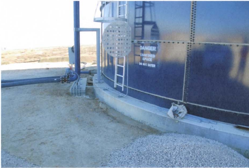
Photo 11: Trench around ring foundation of water tank
