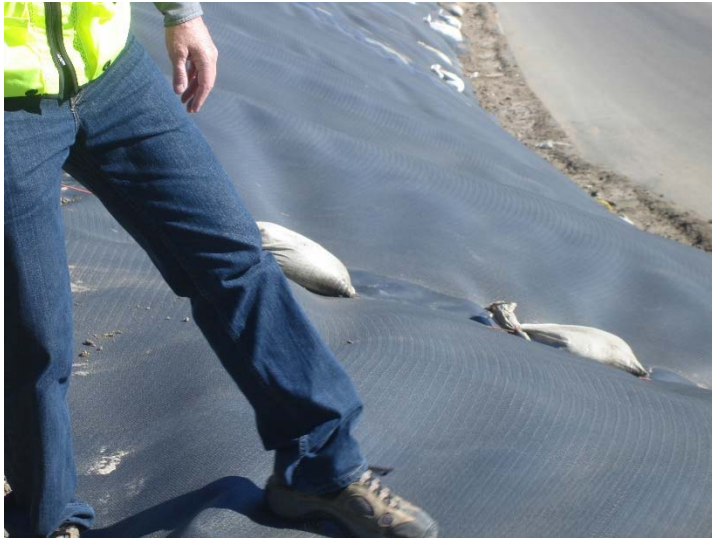
Photo 93: Slope Gas Control Liner Puffing at CC3A: November 29, 2016
