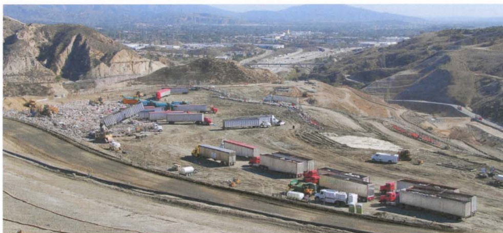
Photo 3: Waste placement in Cell CC3B – Interim cover in middle
