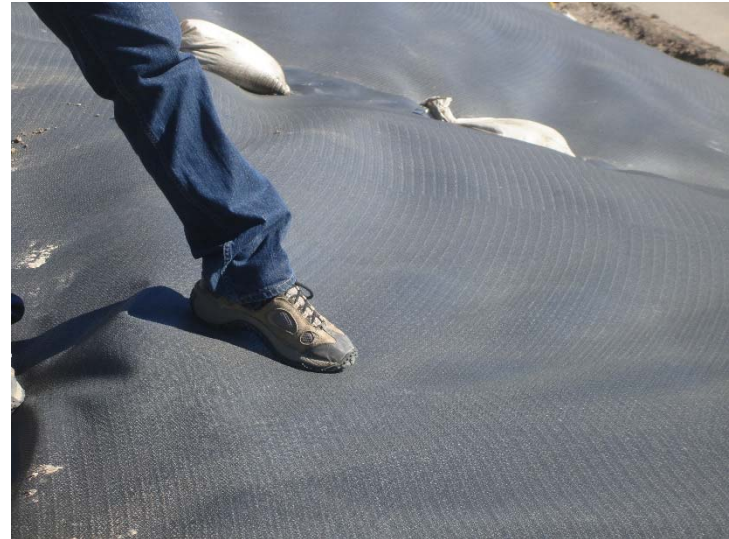
Photo 94 Slope Gas Control Liner Puffing at CC3A: November 29, 2016
