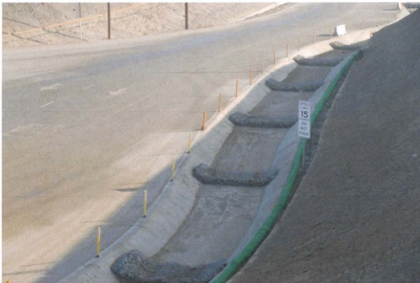
Photo 10: Gabion heads in main channel along access road
