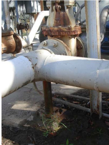
Photo 253: Potable Water Supply Piping Leak: November 29, 2016
