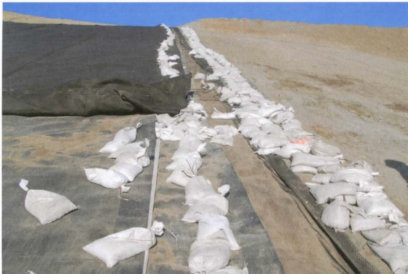
Photo 4: Liner system on slope of CC4
