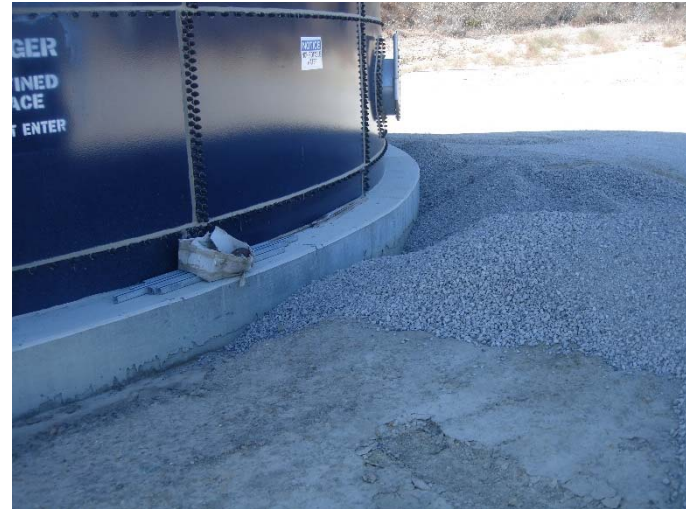
Photo 258: Deck A Water Tank Foundation Not Backfilled: October 11, 2016
