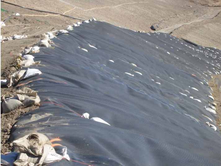
Photo 95: Slope Gas Control Liner Puffing at CC3A: November 29, 2016
