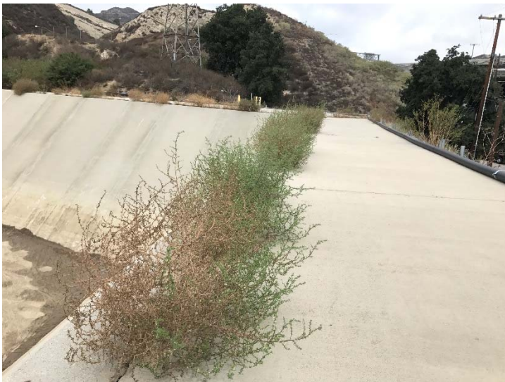
Photo 207: Vegetation in Concrete on Terminal Basin Wall: November 1, 2016
