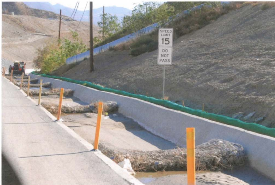
Photo 6: Gabion mats in channel along access road
