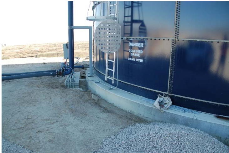
Photo 263: Deck A Water Tank Foundation Not Backfilled: December 14, 2016
