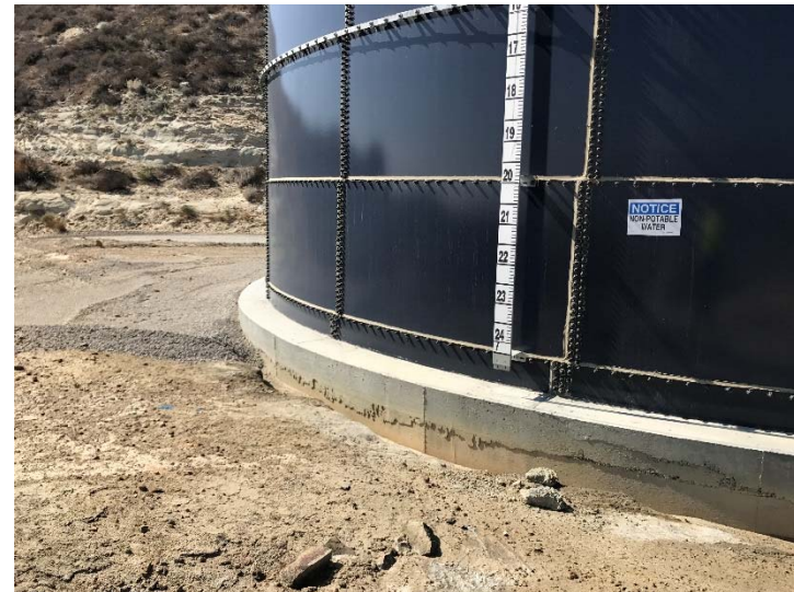
Photo 260: Deck A Water Tank Foundation Not Backfilled: October 11, 2016
