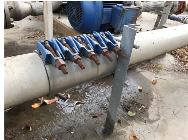
Photo 250: Potable Water Leak in Graywater Handling area: October 11, 2016
