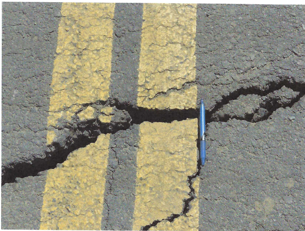
Figure 4: second crack on access road to administration pad: Horizontal offset
