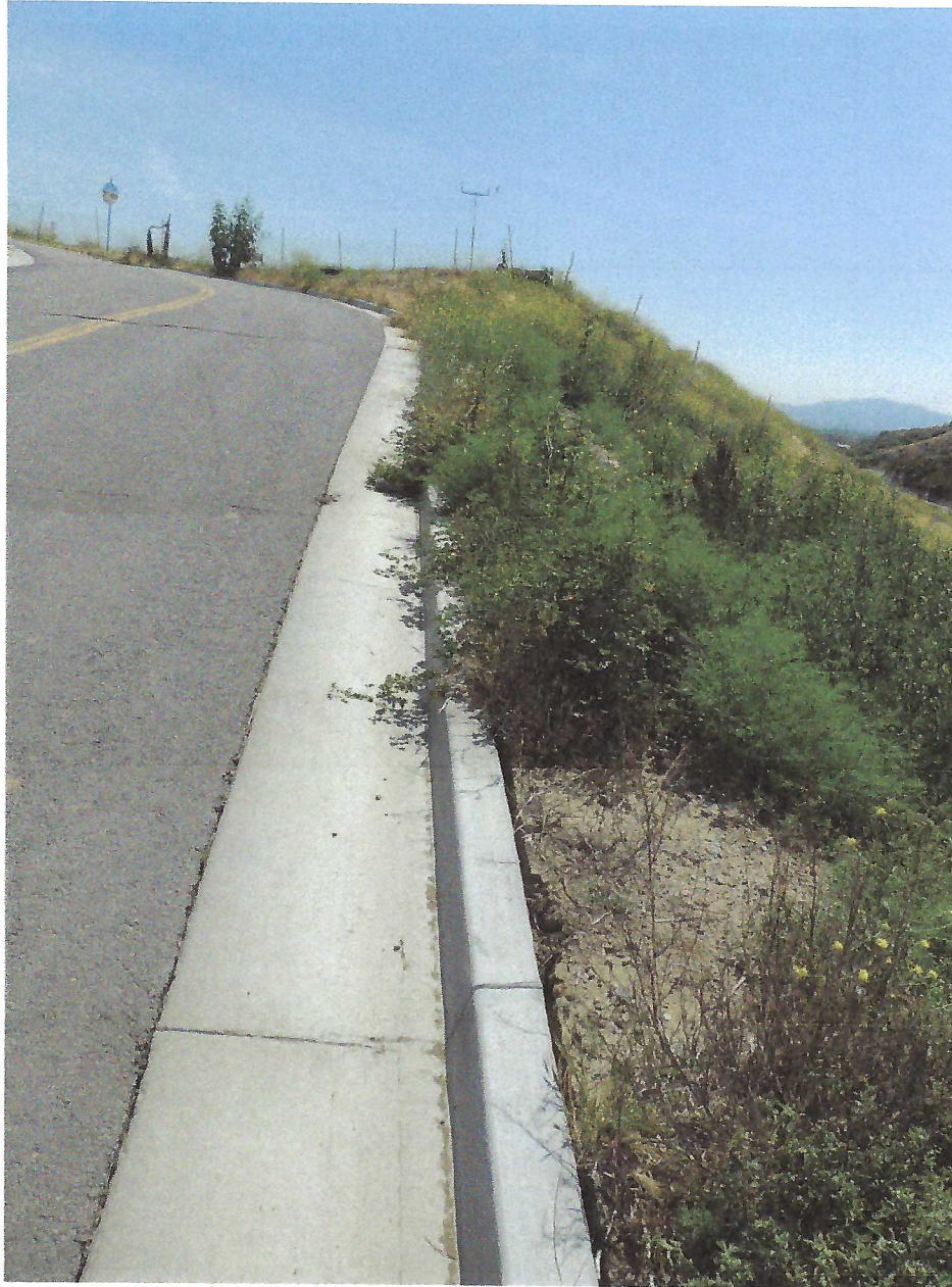
Figure 5: Access road to administration pad: soil separating form curb
