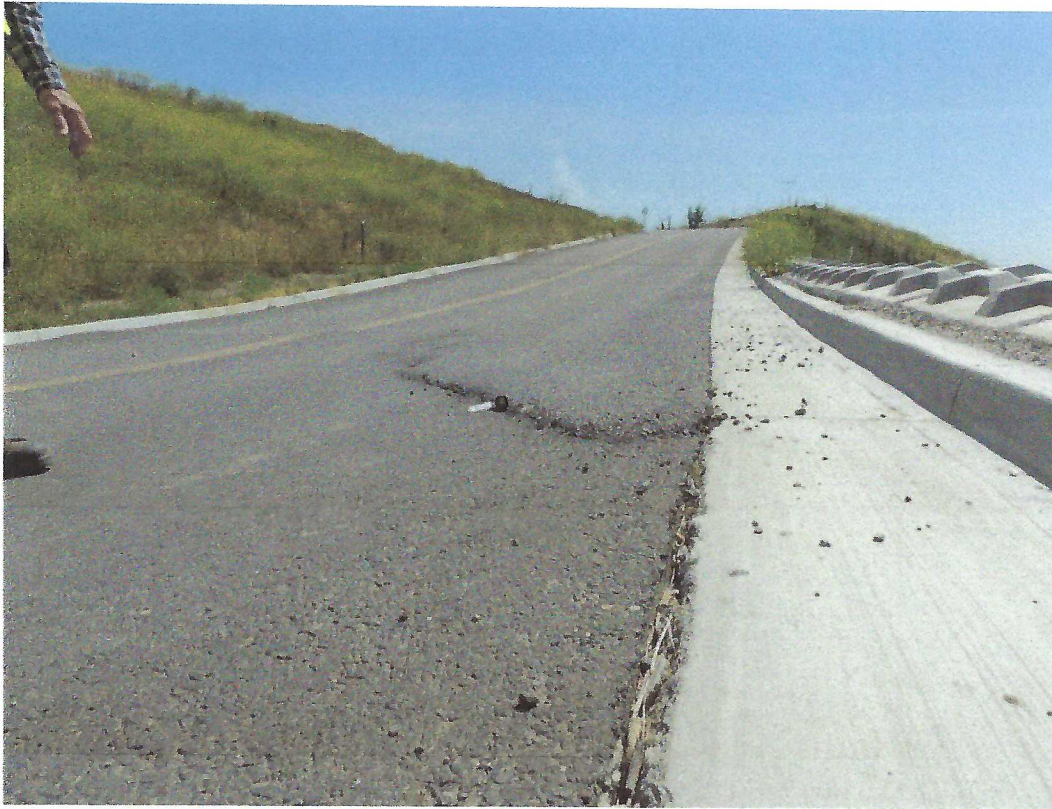
Figure 1 : First crack on access road to the administration pad
