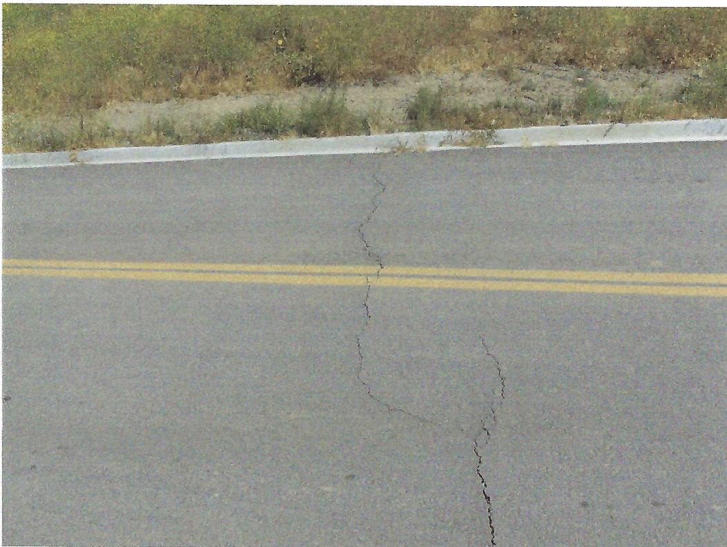
Figure 2 :Second crack on access road to the administration pad
