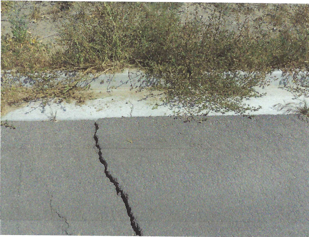
Figure 3 : Second crack on access road to the administration pad, extending through curb
