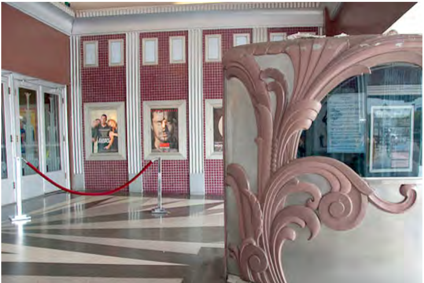
Entry vestibule. The Art Deco fluted pilasters, fluted ceiling molding and starburst-patterned terrazo n floors are original to the 190 theater. The maroon tiles and glass doors date to the 1986 Cineplex Odeon remodel. (Sheri Determan 2009)
