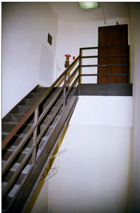
Photo 30: Second floor stairwell, view west (Chattel, 2011)
