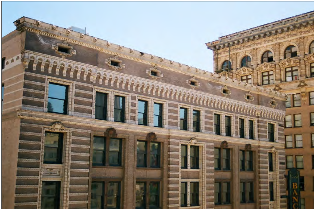
Photo 5: Detail of west façade, view southeast (Chattel, 2011)
