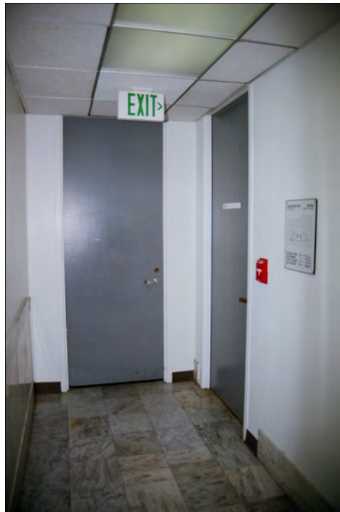
Photo 40: Third floor corridor, view west, note original marble floor and contemporary walls (at end and right) (Chattel, 2011)
