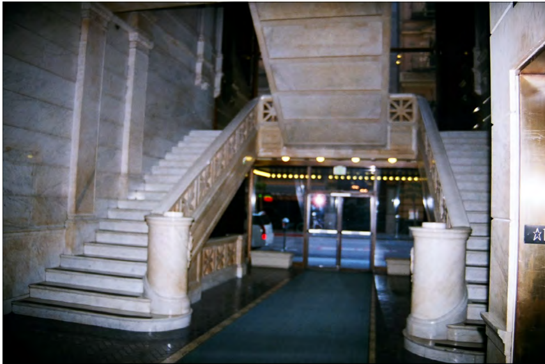
Photo 14: Lobby entrance, view south, note original marble on walls and stairs (Chattel, 2011)
