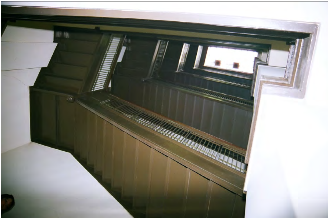
Photo 38: View upward of stairwell from third floor (Chattel, 2011)
