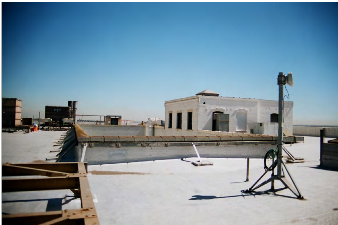
Photo 74: Roof, view east (Chattel, 2011)
