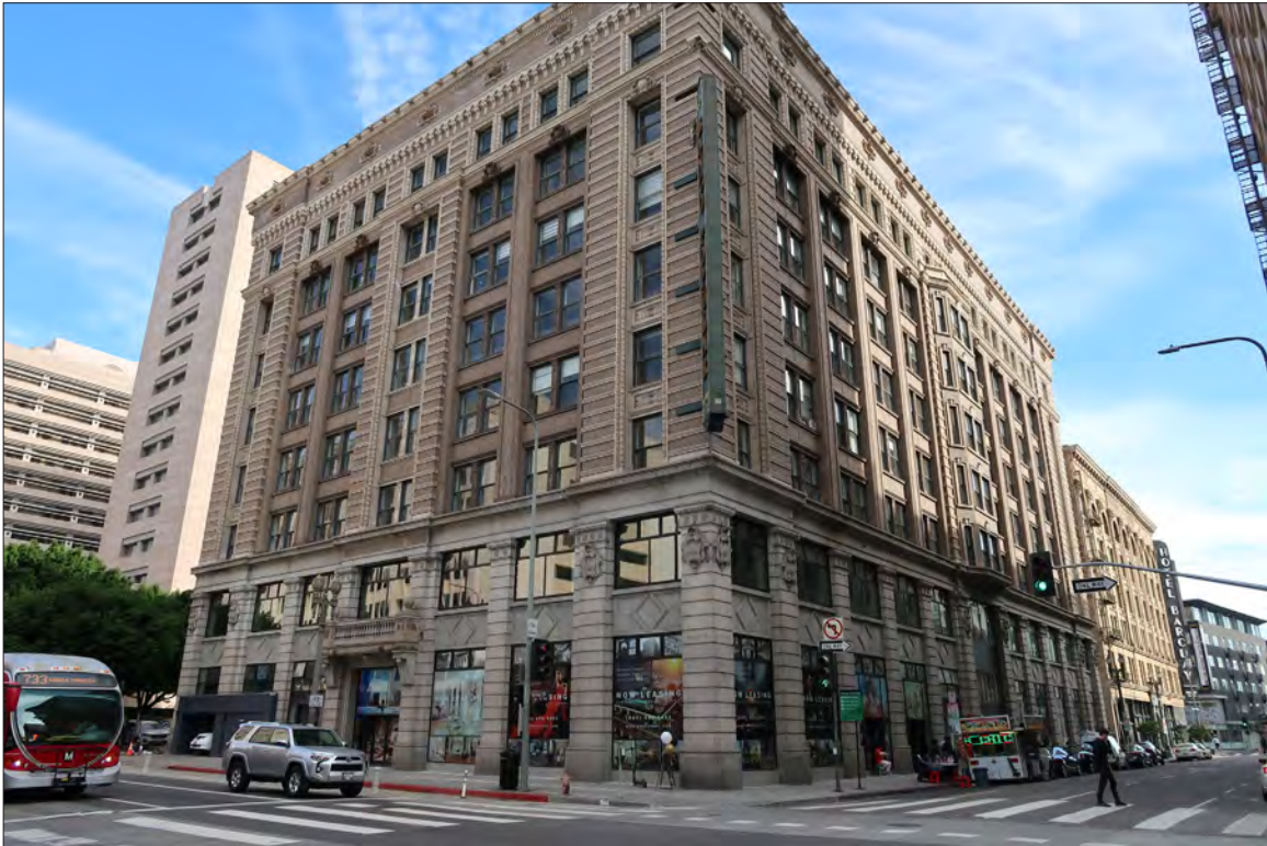
Image 2: 354 S. Spring Street, west elevation (left) and south elevation (right), view northeast (Chattel, 2019)
