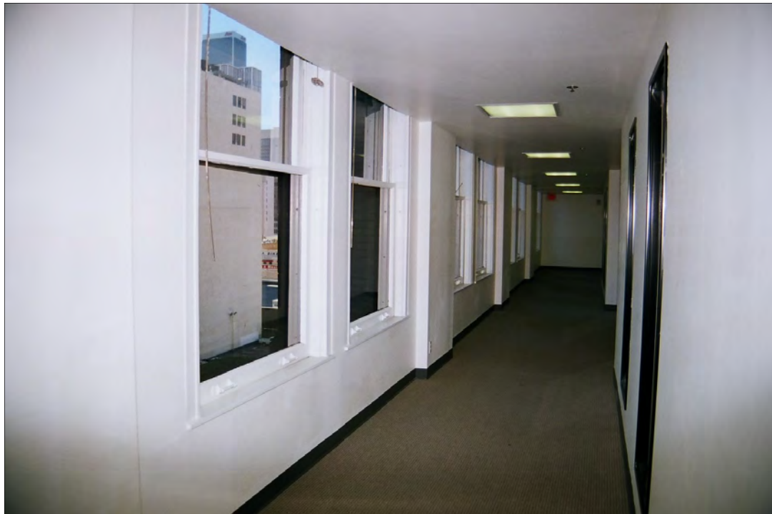
Photo 51: Sixth floor corridor, view west (Chattel, 2011)
