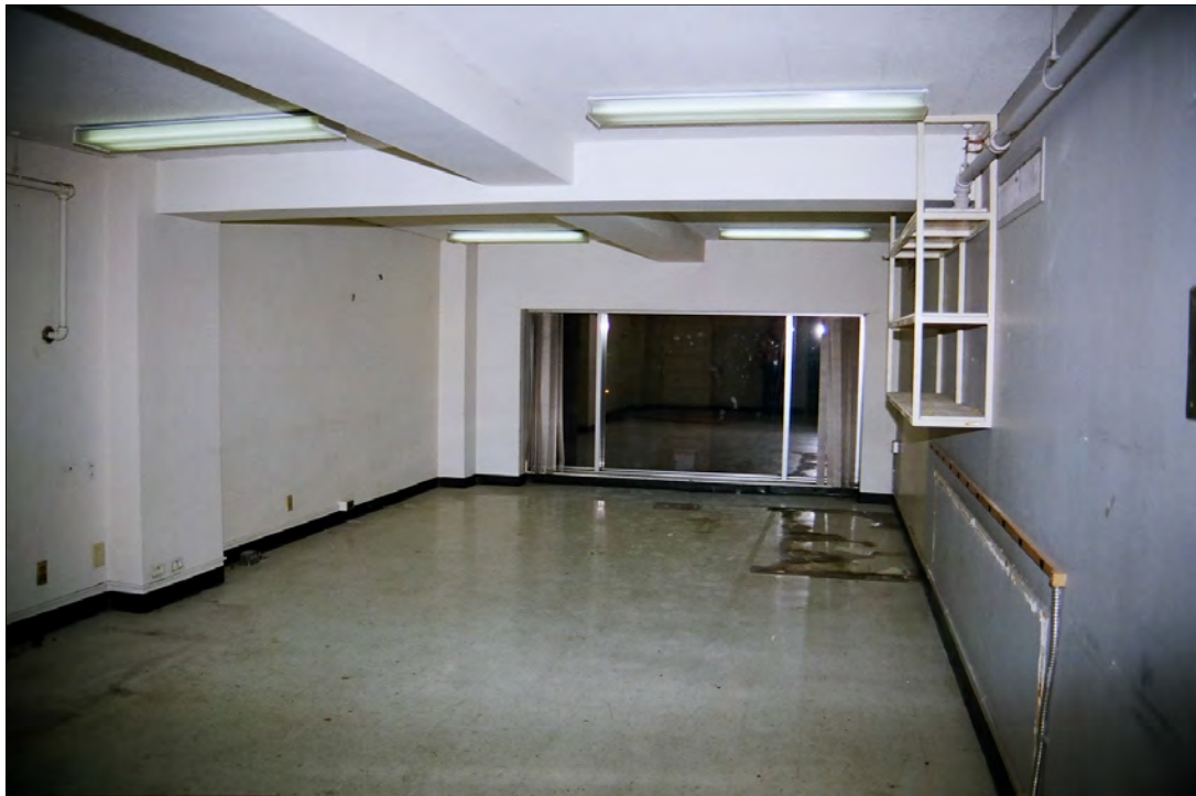
Photo 25: Mezzanine, view south (Chattel, 2011)
