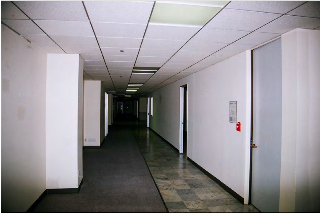
Photo 47: Fifth floor corridor, view west, note original marble floor (Chattel, 2011)
