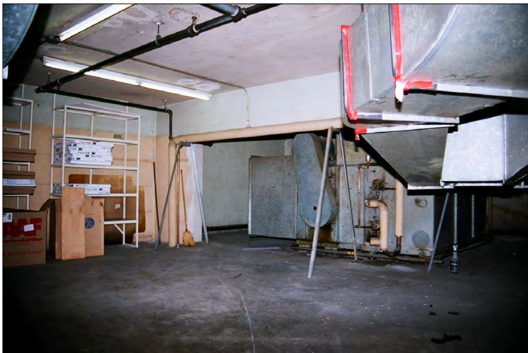
Photo 23: Mezzanine, view east (Chattel, 2011)
