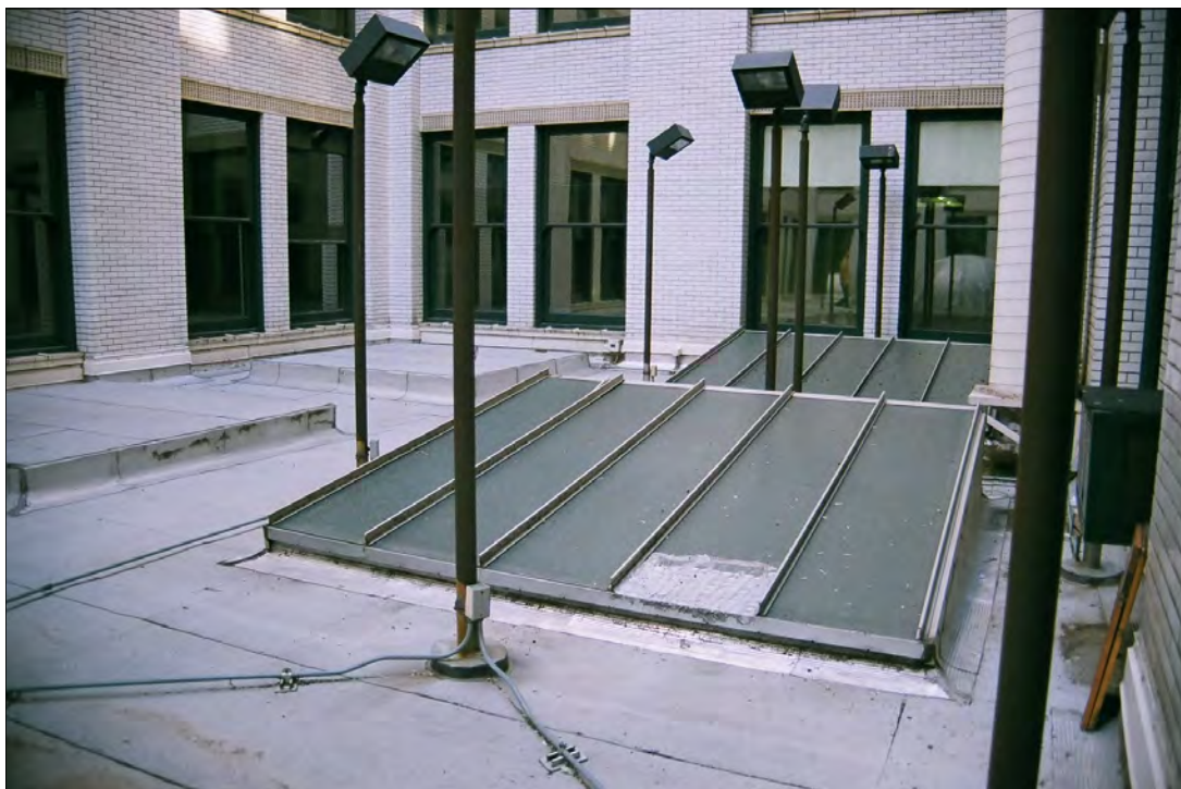
Photo 35: Second floor light court, view east (Chattel, 2011)
