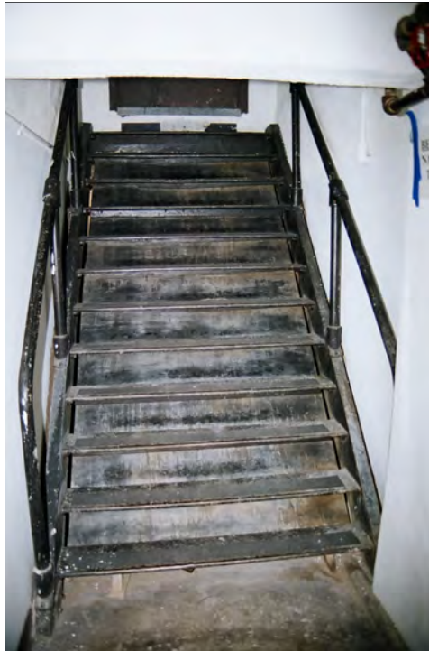
Photo 68: Stairs to roof from ninth floor, view west (Chattel, 2011)
