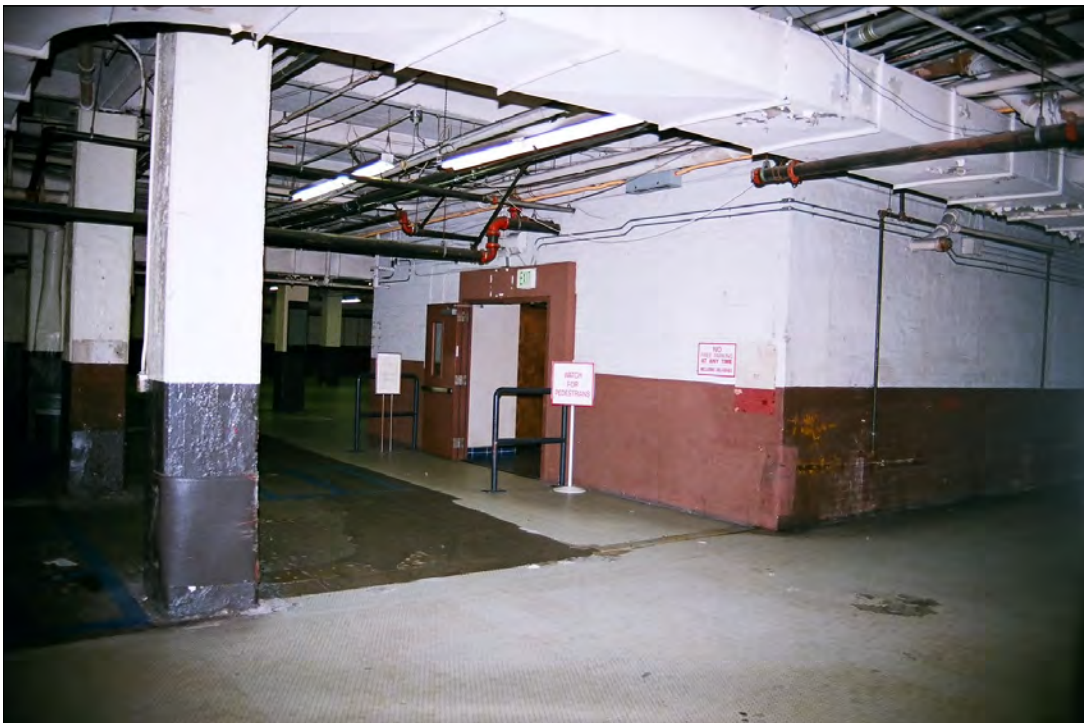
Photo 12: Basement, view southeast (Chattel, 2011)
