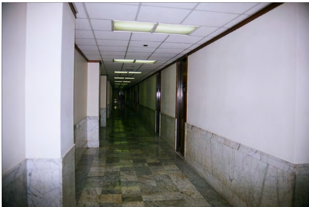
Photo 29: Second floor corridor, view east, note original marble wainscot and floor and original wood doors (Chattel, 2011)
