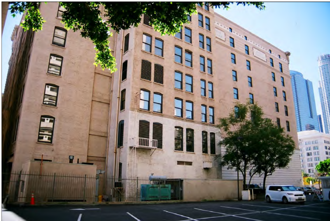
Photo 9: North elevation, view south (Chattel, 2011)
