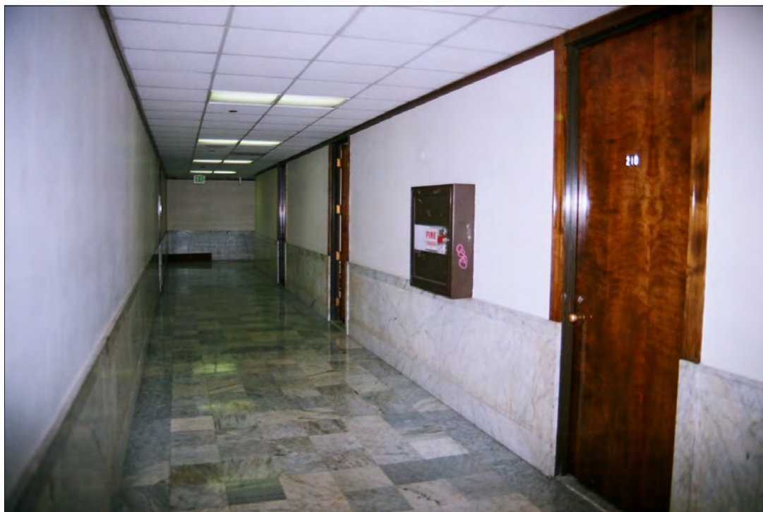
Photo 28: Second floor corridor, view north, note original marble wainscot and floor and original wood doors (Chattel, 2011)
