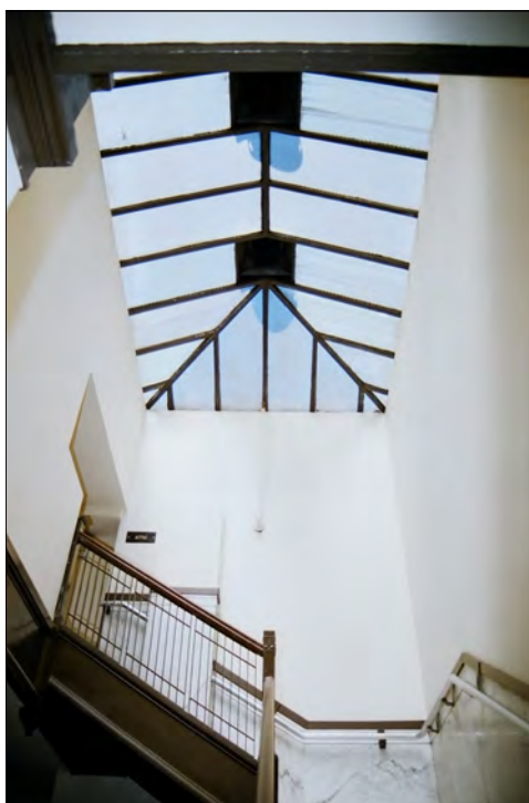
Photo 61: View upward of stairwell and skylight from eighth floor (Chattel, 2011)
