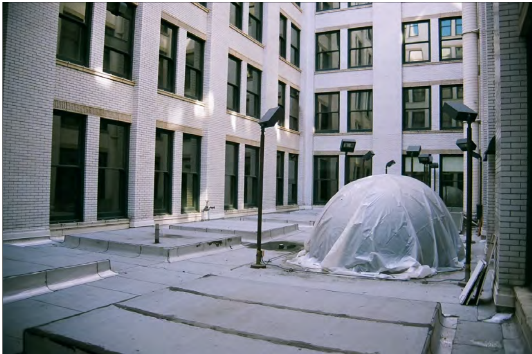
Photo 34: Second floor light court, view east (Chattel, 2011)
