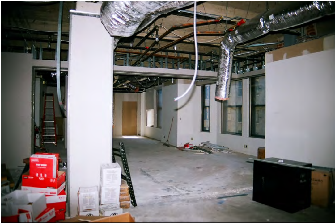
Photo 46: Fourth floor office space, view southeast (Chattel, 2011)
