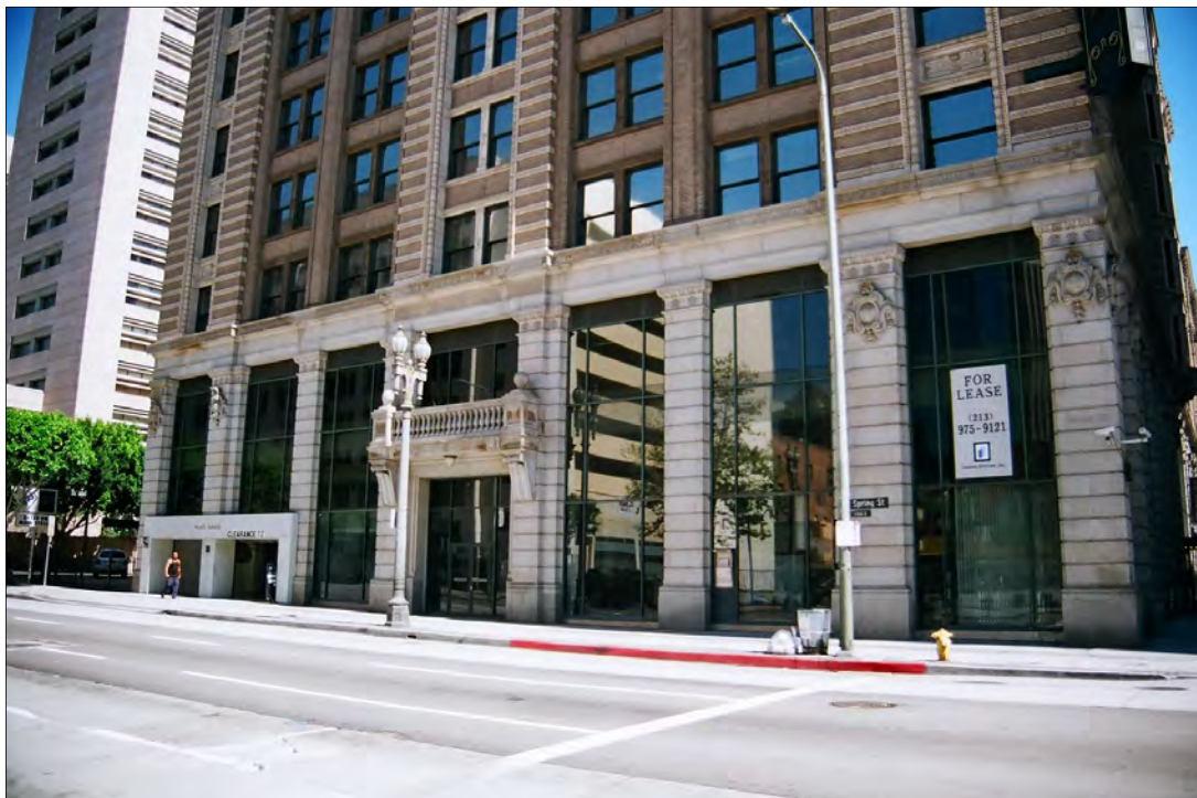
Photo 4: Detail of west façade, view east (Chattel, 2011)
