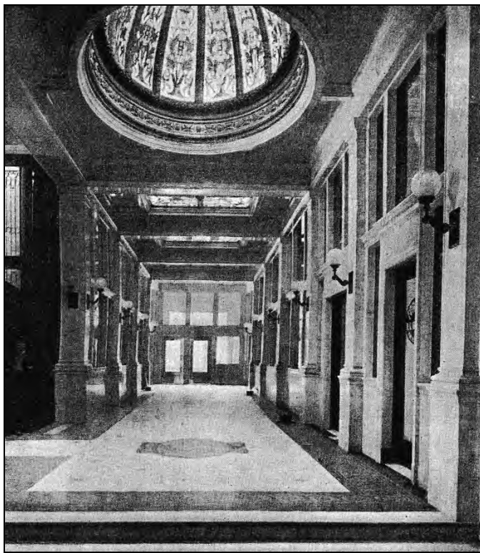
Figure 13: East-west corridor of the lobby. ( The Architect and Engineer of California , 1906)
