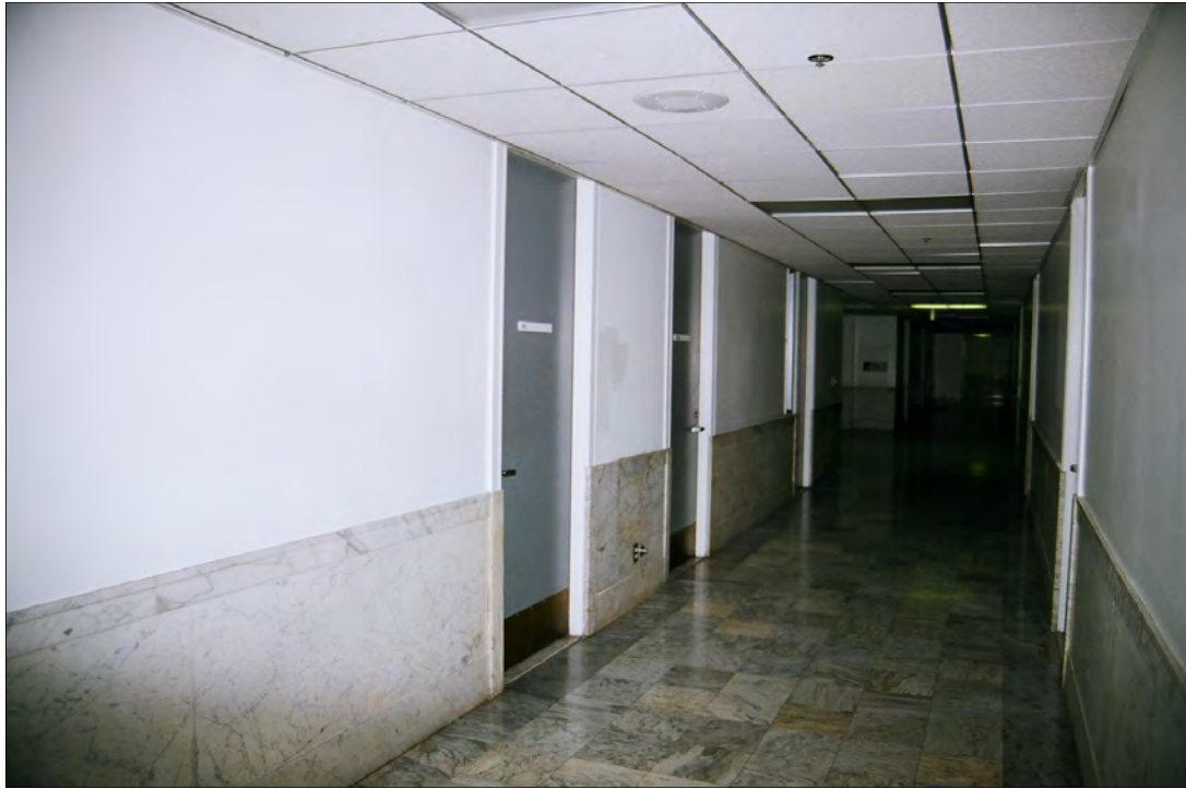
Photo 39: Third floor corridor, view east, note original marble wainscot and floor (Chattel, 2011)
