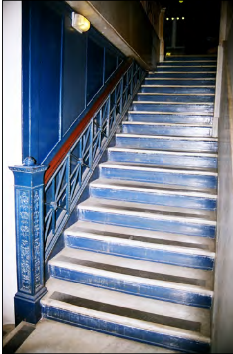
Photo 13: Stairs from basement to lobby, view south (Chattel, 2011)
