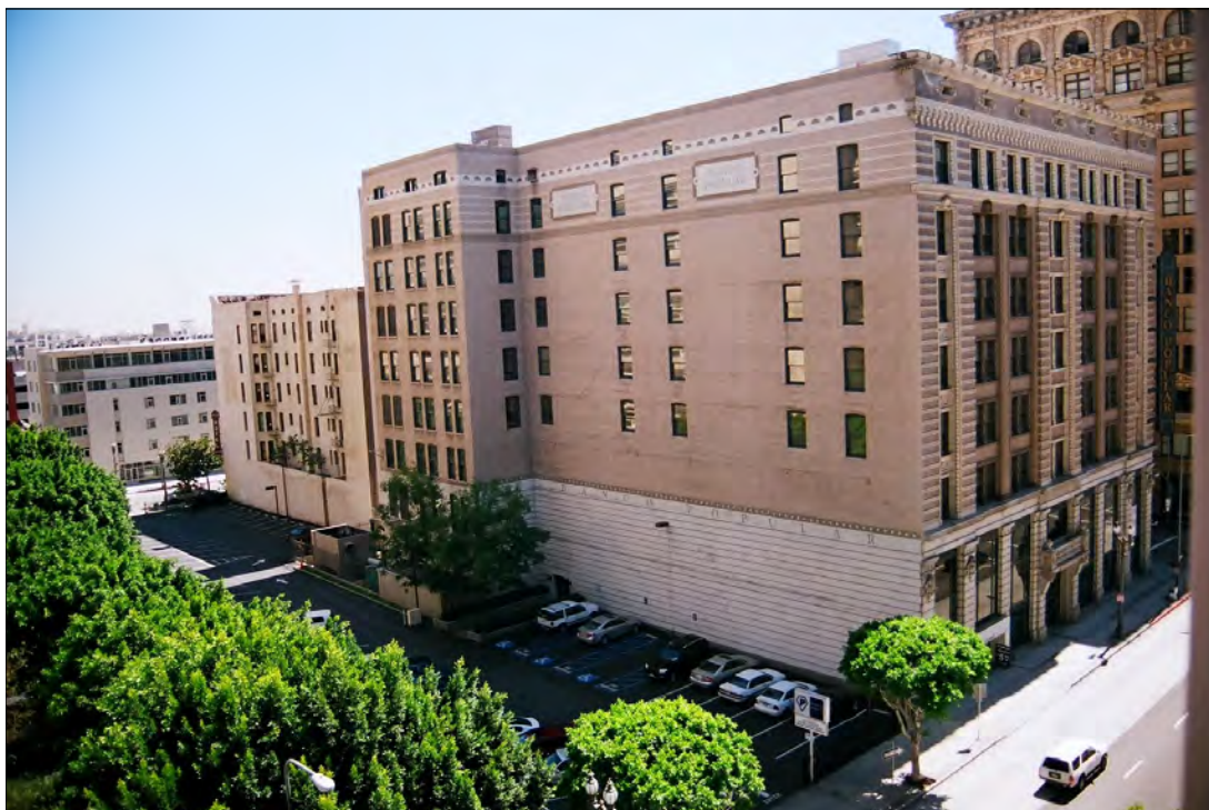
Photo 10: North elevation, view southeast (Chattel, 2011)
