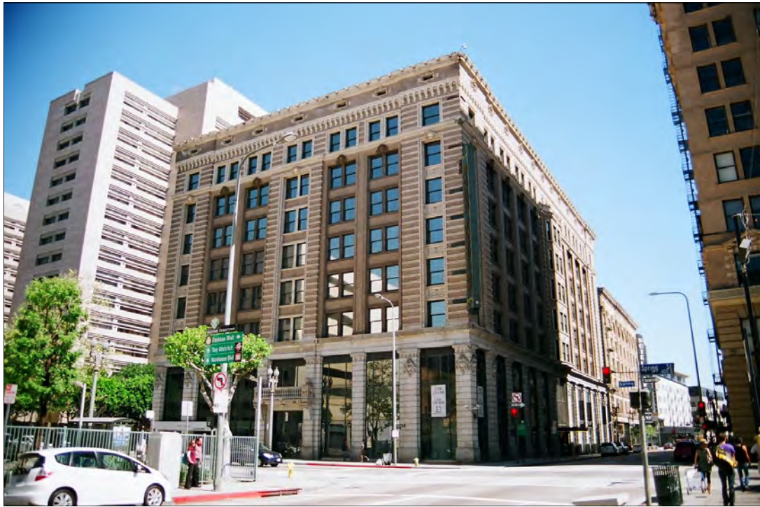
Photo 1: South and west façades, view northeast (Chattel, 2011)
