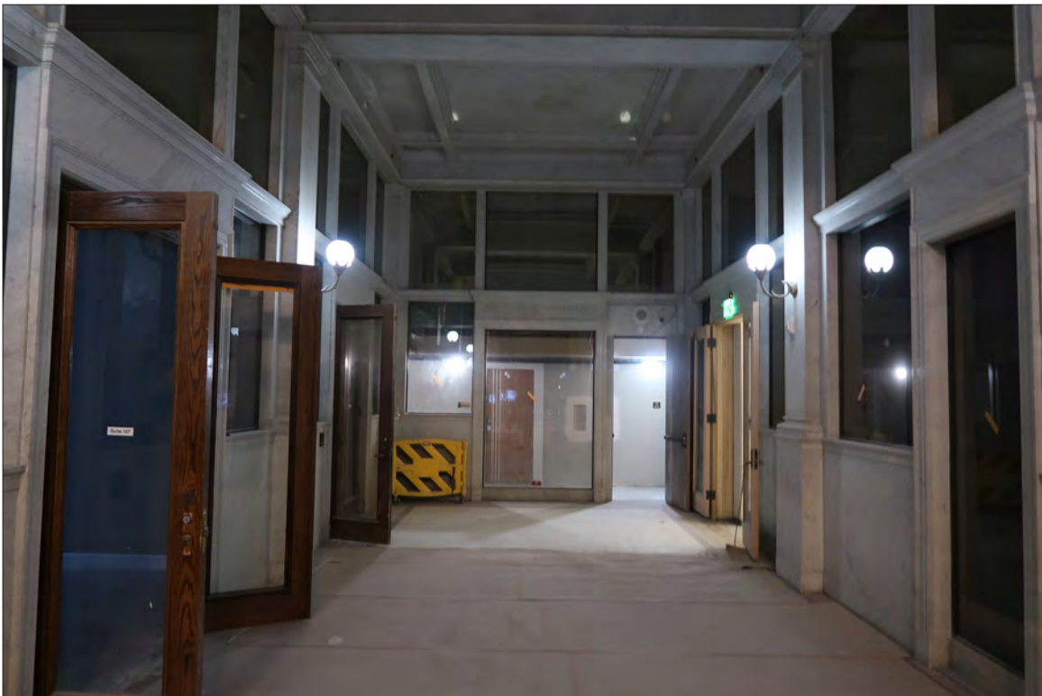
Image 5: 354 S. Spring Street, lobby, view east (Chattel, 2019)
