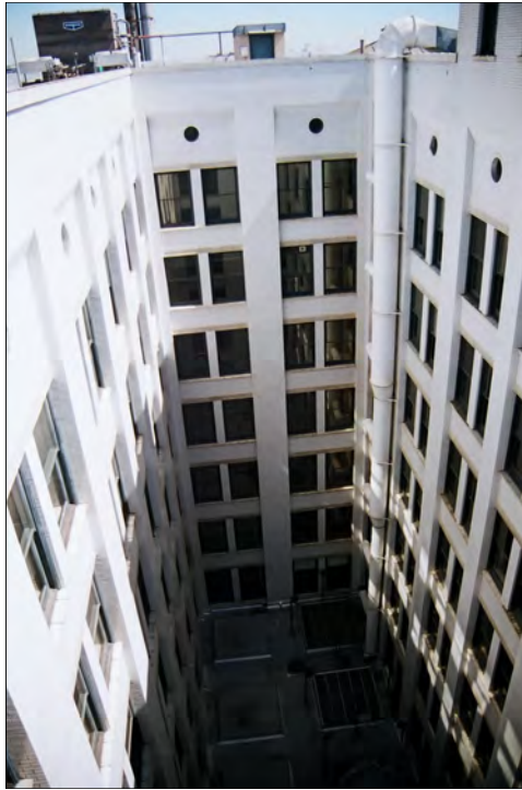
Photo 75: View east of light court from roof (Chattel, 2011)
