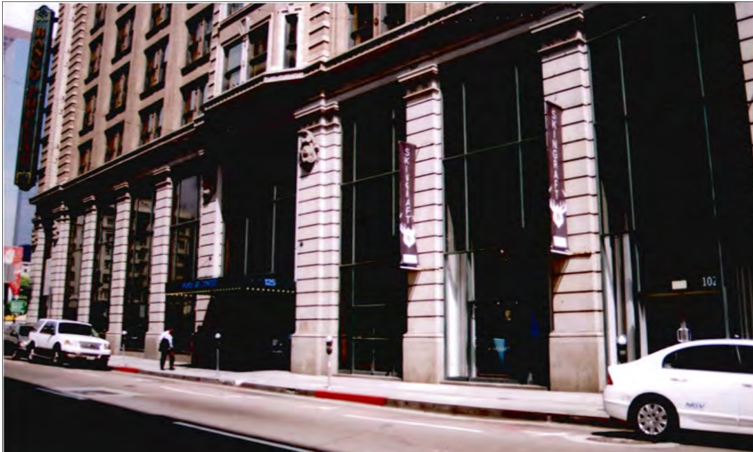
Photo 7: South façade, view northwest (Chattel, 2011)
