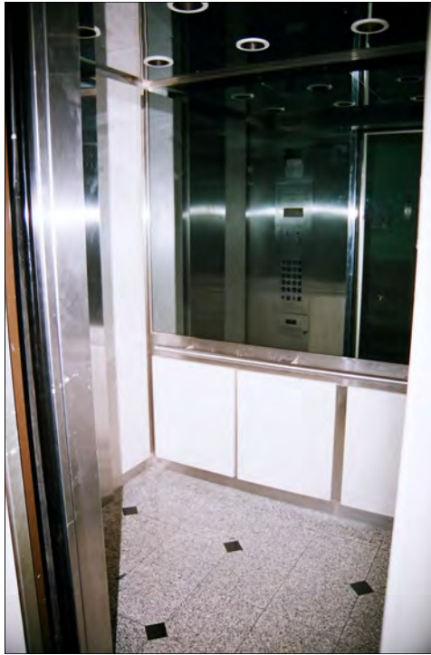
Photo 66: View of elevator at eighth floor (Chattel, 2011)
