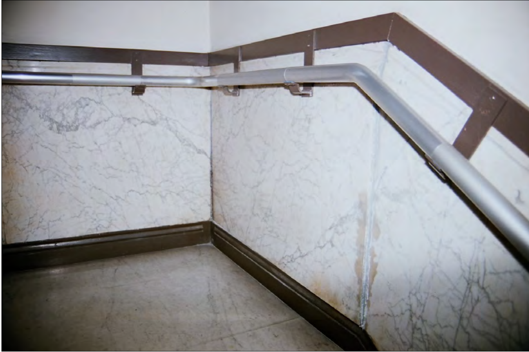
Photo 37: Detail of third floor stairwell, note original marble wainscot and floor (Chattel, 2011)
