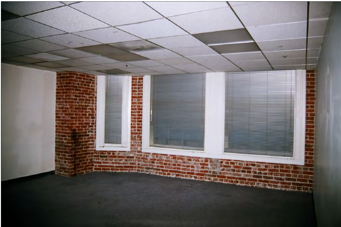
Photo 48: Fifth floor office, view south (Chattel, 2011)
