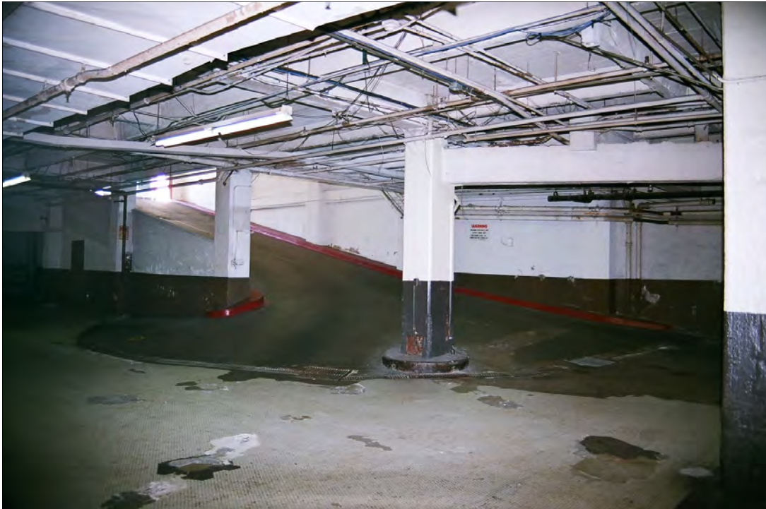
Photo 11: Basement, view northwest, note ramp leading to Spring Street (Chattel, 2011)
