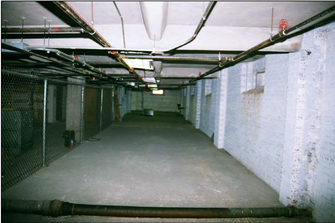
Photo 72: Ninth floor, view east (Chattel, 2011)
