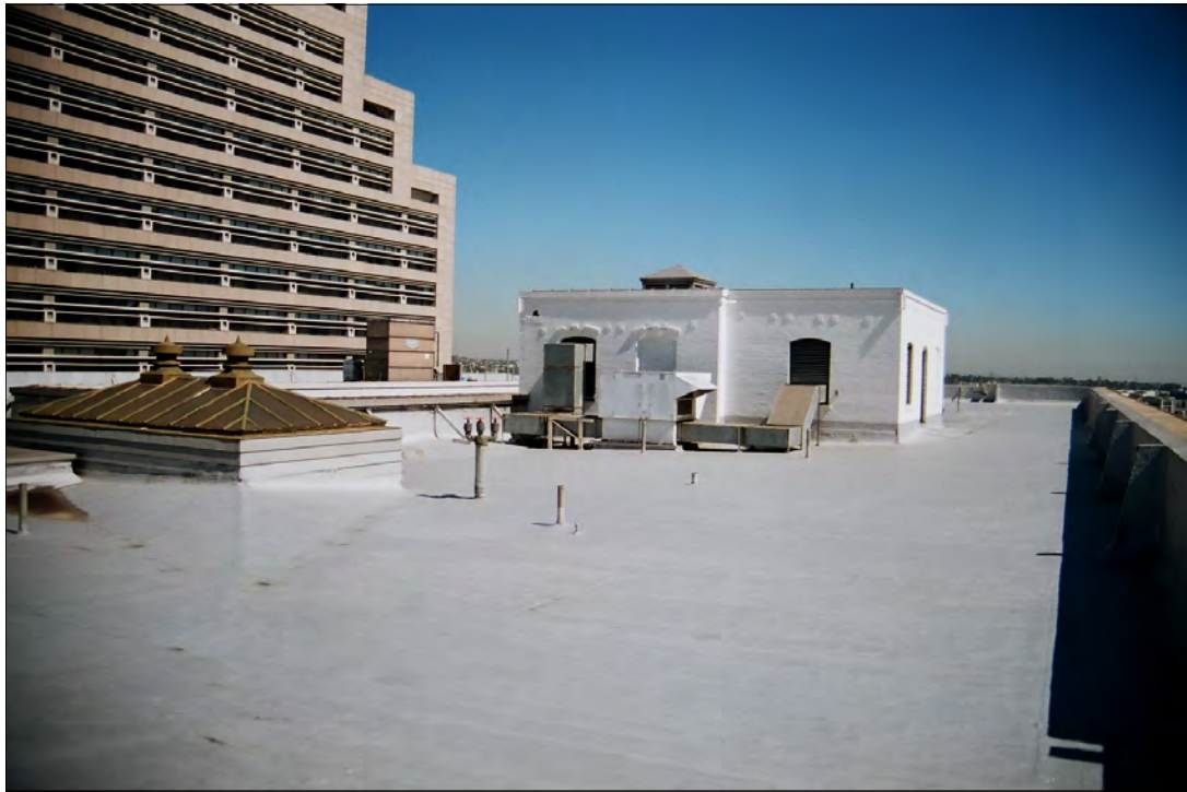
Photo 73: Roof, view east (Chattel, 2011)
