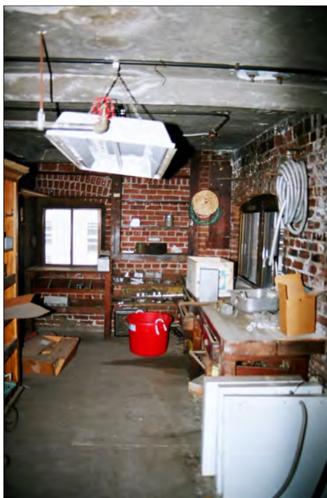
Photo 71: Ninth floor, view north (Chattel, 2011)
