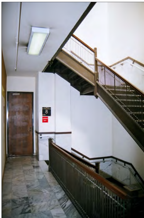
Photo 60: Eighth floor stairwell, view north, note original marble flooring and wainscot (Chattel, 2011)
