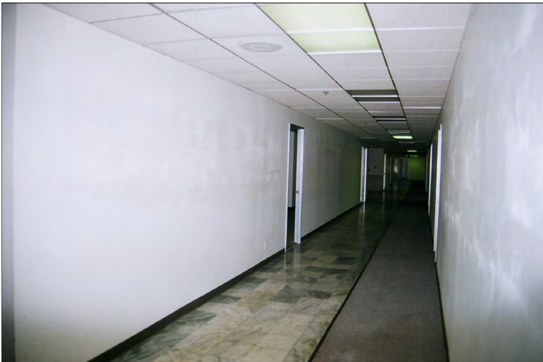
Photo 63: Eighth floor corridor, view east, note original marble floor (Chattel, 2011)
