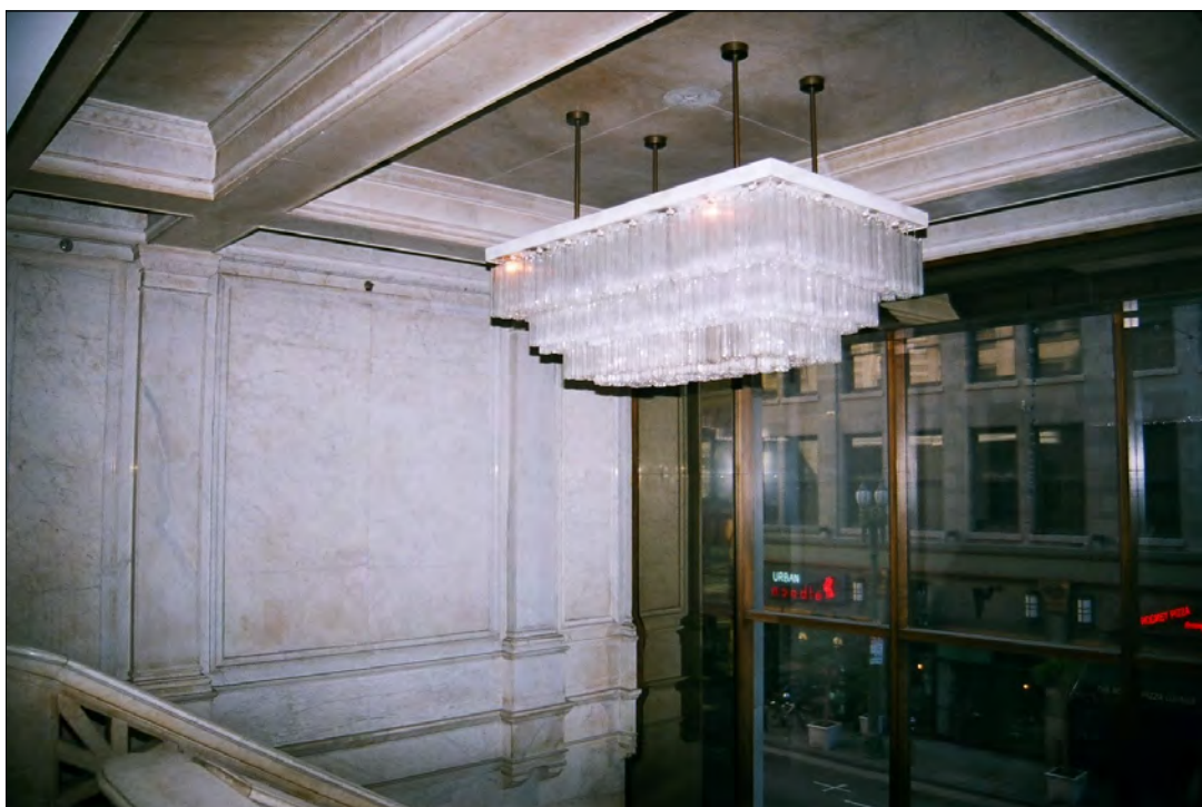
Photo 27: Second floor stairs to lobby entrance, view southeast, note original marble on walls, ceiling, and banisters (Chattel, 2011)
