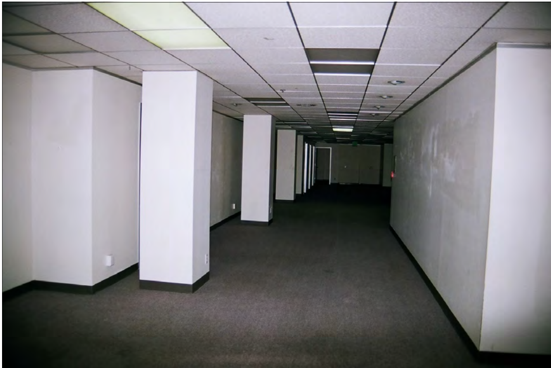
Photo 57: Seventh floor open office space, view north (Chattel, 2011)
