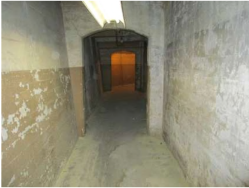
Photograph 10 Five Story Building at 2060 East 7 th Street – Basement walkway
