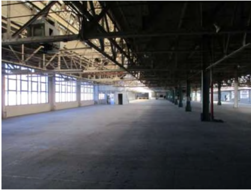
Photograph 3 2-Story 2060 East 7 th Street Building
