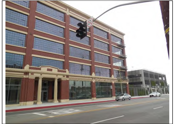
2. View of the subject property from northeast
