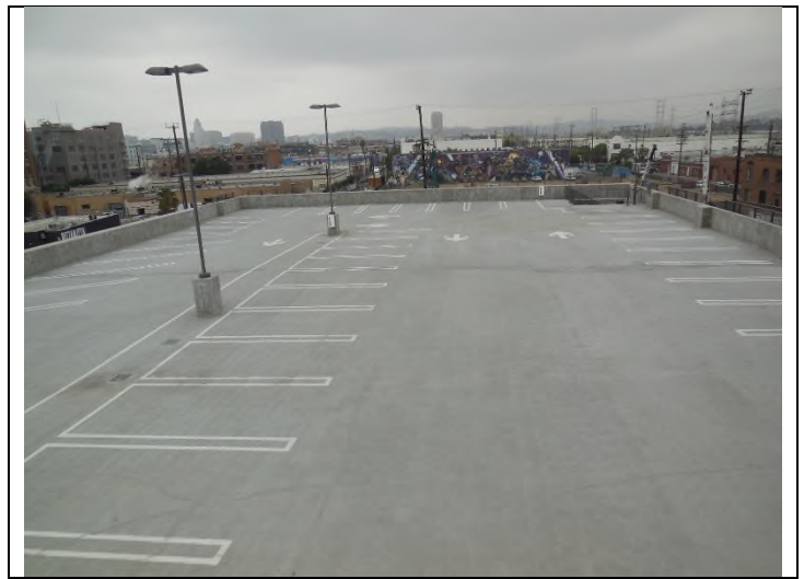
20. View of parking structure
