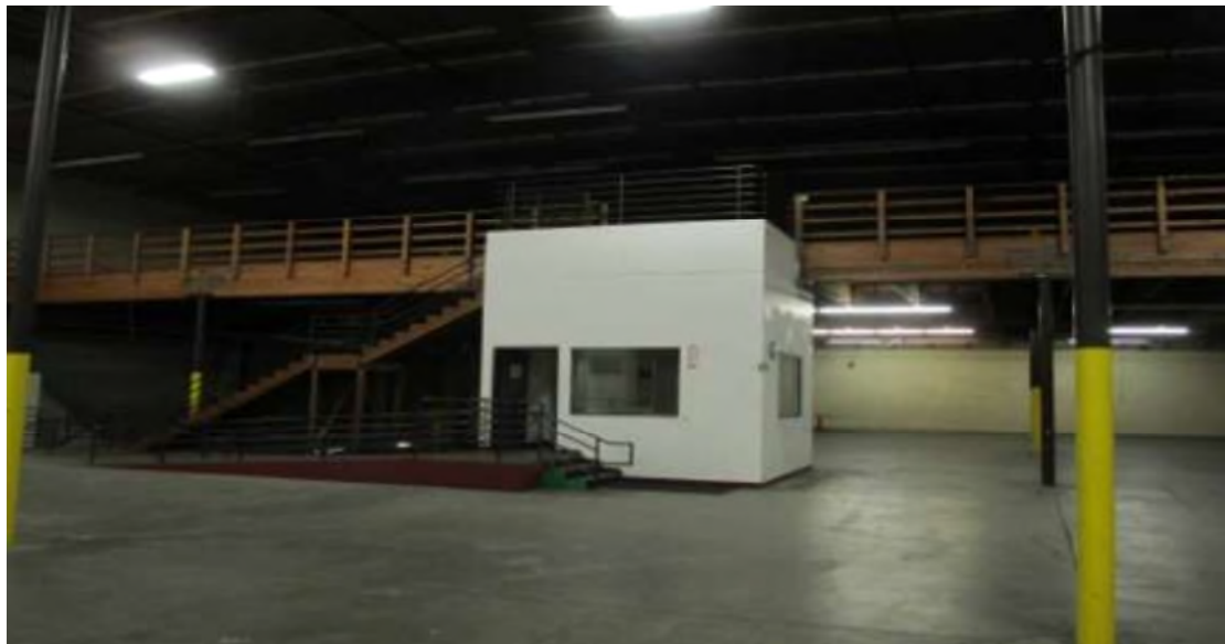
Photograph 2 821 South Santa Fe Avenue & 2053 Violet Street – Looking toward mezzanine
