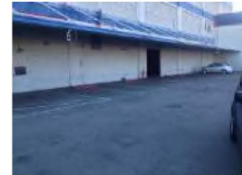
Canopy on west side of building
