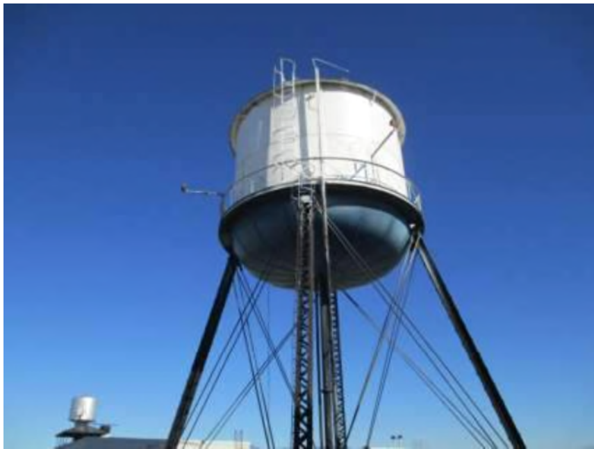
Photograph 7 Water Tower on top of 2060 East 7 th Street five-story building
