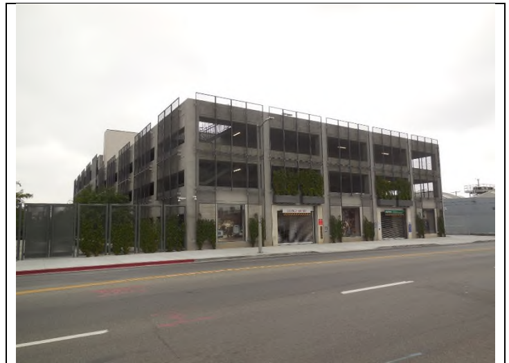
6. View of parking structure
