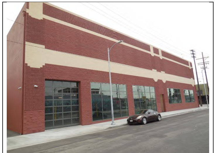
4. View of the subject property from southwest
