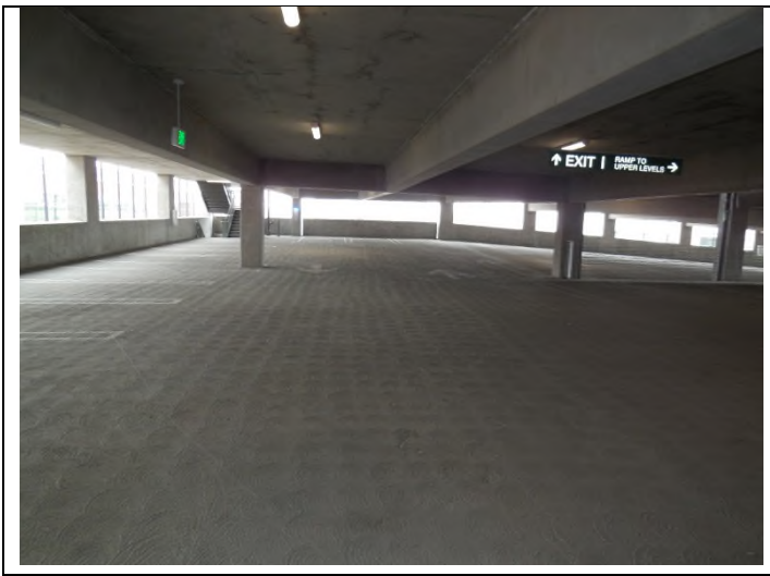
19. View of parking structure
