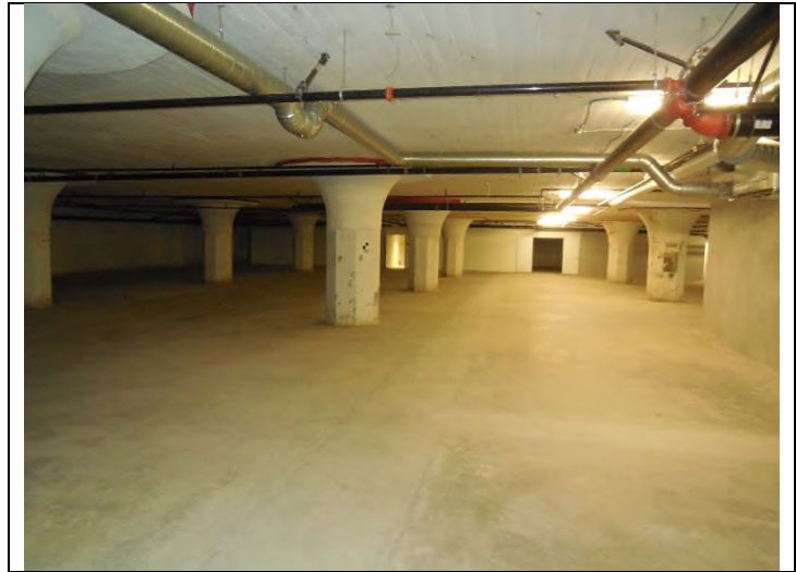
16. View of basement
