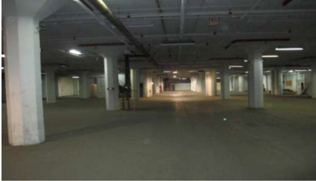
Photograph 1 Five Story Building at 2060 East 7 th Street - Basement
