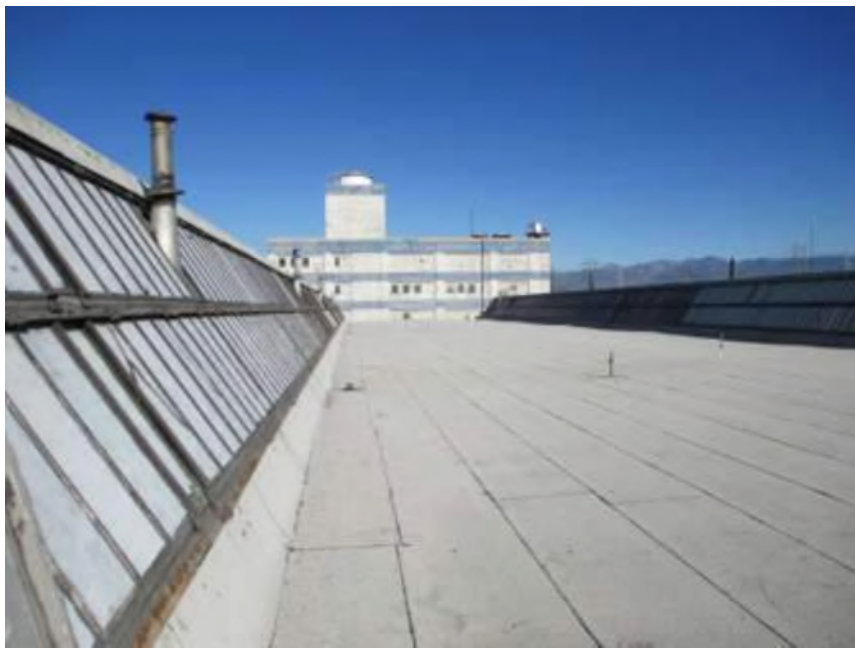
Photograph 4 2-Story 2060 East 7 th Street Building – From roof.
