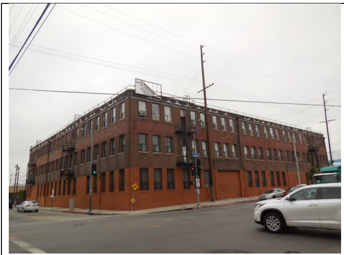
29. View of industrial building to the northeast
