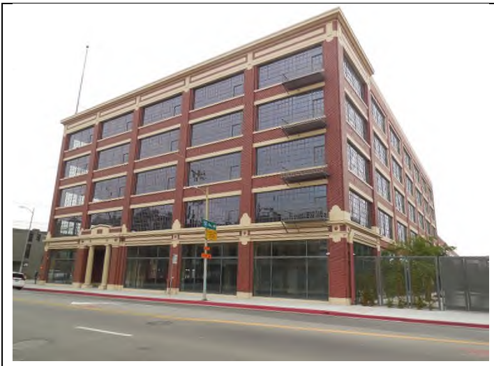
5. View of office building
