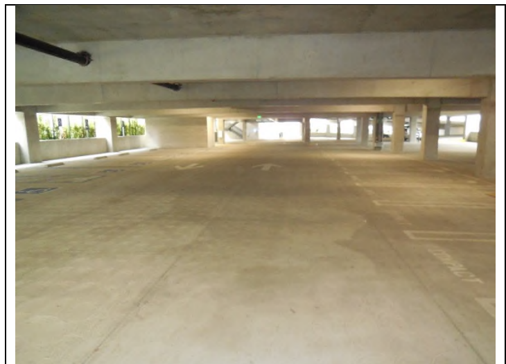
18. View of parking structure
