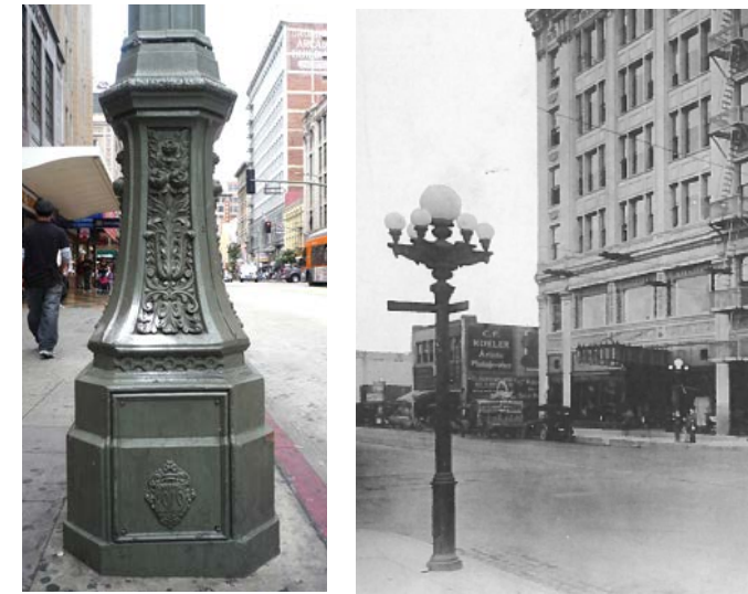
Existing “Broadway Rose” Streetlight Base; Historic photo of a 7-globe Llewellyn.
