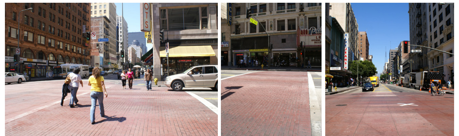
Crosswalks at Intersections and Midblocks have red integral colored concrete with a faux brick imprint pattern. Interior fields of intersections also have red integral colored concrete.
