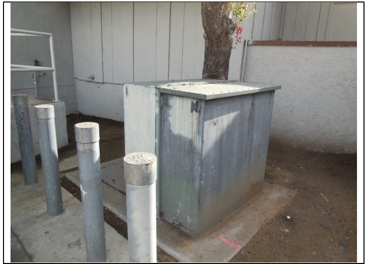
26. View of pad-mounted transformer on the property
