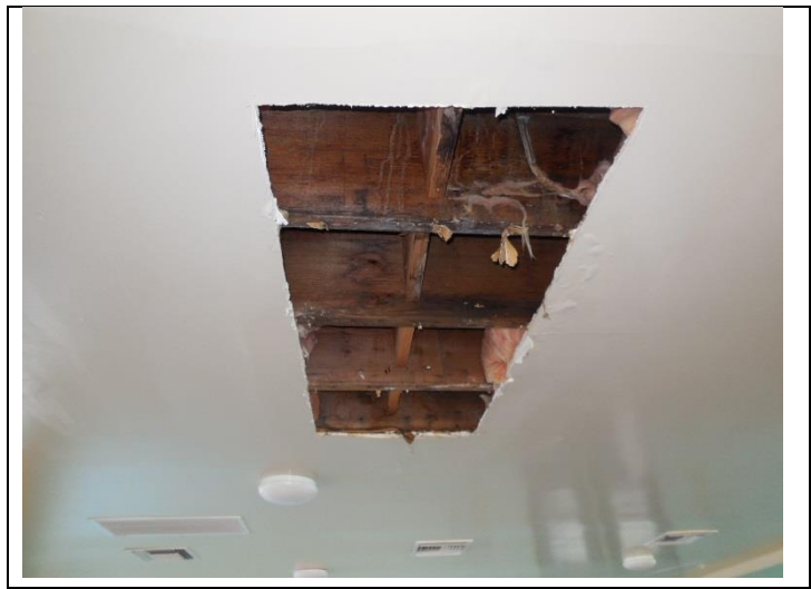
20. View of water intrusion
