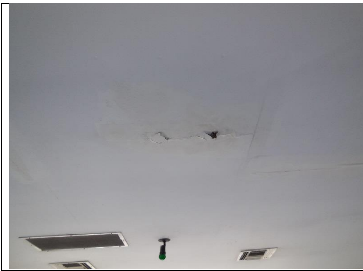
19. View of water intrusion
