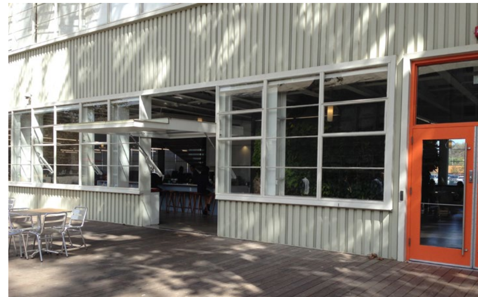
An easy to locate, and clearly distinguishable, building entrance creates a welcoming user experience.
