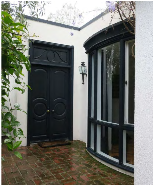
Seiter Residence, view southeast of the primary (north) façade and front door (ARG, 2019).
