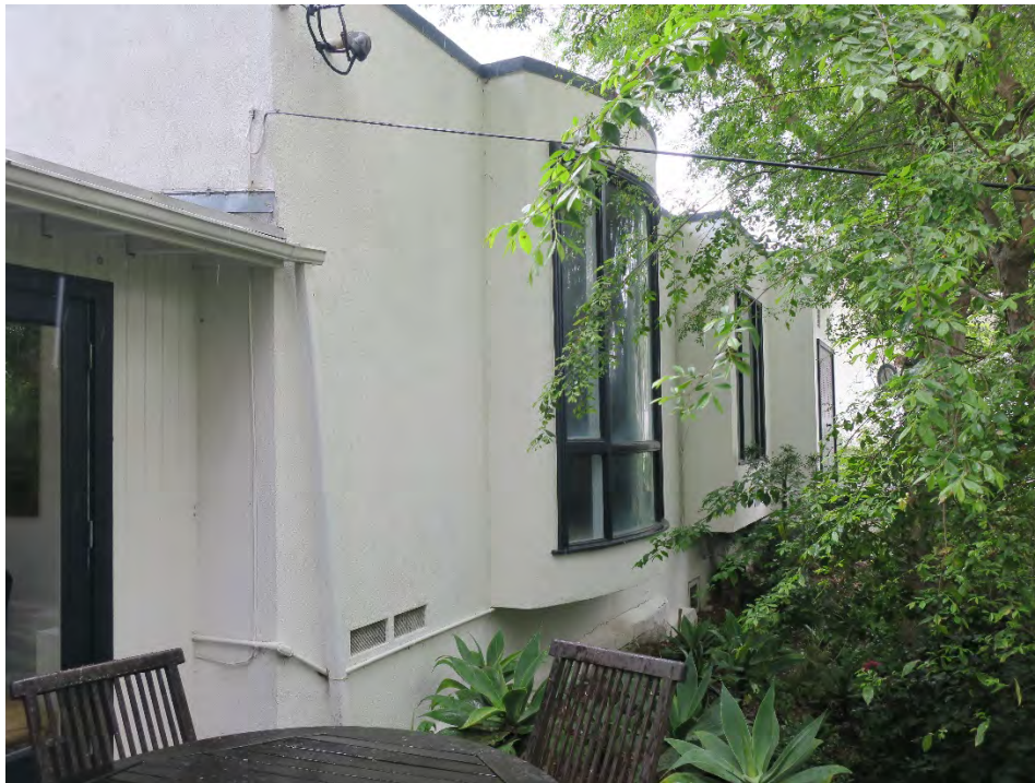
Seiter Residence, view northeast of the south façade (ARG, 2020).
