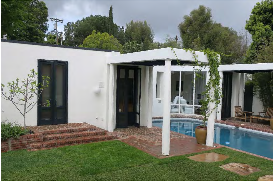
Seiter Residence, view northwest of the east façade (ARG, 2019).
