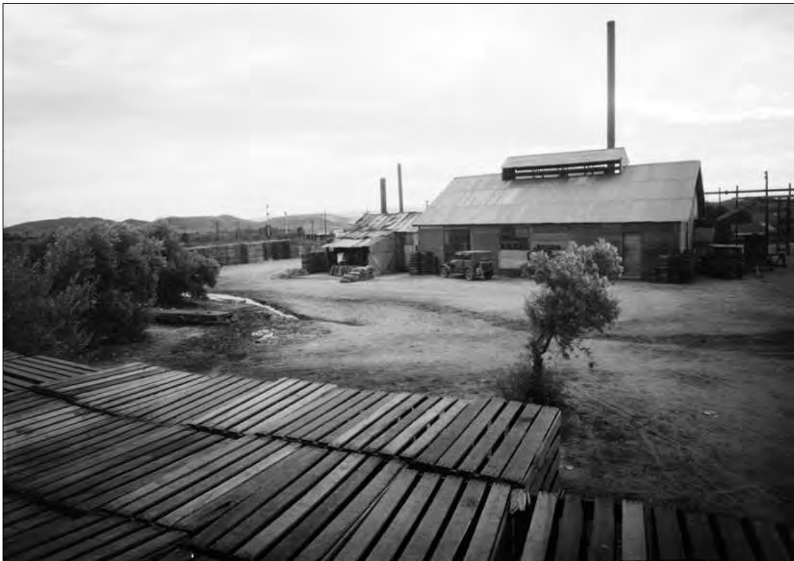
Olive packing house, Los Angeles Olive Growers Association, Sylmar, before 1932. The building features a monitor roof to provide ventilation to the interior workspace. Source: Title Insurance and Trust/C.C. Pierce Photography Collection, 1860-1960, California Historical Society, University of Southern California Libraries Special Collections.
