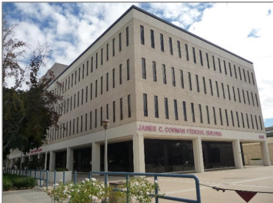
District: San Fernando Valley Administrative Center Name: James C. Corman Federal Building Architect: Honnold, Rex, Rochlin & Baran Date: 1974
