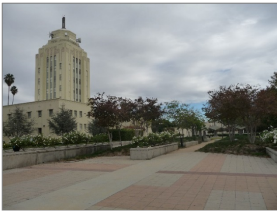
District: San Fernando Valley Administrative Center Description: Overview with Valley Municipal Building Architect: Peter K. Schabarum Period of Significance: 1932-1988
