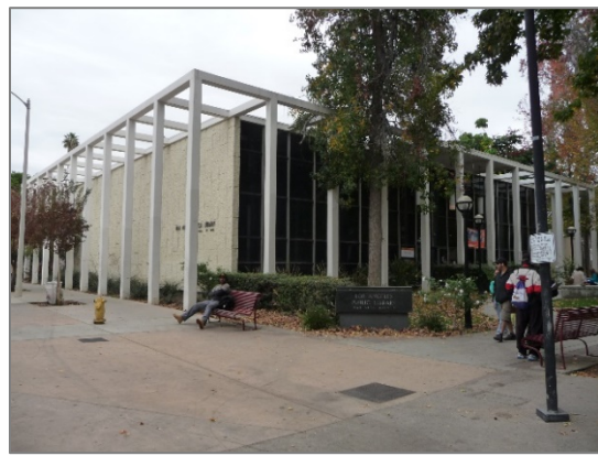
District: San Fernando Valley Administrative Center Name: Los Angeles Public Library, Van Nuys Branch Architect: Kegley, Westphall, Arbogast & Stewart Date: 1964
