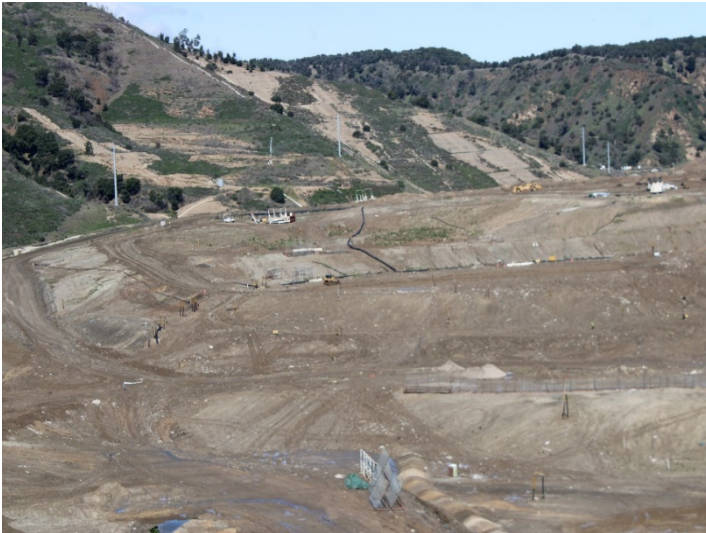
Photo 461: General Site: March 7, 2024
