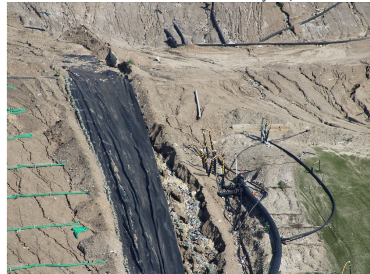
Photo 412: General Site: February 15, 2024
