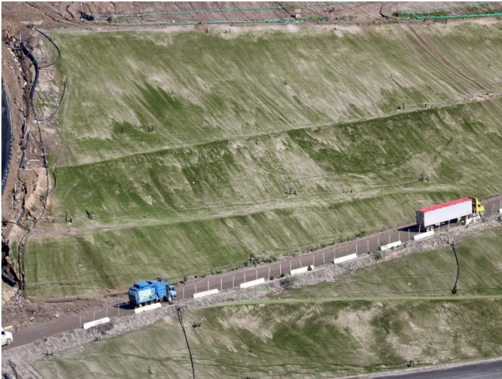
Photo 93: Closure Turf: March 7, 2024
