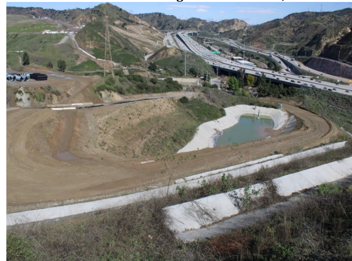
Photo 556: Road Realignment: March 7, 2024
