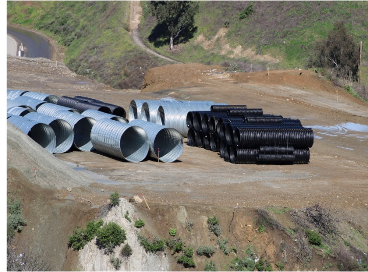
Photo 578: Road Realignment: March 7, 2024
