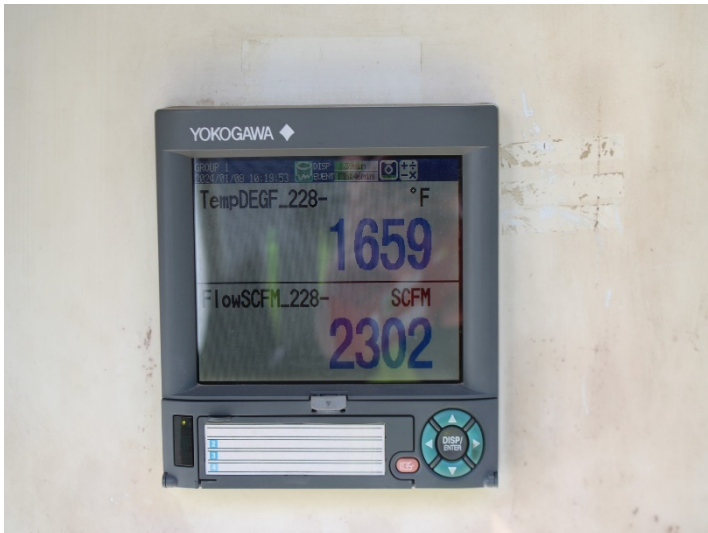
Photo 353: General Site: January 8, 2024
