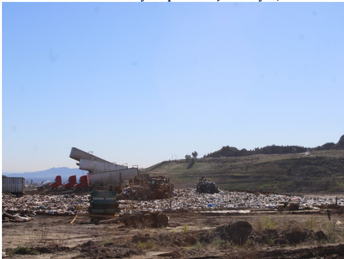
Photo 167: County Top Deck: January 8, 2024
