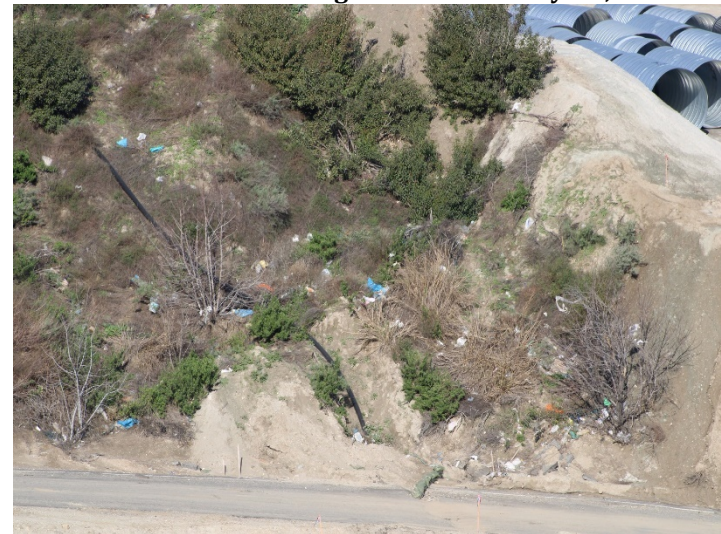
Photo 540: Road Realignment: February 15, 2024
