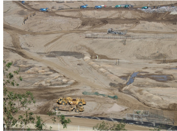
Photo 26: Working Area, CC4 Part 1/2: February 15, 2024
