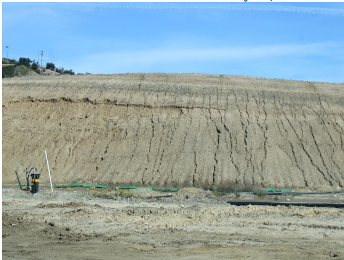
Photo 435: General Site: February 15, 2024
