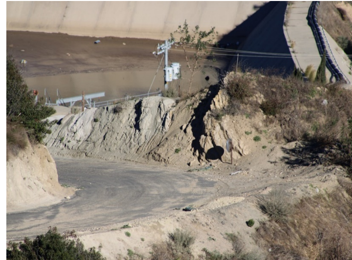
Photo 510: Road Realignment: January 8, 2024
