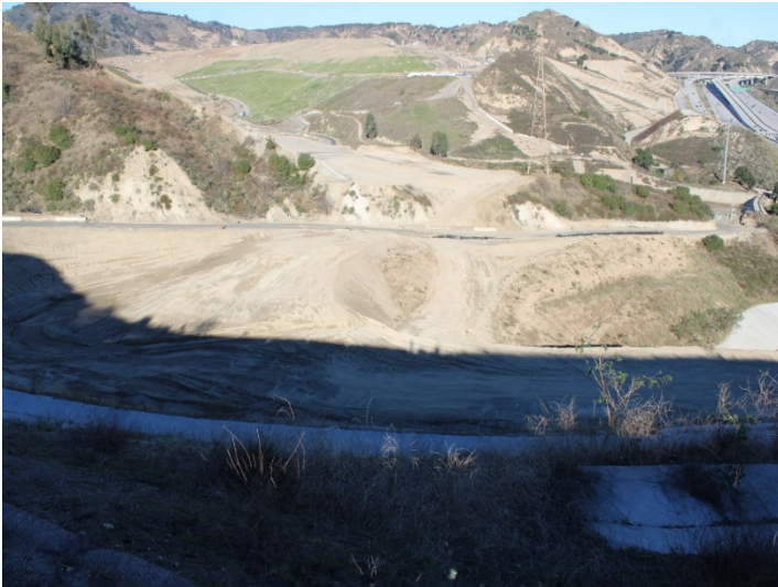
Photo 493: Road Realignment: January 8, 2024
