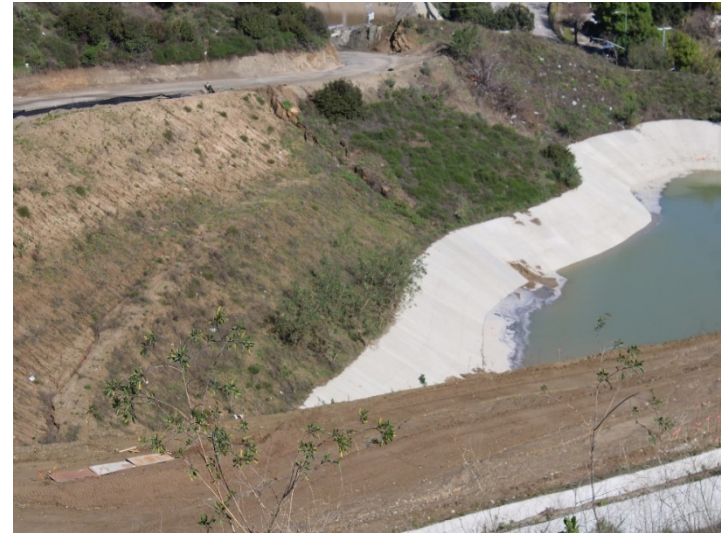
Photo 562: Road Realignment: March 7, 2024
