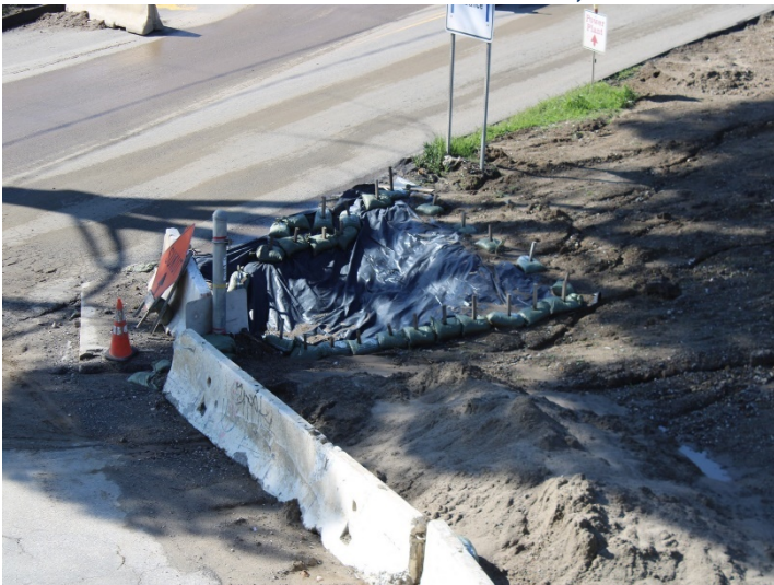
Photo 443: General Site: March 7, 2024
