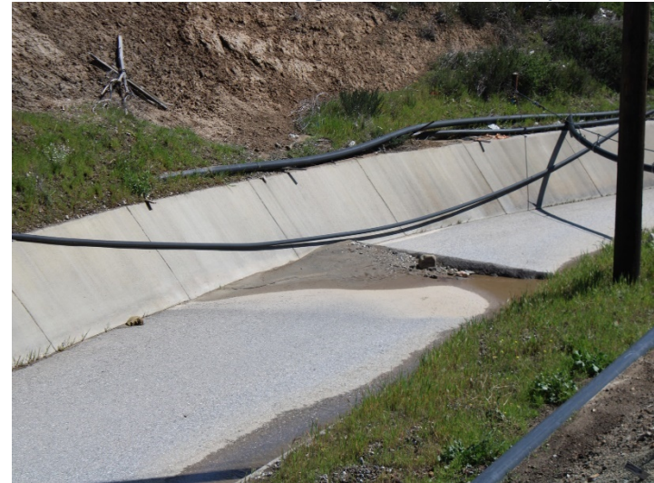
Photo 220: Eastside Drainage Channel: March 7, 2024
