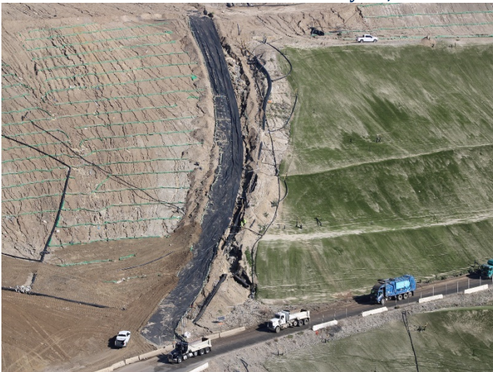
Photo 411: General Site: February 15, 2024
