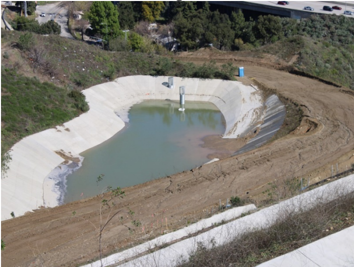
Photo 563: Road Realignment: March 7, 2024
