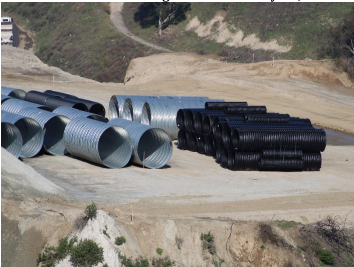
Photo 543: Road Realignment: February 15, 2024
