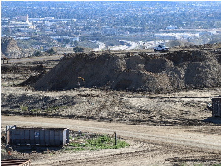
Photo 373: General Site: January 8, 2024
