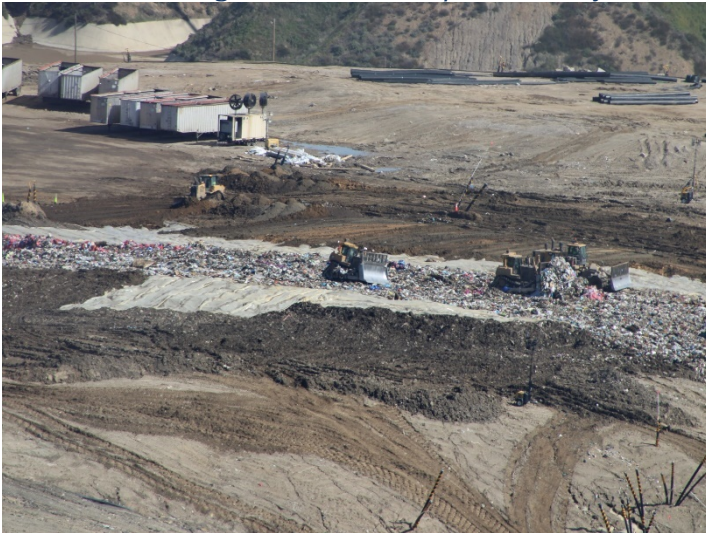
Photo 35: Working Area, CC4 Part 1/2: February 15, 2024
