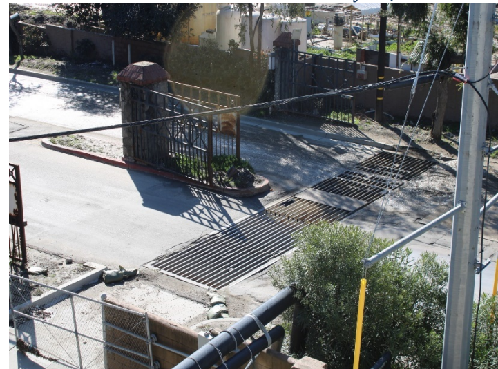
Photo 440: General Site: March 7, 2024
