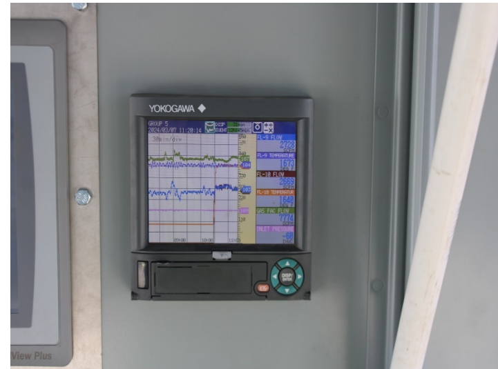
Photo 154: Flares 9, 10, 11 and Gas-to-Energy Facility: March 7, 2024
