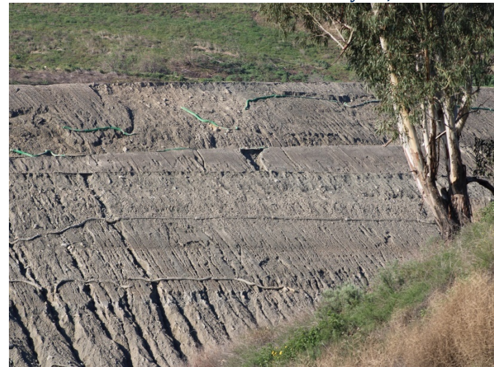
Photo 392: General Site: February 15, 2024
