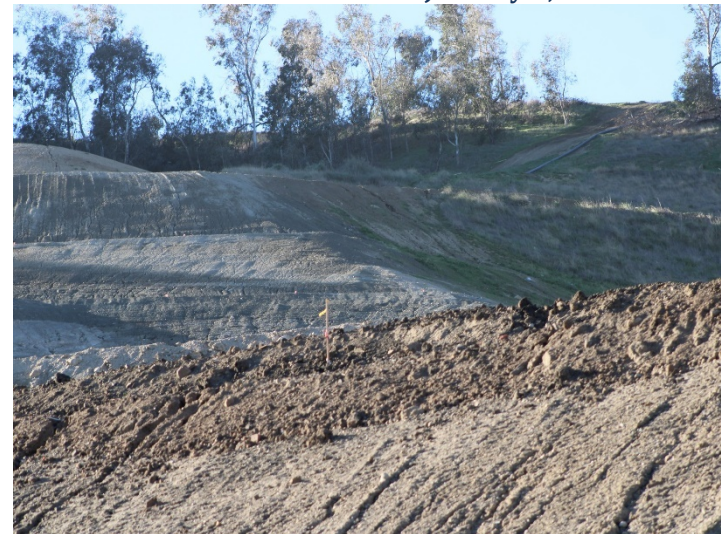
Photo 340: General Site: January 8, 2024
