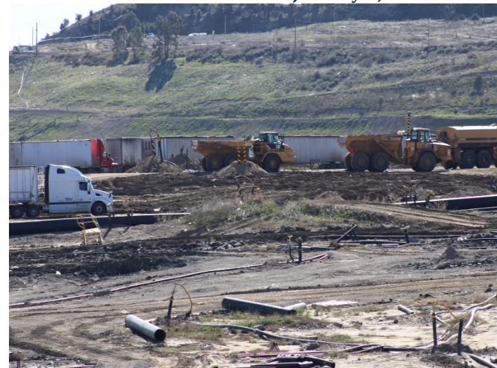
Photo 376: General Site: January 8, 2024
