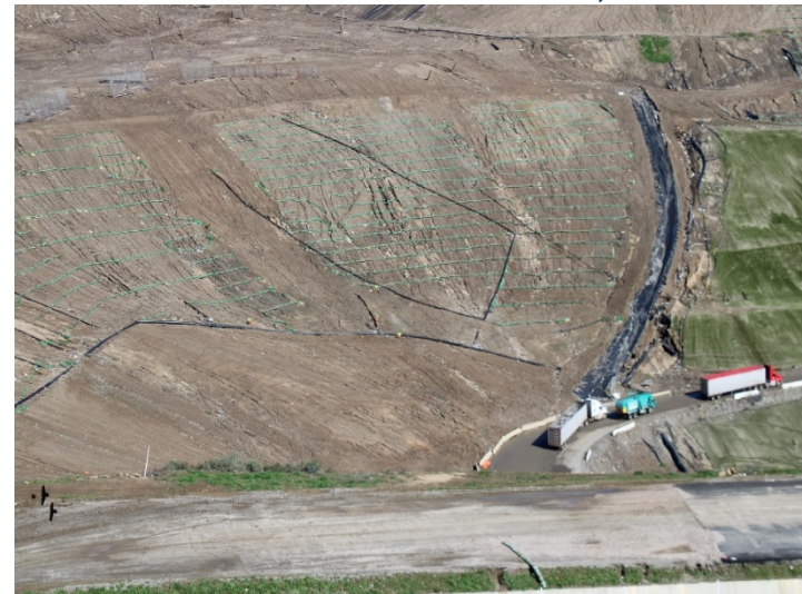
Photo 460: General Site: March 7, 2024
