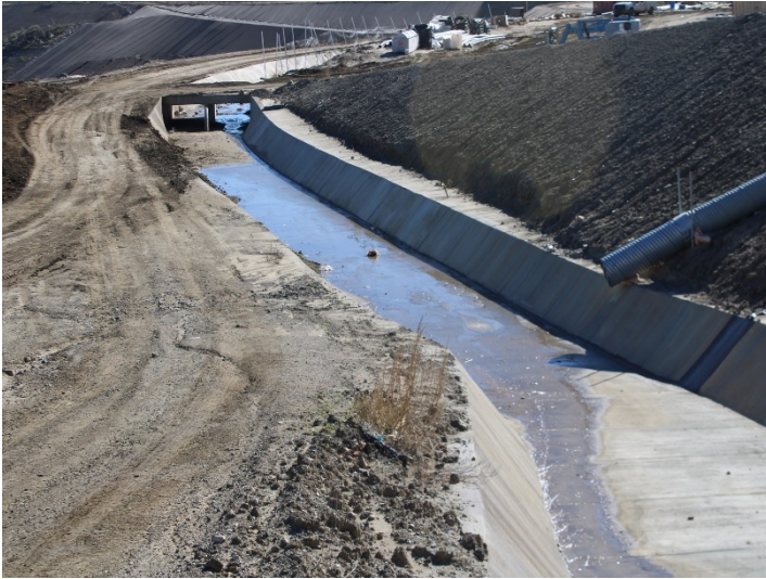
Photo 209: Eastside Drainage Channel: January 8, 2024
