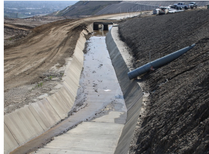
Photo 218: Eastside Drainage Channel: February 15, 2024
