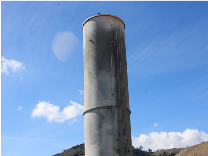
Photo 133: Flares 9, 10, 11 and Gas-to-Energy Facility: February 15, 2024
