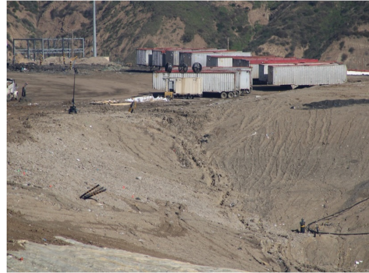
Photo 58: Working Area, CC-4 Part 3: February 15, 2024
