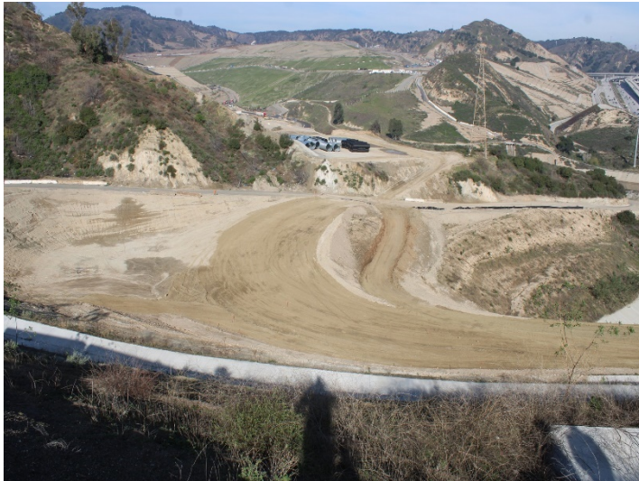
Photo 533: Road Realignment: February 15, 2024
