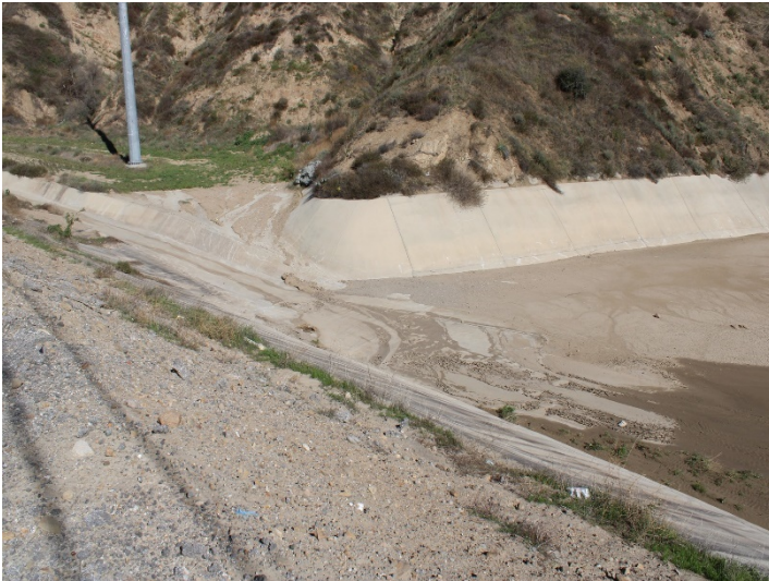
Photo 177: Basin B: January 8, 2024
