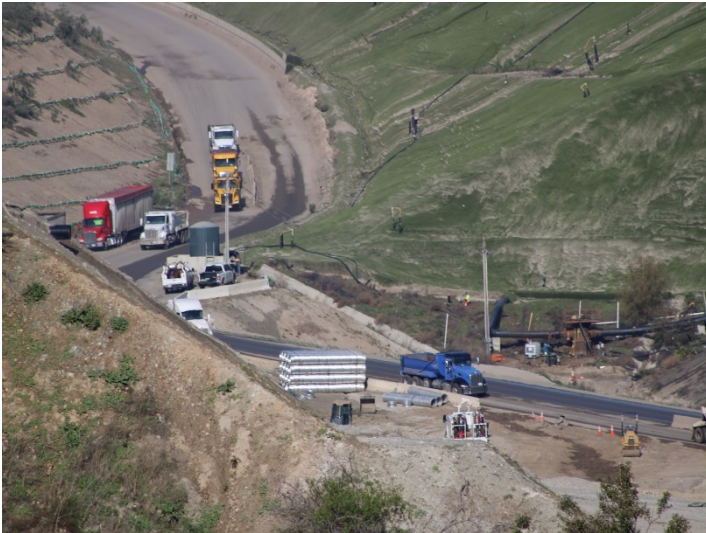
Photo 541: Road Realignment: February 15, 2024
