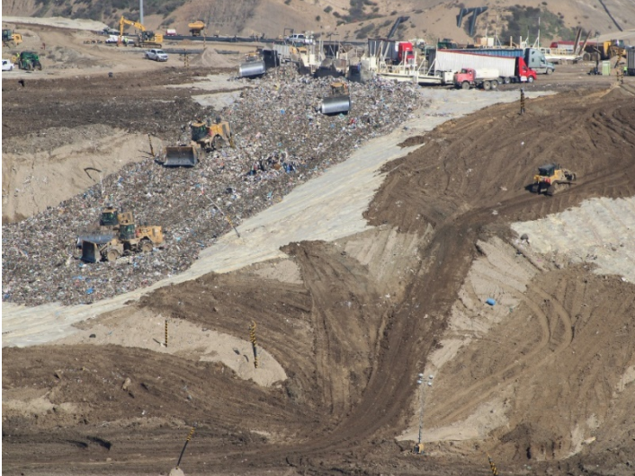
Photo 51: Working Area, CC-4 Part 3: February 15, 2024
