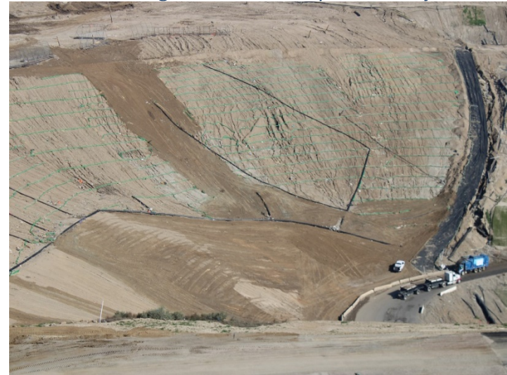
Photo 28: Working Area, CC4 Part 1/2: February 15, 2024
