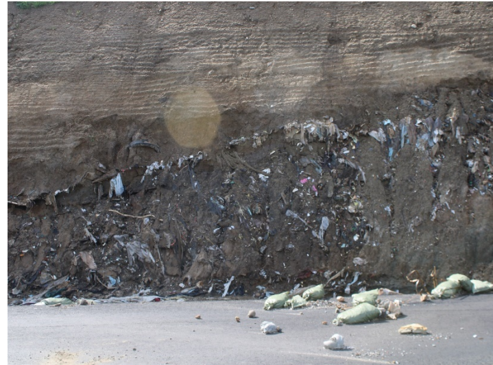
Photo 418: General Site: February 15, 2024
