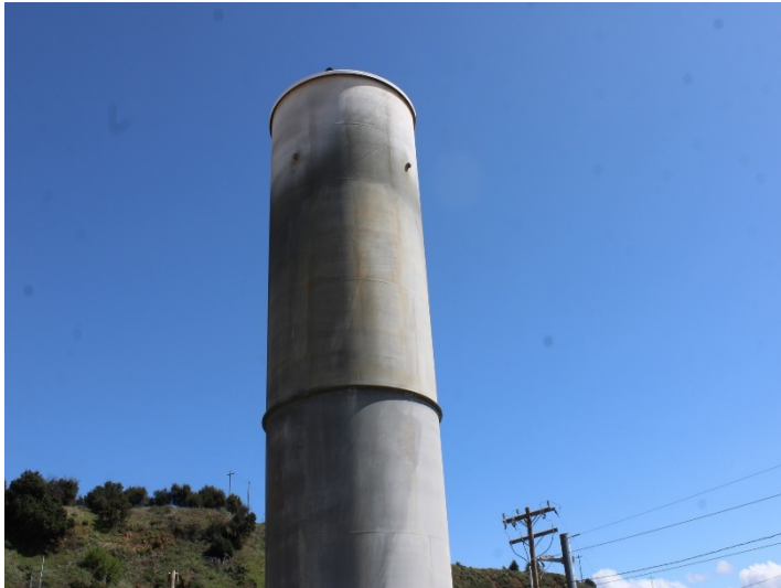
Photo 145: Flares 9, 10, 11 and Gas-to-Energy Facility: March 7, 2024
