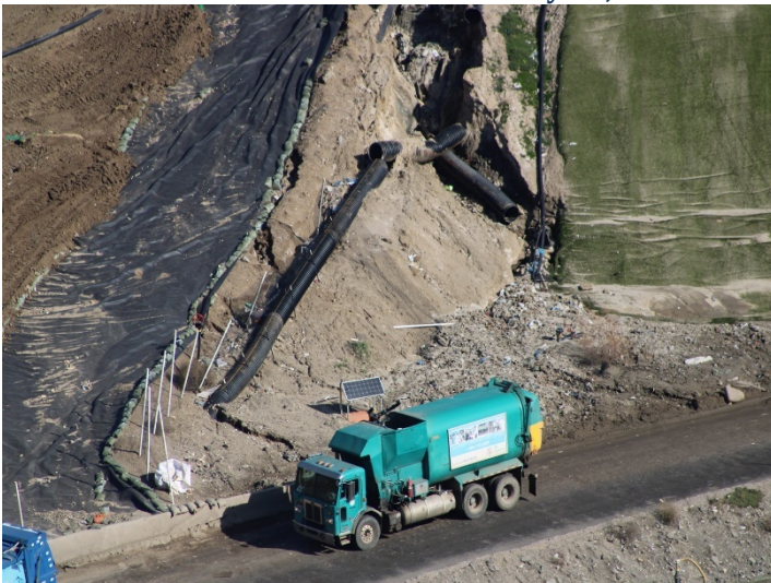
Photo 415: General Site: February 15, 2024
