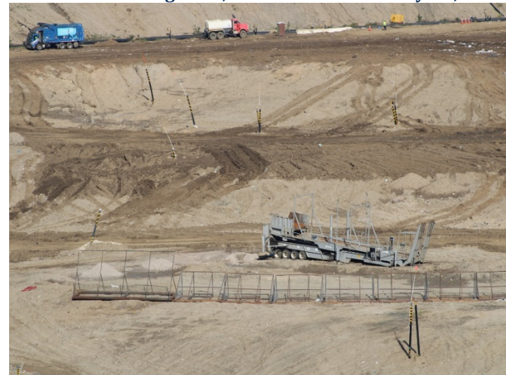
Photo 48: Working Area, CC-4 Part 3: February 15, 2024
