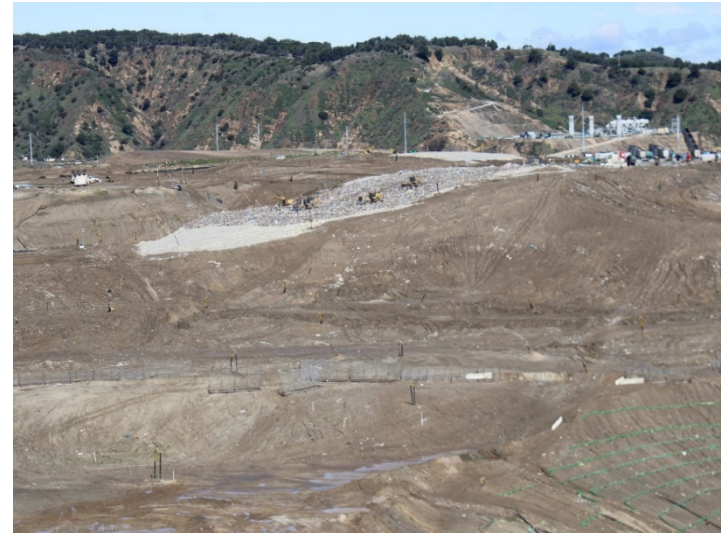
Photo 462: General Site: March 7, 2024
