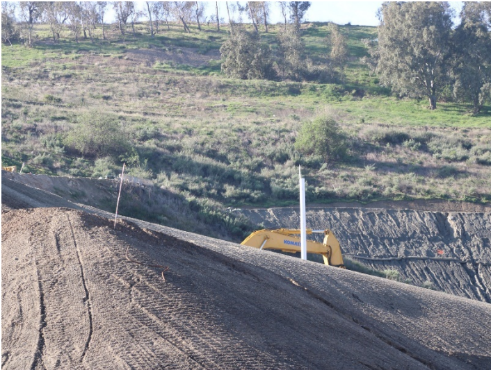
Photo 389: General Site: February 15, 2024
