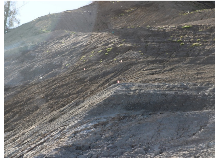
Photo 526: Road Realignment: January 8, 2024
