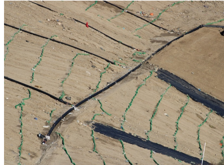
Photo 74: Working Area, CC-4 Part 4/5: January 8, 2024
