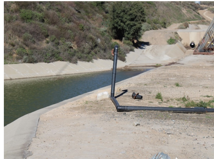
Photo 8: Basin A: January 8, 2024
