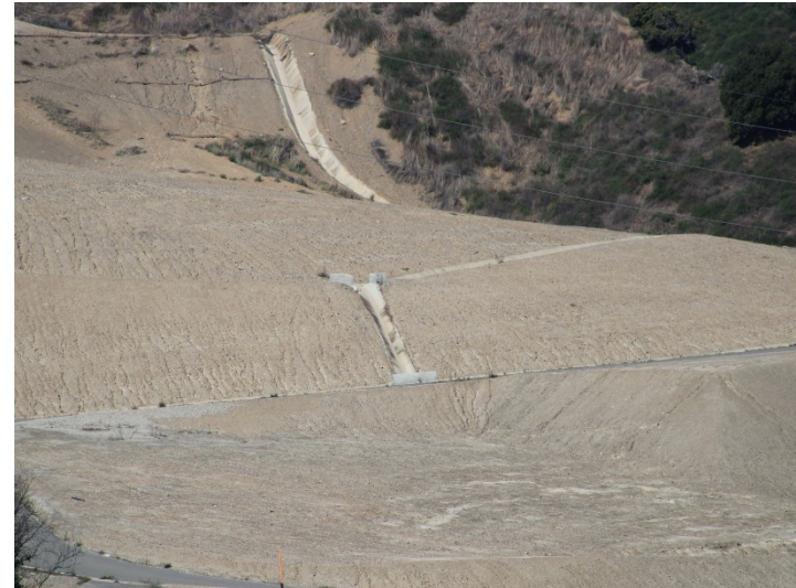
Photo 410: General Site: February 15, 2024
