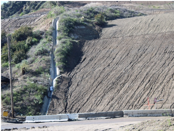
Photo 447: General Site: March 7, 2024
