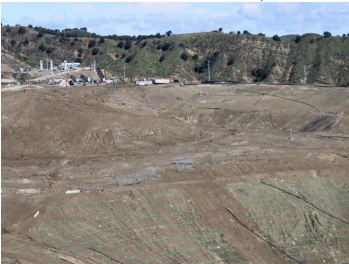
Photo 463: General Site: March 7, 2024
