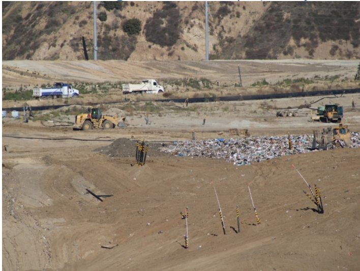
Photo 79: Working Area, CC-4 Part 4/5: January 8, 2024
