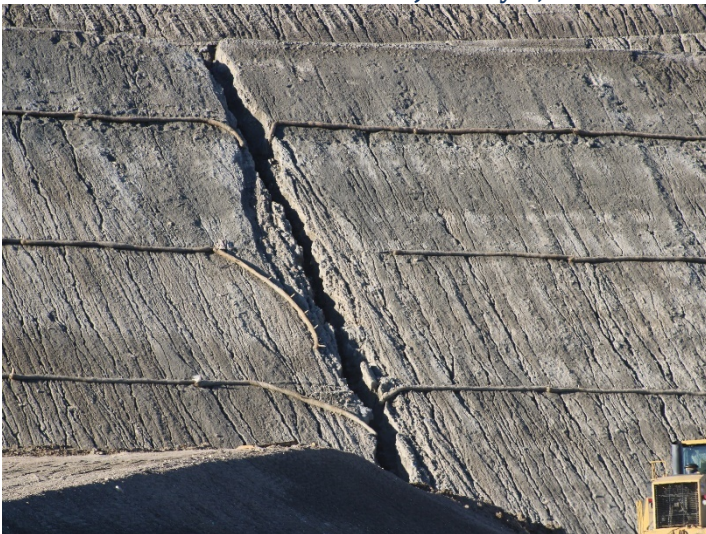
Photo 343: General Site: January 8, 2024
