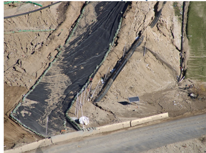
Photo 348: General Site: January 8, 2024
