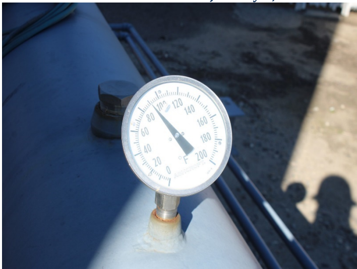
Photo 355: General Site: January 8, 2024
