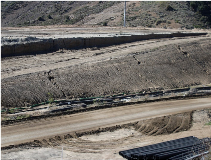
Photo 169: County Top Deck: January 8, 2024
