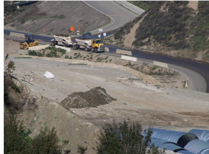
Photo 542: Road Realignment: February 15, 2024
