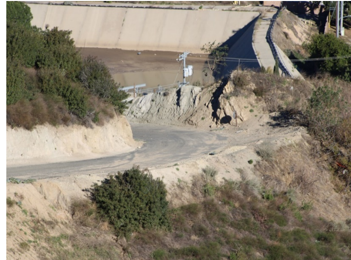
Photo 506: Road Realignment: January 8, 2024
