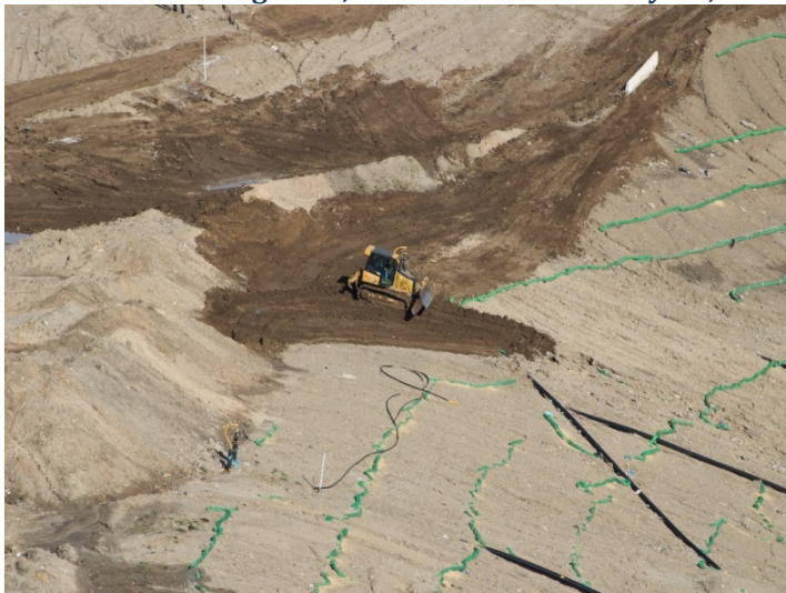
Photo 47: Working Area, CC-4 Part 3: February 15, 2024
