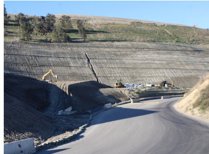
Photo 338: General Site: January 8, 2024
