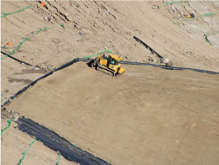
Photo 75: Working Area, CC-4 Part 4/5: January 8, 2024
