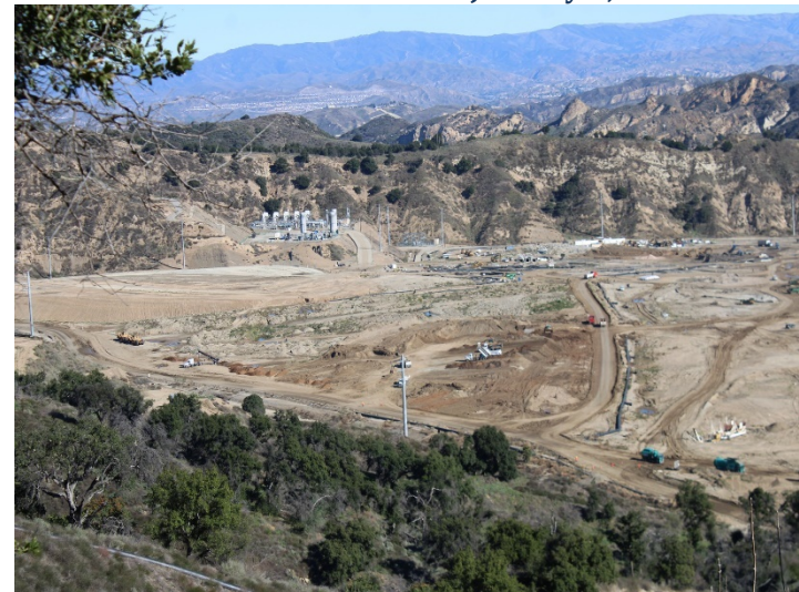
Photo 364: General Site: January 8, 2024
