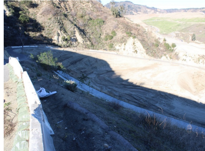
Photo 492: Road Realignment: January 8, 2024
