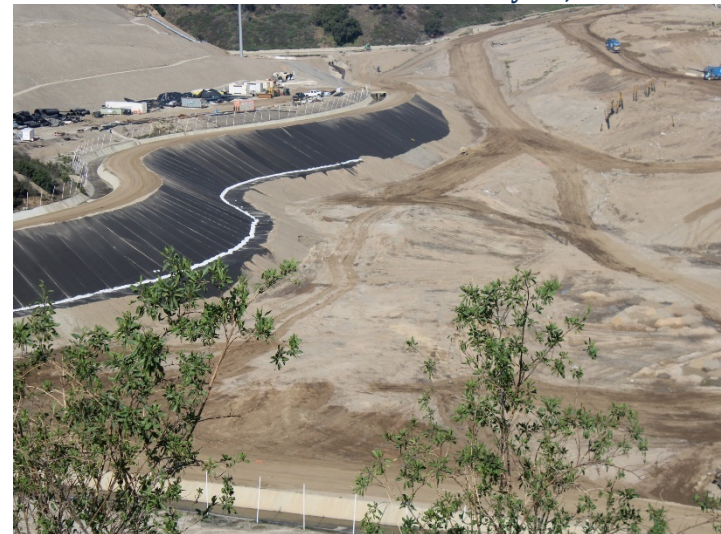
Photo 404: General Site: February 15, 2024
