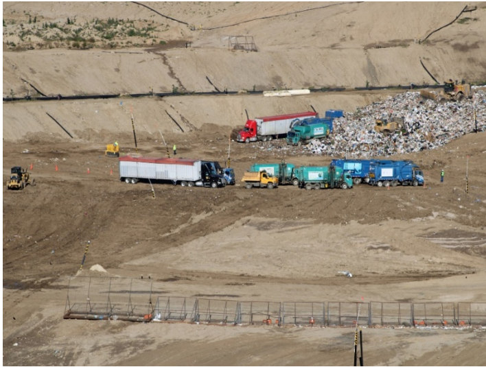
Photo 69: Working Area, CC-4 Part 4/5: January 8, 2024
