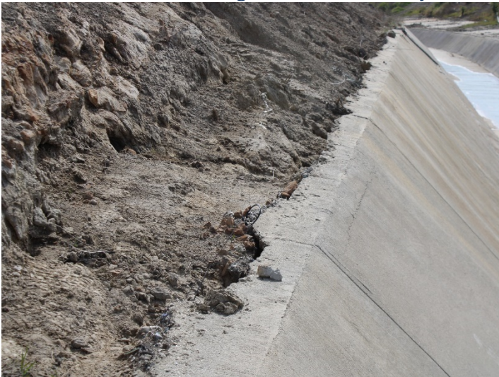
Photo 215: Eastside Drainage Channel: February 15, 2024
