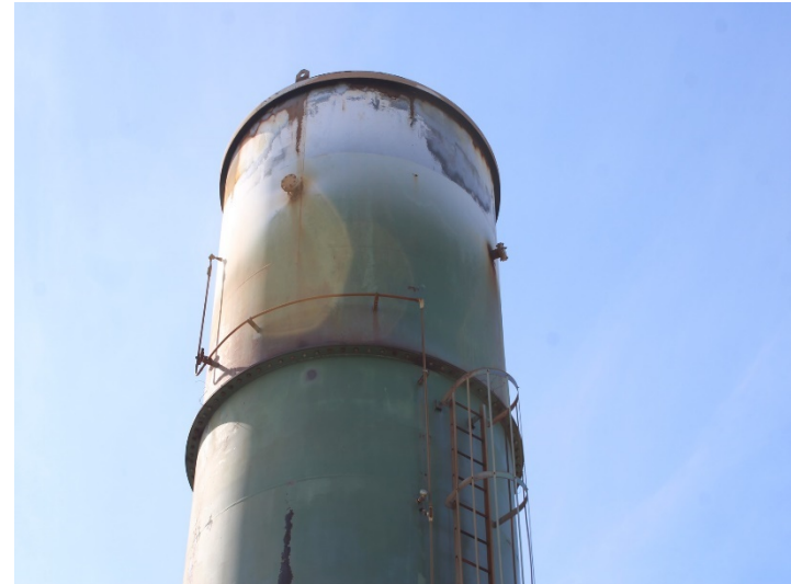
Photo 426: General Site: February 15, 2024
