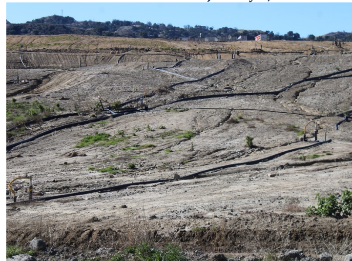
Photo 380: General Site: January 8, 2024
