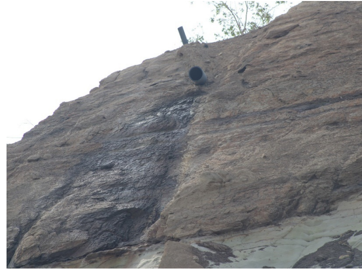
Photo 422: General Site: February 15, 2024
