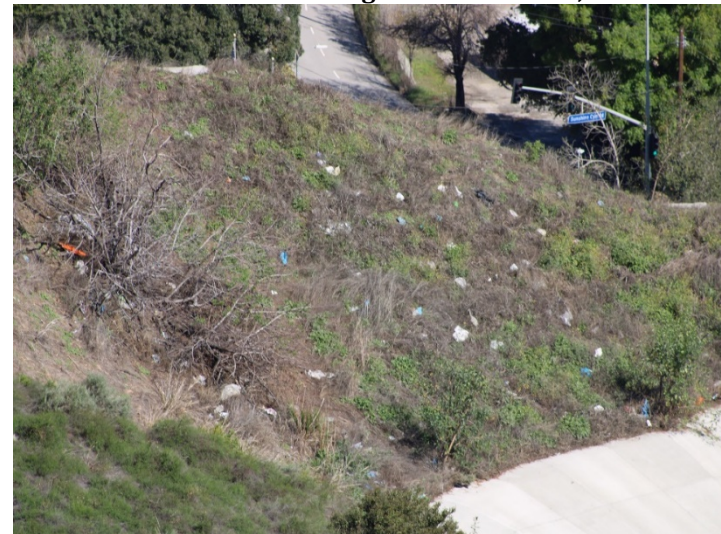
Photo 568: Road Realignment: March 7, 2024
