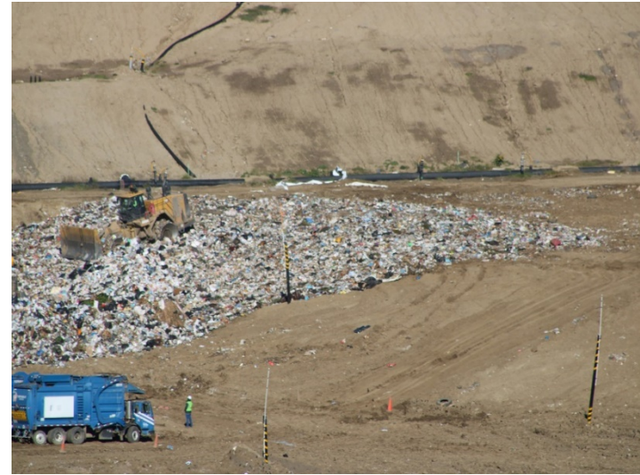
Photo 78: Working Area, CC-4 Part 4/5: January 8, 2024
