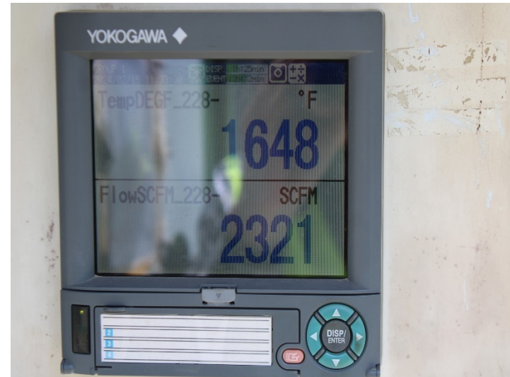
Photo 430: General Site: February 15, 2024
