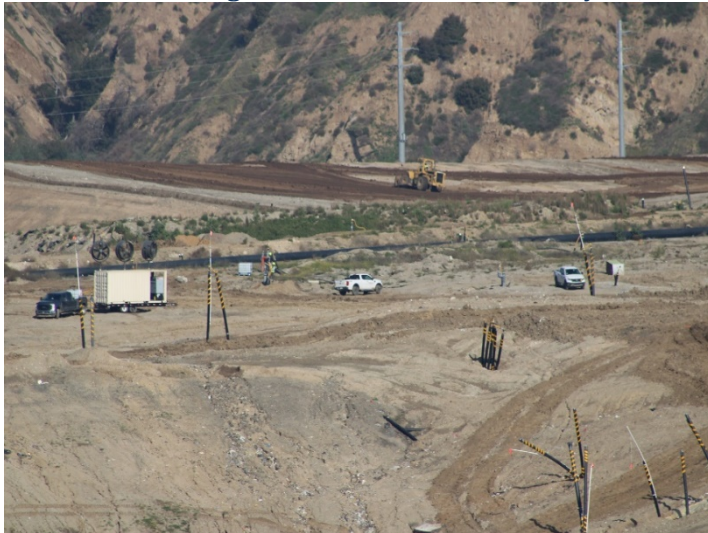
Photo 55: Working Area, CC-4 Part 3: February 15, 2024
