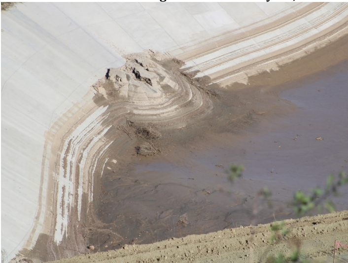
Photo 547: Road Realignment: February 15, 2024
