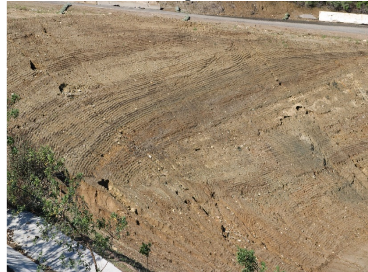
Photo 564: Road Realignment: March 7, 2024
