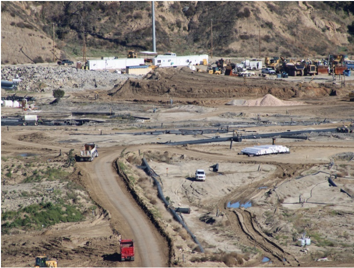
Photo 21: Working Area, CC4 Part 1/2: January 8, 2024
