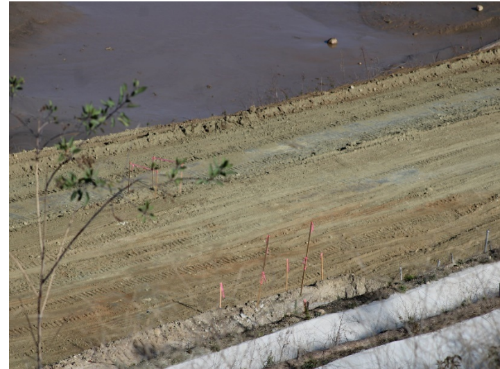
Photo 550: Road Realignment: February 15, 2024
