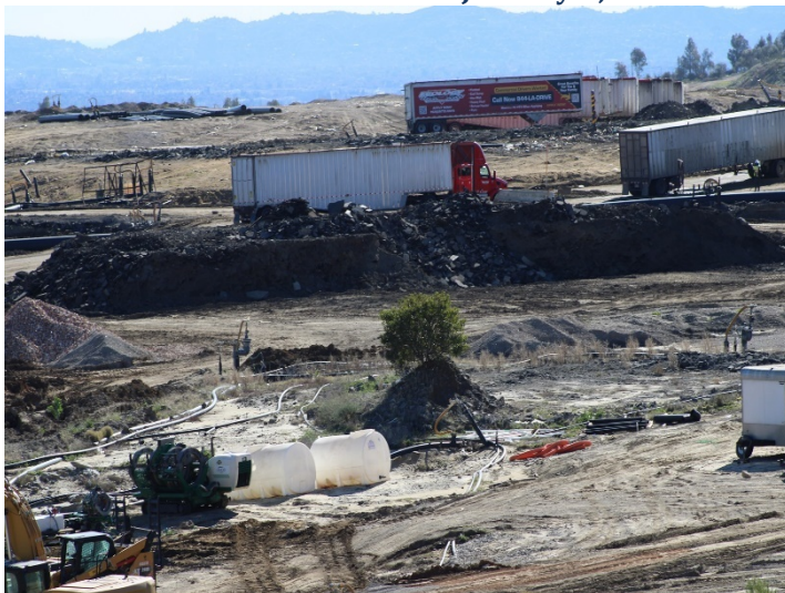
Photo 375: General Site: January 8, 2024
