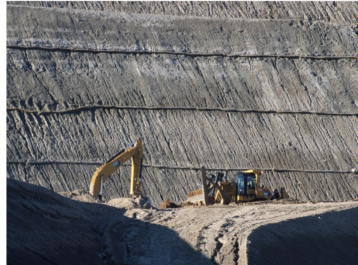
Photo 342: General Site: January 8, 2024
