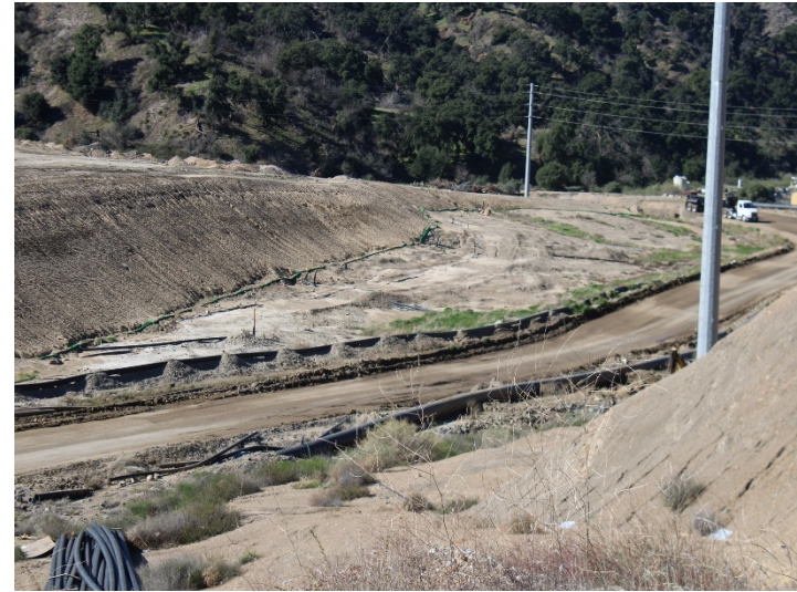
Photo 170: County Top Deck: January 8, 2024
