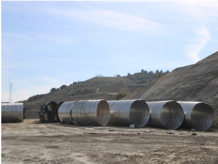
Photo 417: General Site: February 15, 2024
