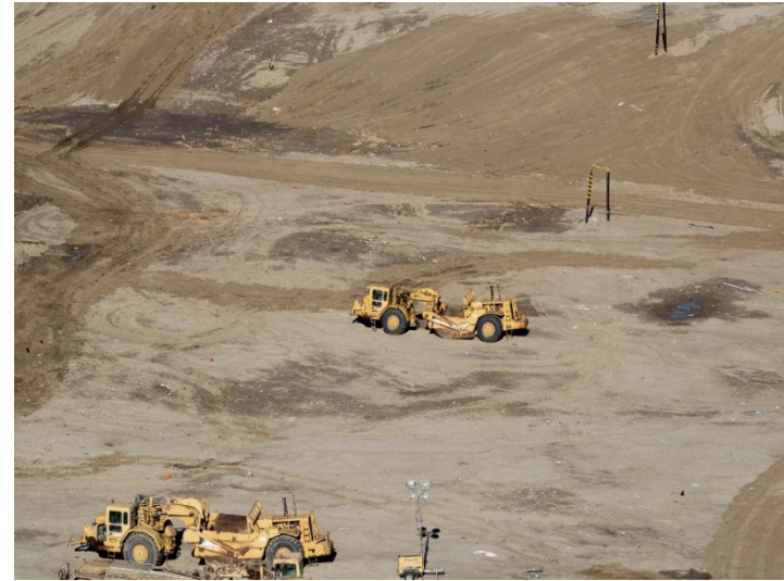
Photo 66: Working Area, CC-4 Part 4/5: January 8, 2024
