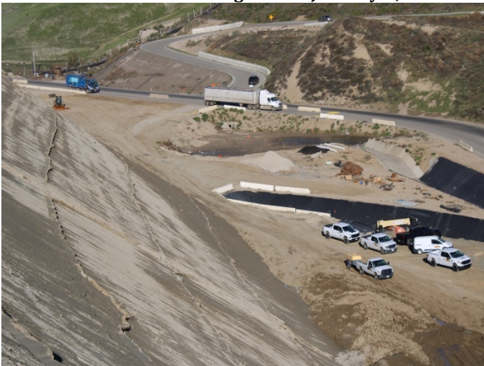
Photo 515: Road Realignment: January 8, 2024
