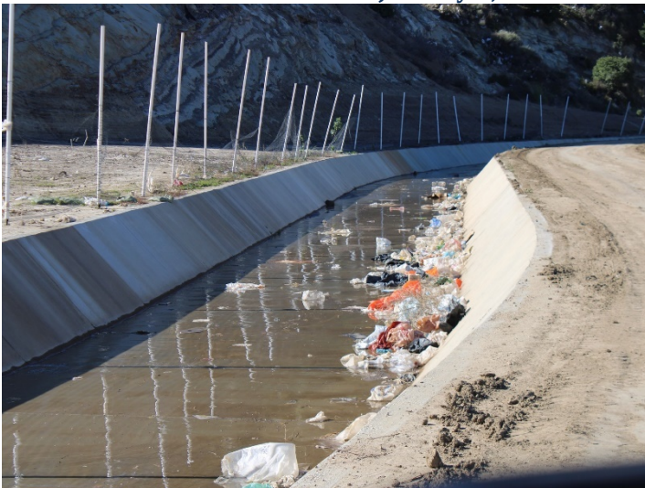
Photo 359: General Site: January 8, 2024
