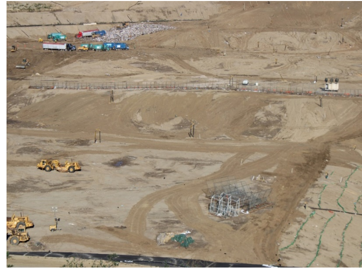
Photo 62: Working Area, CC-4 Part 4/5: January 8, 2024
