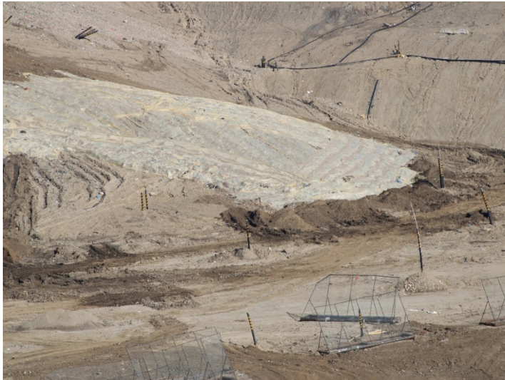
Photo 53: Working Area, CC-4 Part 3: February 15, 2024
