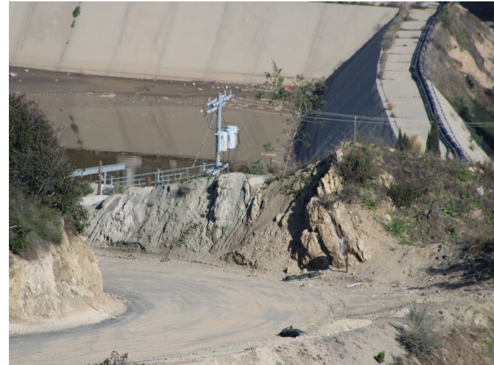
Photo 546: Road Realignment: February 15, 2024
