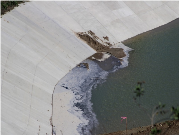
Photo 569: Road Realignment: March 7, 2024
