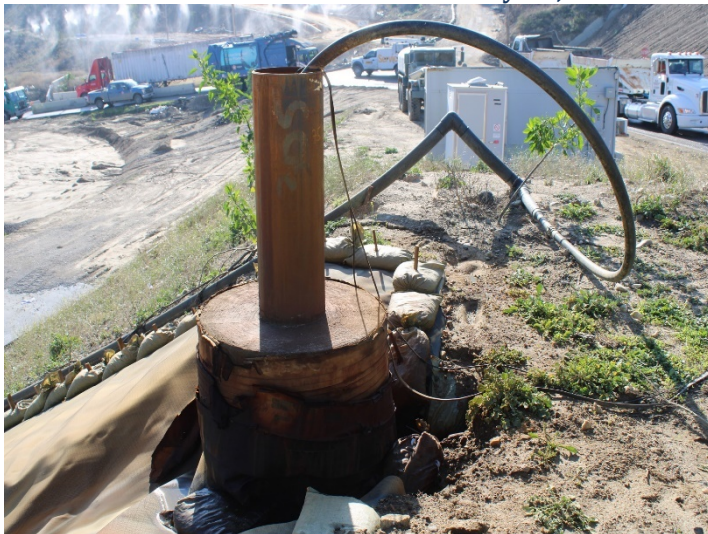
Photo 399: General Site: February 15, 2024
