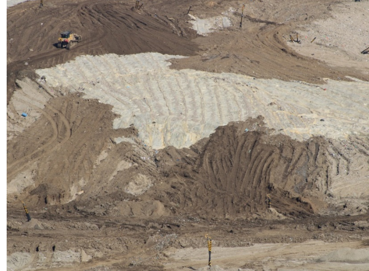
Photo 52: Working Area, CC-4 Part 3: February 15, 2024
