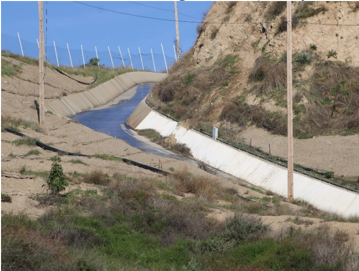
Photo 211: Eastside Drainage Channel: February 15, 2024
