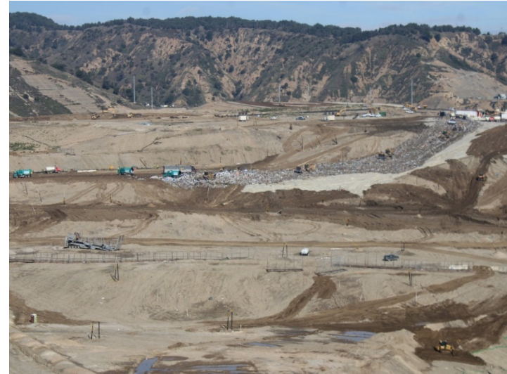
Photo 30: Working Area, CC4 Part 1/2: February 15, 2024
