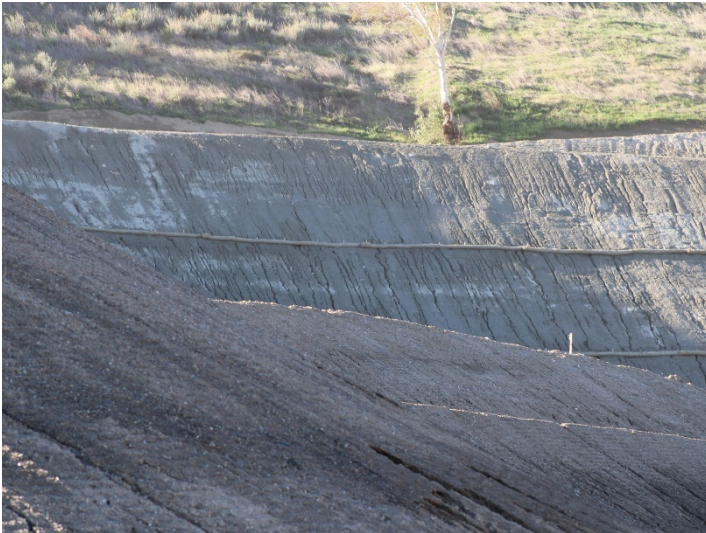
Photo 341: General Site: January 8, 2024
