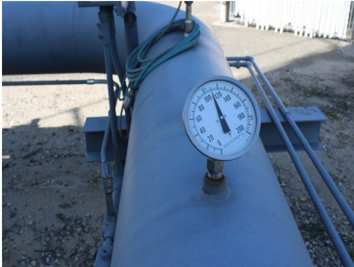
Photo 433: General Site: February 15, 2024
