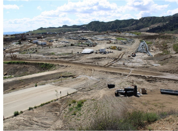
Photo 490: General Site: March 7, 2024
