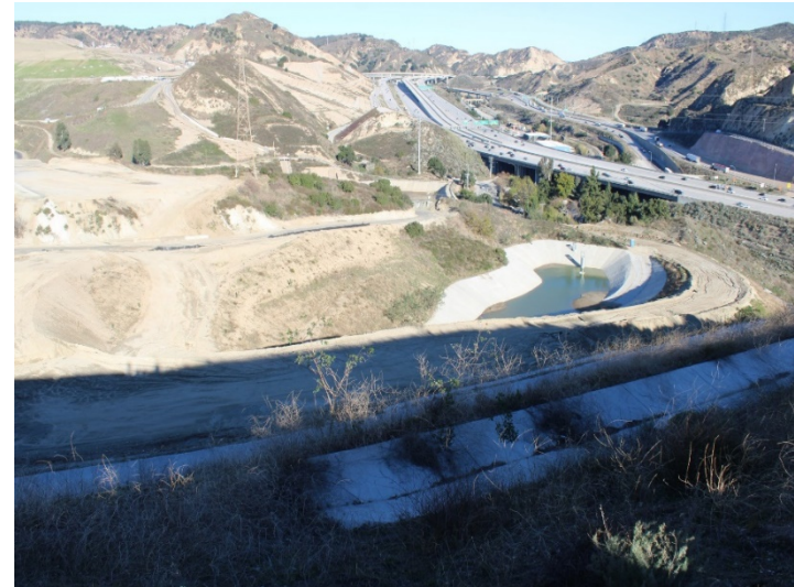
Photo 494: Road Realignment: January 8, 2024
