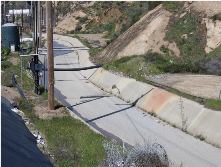
Photo 219: Eastside Drainage Channel: March 7, 2024
