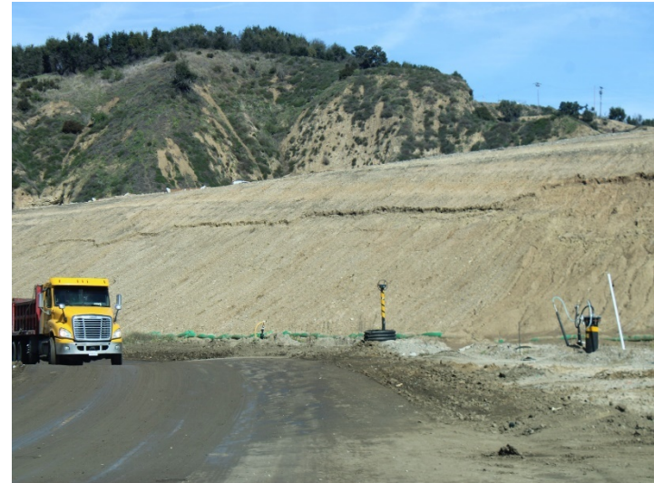
Photo 434: General Site: February 15, 2024
