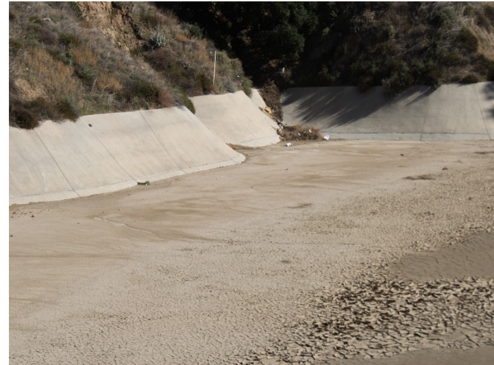
Photo 182: Basin B: January 8, 2024
