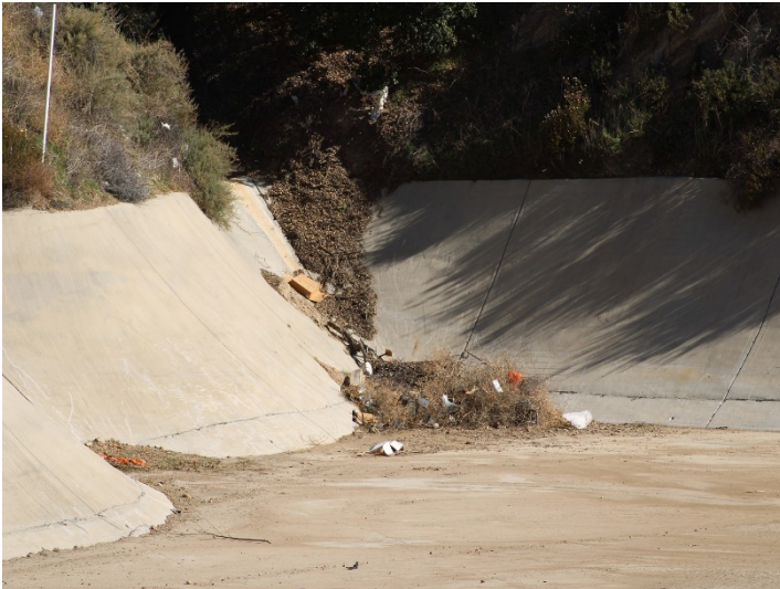
Photo 185: Basin B: January 8, 2024
