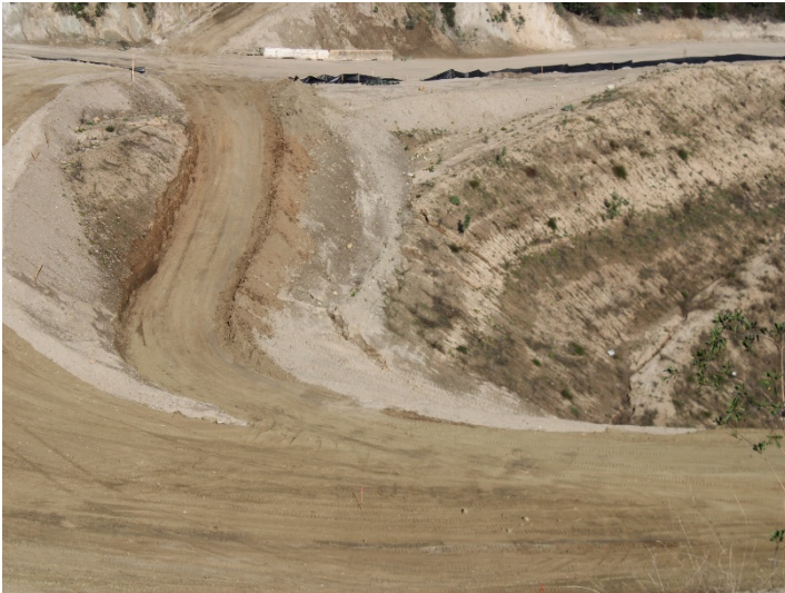
Photo 537: Road Realignment: February 15, 2024
