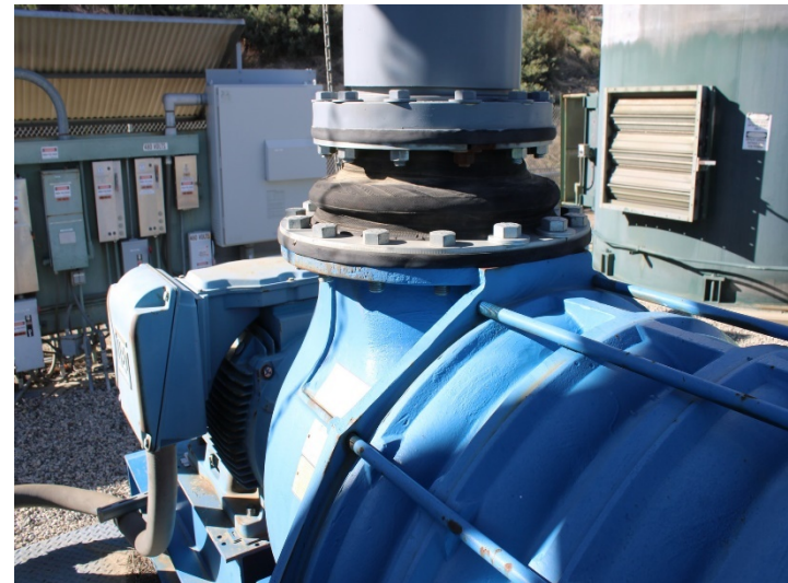
Photo 354: General Site: January 8, 2024
