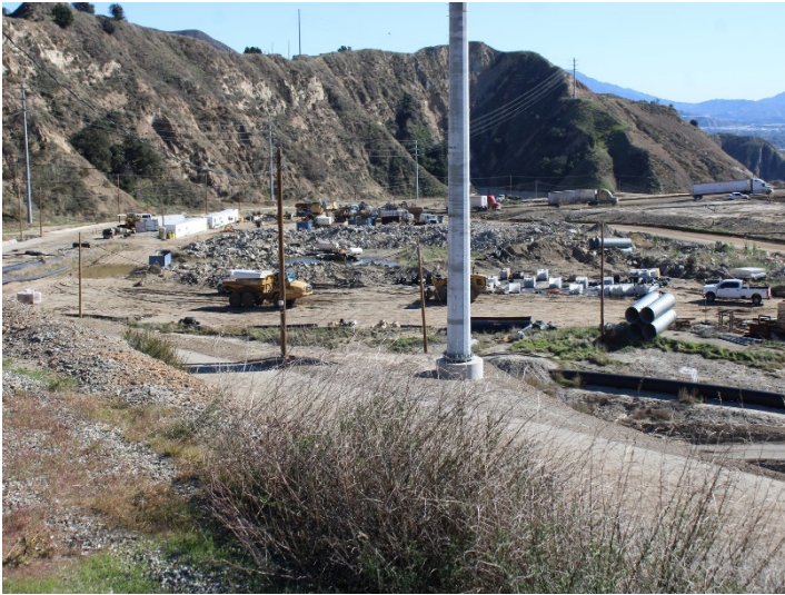
Photo 369: General Site: January 8, 2024
