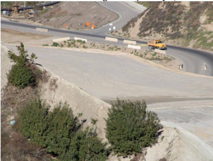
Photo 507: Road Realignment: January 8, 2024
