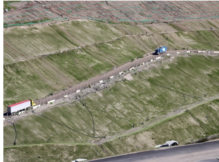
Photo 94: Closure Turf: March 7, 2024
