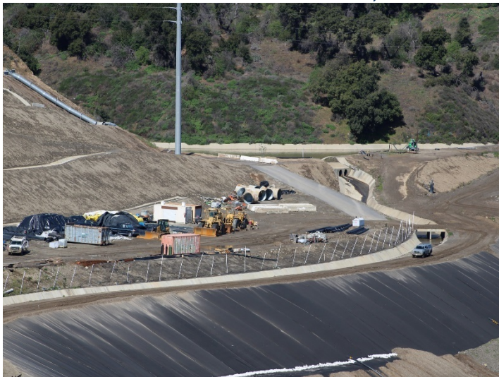
Photo 475: General Site: March 7, 2024
