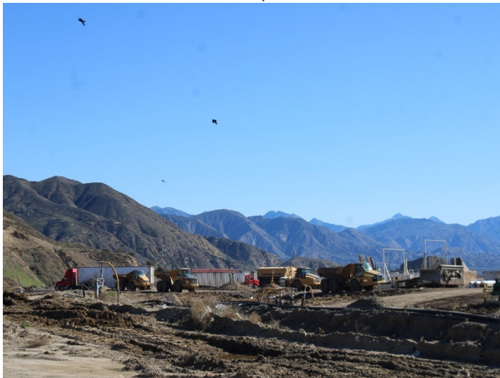
Photo 163: County Top Deck: January 8, 2024
