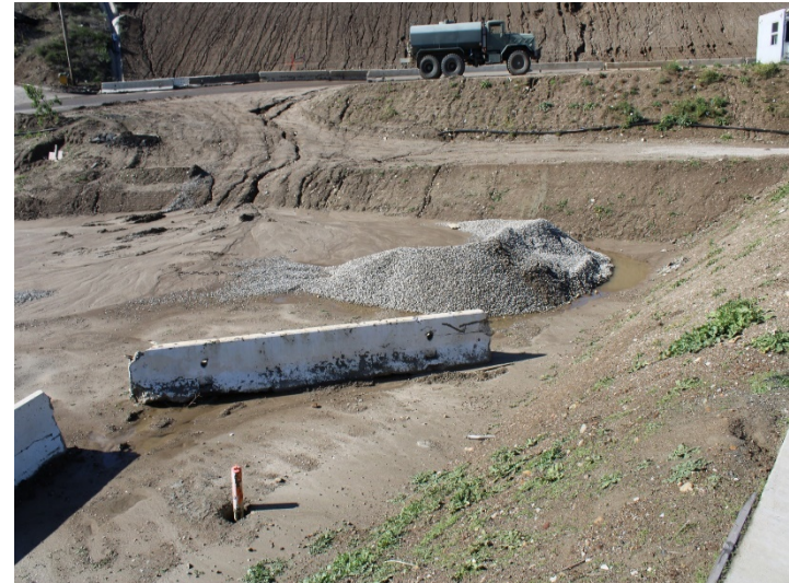
Photo 446: General Site: March 7, 2024
