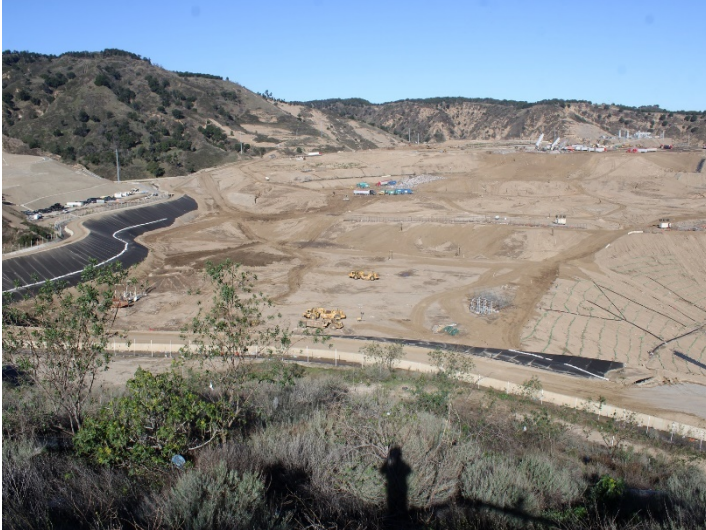
Photo 59: Working Area, CC-4 Part 4/5: January 8, 2024
