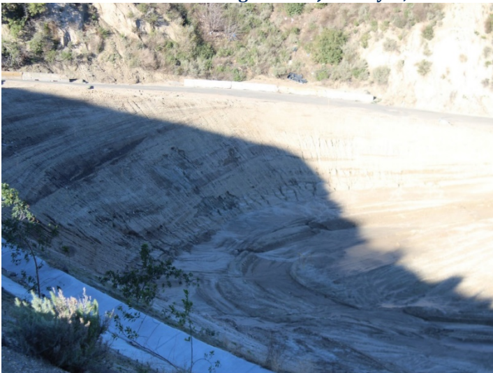
Photo 495: Road Realignment: January 8, 2024
