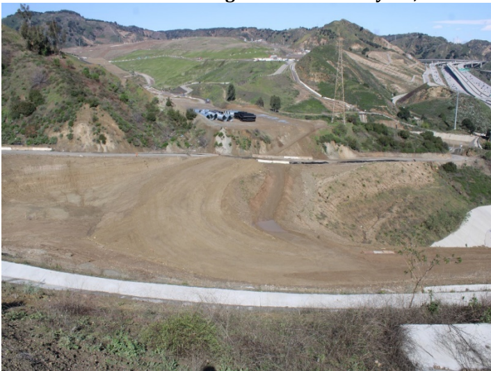
Photo 555: Road Realignment: March 7, 2024
