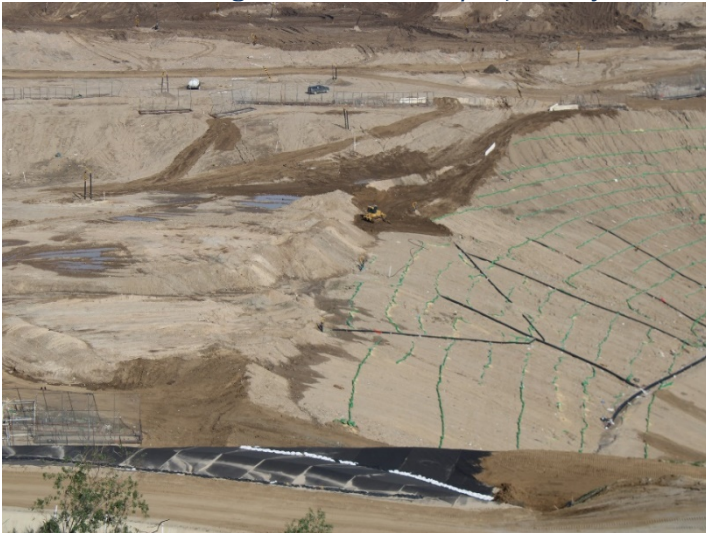
Photo 27: Working Area, CC4 Part 1/2: February 15, 2024
