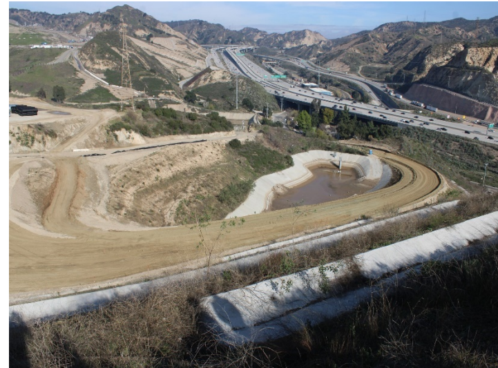
Photo 534: Road Realignment: February 15, 2024
