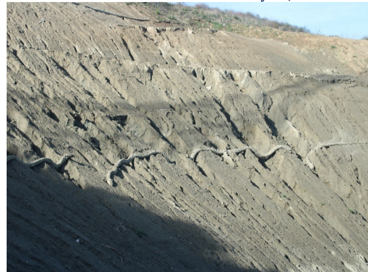
Photo 400: General Site: February 15, 2024
