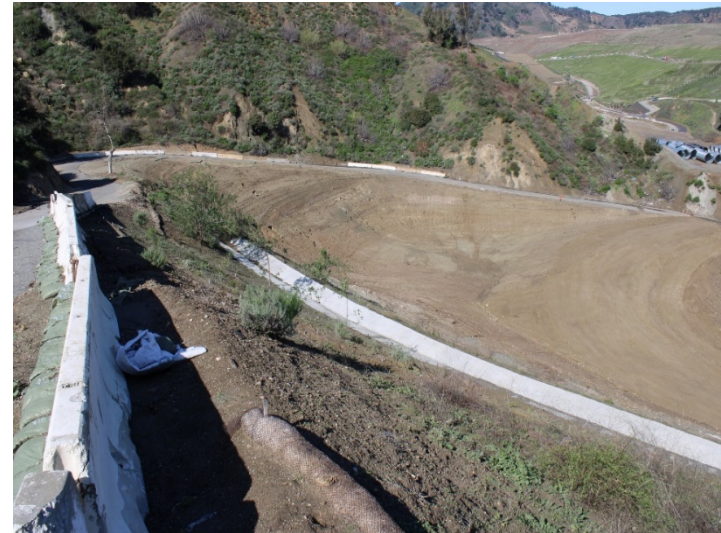
Photo 554: Road Realignment: March 7, 2024
