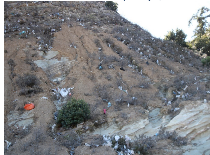
Photo 360: General Site: January 8, 2024
