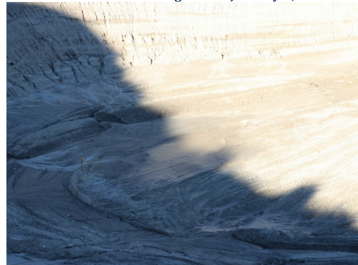
Photo 500: Road Realignment: January 8, 2024
