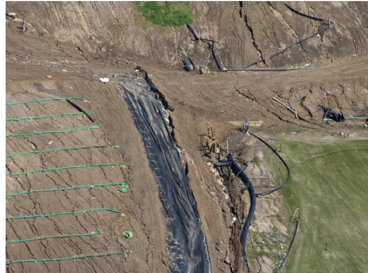
Photo 470: General Site: March 7, 2024
