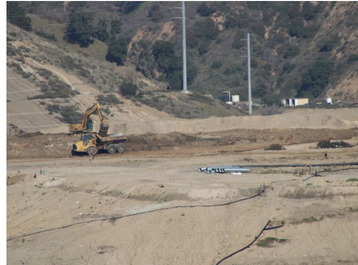
Photo 54: Working Area, CC-4 Part 3: February 15, 2024
