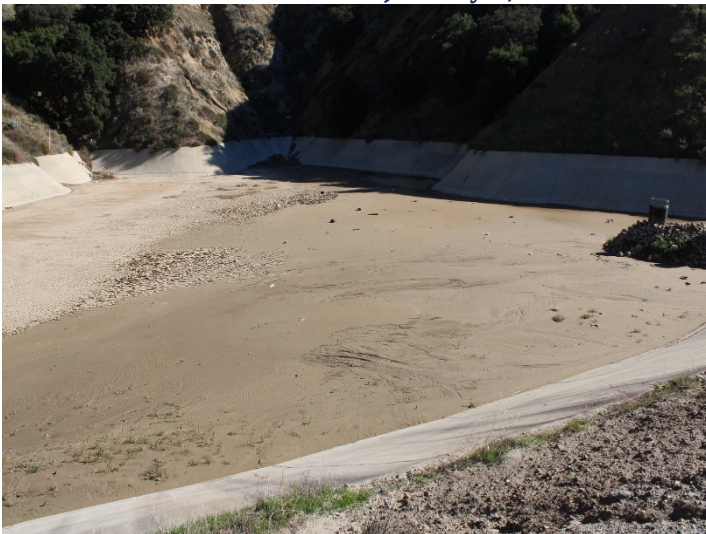
Photo 179: Basin B: January 8, 2024
