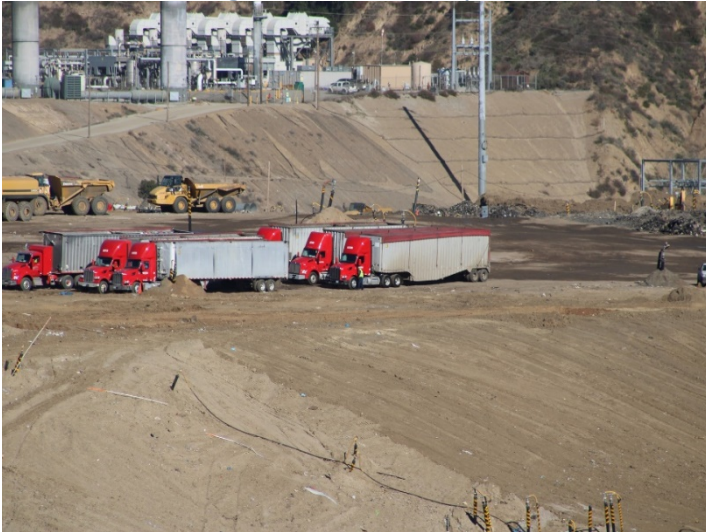
Photo 83: Working Area, CC-4 Part 4/5: January 8, 2024
