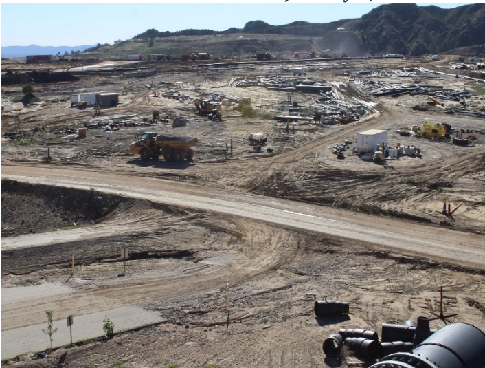
Photo 371: General Site: January 8, 2024
