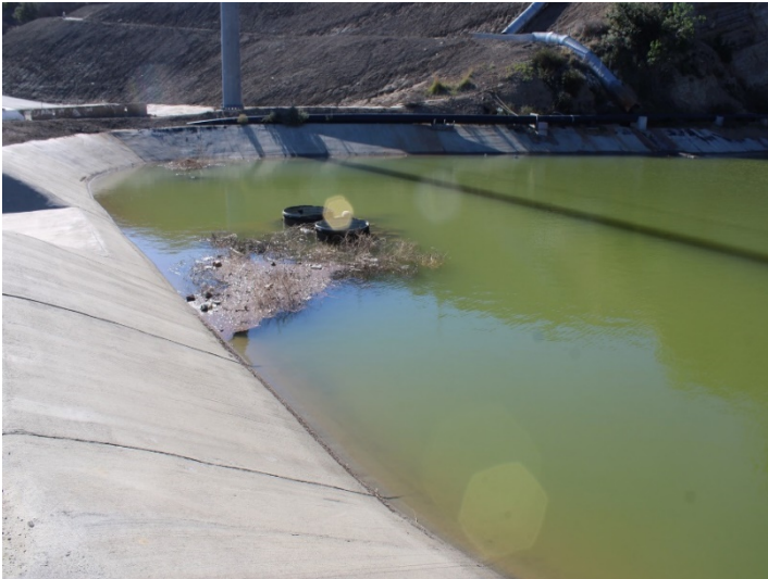
Photo 1: Basin A: January 8, 2024
