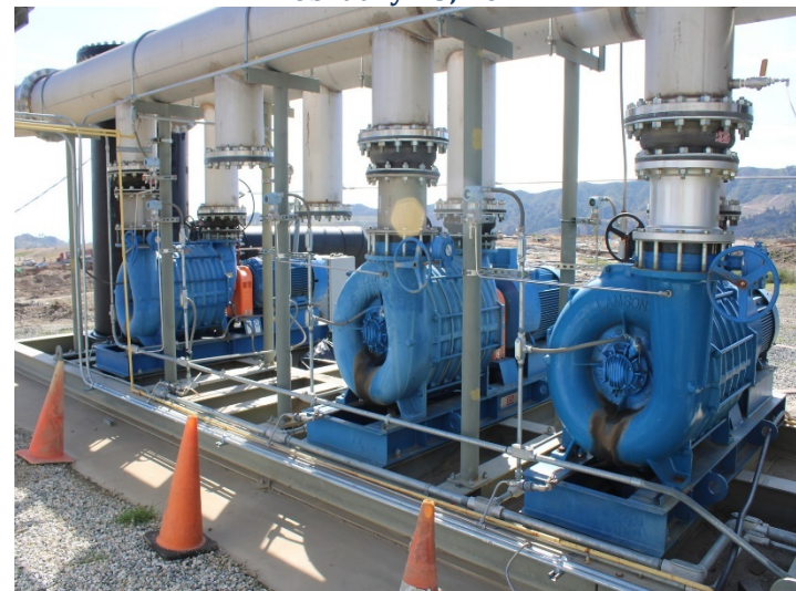
Photo 136: Flares 9, 10, 11 and Gas-to-Energy Facility: February 15, 2024
