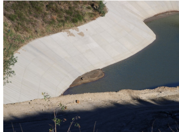
Photo 502: Road Realignment: January 8, 2024
