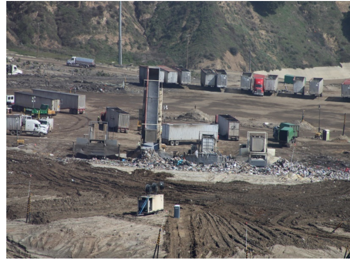
Photo 34: Working Area, CC4 Part 1/2: February 15, 2024
