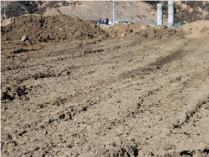
Photo 385: General Site: January 8, 2024
