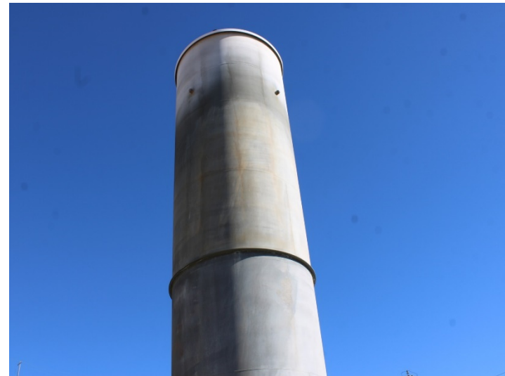
Photo 114: Flares 9, 10, 11 and Gas-to-Energy Facility: January 8, 2024
