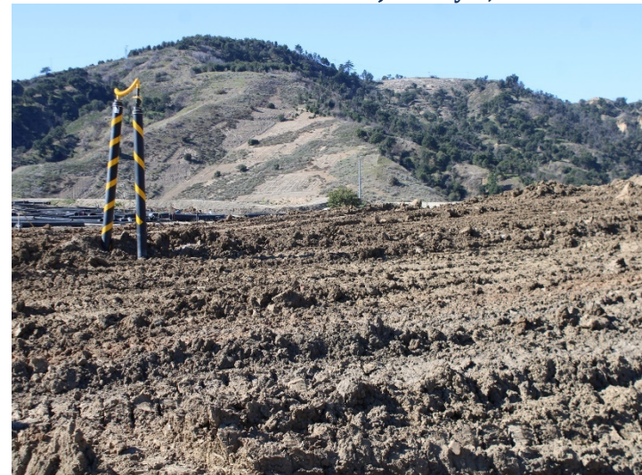
Photo 384: General Site: January 8, 2024
