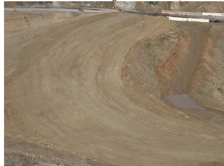
Photo 560: Road Realignment: March 7, 2024
