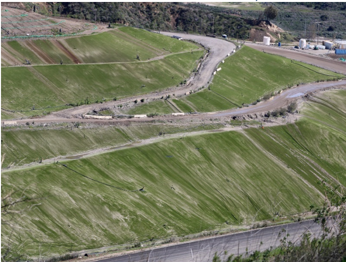
Photo 95: Closure Turf: March 7, 2024
