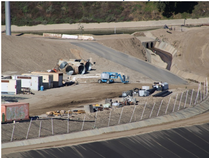
Photo 351: General Site: January 8, 2024
