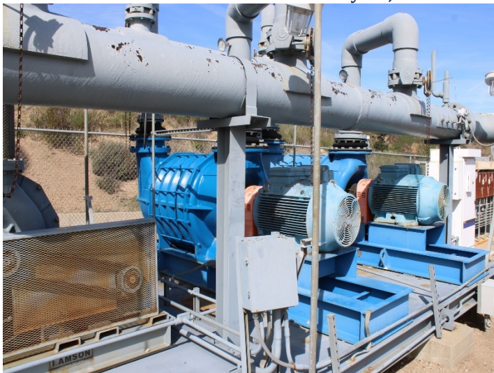
Photo 427: General Site: February 15, 2024
