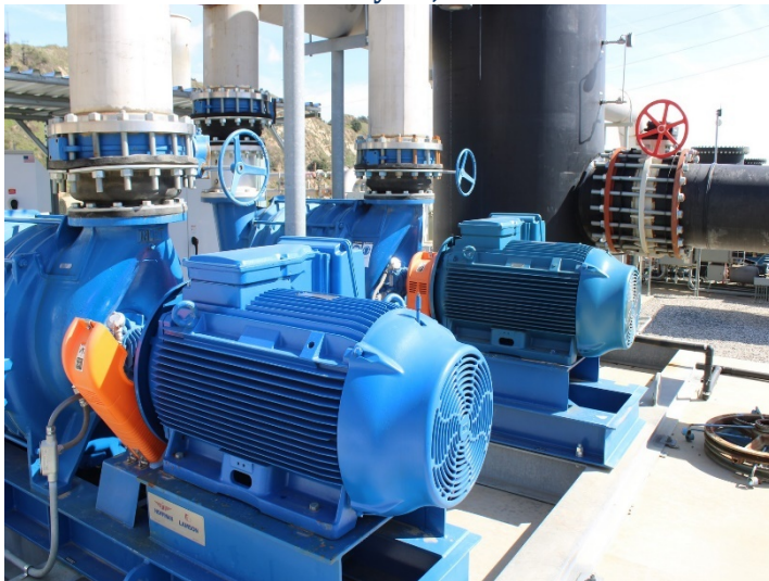
Photo 139: Flares 9, 10, 11 and Gas-to-Energy Facility: February 15, 2024
