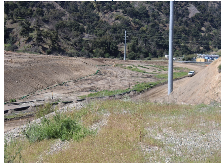
Photo 176: County Top Deck: March 7, 2024
