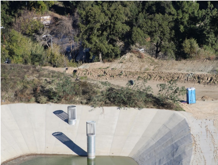
Photo 505: Road Realignment: January 8, 2024
