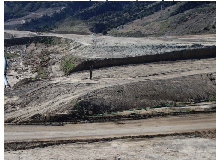
Photo 168: County Top Deck: January 8, 2024
