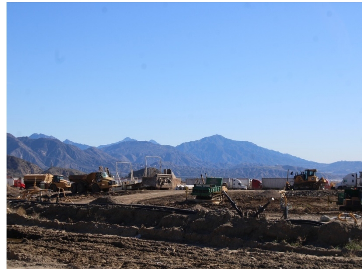
Photo 164: County Top Deck: January 8, 2024
