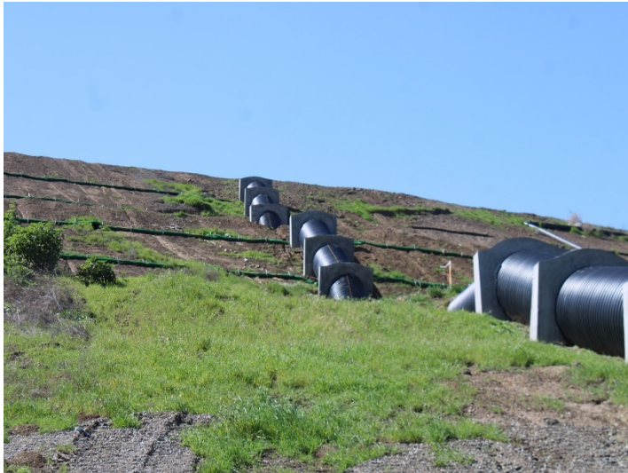
Photo 481: General Site: March 7, 2024
