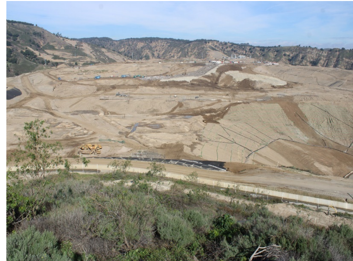
Photo 402: General Site: February 15, 2024
