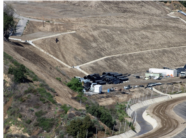
Photo 474: General Site: March 7, 2024
