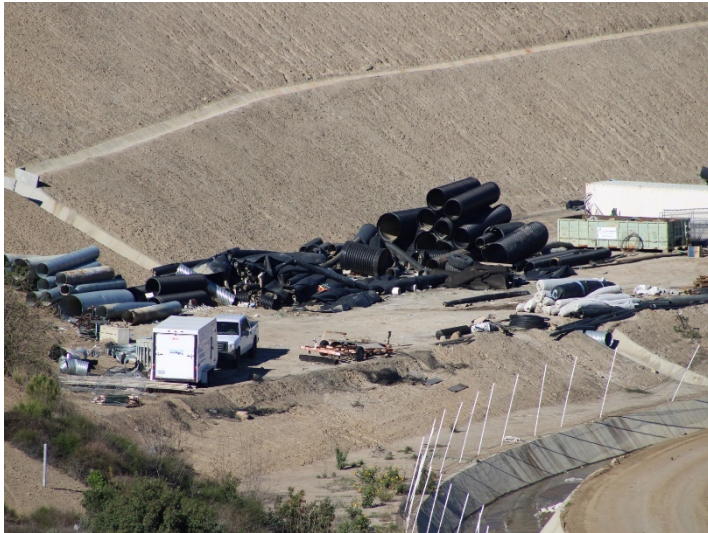
Photo 349: General Site: January 8, 2024
