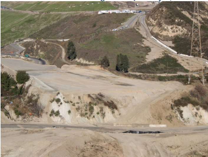
Photo 499: Road Realignment: January 8, 2024
