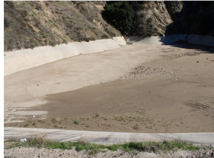
Photo 178: Basin B: January 8, 2024
