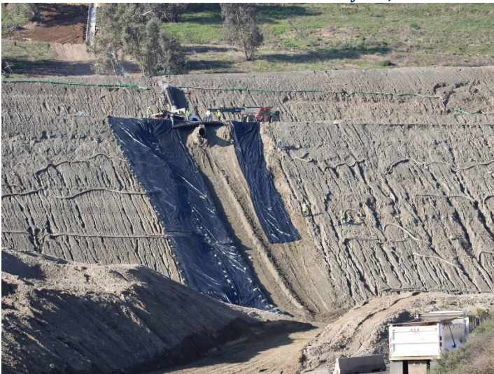
Photo 391: General Site: February 15, 2024
