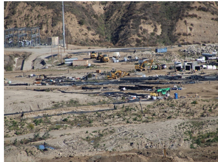
Photo 20: Working Area, CC4 Part 1/2: January 8, 2024
