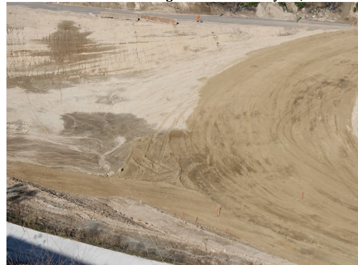
Photo 536: Road Realignment: February 15, 2024
