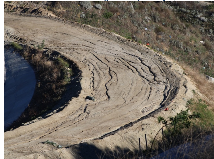
Photo 504: Road Realignment: January 8, 2024
