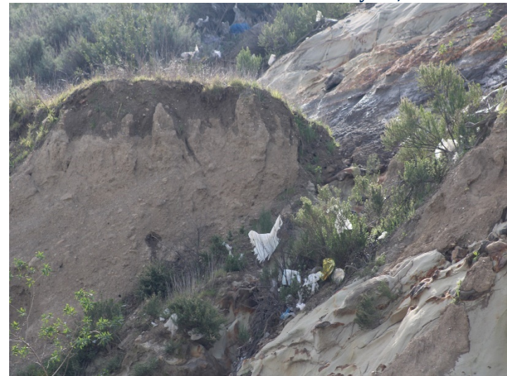
Photo 424: General Site: February 15, 2024
