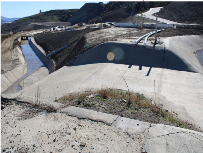
Photo 207: Eastside Drainage Channel: January 8, 2024
