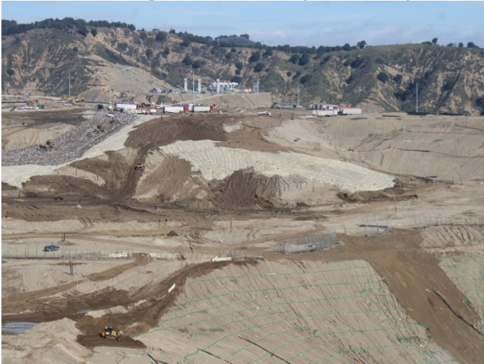
Photo 31: Working Area, CC4 Part 1/2: February 15, 2024
