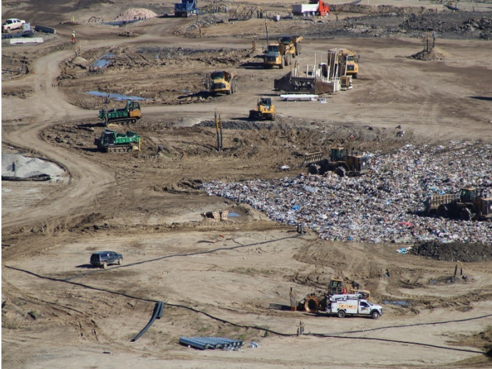
Photo 23: Working Area, CC4 Part 1/2: January 8, 2024
