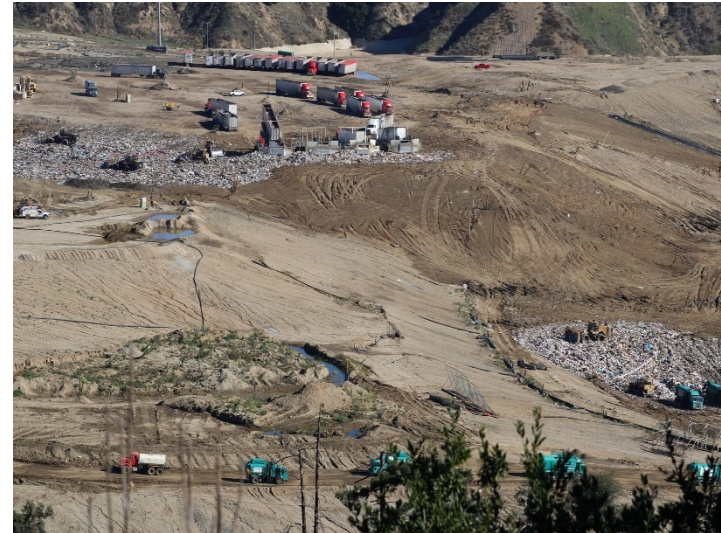
Photo 18: Working Area, CC4 Part 1/2: January 8, 2024
