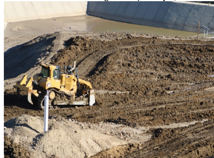
Photo 520: Road Realignment: January 8, 2024
