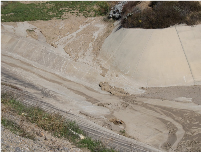
Photo 181: Basin B: January 8, 2024
