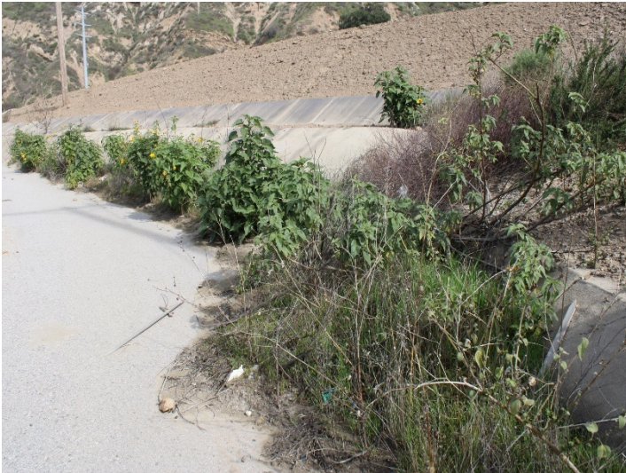
Photo 213: Eastside Drainage Channel: February 15, 2024
