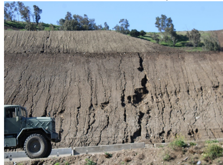
Photo 448: General Site: March 7, 2024
