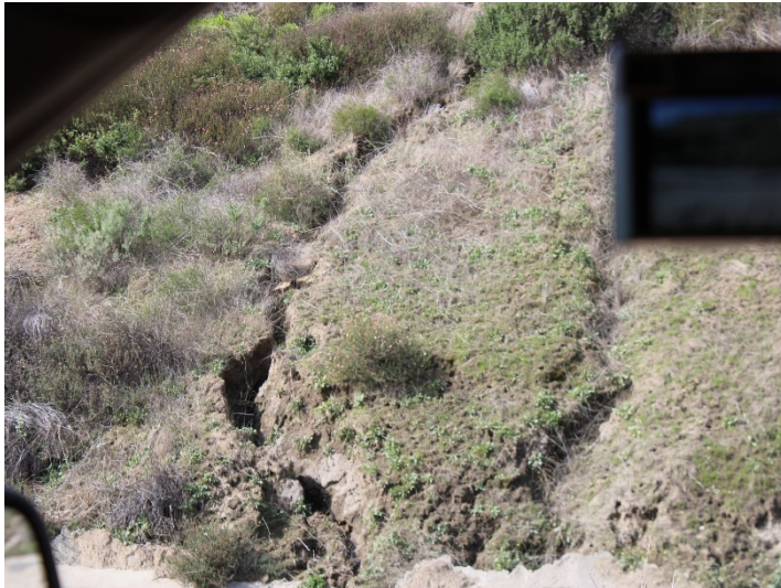
Photo 425: General Site: February 15, 2024
