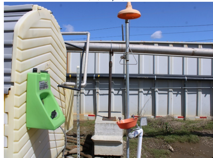
Photo 104: Alder Tank Liquids Treatment System: March 7, 2024
