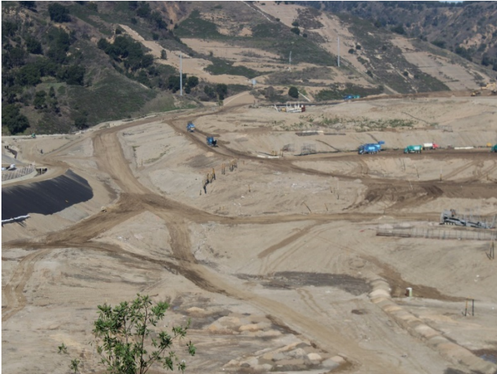
Photo 29: Working Area, CC4 Part 1/2: February 15, 2024
