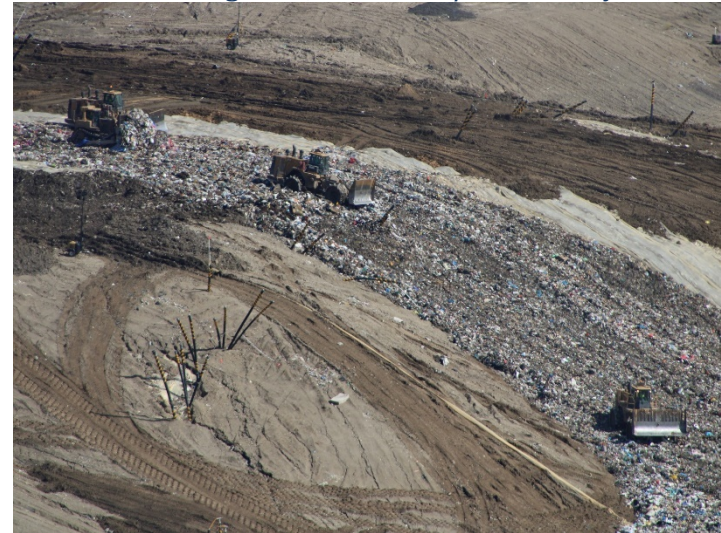
Photo 36: Working Area, CC4 Part 1/2: February 15, 2024
