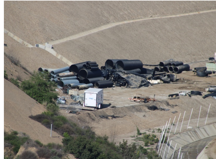
Photo 406: General Site: February 15, 2024
