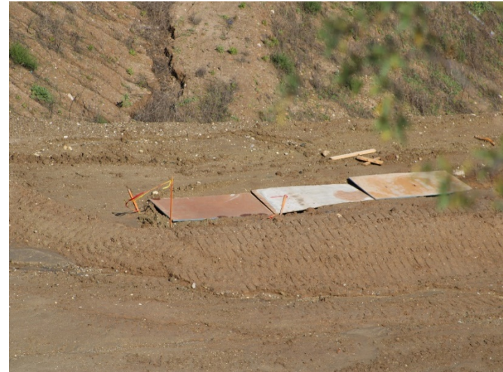
Photo 566: Road Realignment: March 7, 2024
