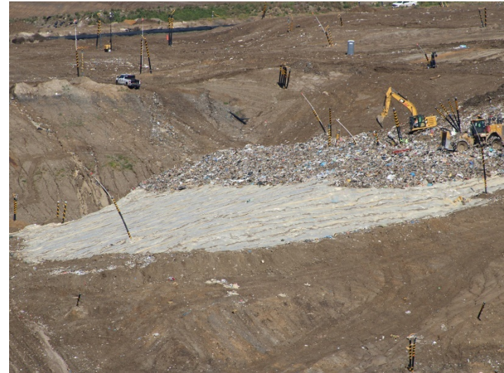
Photo 42: Working Area, CC4 Part 1/2: March 7, 2024
