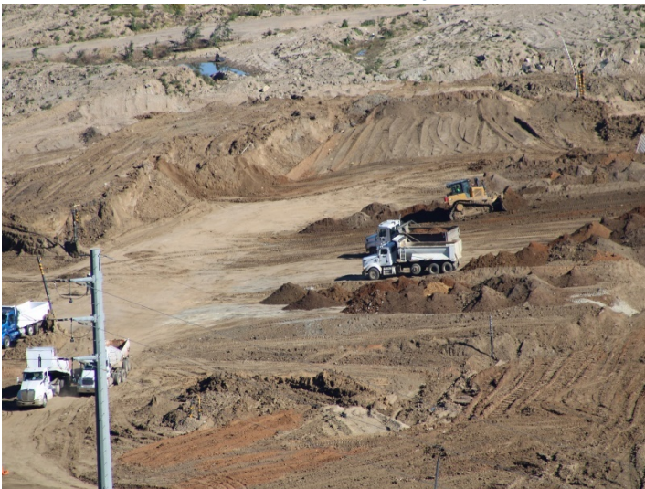
Photo 19: Working Area, CC4 Part 1/2: January 8, 2024
