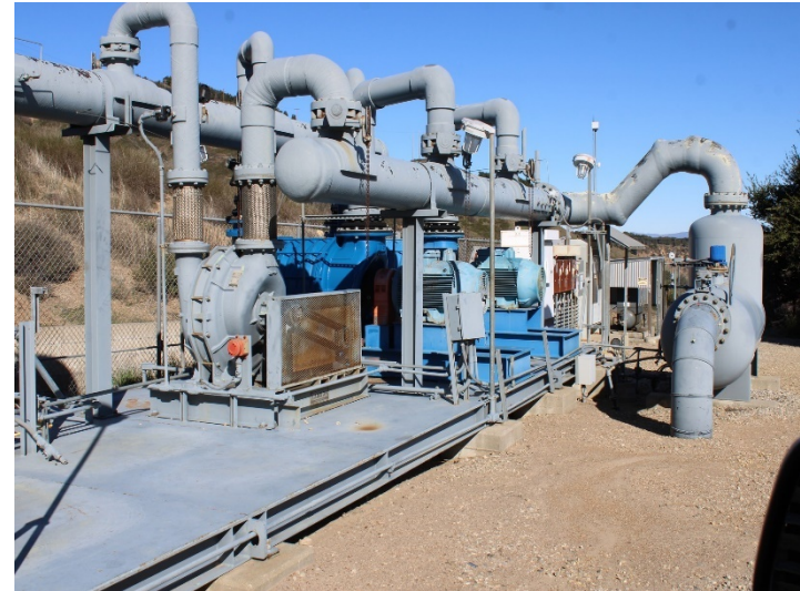
Photo 362: General Site: January 8, 2024
