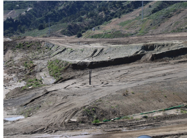
Photo 174: County Top Deck: March 7, 2024
