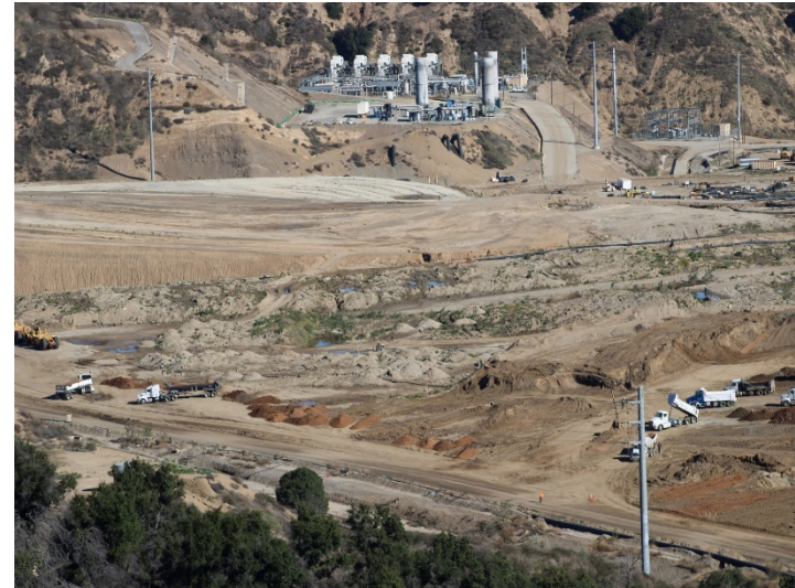
Photo 366: General Site: January 8, 2024
