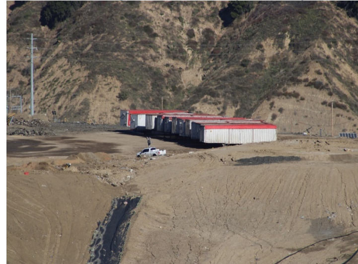
Photo 84: Working Area, CC-4 Part 4/5: January 8, 2024
