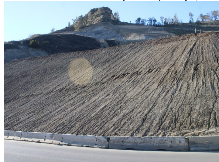
Photo 336: General Site: January 8, 2024
