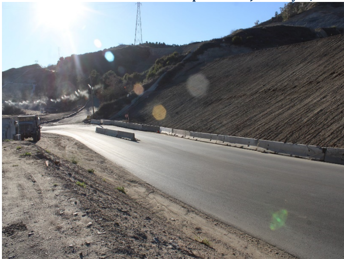
Photo 335: General Site: January 8, 2024
