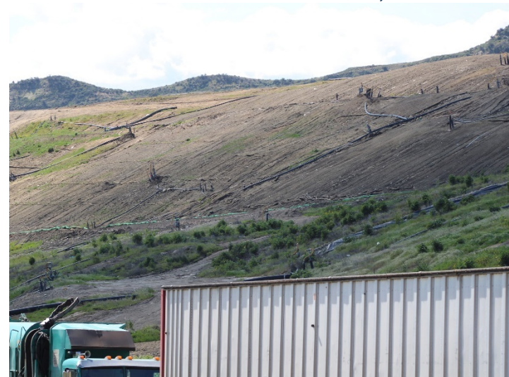
Photo 484: General Site: March 7, 2024
