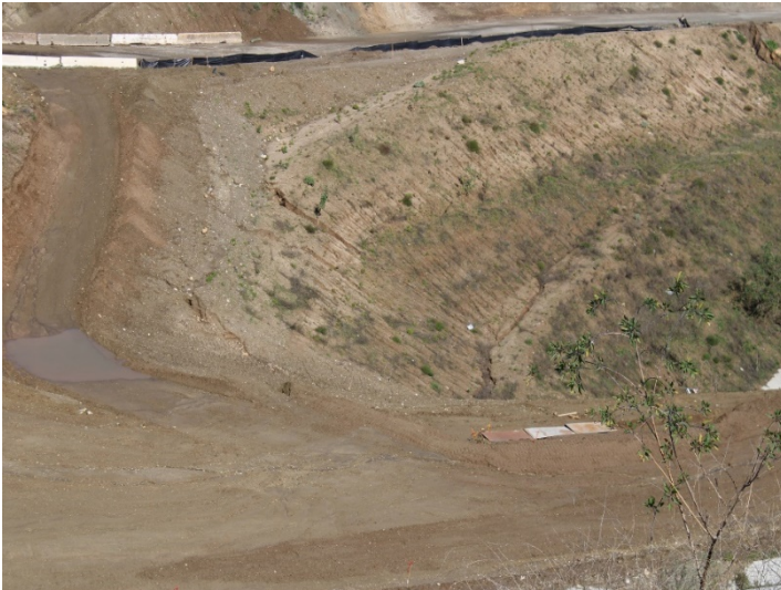
Photo 561: Road Realignment: March 7, 2024
