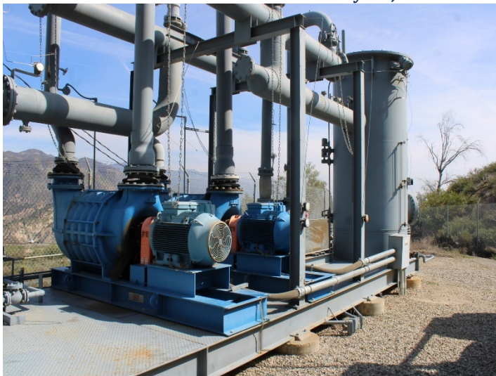
Photo 431: General Site: February 15, 2024
