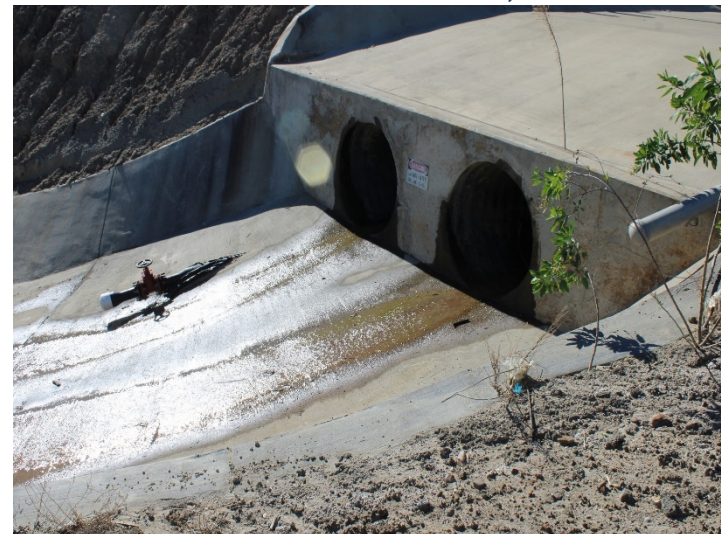
Photo 208: Eastside Drainage Channel: January 8, 2024
