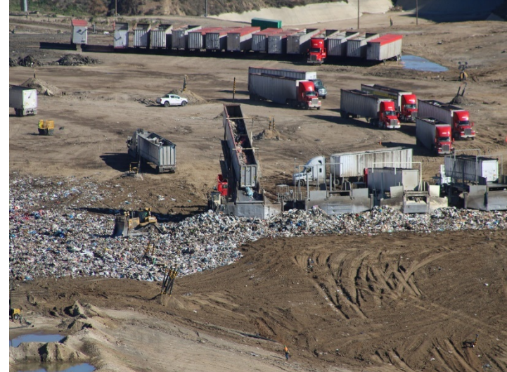
Photo 24: Working Area, CC4 Part 1/2: January 8, 2024
