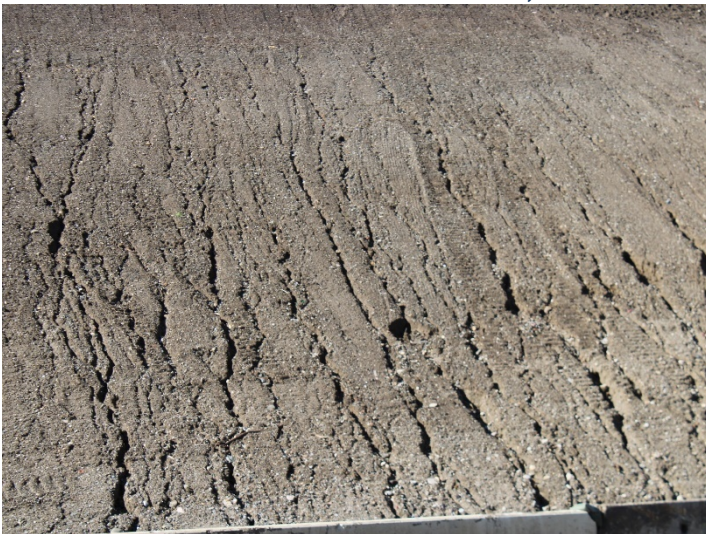
Photo 451: General Site: March 7, 2024
