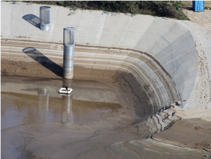
Photo 549: Road Realignment: February 15, 2024
