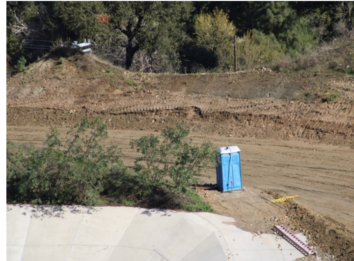
Photo 574: Road Realignment: March 7, 2024
