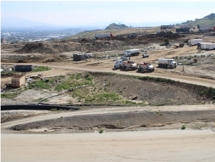
Photo 437: General Site: February 15, 2024
