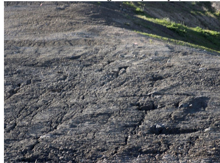
Photo 528: Road Realignment: January 8, 2024
