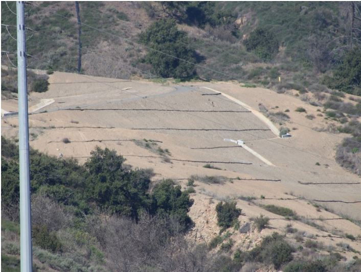
Photo 409: General Site: February 15, 2024
