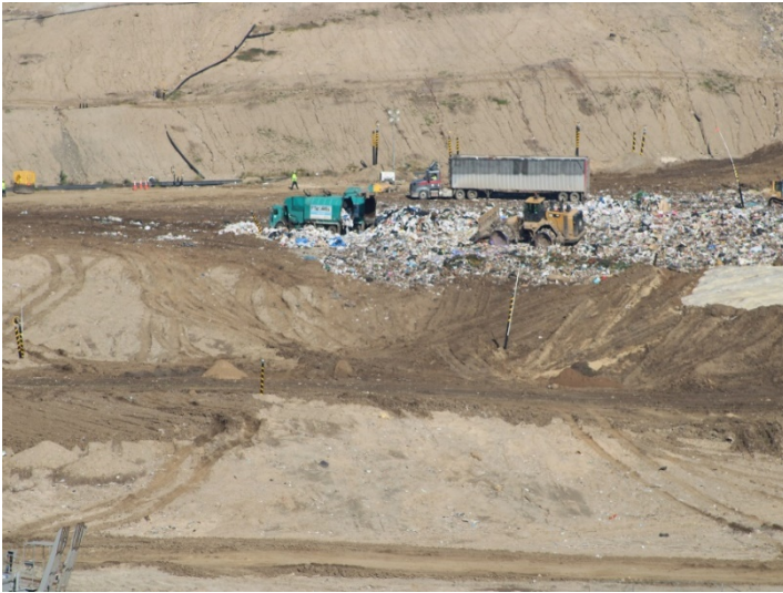
Photo 49: Working Area, CC-4 Part 3: February 15, 2024
