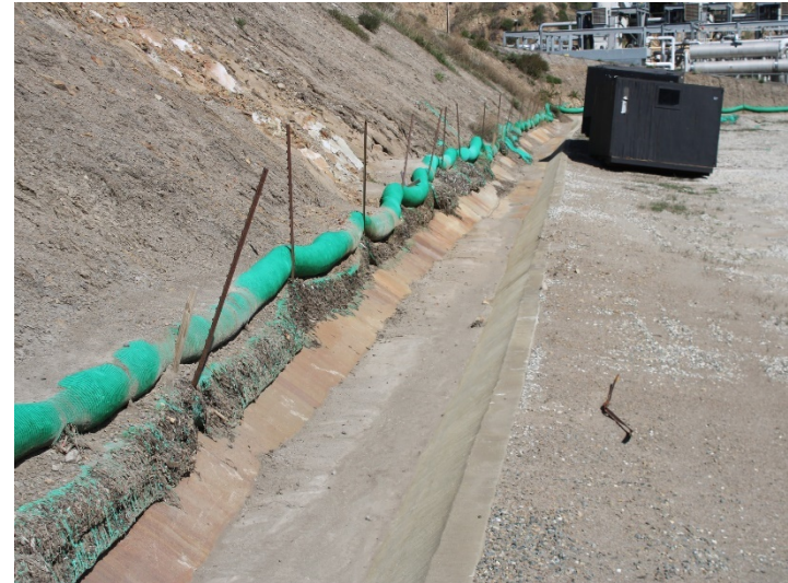
Photo 142: Flares 9, 10, 11 and Gas-to-Energy Facility: February 15, 2024
