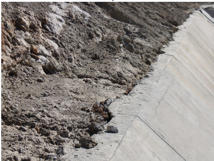
Photo 107: County Sage Mitigation Area and Westside Drainage Channels: January 8, 2024
