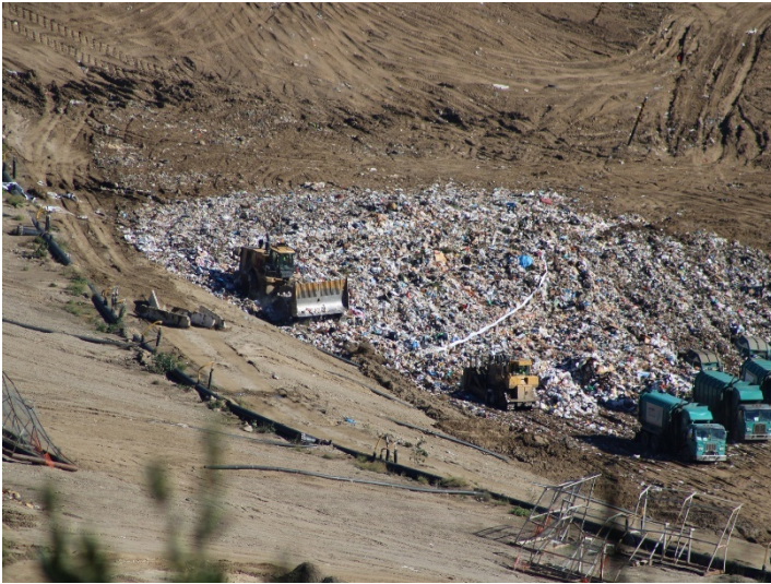
Photo 25: Working Area, CC4 Part 1/2: January 8, 2024
