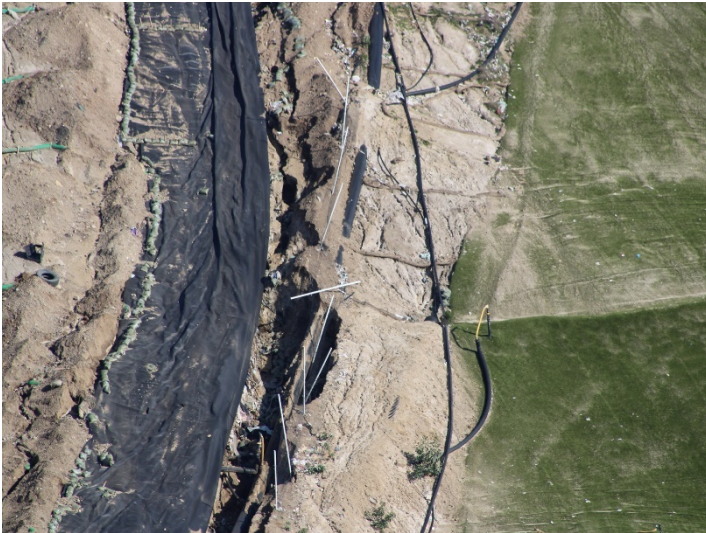
Photo 413: General Site: February 15, 2024
