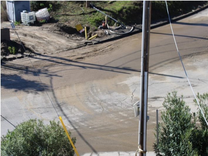
Photo 441: General Site: March 7, 2024
