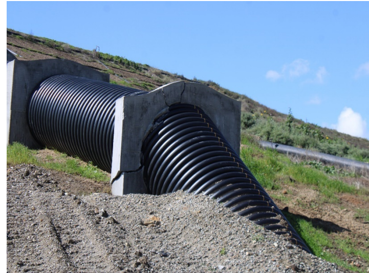
Photo 482: General Site: March 7, 2024
