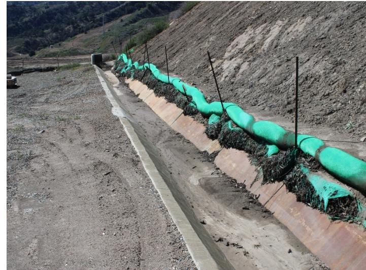
Photo 158: Flares 9, 10, 11 and Gas-to-Energy Facility: March 7, 2024
