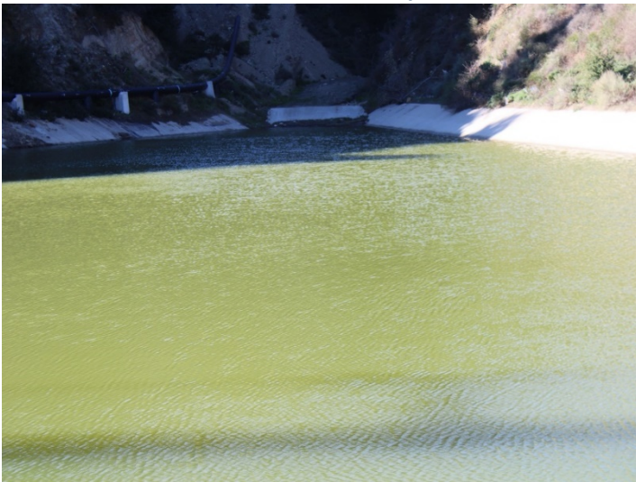
Photo 7: Basin A: January 8, 2024
