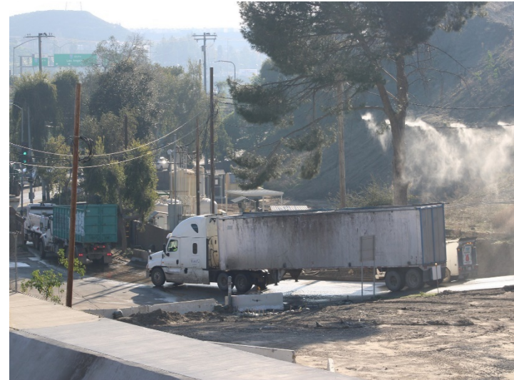
Photo 394: General Site: February 15, 2024
