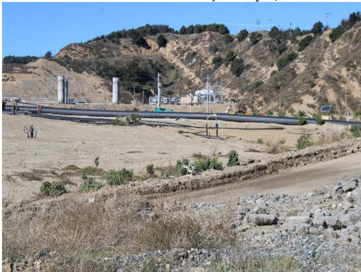
Photo 383: General Site: January 8, 2024
