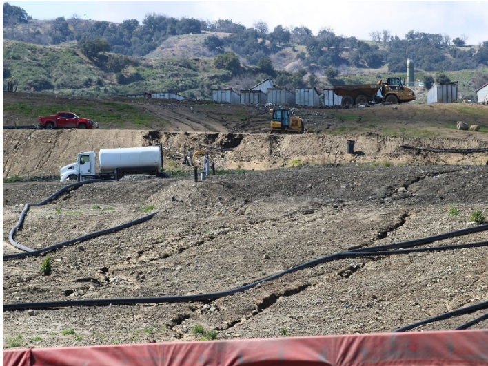
Photo 485: General Site: March 7, 2024
