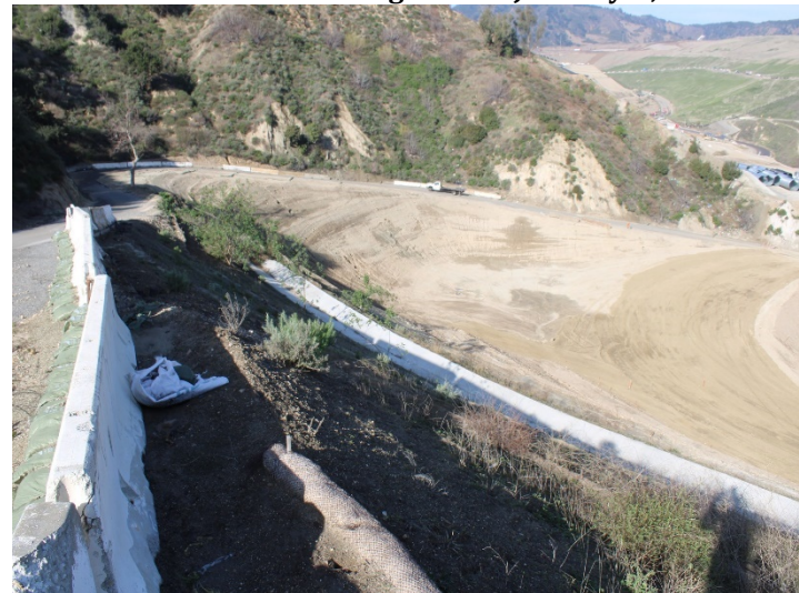
Photo 532: Road Realignment: February 15, 2024
