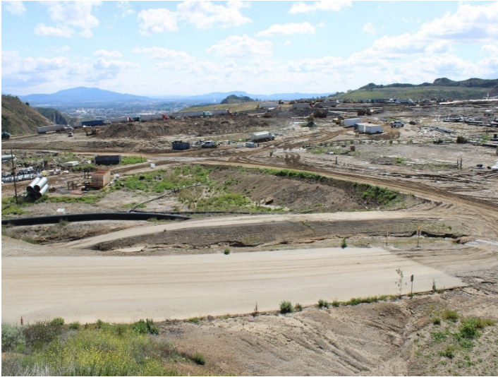
Photo 489: General Site: March 7, 2024
