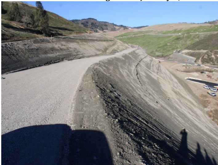
Photo 511: Road Realignment: January 8, 2024
