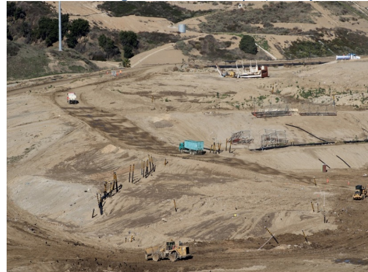
Photo 68: Working Area, CC-4 Part 4/5: January 8, 2024
