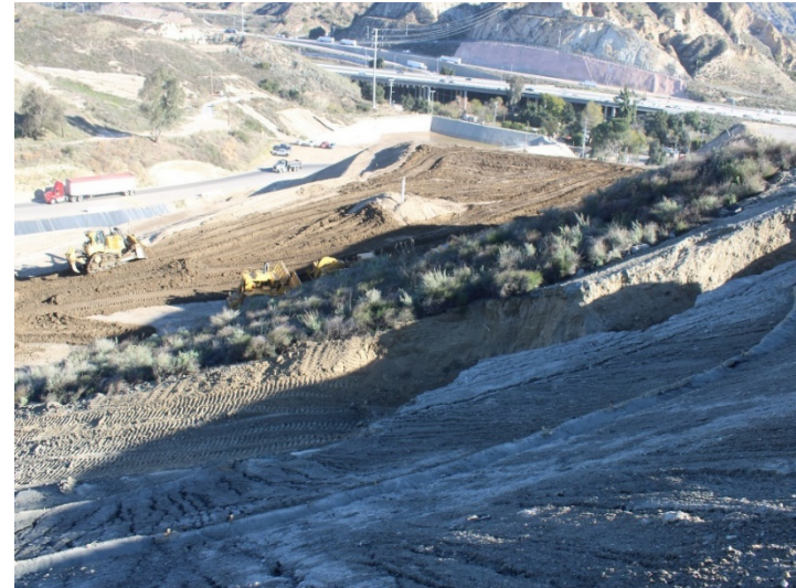
Photo 514: Road Realignment: January 8, 2024
