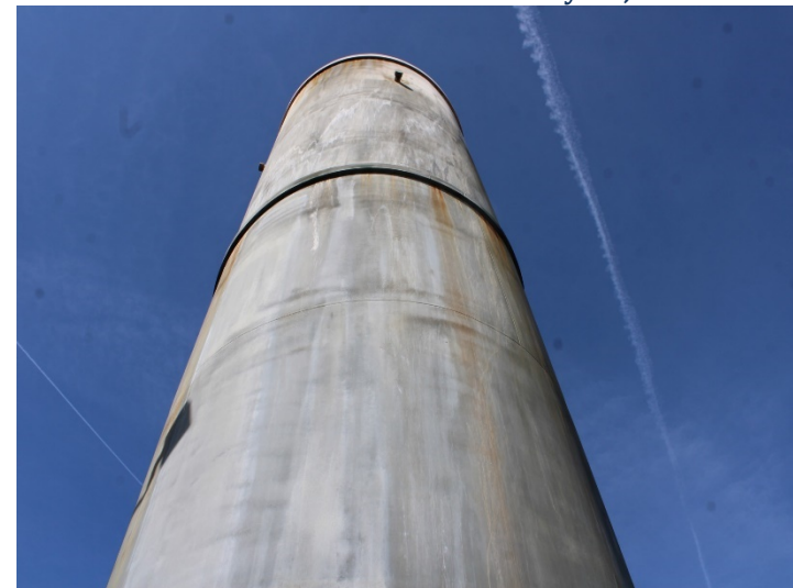
Photo 432: General Site: February 15, 2024
