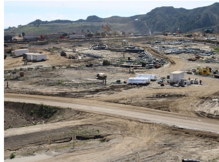
Photo 438: General Site: February 15, 2024
