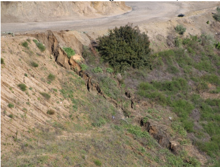
Photo 567: Road Realignment: March 7, 2024
