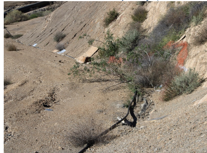
Photo 368: General Site: January 8, 2024
