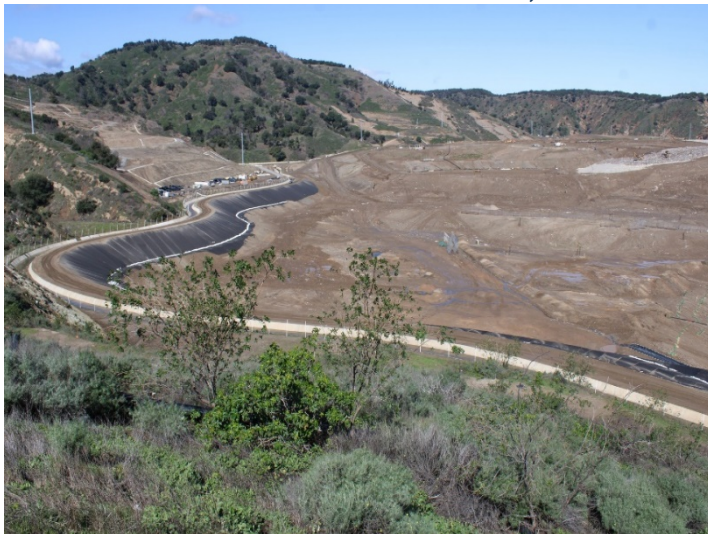
Photo 455: General Site: March 7, 2024
