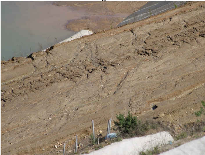
Photo 571: Road Realignment: March 7, 2024
