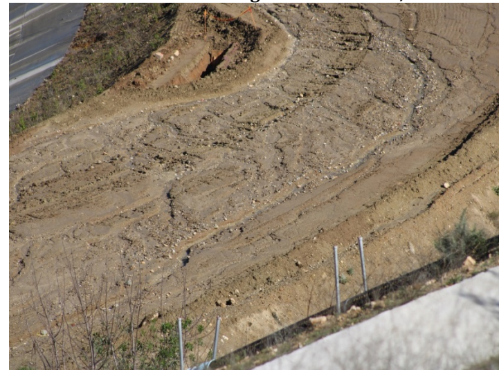
Photo 572: Road Realignment: March 7, 2024
