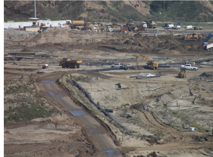
Photo 32: Working Area, CC4 Part 1/2: February 15, 2024
