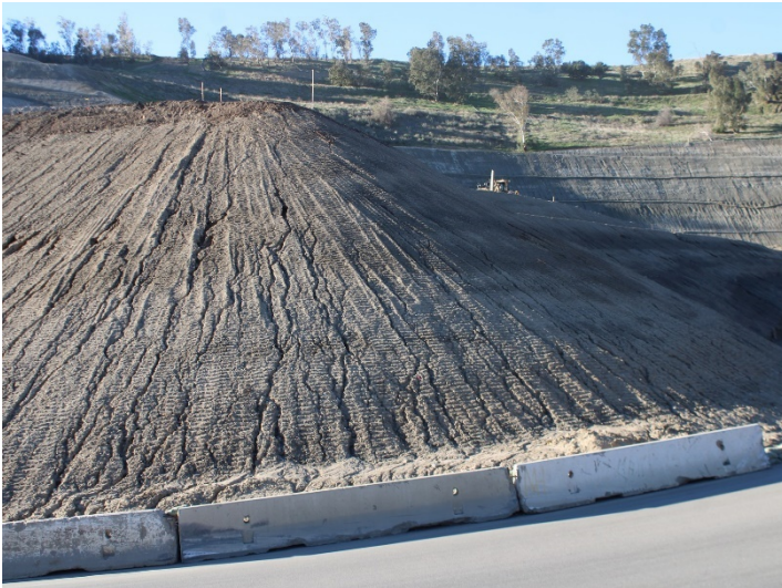
Photo 337: General Site: January 8, 2024
