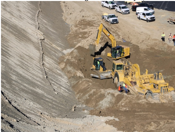
Photo 523: Road Realignment: January 8, 2024
