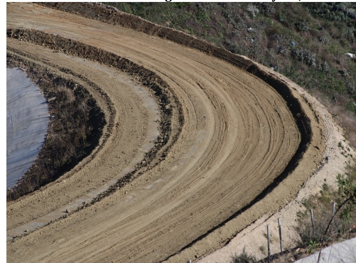
Photo 552: Road Realignment: February 15, 2024
