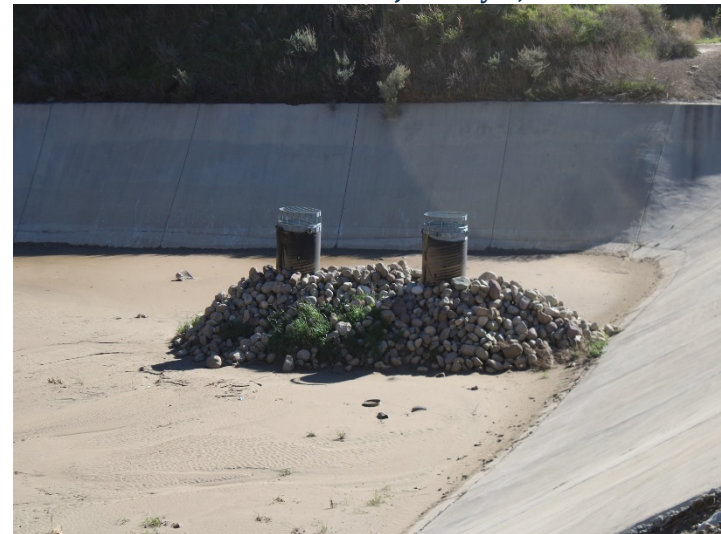
Photo 184: Basin B: January 8, 2024
