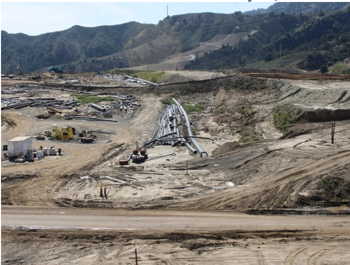
Photo 439: General Site: February 15, 2024
