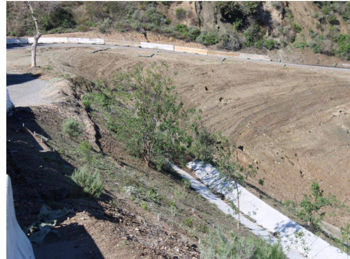
Photo 558: Road Realignment: March 7, 2024
