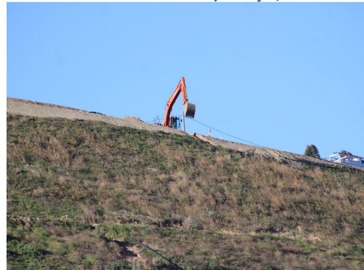
Photo 344: General Site: January 8, 2024
