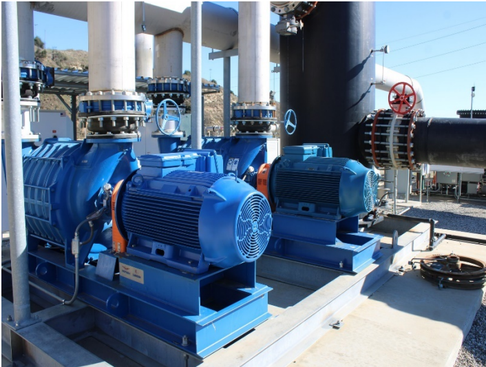
Photo 121: Flares 9, 10, 11 and Gas-to-Energy Facility: January 8, 2024
