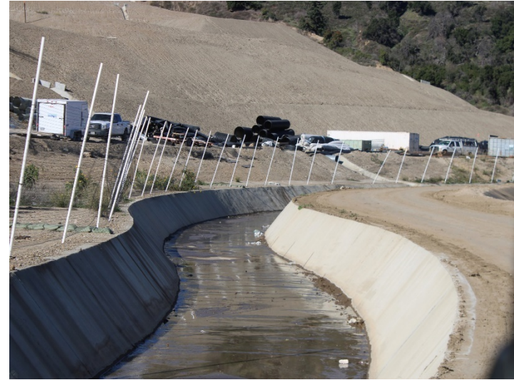
Photo 210: Eastside Drainage Channel: January 8, 2024
