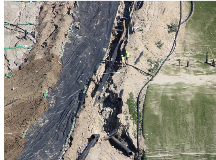
Photo 414: General Site: February 15, 2024
