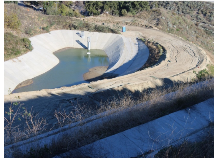
Photo 498: Road Realignment: January 8, 2024
