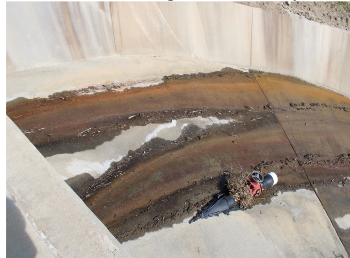
Photo 216: Eastside Drainage Channel: February 15, 2024
