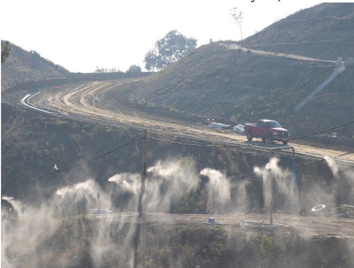
Photo 395: General Site: February 15, 2024
