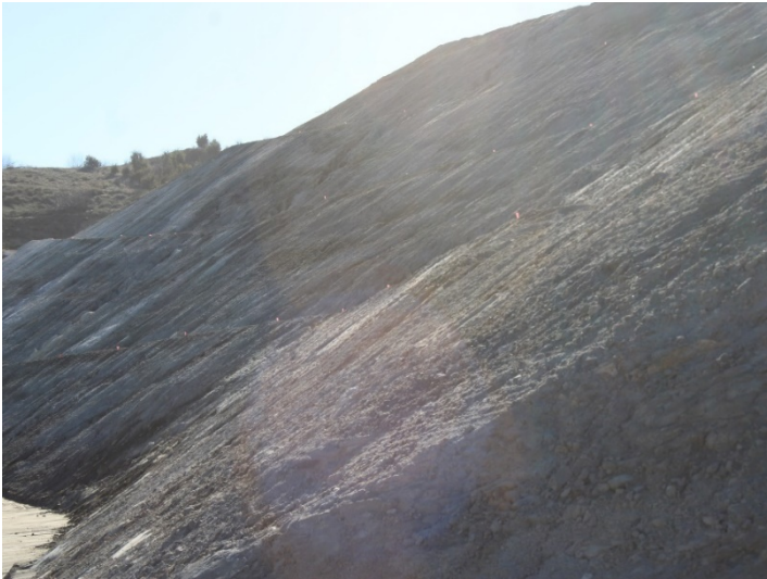
Photo 529: Road Realignment: January 8, 2024
