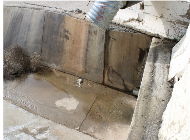
Photo 214: Eastside Drainage Channel: February 15, 2024
