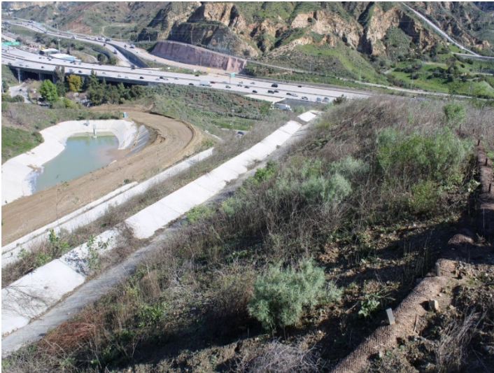
Photo 557: Road Realignment: March 7, 2024
