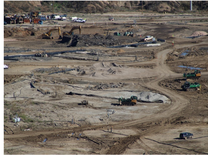
Photo 22: Working Area, CC4 Part 1/2: January 8, 2024
