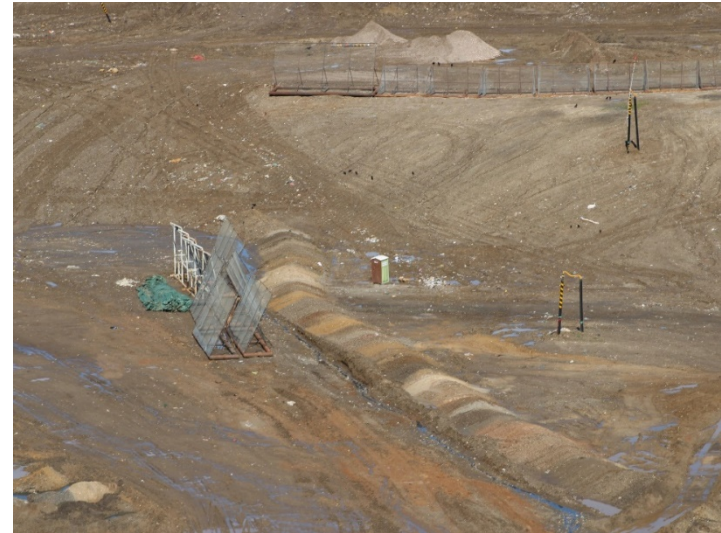
Photo 466: General Site: March 7, 2024
