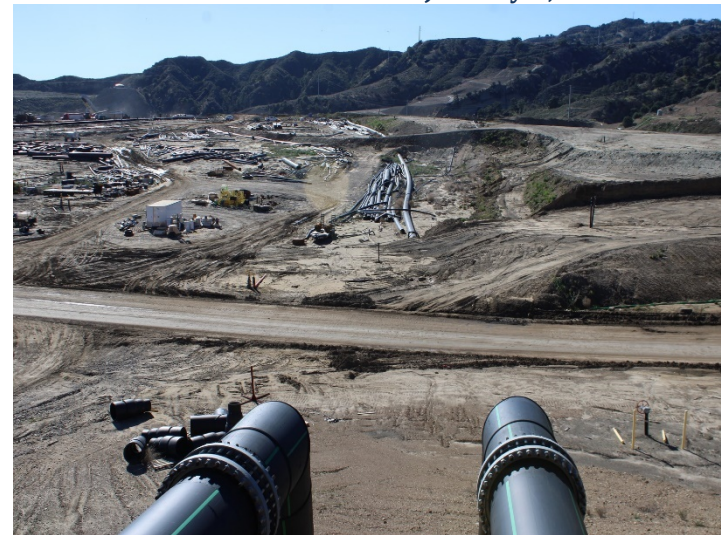
Photo 372: General Site: January 8, 2024
