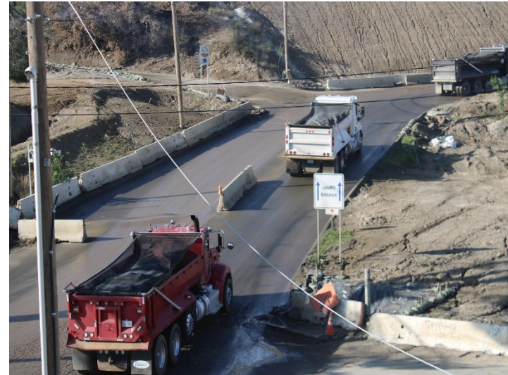
Photo 398: General Site: February 15, 2024
