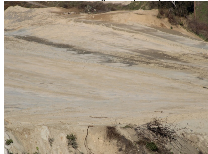
Photo 508: Road Realignment: January 8, 2024
