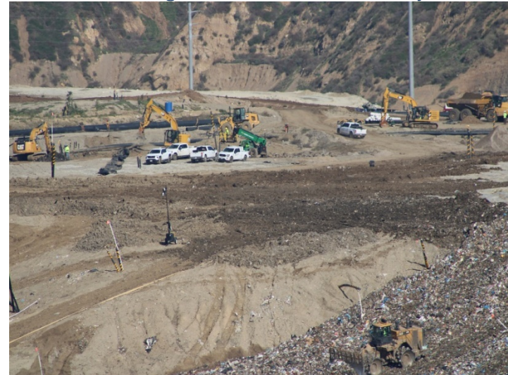
Photo 56: Working Area, CC-4 Part 3: February 15, 2024
