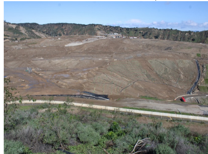
Photo 456: General Site: March 7, 2024
