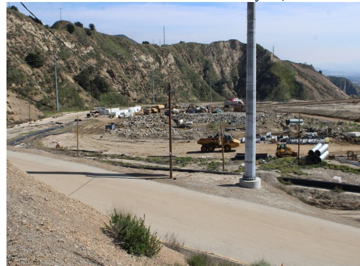
Photo 436: General Site: February 15, 2024
