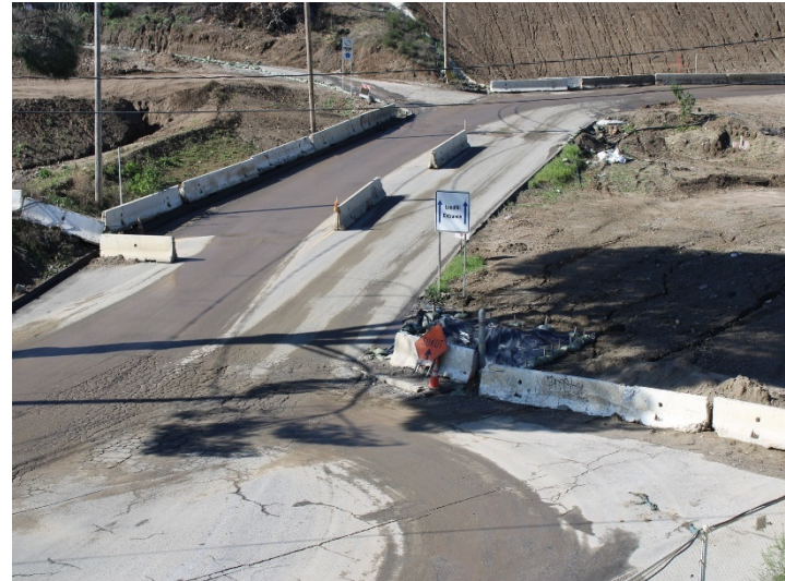
Photo 442: General Site: March 7, 2024
