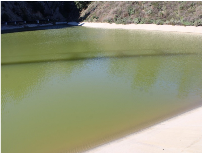
Photo 3: Basin A: January 8, 2024
