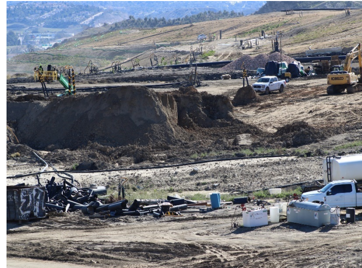
Photo 374: General Site: January 8, 2024
