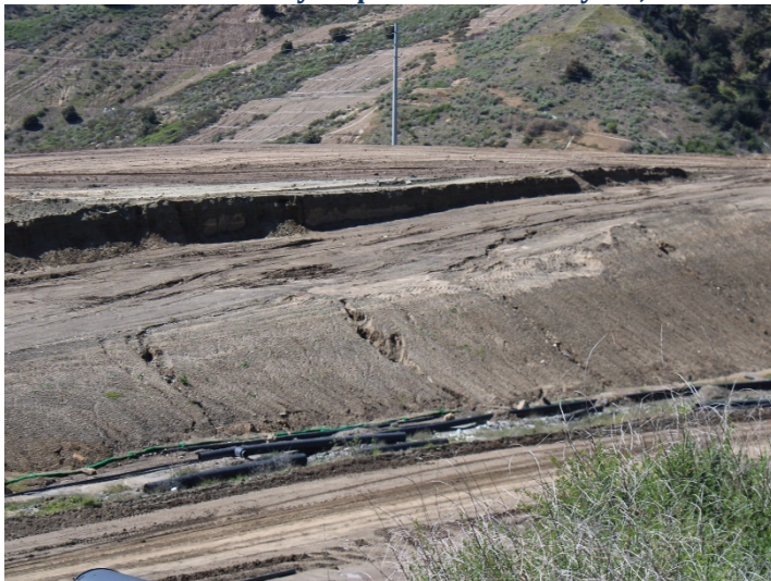
Photo 175: County Top Deck: March 7, 2024
