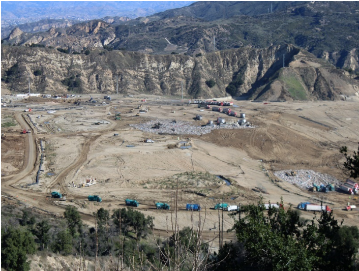
Photo 365: General Site: January 8, 2024
