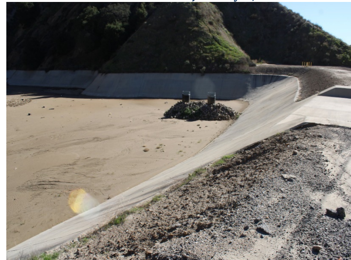
Photo 180: Basin B: January 8, 2024
