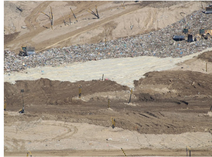
Photo 50: Working Area, CC-4 Part 3: February 15, 2024
