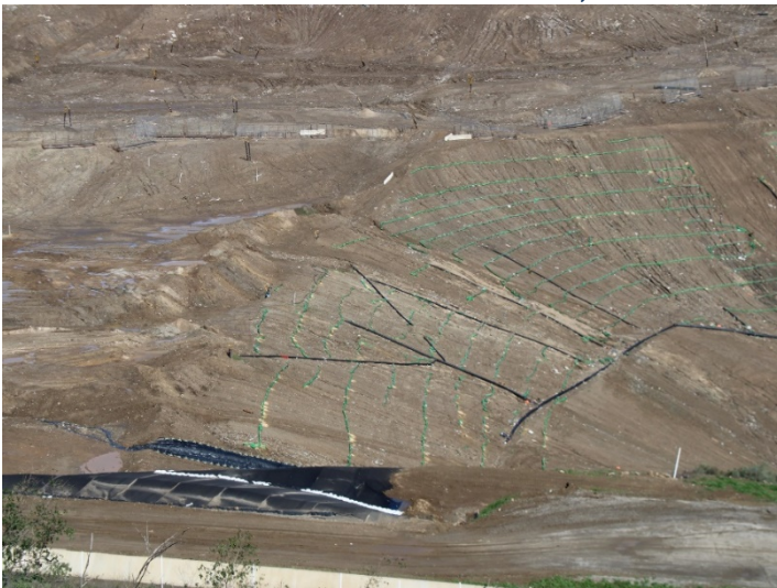
Photo 459: General Site: March 7, 2024
