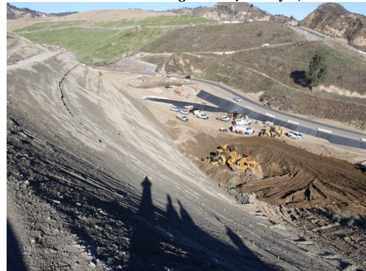
Photo 512: Road Realignment: January 8, 2024
