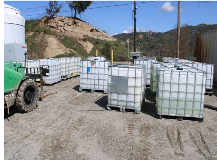
Photo 98: Alder Tank Liquids Treatment System: March 7, 2024
