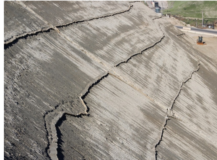
Photo 522: Road Realignment: January 8, 2024
