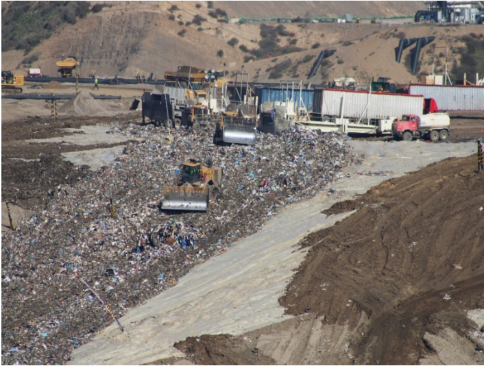
Photo 57: Working Area, CC-4 Part 3: February 15, 2024
