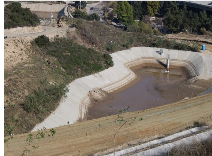
Photo 538: Road Realignment: February 15, 2024
