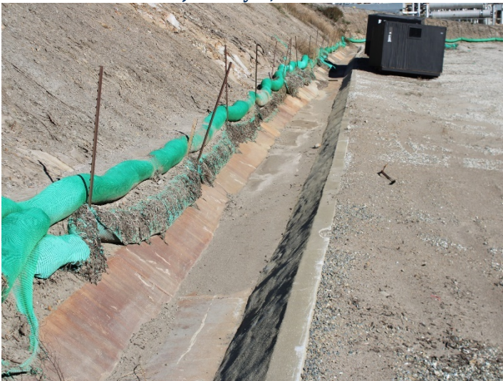
Photo 123: Flares 9, 10, 11 and Gas-to-Energy Facility: January 8, 2024
