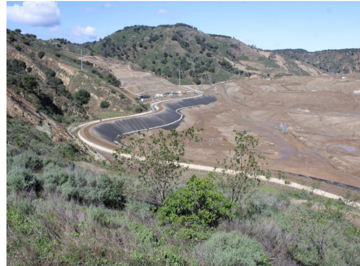
Photo 454: General Site: March 7, 2024
