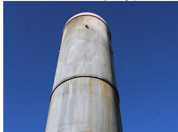
Photo 352: General Site: January 8, 2024
