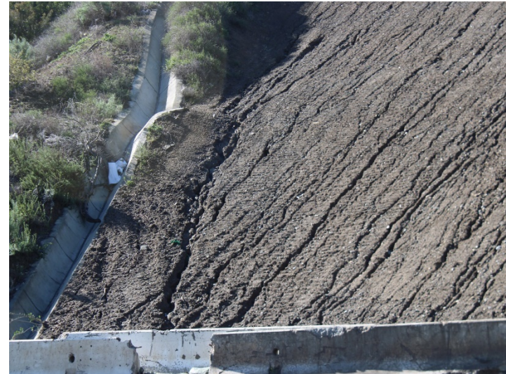
Photo 450: General Site: March 7, 2024
