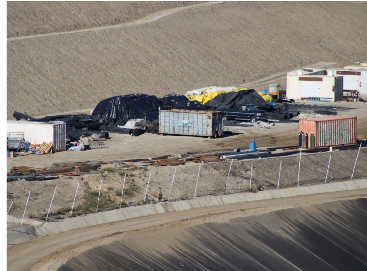
Photo 350: General Site: January 8, 2024
