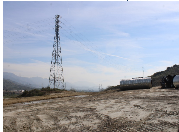
Photo 416: General Site: February 15, 2024
