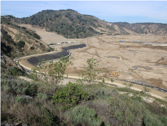
Photo 401: General Site: February 15, 2024
