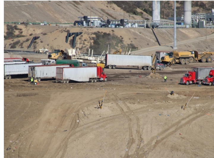
Photo 82: Working Area, CC-4 Part 4/5: January 8, 2024
