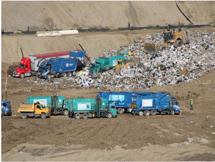
Photo 77: Working Area, CC-4 Part 4/5: January 8, 2024
