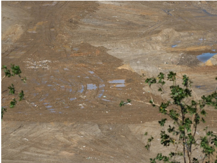
Photo 465: General Site: March 7, 2024
