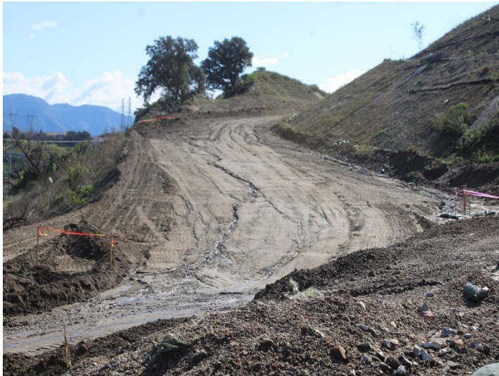
Photo 453: General Site: March 7, 2024
