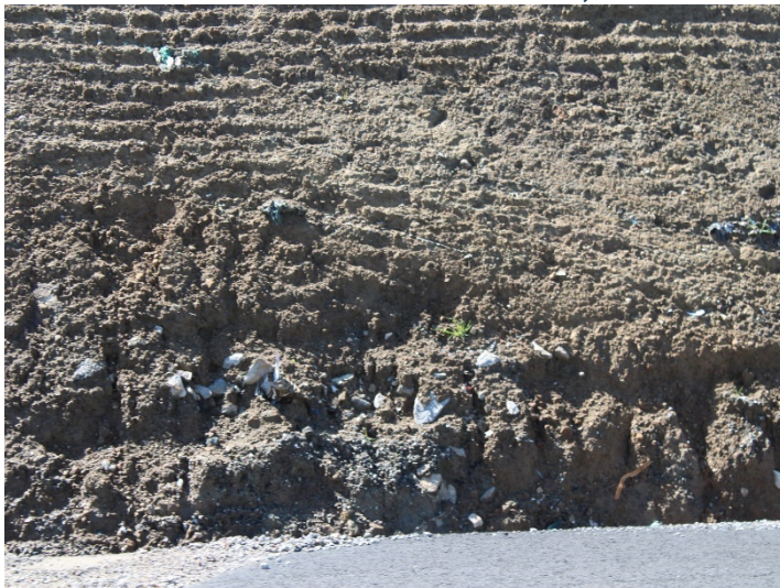
Photo 479: General Site: March 7, 2024
