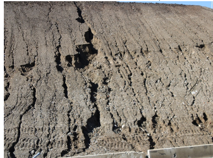
Photo 452: General Site: March 7, 2024
