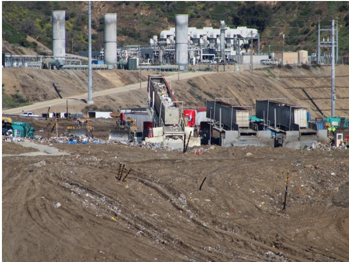
Photo 473: General Site: March 7, 2024
