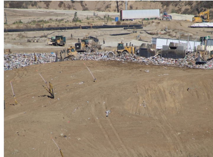
Photo 80: Working Area, CC-4 Part 4/5: January 8, 2024
