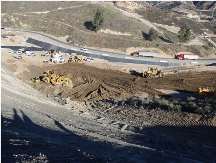
Photo 513: Road Realignment: January 8, 2024
