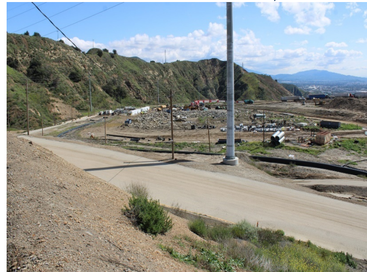
Photo 488: General Site: March 7, 2024
