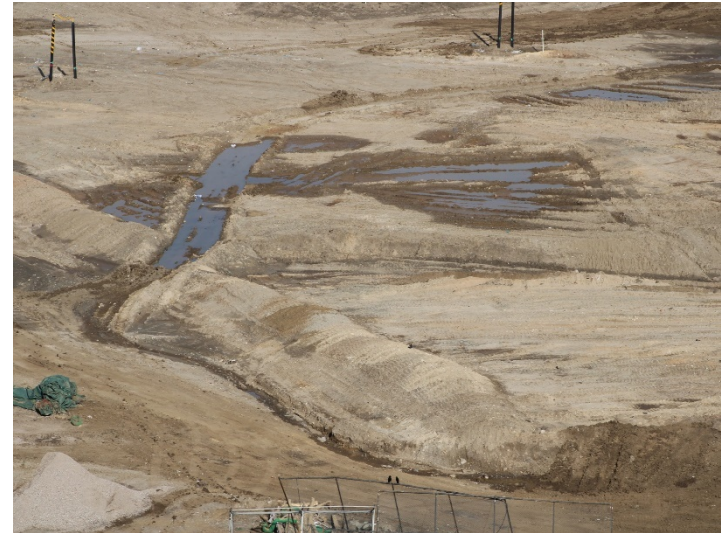
Photo 46: Working Area, CC-4 Part 3: February 15, 2024
