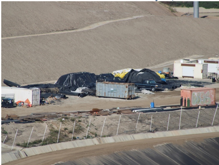
Photo 407: General Site: February 15, 2024
