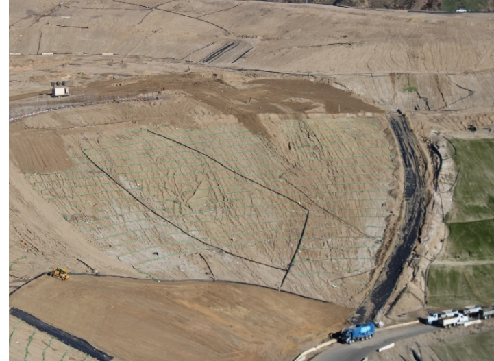
Photo 64: Working Area, CC-4 Part 4/5: January 8, 2024
