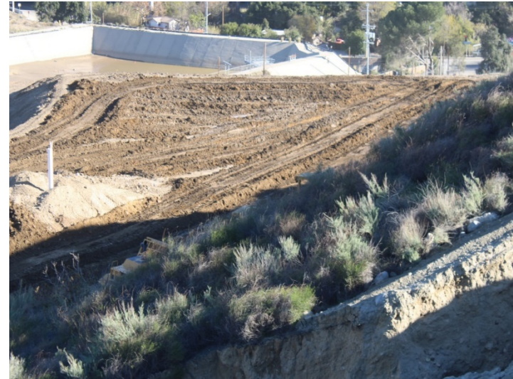
Photo 518: Road Realignment: January 8, 2024
