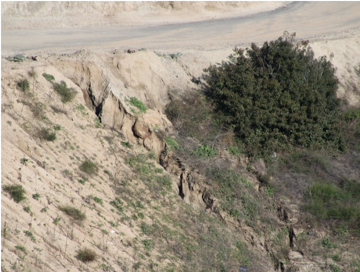
Photo 545: Road Realignment: February 15, 2024
