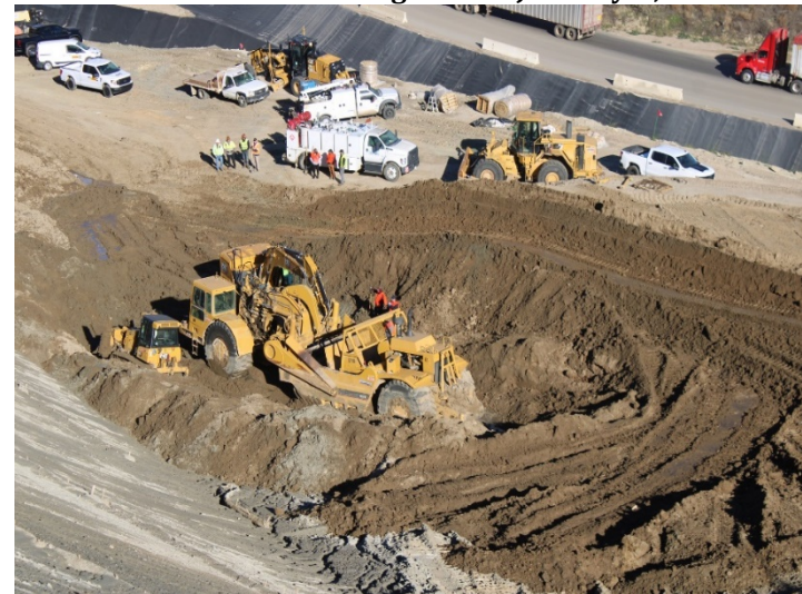
Photo 516: Road Realignment: January 8, 2024
