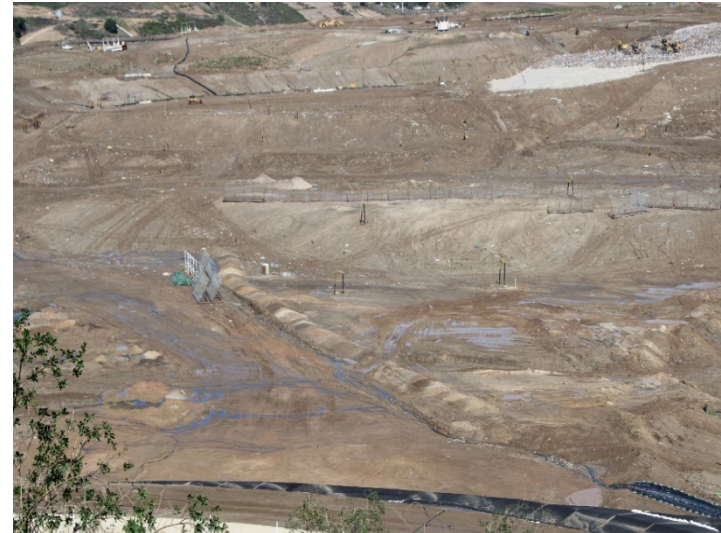
Photo 458: General Site: March 7, 2024
