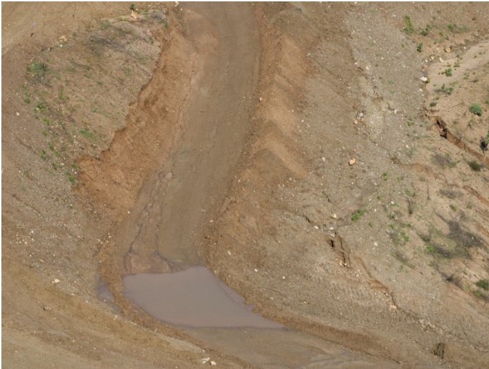
Photo 565: Road Realignment: March 7, 2024
