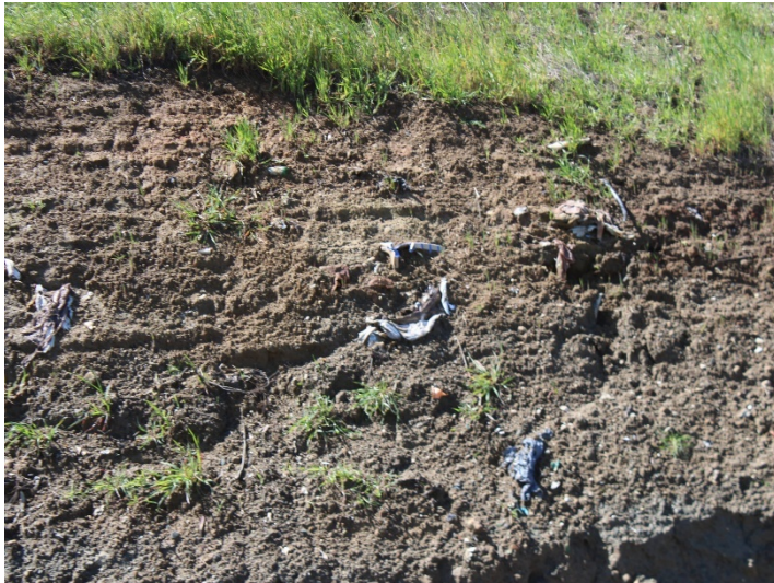
Photo 477: General Site: March 7, 2024
