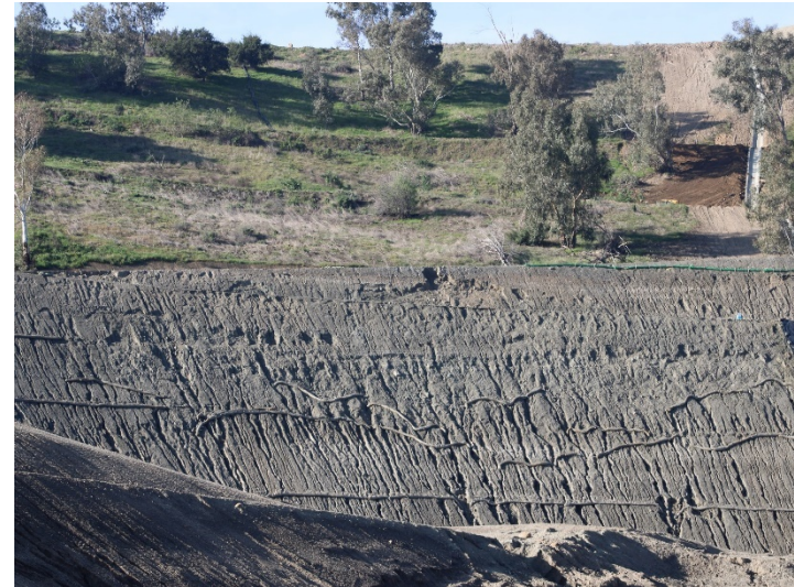
Photo 390: General Site: February 15, 2024
