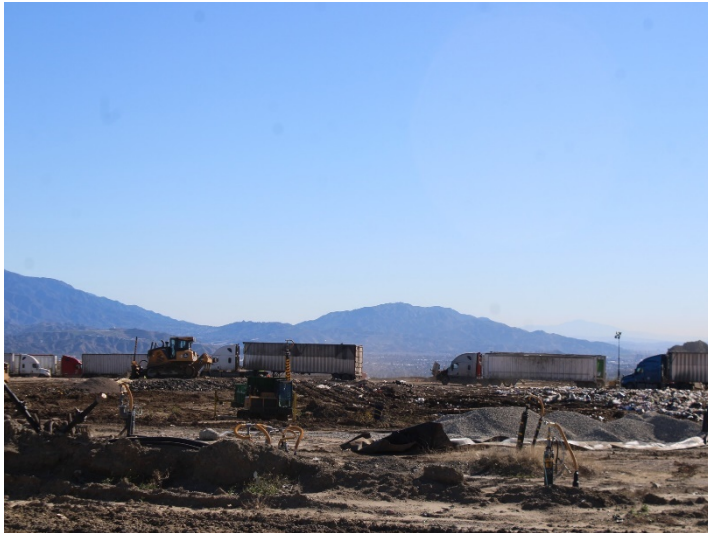
Photo 165: County Top Deck: January 8, 2024
