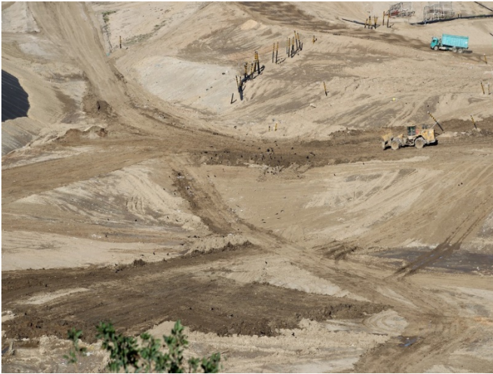
Photo 65: Working Area, CC-4 Part 4/5: January 8, 2024
