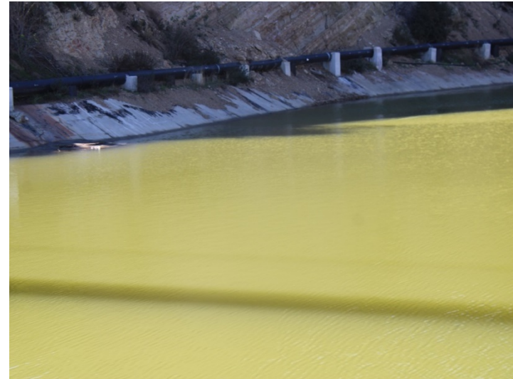
Photo 6: Basin A: January 8, 2024
