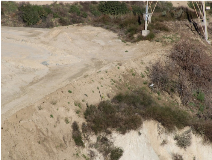
Photo 509: Road Realignment: January 8, 2024
