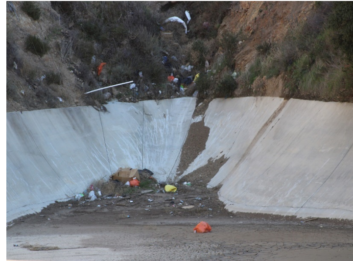
Photo 186: Basin B: January 8, 2024
