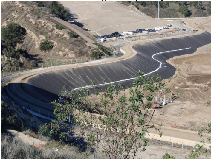
Photo 531: Road Realignment: January 8, 2024
