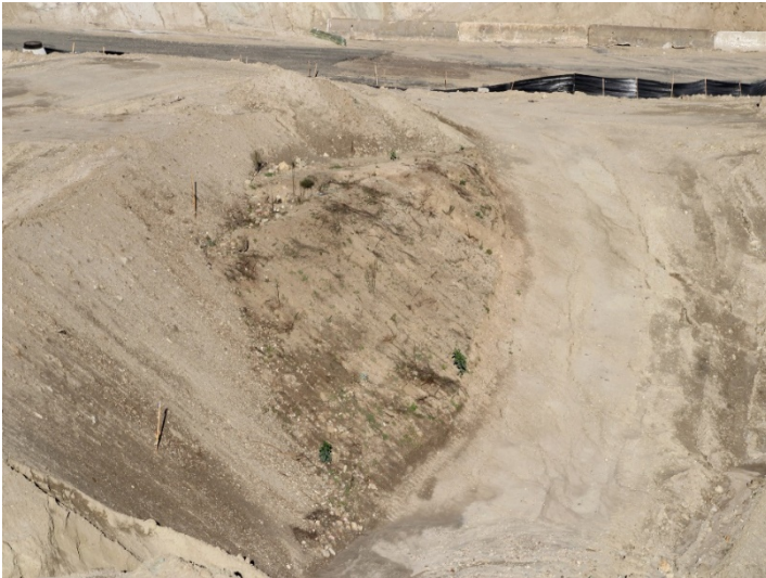
Photo 501: Road Realignment: January 8, 2024
