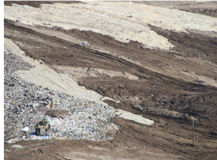
Photo 38: Working Area, CC4 Part 1/2: February 15, 2024
