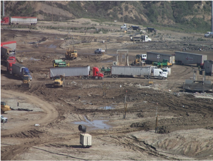
Photo 33: Working Area, CC4 Part 1/2: February 15, 2024
