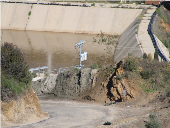
Photo 575: Road Realignment: March 7, 2024
