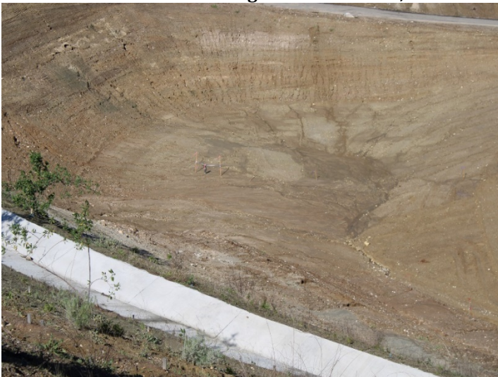
Photo 559: Road Realignment: March 7, 2024
