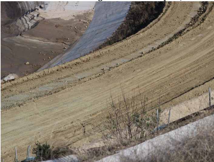
Photo 551: Road Realignment: February 15, 2024
