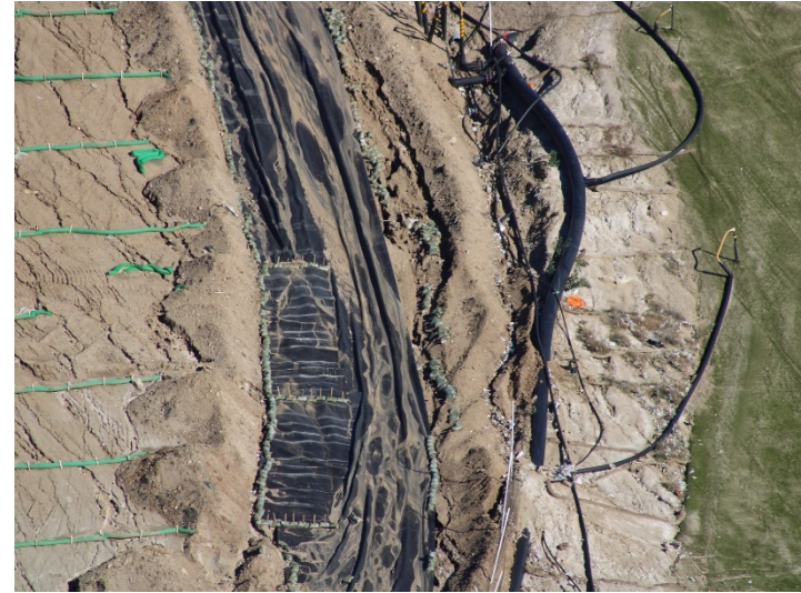
Photo 346: General Site: January 8, 2024
