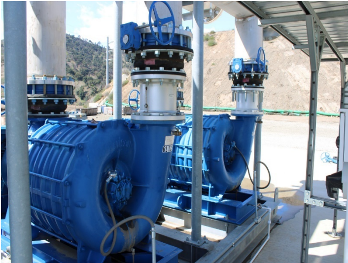
Photo 157: Flares 9, 10, 11 and Gas-to-Energy Facility: March 7, 2024
