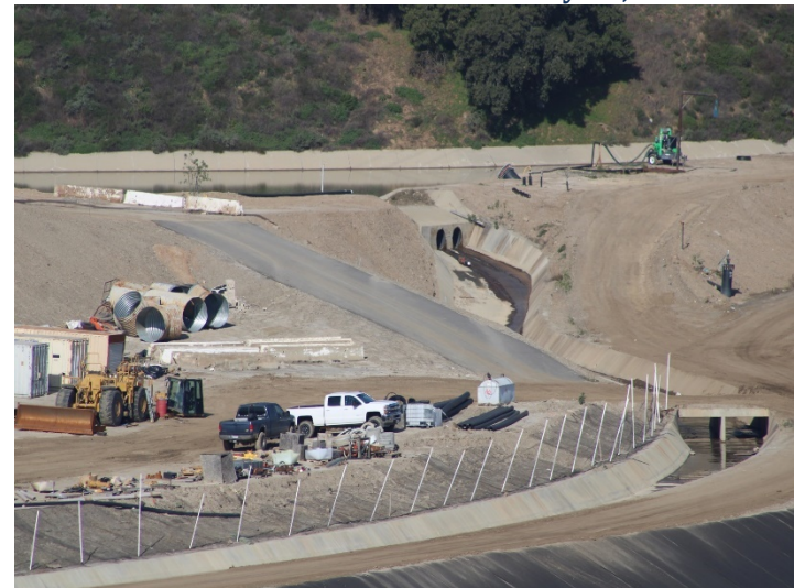
Photo 408: General Site: February 15, 2024
