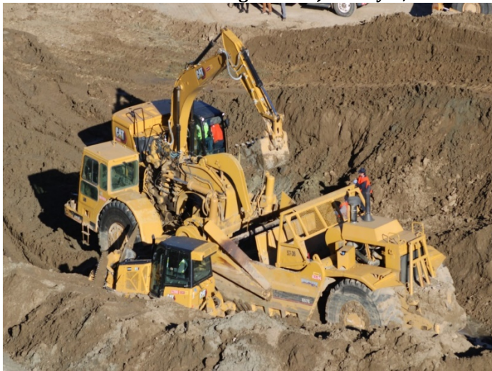
Photo 519: Road Realignment: January 8, 2024
