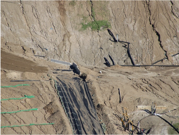
Photo 345: General Site: January 8, 2024
