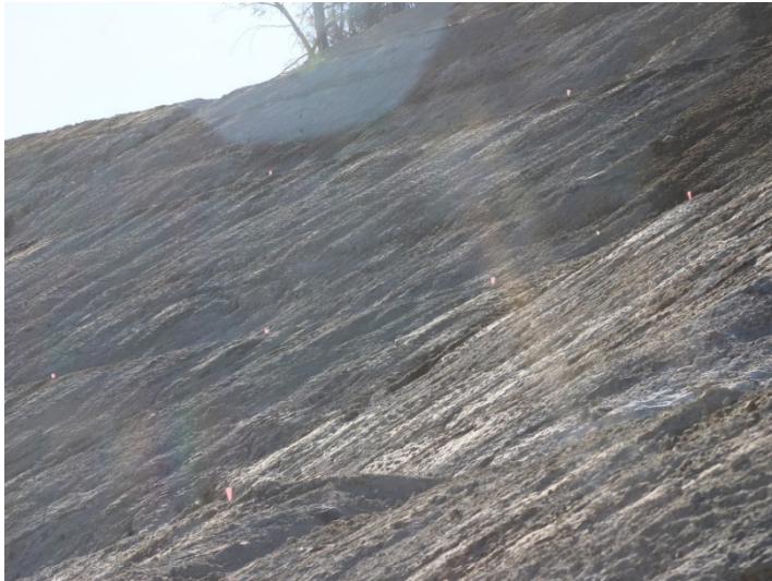
Photo 525: Road Realignment: January 8, 2024
