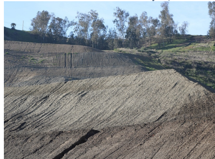
Photo 388: General Site: February 15, 2024
