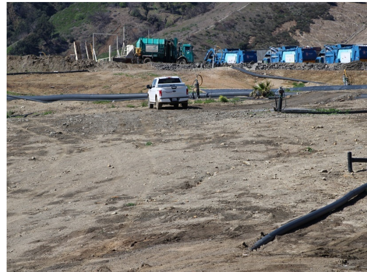
Photo 486: General Site: March 7, 2024
