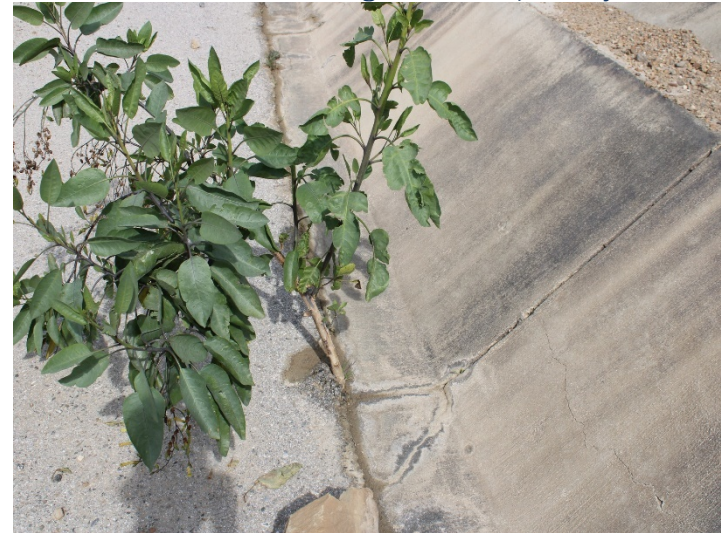
Photo 212: Eastside Drainage Channel: February 15, 2024
