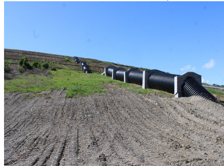
Photo 480: General Site: March 7, 2024
