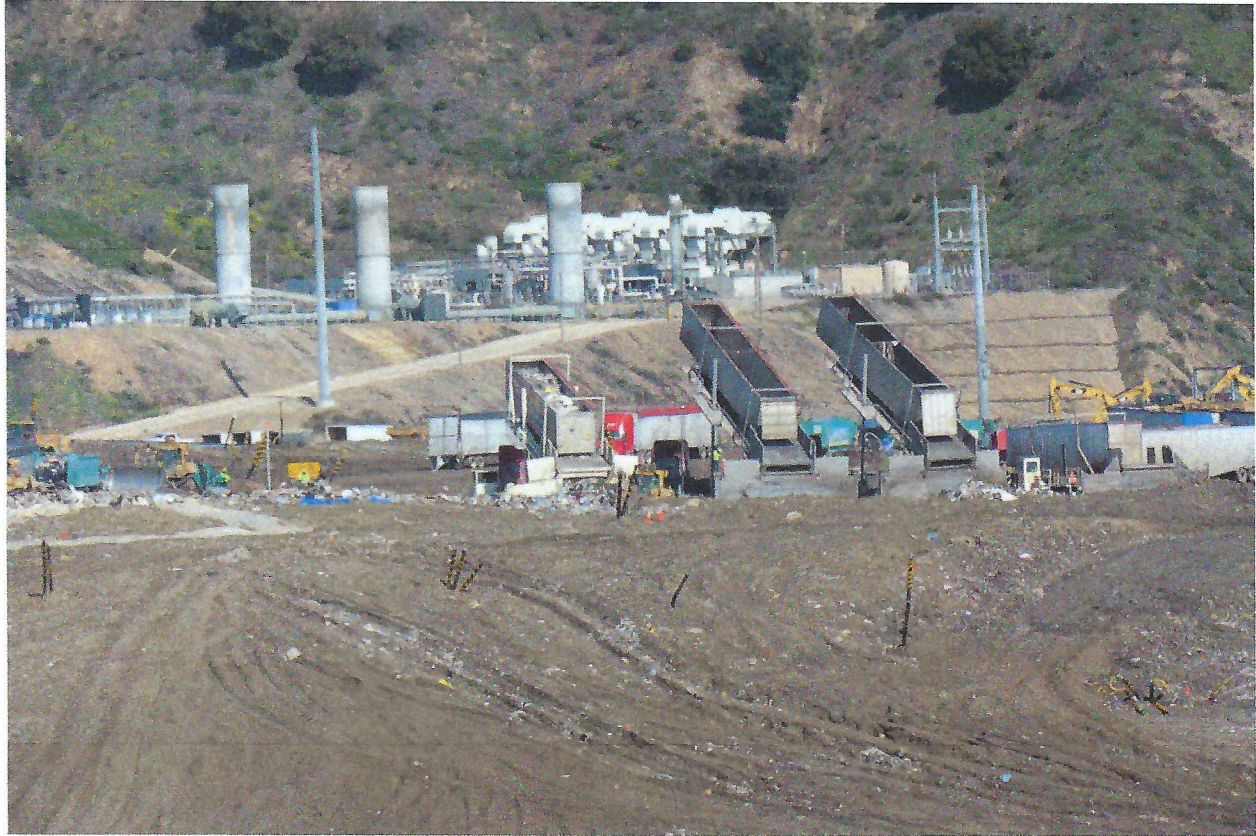
Figure 2: Filters at the waste face
