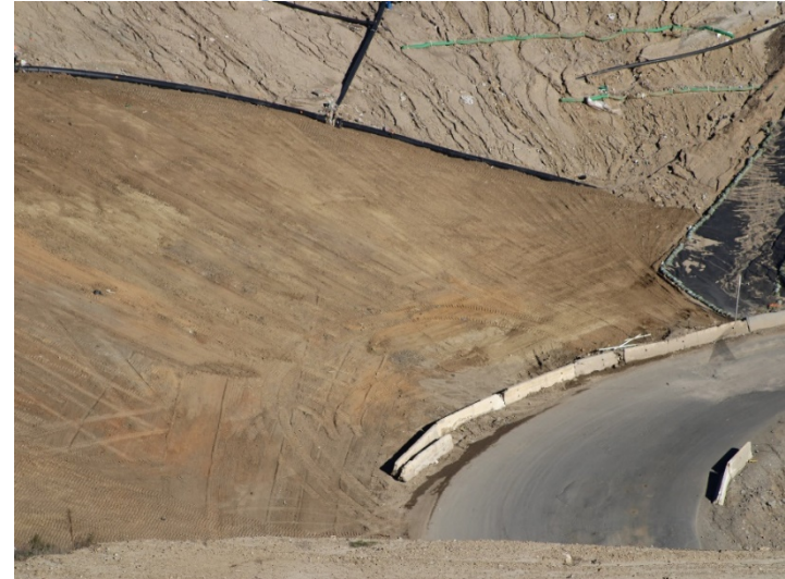
Photo 76: Working Area, CC-4 Part 4/5: January 8, 2024
