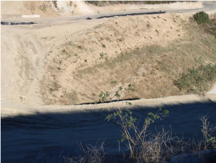
Photo 497: Road Realignment: January 8, 2024
