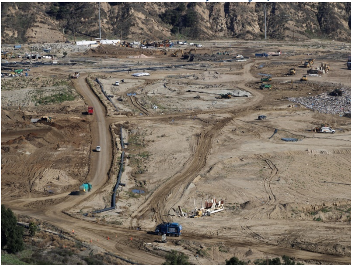
Photo 367: General Site: January 8, 2024
