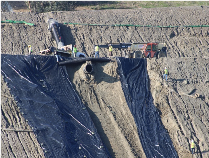
Photo 393: General Site: February 15, 2024
