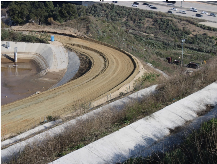
Photo 539: Road Realignment: February 15, 2024
