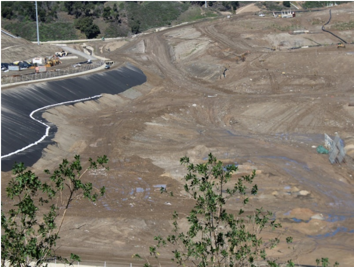
Photo 457: General Site: March 7, 2024
