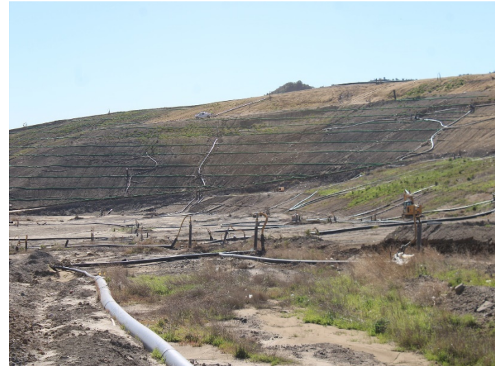
Photo 378: General Site: January 8, 2024
