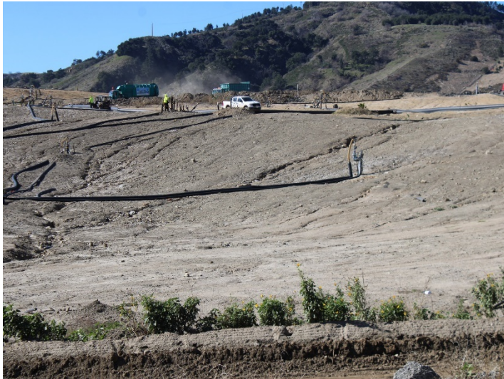
Photo 381: General Site: January 8, 2024
