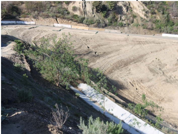
Photo 535: Road Realignment: February 15, 2024
