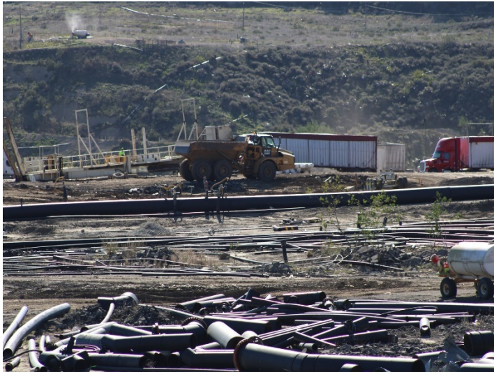
Photo 377: General Site: January 8, 2024
