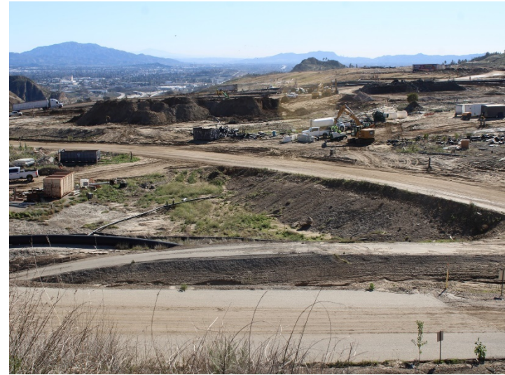
Photo 370: General Site: January 8, 2024
