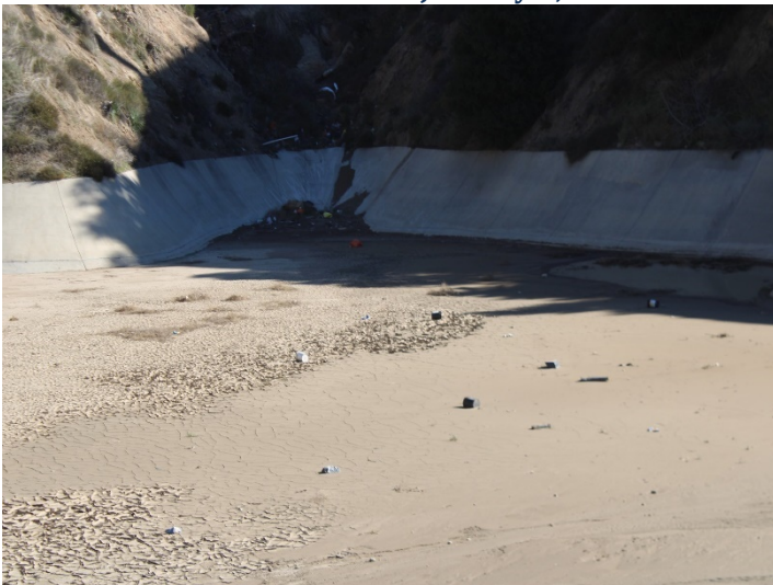
Photo 183: Basin B: January 8, 2024
