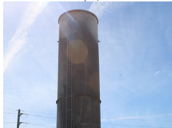
Photo 132: Flares 9, 10, 11 and Gas-to-Energy Facility: February 15, 2024
