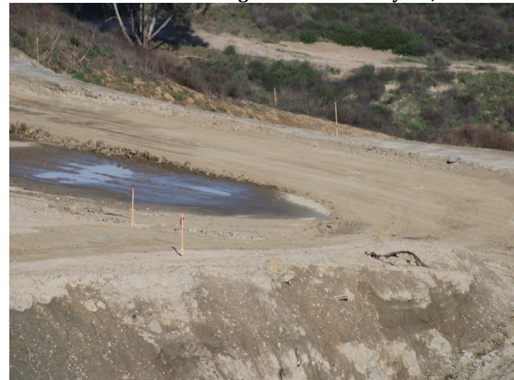
Photo 544: Road Realignment: February 15, 2024
