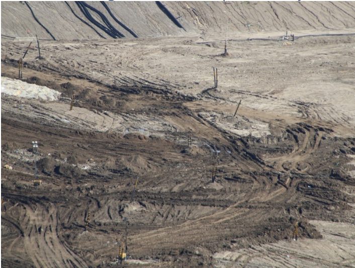
Photo 39: Working Area, CC4 Part 1/2: February 15, 2024
