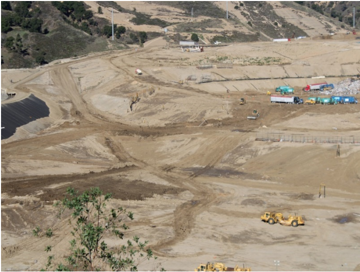
Photo 61: Working Area, CC-4 Part 4/5: January 8, 2024
