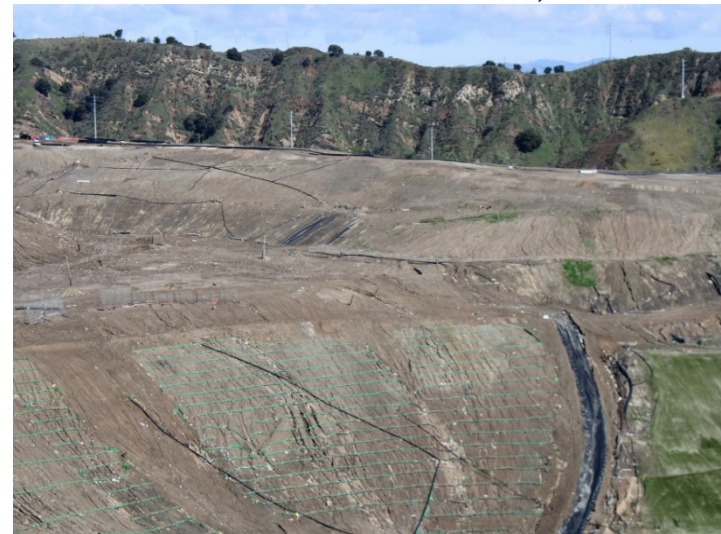
Photo 464: General Site: March 7, 2024
