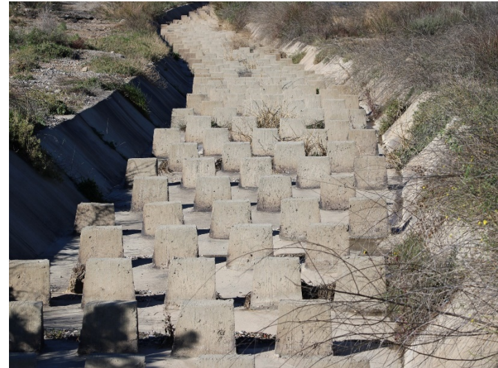
Photo 358: General Site: January 8, 2024
