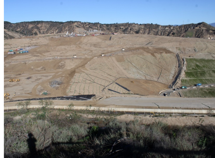
Photo 60: Working Area, CC-4 Part 4/5: January 8, 2024
