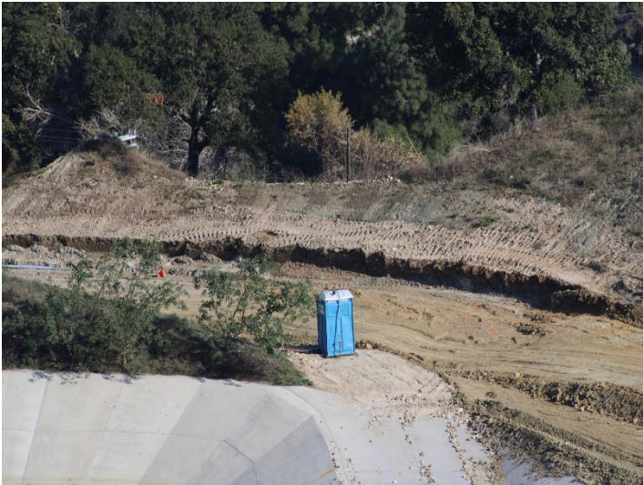
Photo 553: Road Realignment: February 15, 2024
