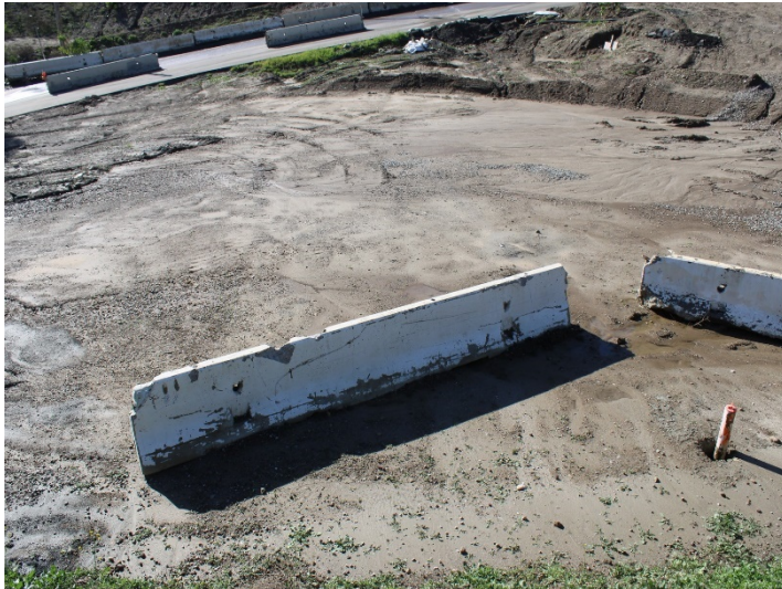
Photo 445: General Site: March 7, 2024
