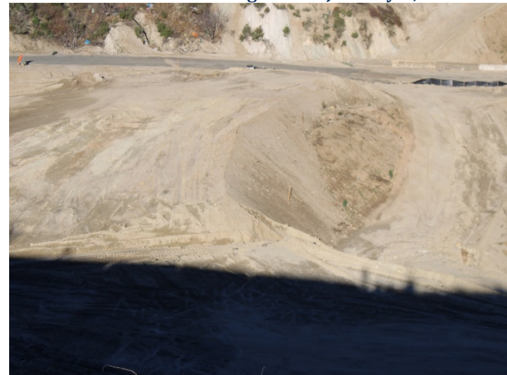
Photo 496: Road Realignment: January 8, 2024
