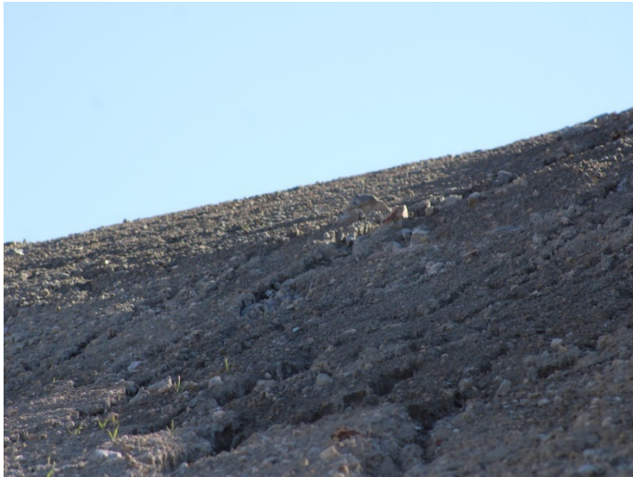
Photo 521: Road Realignment: January 8, 2024
