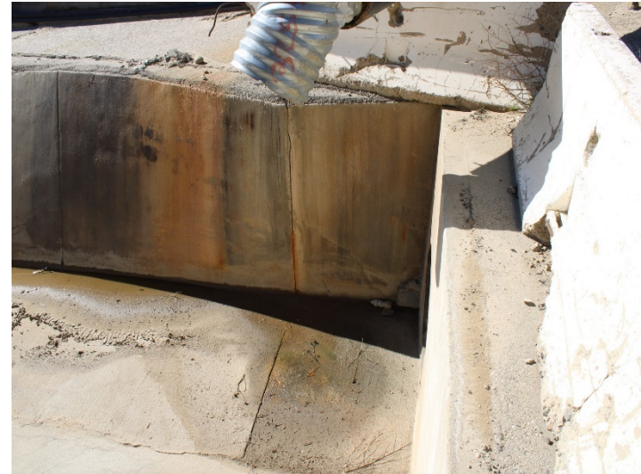
Photo 106: County Sage Mitigation Area and Westside Drainage Channels: January 8, 2024
