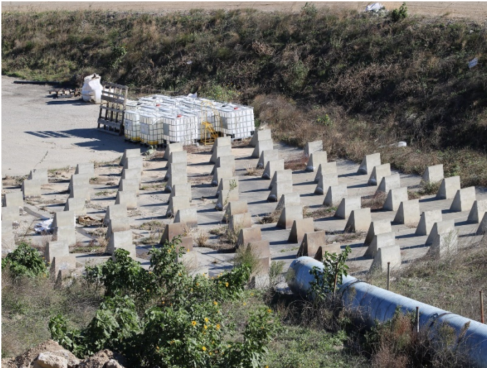
Photo 357: General Site: January 8, 2024
