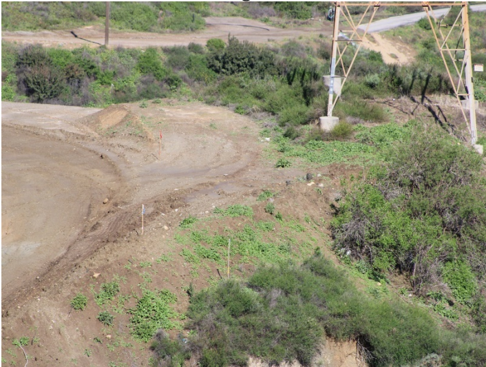
Photo 579: Road Realignment: March 7, 2024
