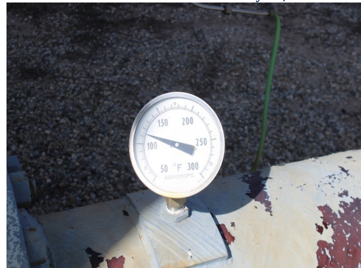
Photo 428: General Site: February 15, 2024
