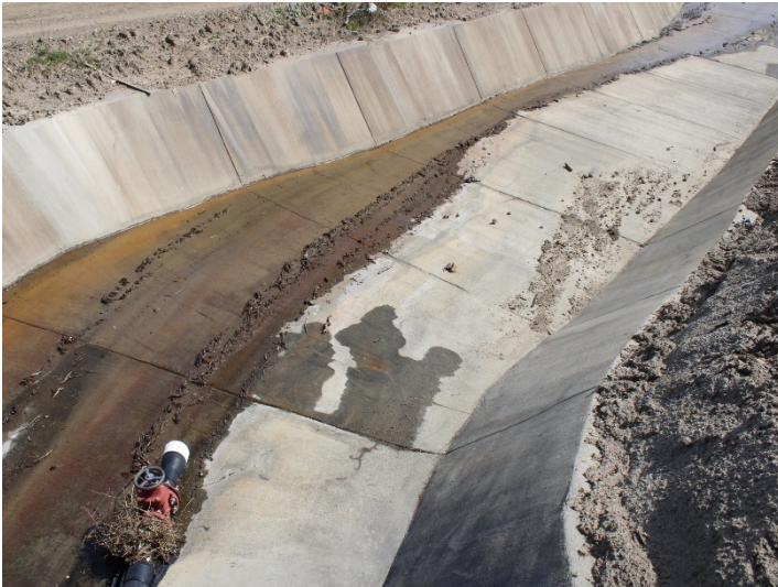
Photo 217: Eastside Drainage Channel: February 15, 2024
