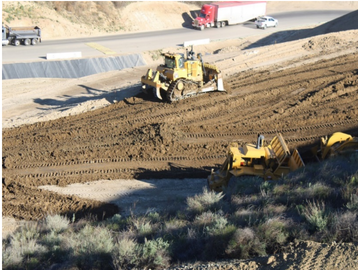
Photo 517: Road Realignment: January 8, 2024
