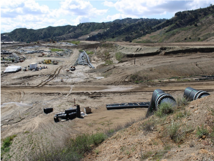
Photo 491: General Site: March 7, 2024
