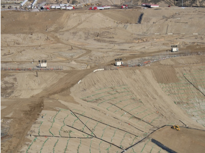
Photo 63: Working Area, CC-4 Part 4/5: January 8, 2024
