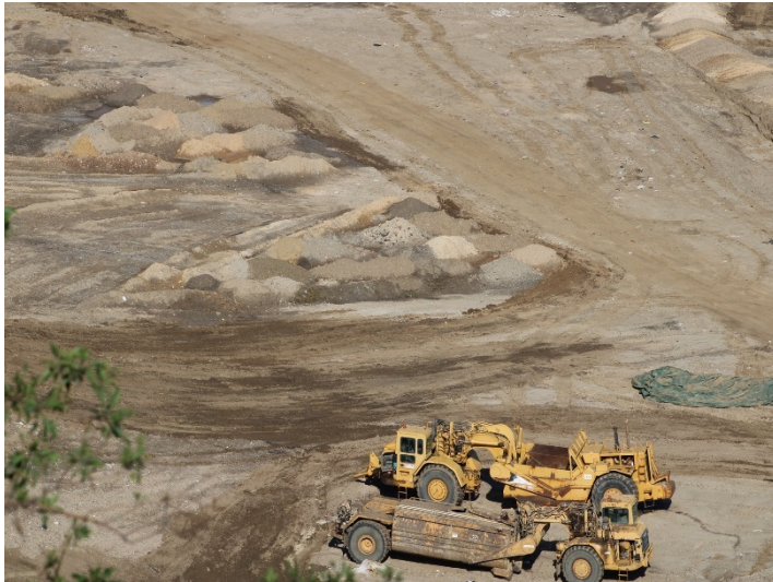
Photo 45: Working Area, CC-4 Part 3: February 15, 2024
