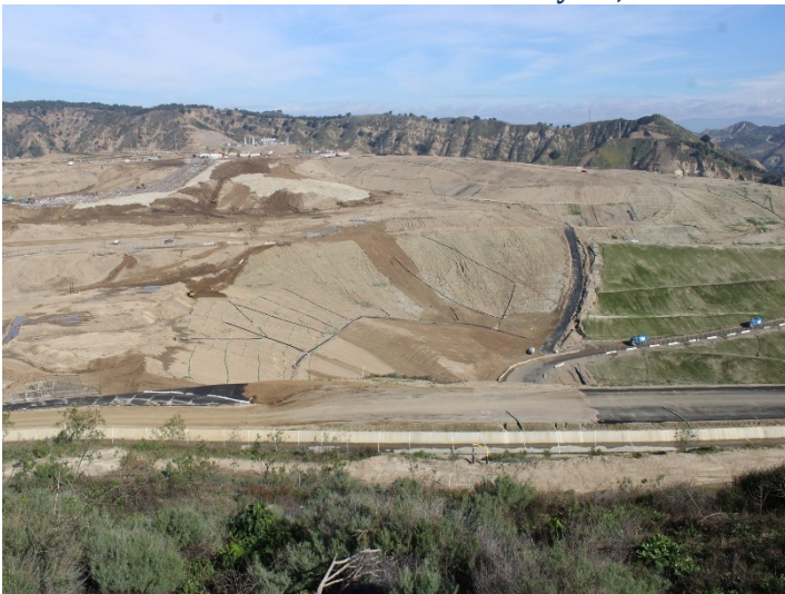
Photo 403: General Site: February 15, 2024
