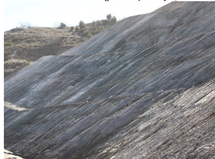
Photo 524: Road Realignment: January 8, 2024
