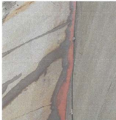
Photo 6: Reddish deposit from water seeping through weep holes at the bottom of the wall
