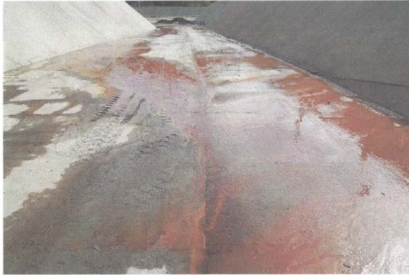
Photo 5: Water flowing out between floor slab joints at Terminal basin
