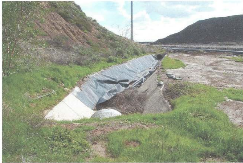
Photo 11: Damage to membrane on first segment of channel west of the access road to Flares 9-11
