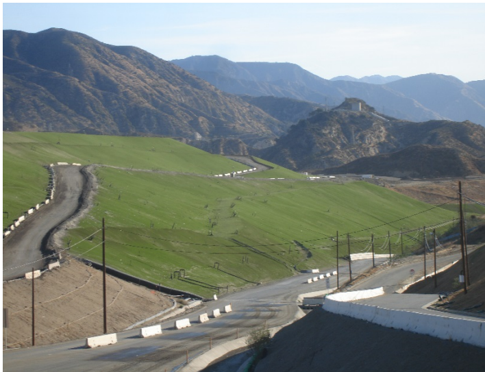
Photo 171: Posi-Shell and Closure Turf: January 22, 2019
