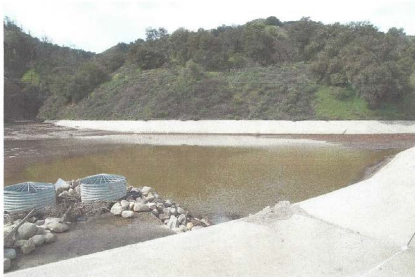
Photo 13: Low water volume and limited sediment accumulation in Basin A
