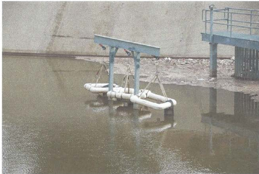
Photo 4: Raised skimmers at Terminal Basin
