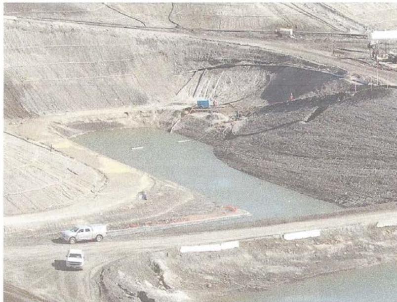
Figure 16: Pumping water out of the moat around Cell CC4 Phase 3
