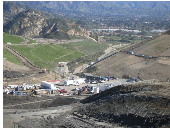
Photo 116: Posi-Shell and Closure Turf: January 22, 2019
