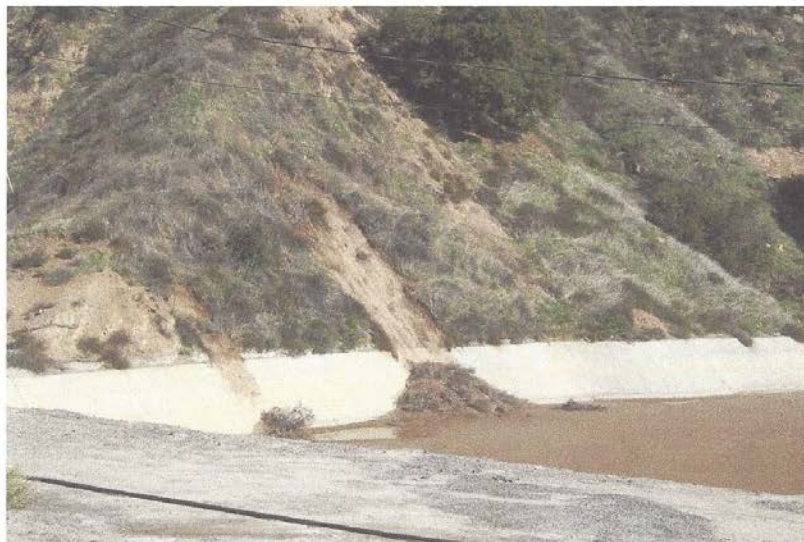
Photo 12: Sloughing on side of Basin B with sediments
