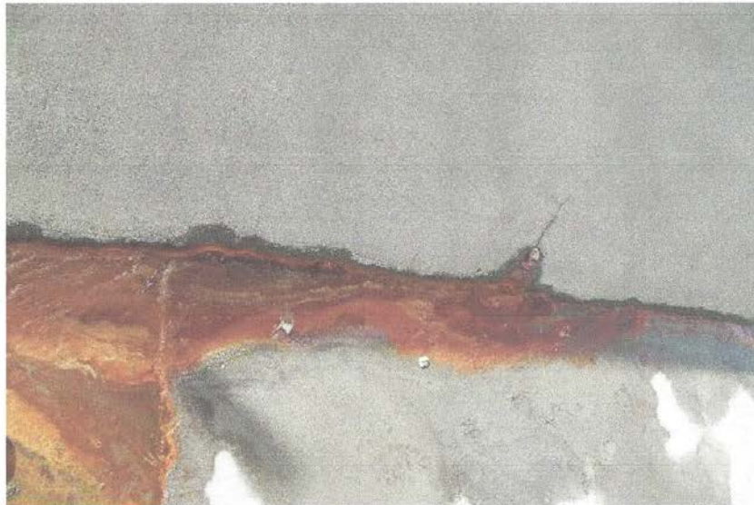
Photo 6: Reddish deposit from water seeping through weep holes at the bottom of the wall
