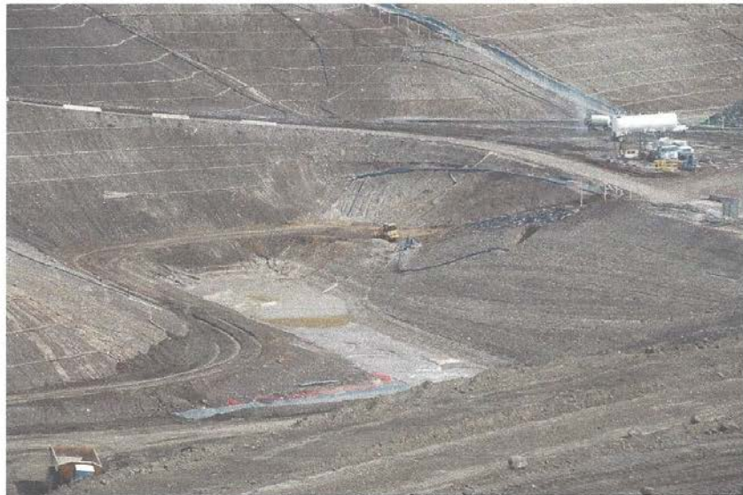
Photo 14: Sediment accumulation in moat around Cell CC4 Phase 3
