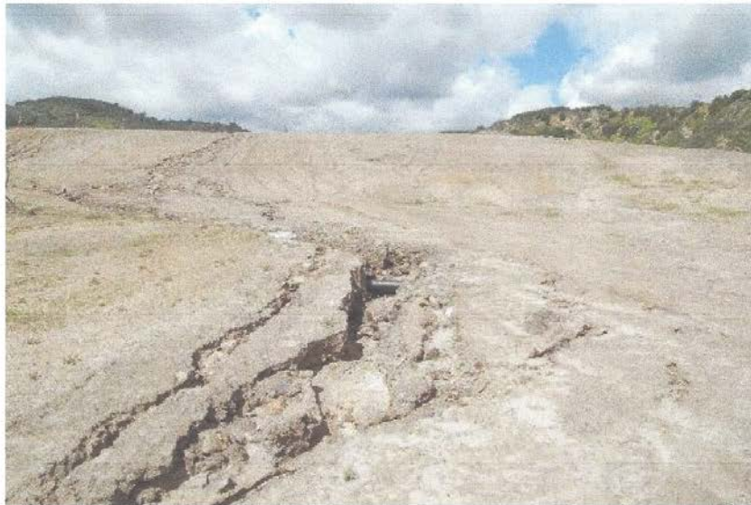
Figure 20: Deep erosion gullies on interim cover – County landfill deck
