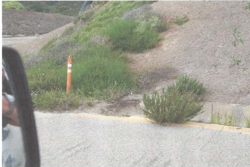
Photo 11: Sediments plugging drain at end of ditch along access road to Flares 9-11
