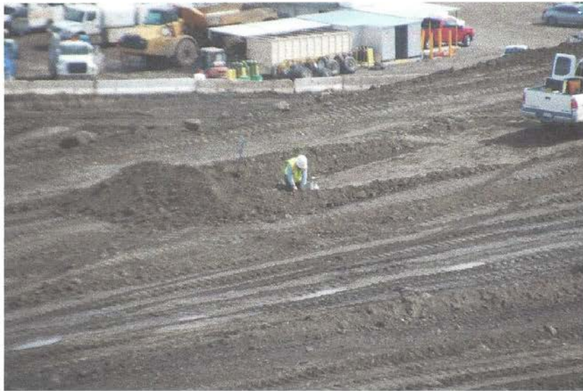
Figure 15: CQA monitoring of buttress
