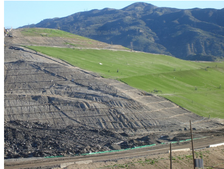
Photo 118: Posi-Shell and Closure Turf: January 22, 2019
