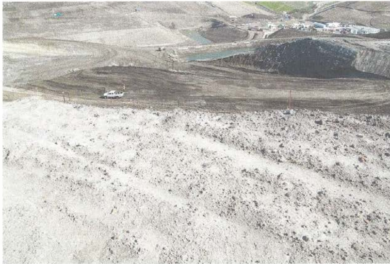
Figure 17: CQA monitoring of buttress – Note stakes for new movement monitoring prisms
