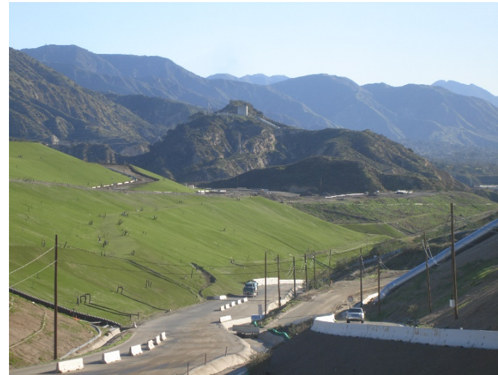
Photo 120: Posi-Shell and Closure Turf: January 22, 2019
