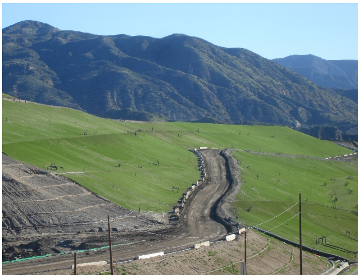
Photo 119: Posi-Shell and Closure Turf: January 22, 2019
