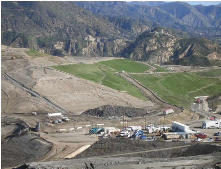
Photo 115: Posi-Shell and Closure Turf: January 22, 2019
