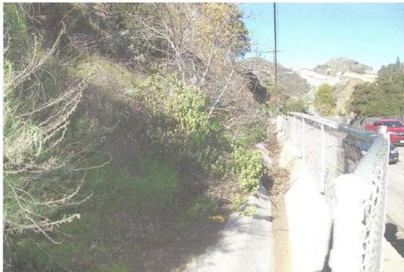
Figure 20: Sediments in drainage swale at wall along San Fernando road
