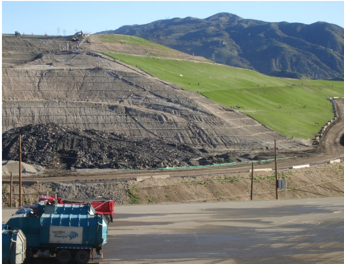
Photo 117: Posi-Shell and Closure Turf: January 22, 2019
