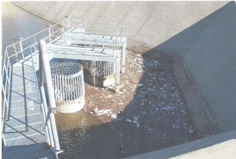
Photo 5: Waste collected behind decant towers at Terminal basin
