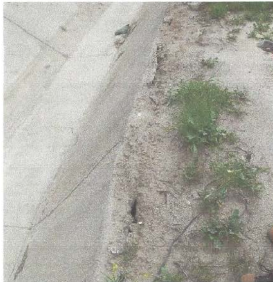
Phot 15: erosion along the edge of concrete channel between power pole and access road to Flares 9-11
