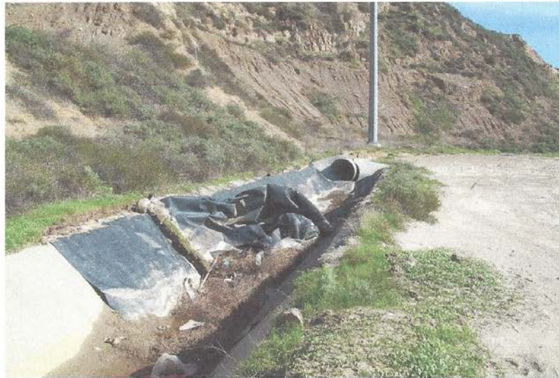
Photo 15: Damage to membrane and culvert on second segment of channel west of the access road to Flares 9-11
