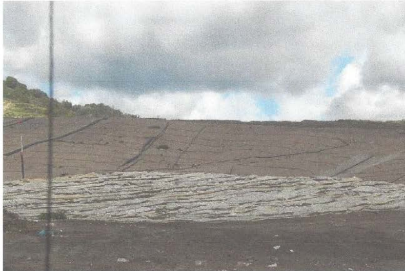
Photo 1: Use of ADC at the waste face in Cell CC4
