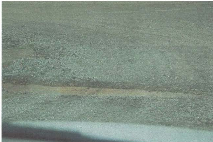
Photo 12: Erosion gully at edge of access road to Flares 9-11
