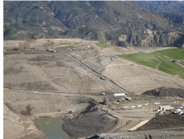
Photo 114: Posi-Shell and Closure Turf: January 22, 2019
