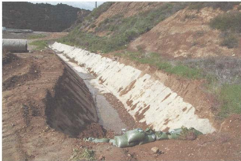
Photo 12: Culvert removed on second segment of channel west of the access road to Flares 9-11
