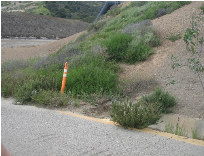
Photo 183: County Flare Road Plugged Drainage: March 28, 2019
