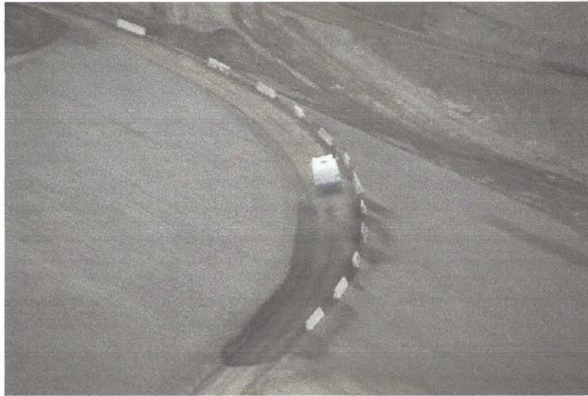
Figure 19: Moisture conditioning on roads
