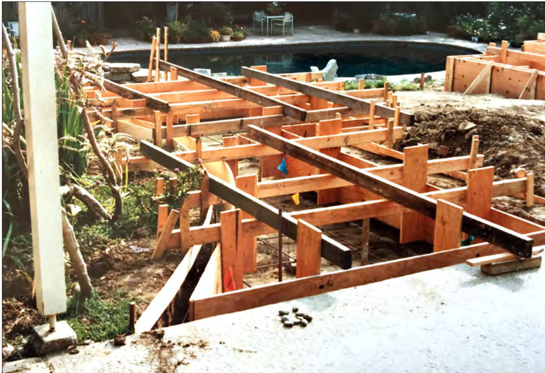
Image 31: Garden, coy pond construction (Ray Borun, 1985)
