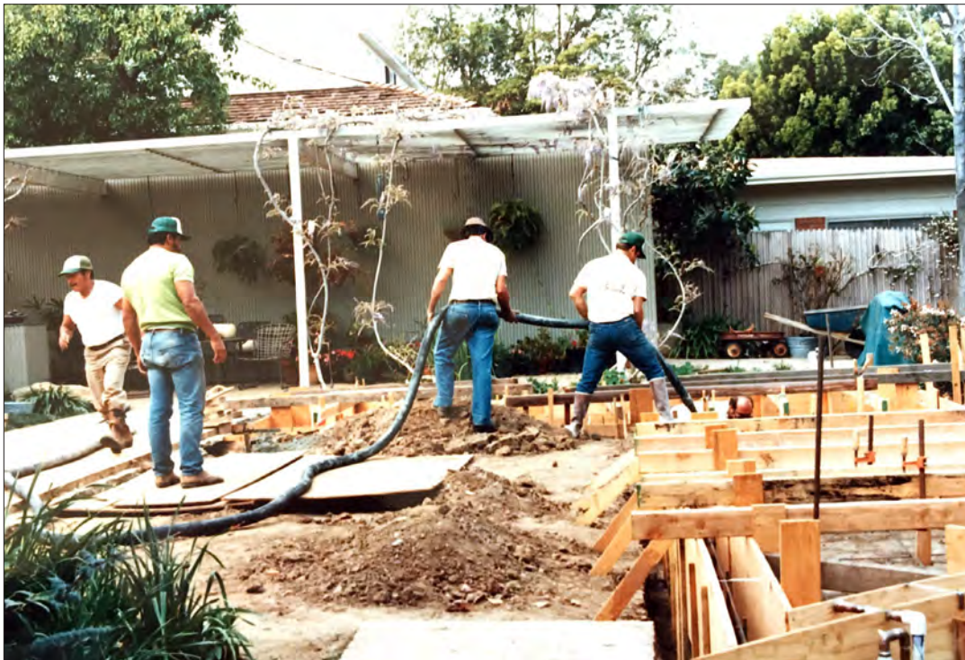
Image 32: Garden, coy pond construction (Ray Borun, 1985)
