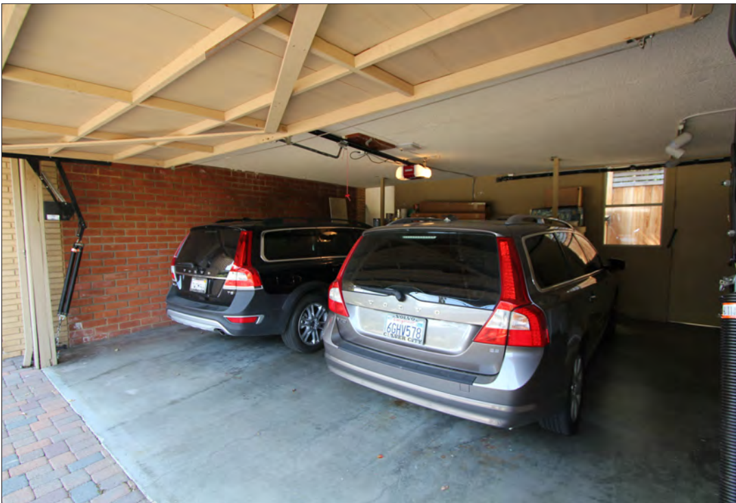
Image 54: Garage, view northwest (Chattel, 2019)
