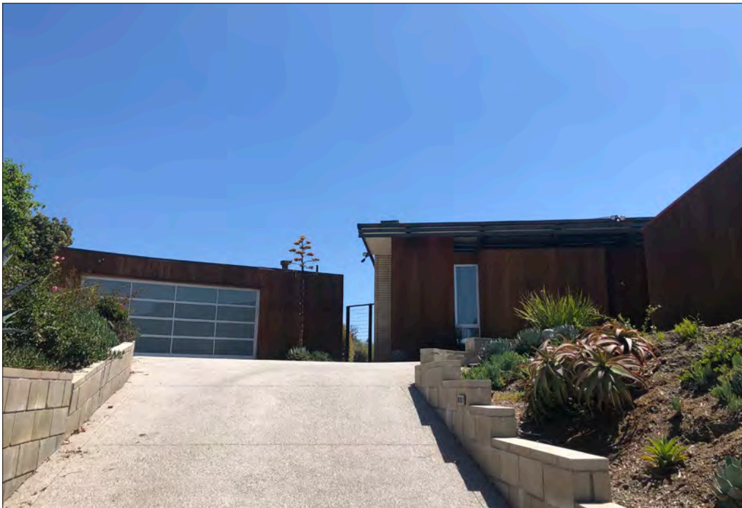
Image 8: Neiburger House (HCM #1122), 1220 North Kenter Avenue, Brentwood, 1962 (Chattel, 2019)
