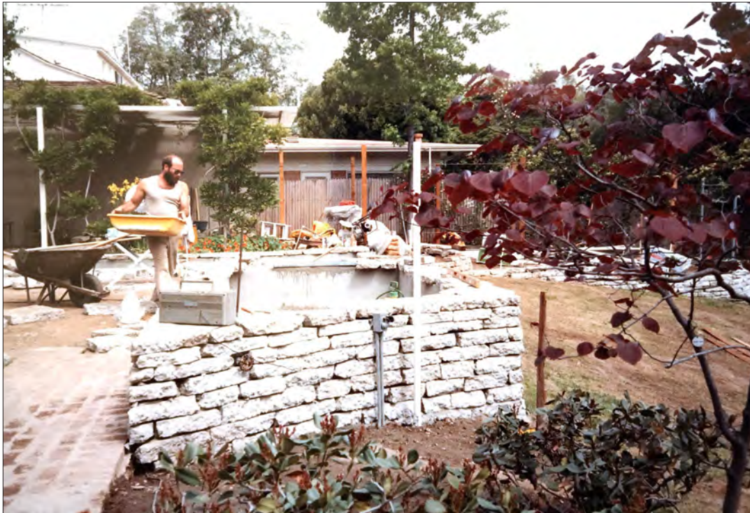
Image 39: Garden, coy pond construction (Ray Borun, 1985)
