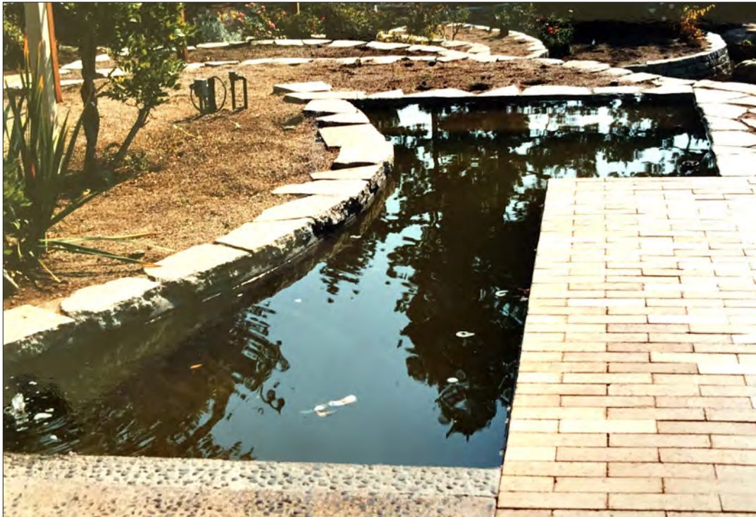
Image 47: Garden, coy pond construction (Ray Borun, 1985)
