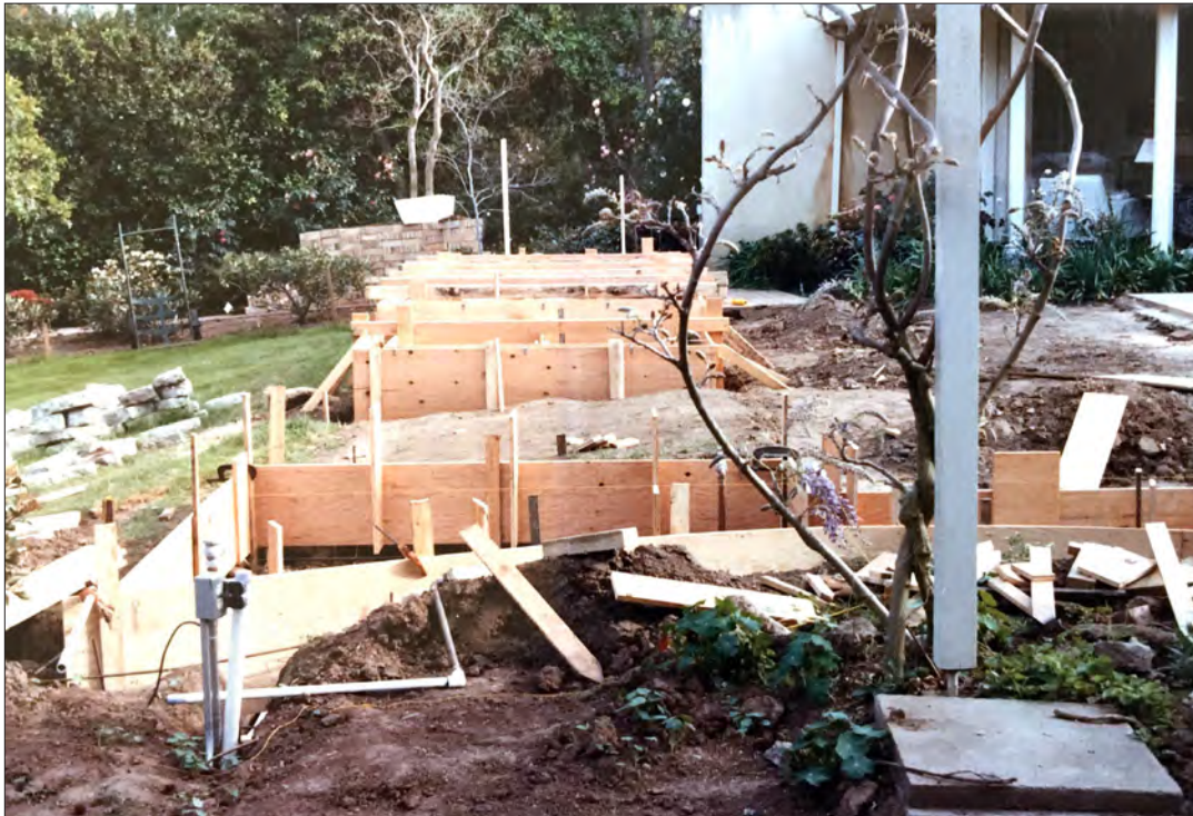
Image 29: Garden, coy pond construction (Ray Borun, 1985)
