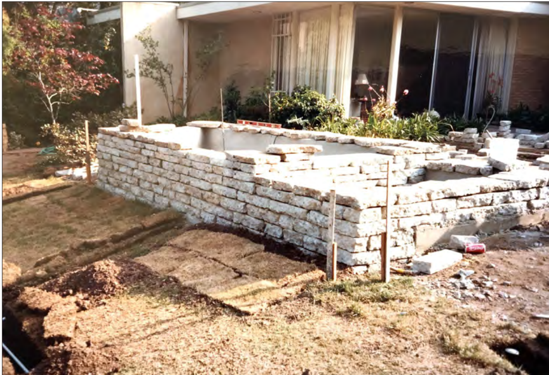
Image 49: Garden, coy pond construction (Ray Borun, 1985)
