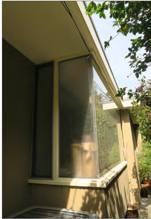
Image 15: South elevation, view east (Chattel, 2019)
