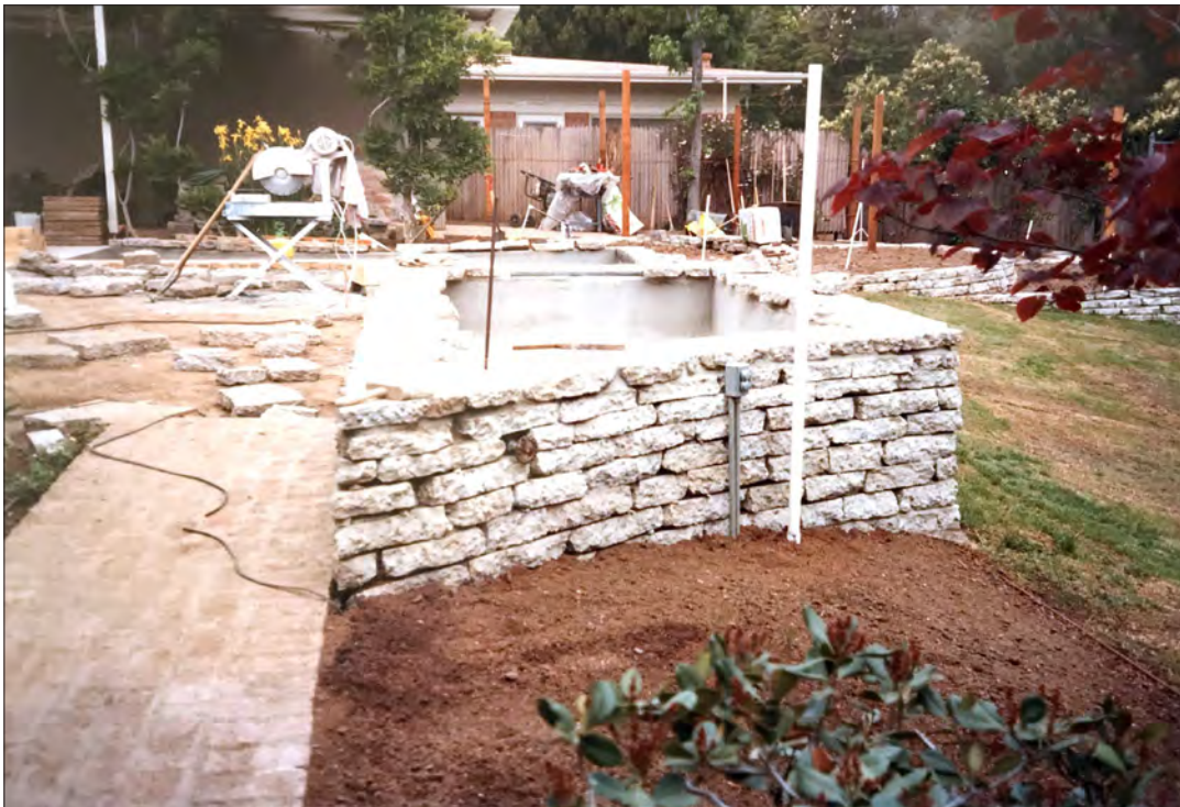
Image 46: Garden, coy pond construction (Ray Borun, 1985)
