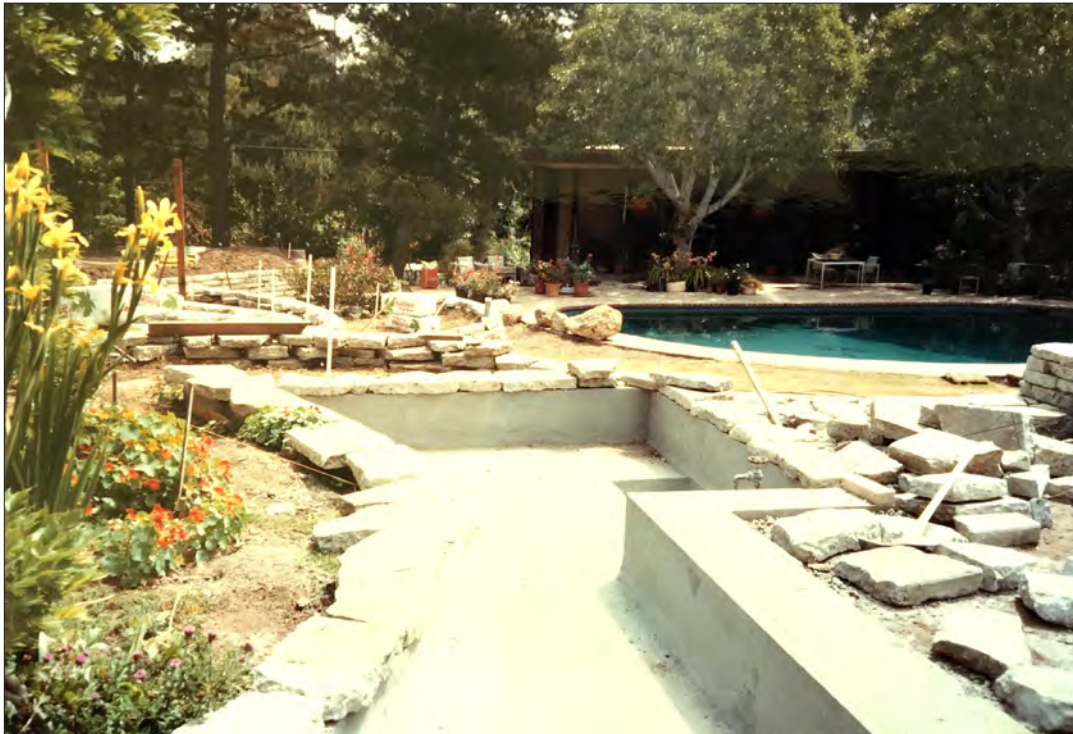
Image 33: Garden, coy pond construction (Ray Borun, 1985)
