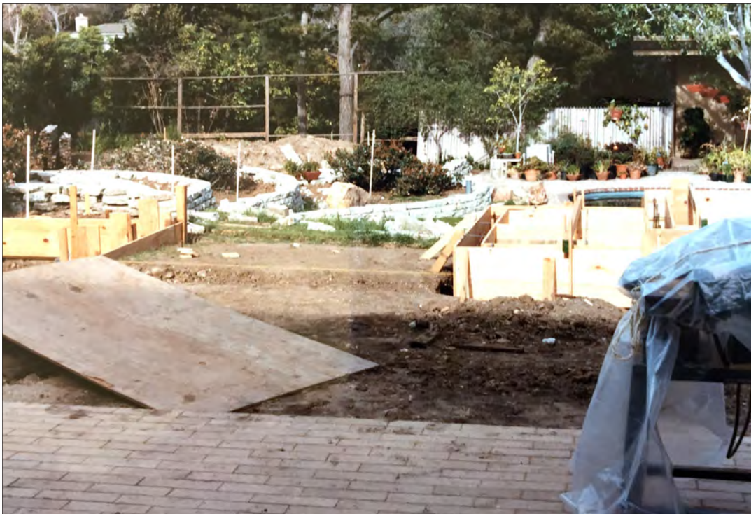
Image 38: Garden, coy pond construction (Ray Borun, 1985)
