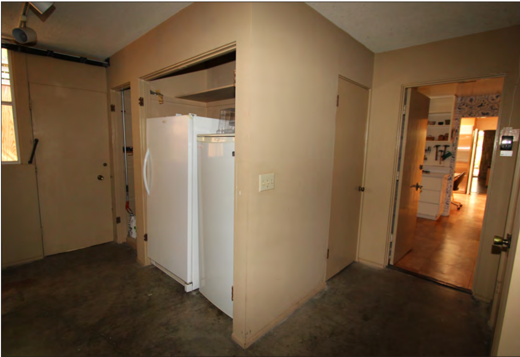
Image 53: Space adjacent to garage, view northwest (Chattel, 2019)
