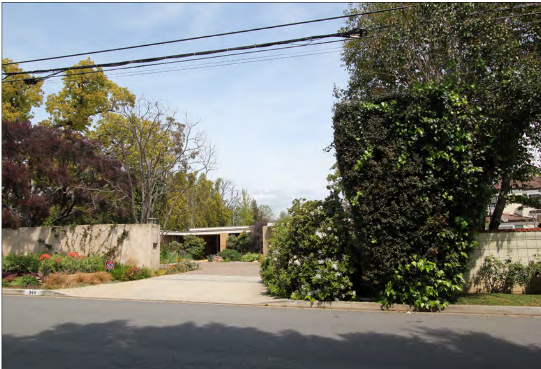
Image 4: Borun House and driveway, view east (Chattel, 2019)
