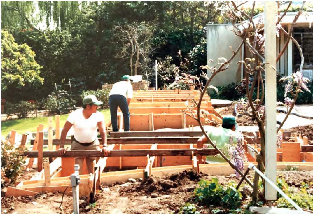
Image 37: Garden, coy pond construction (Ray Borun, 1985)
