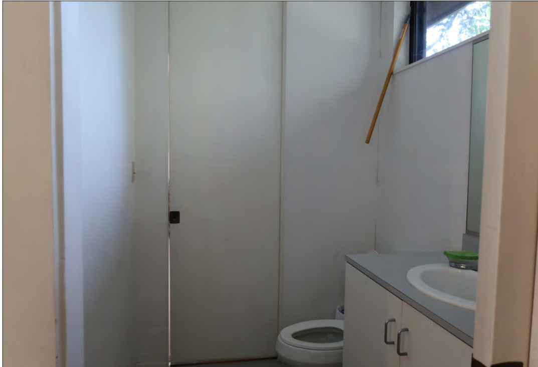
Image 69: Bathroom in office building, view north (Chattel, 2019)
