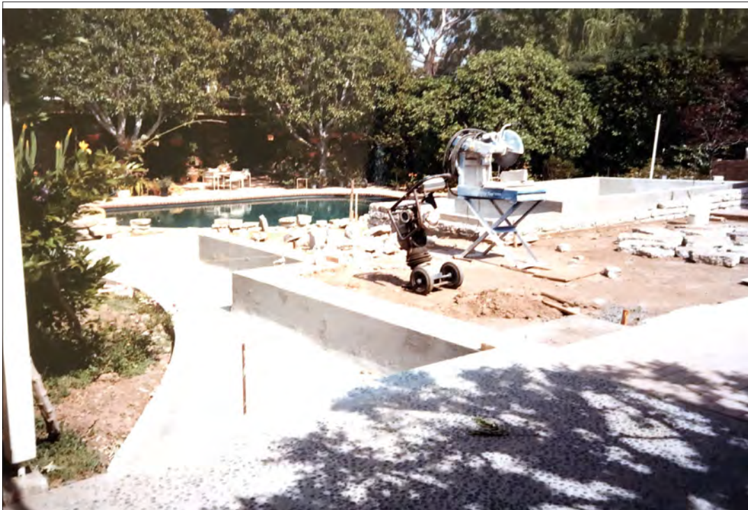
Image 30: Garden, coy pond construction (Ray Borun, 1985)
