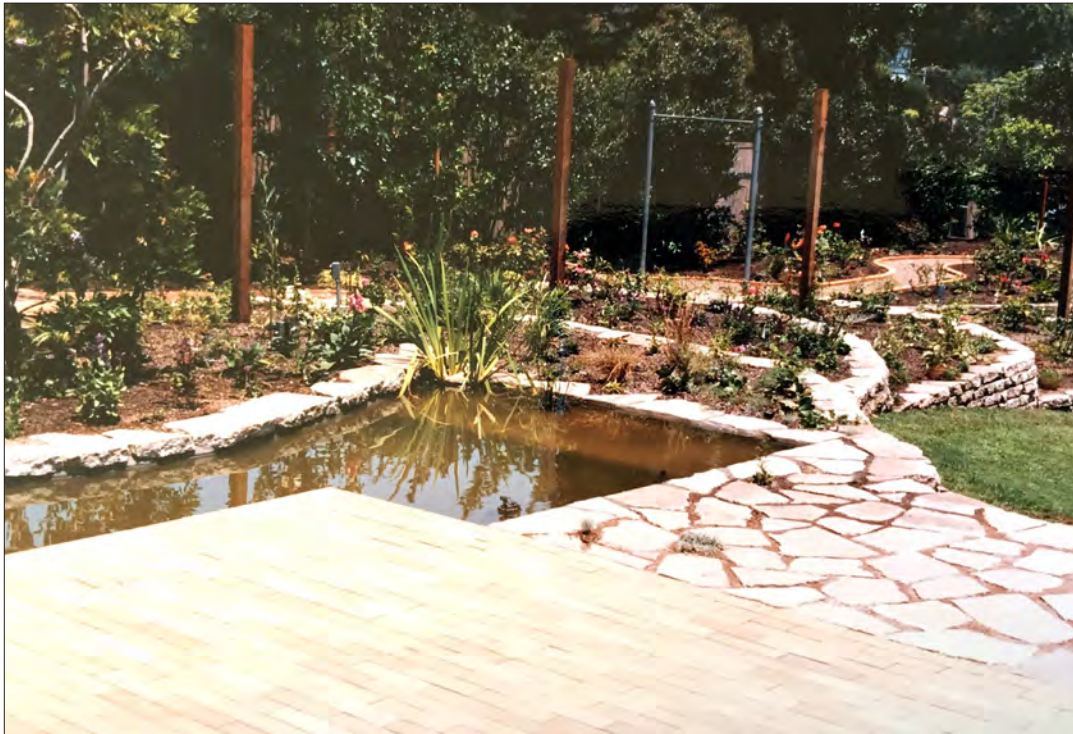
Image 35: Garden, coy pond construction (Ray Borun, 1985)
