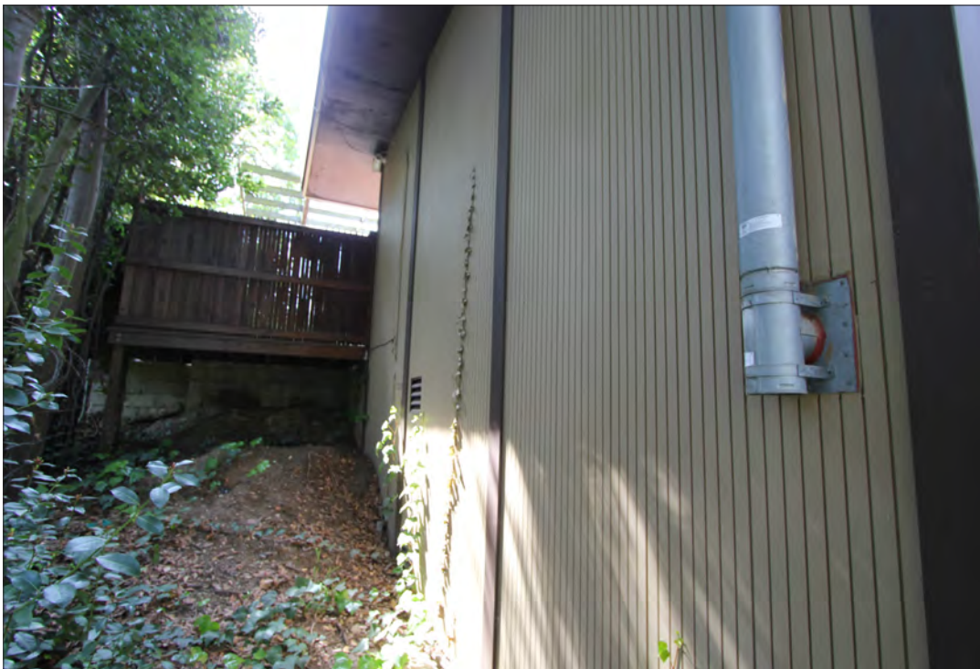
Image 64: Garden and pathway, view north (Chattel, 2019)
