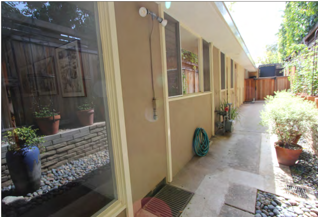
Image 24: North elevation, view west (Chattel, 2019)
