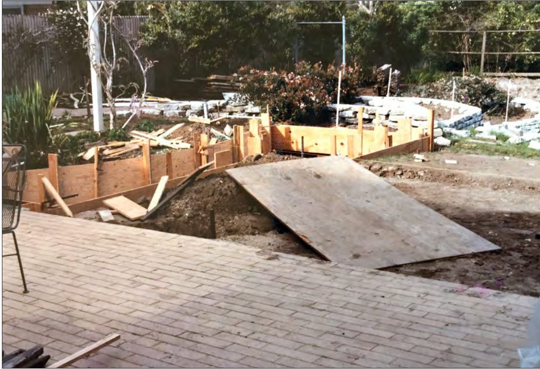
Image 28: Garden, coy pond construction (Ray Borun, 1985)
