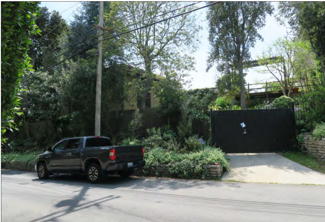
Image 66: Accessory Building, east (left) and north (right) elevations, view west (Chattel, 2019)
