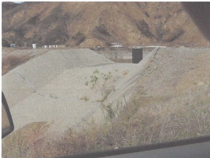
Photo 8: Vegetation and concrete crack in spillway of Basin D
