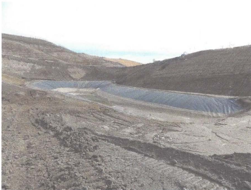
Photo 10: Temporary lined basin at Cell CC4 – Phase 3
