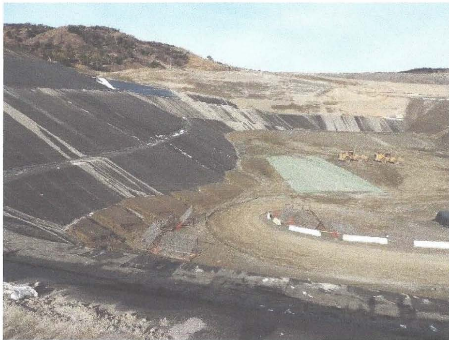
Photo 13: Damage to operation layers on slope of Cell 4 Phase 3
