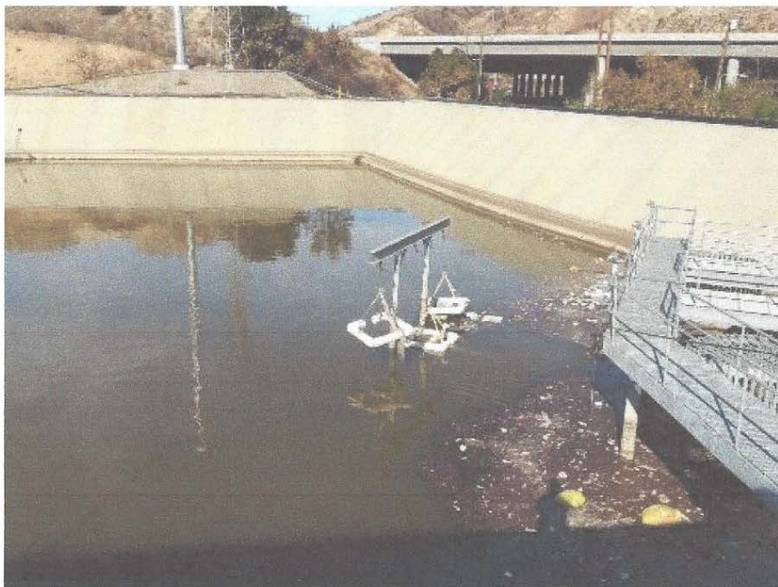
Photo 4: Skimmer at Terminal basin – one skimmer was on
