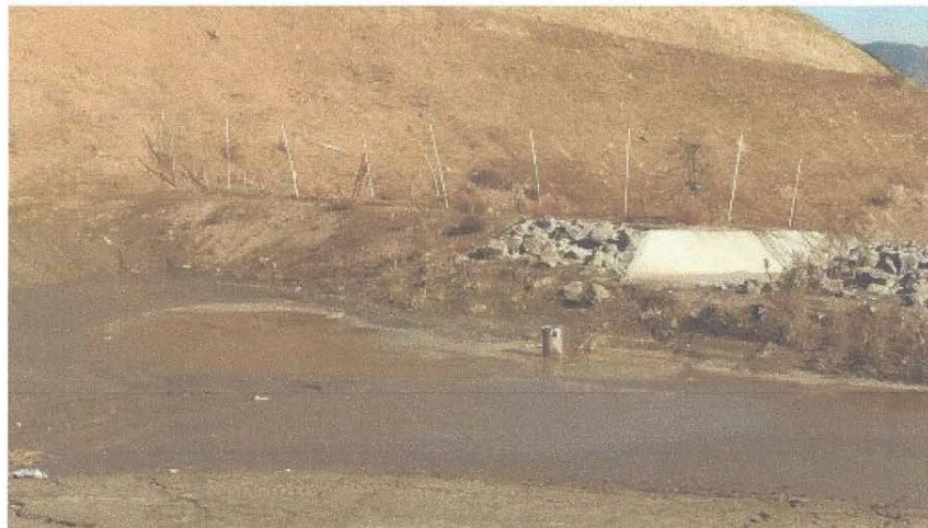
Photo 6: Trash Gard on outlet of Cell CC3 earthen basin
