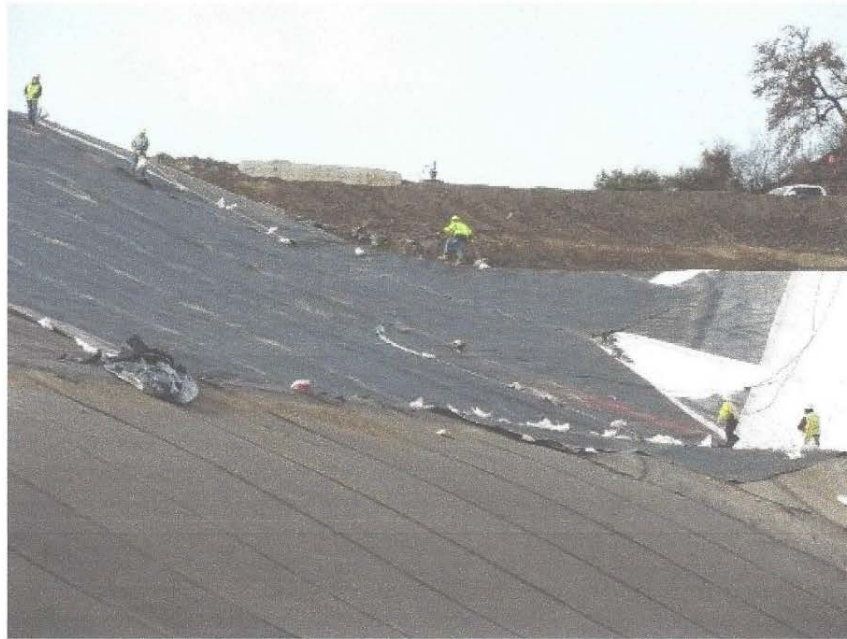
Photo 11: Deployment of geosynthetics on slope at Cell CC4 – Phase 3
