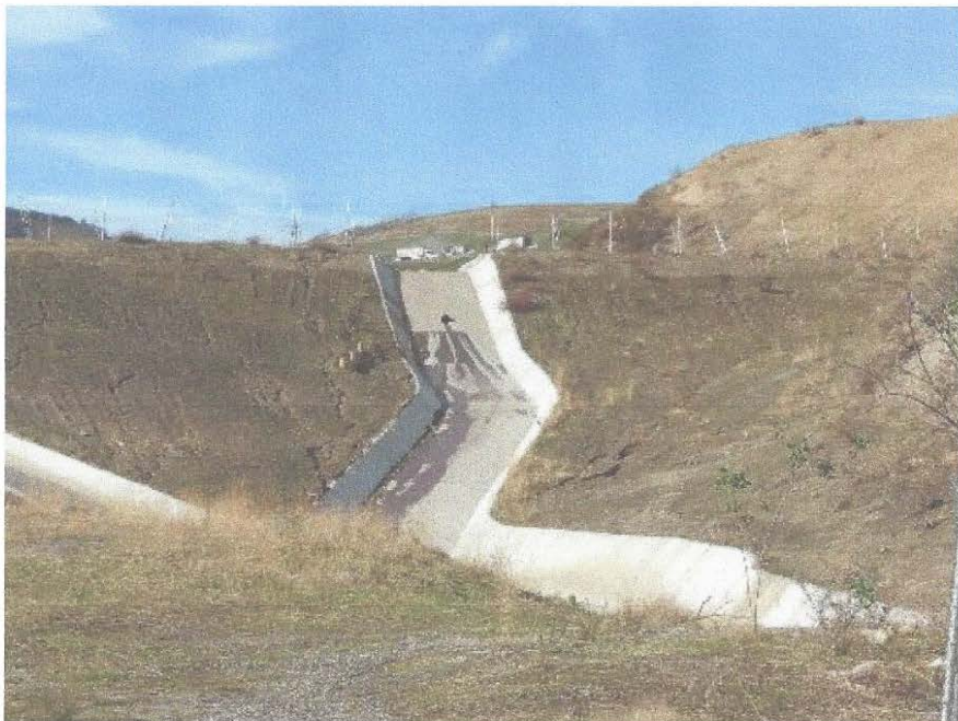
Photo 14: erosion gullies on downstream slope of Cell CC3 earthen basin
