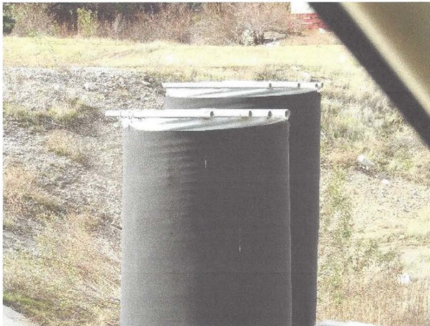
Photo 9: Decant towers at Basin D Equipped with safety bars
