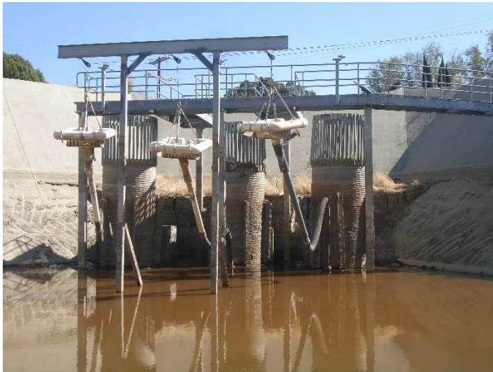
Photo 241: Terminal Basin Outlet Risers: October 29, 2019
