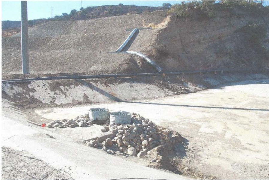
Photo 7: Sediments against rock around the decant towers at Basin A
